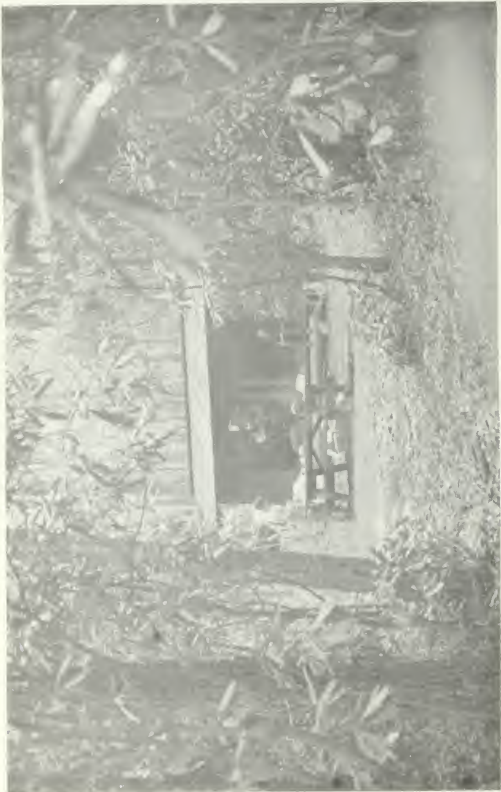
Three-sided shelters are found at 7- to 8-mile intervals along much of the Appalachian Trail. (Photo courtesy of Zellie G. Earnest.)
