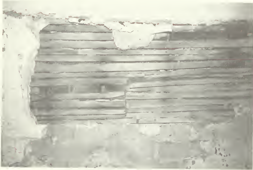
Illustration 40. Antram-Gray House: Type-III Lath and Plaster, Circa 1798, on West Wall of Room 202.
