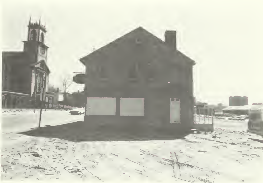
Illustration 69. Antram-Gray House: North Facade.
