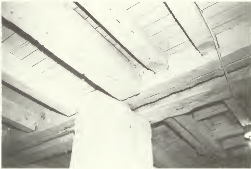
Illustration 36. Antram-Gray House: First-Floor Framing, Showing Adjacent Circa-1730 and Circa-1798 Sills.
