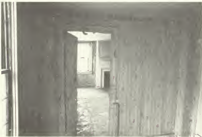
Illustration 66. Antram-Gray House: Room 205, Looking South.
