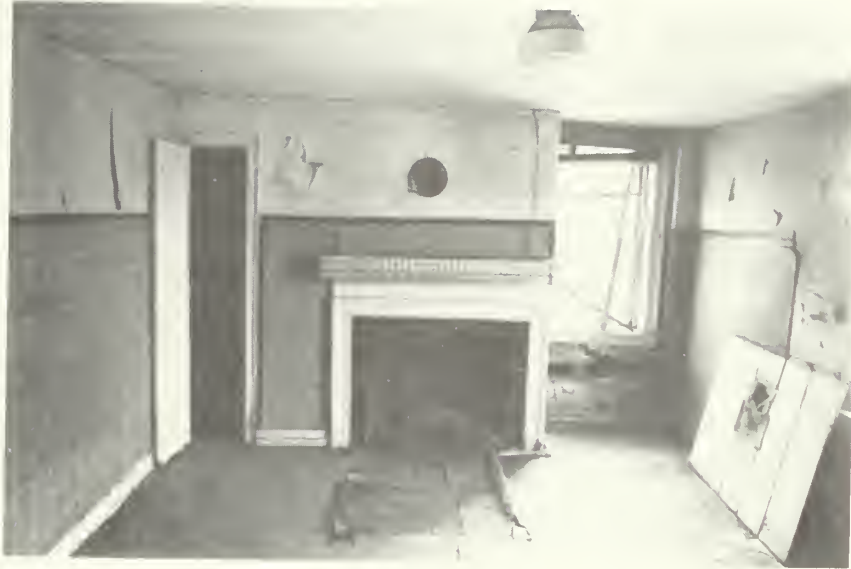
Illustration 63. Antram-Gray House: Room 202, Looking South.
