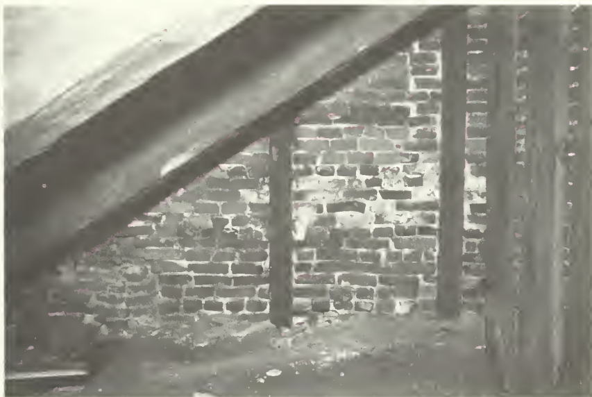
Illustration 37. Antram-Gray House: South Wall of Attic, East End, Showing Studs Embedded in Brickwork.
