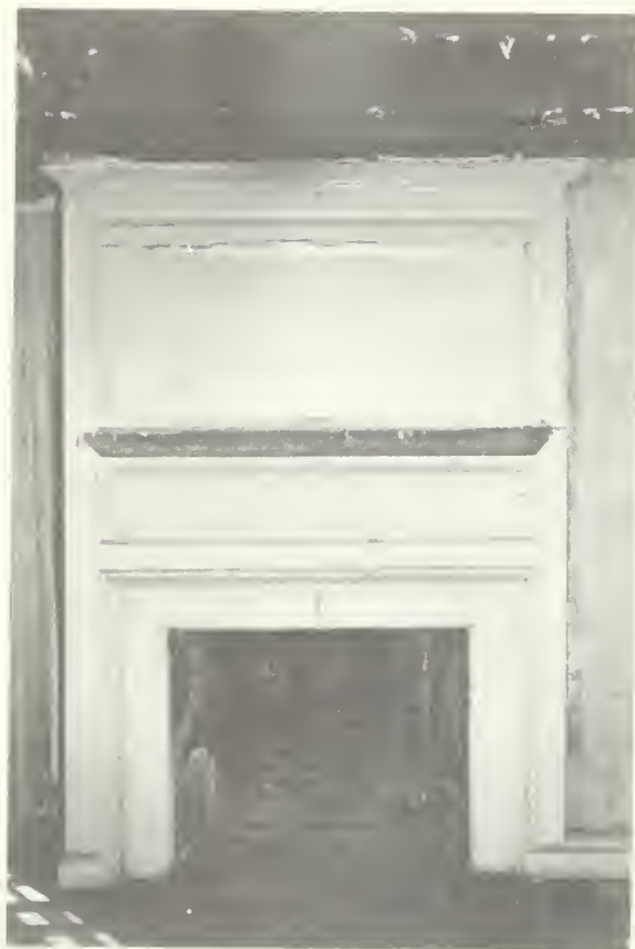
Illustration 42. Antram-Gray House: Fireplace in Room 201.
