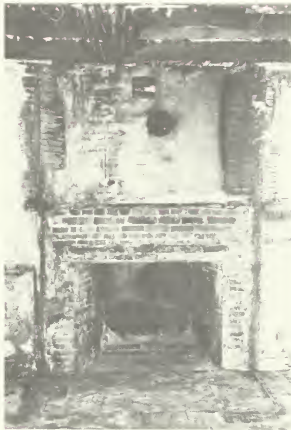
Illustration 53. Antram-Gray House: Fireplace in Room 204, Showing Circa-1798 Recessed Overmantel and Circa-1820 Firebox.
