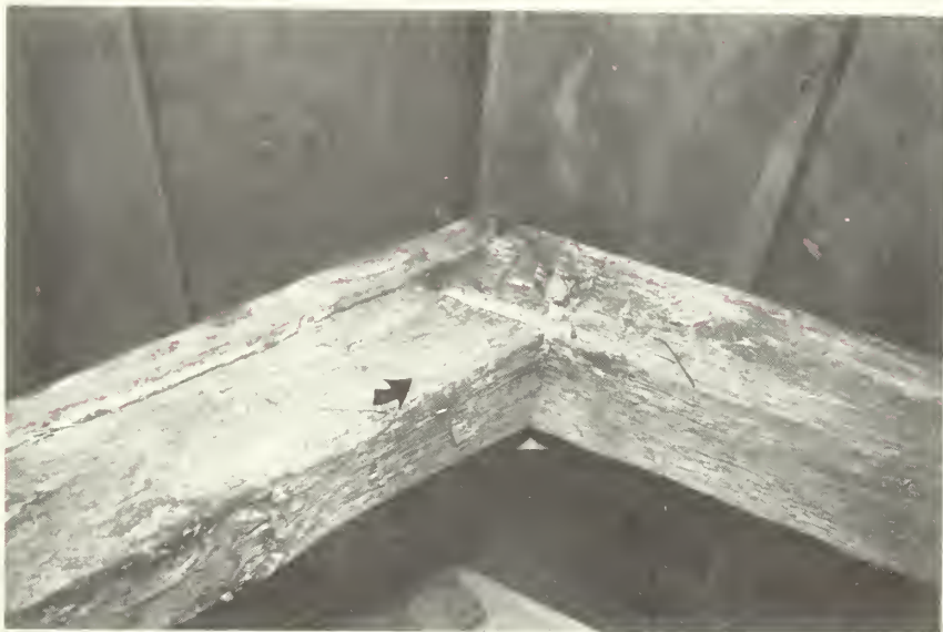
Illustration 25. Antram-Gray House: Raising Numerals on Roof Rafters.
