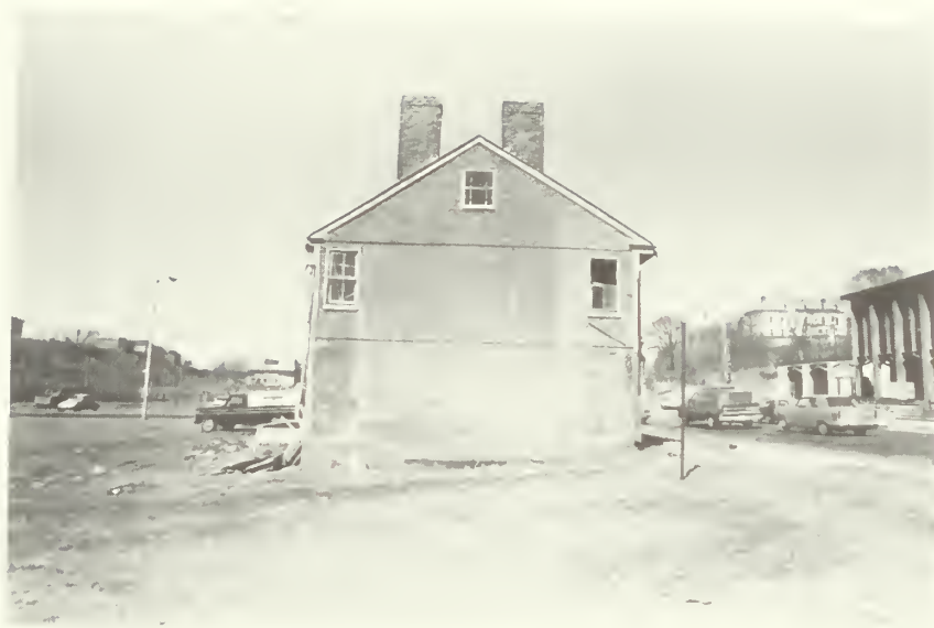
Illustration 70. Antram-Gray House: South Facade.
