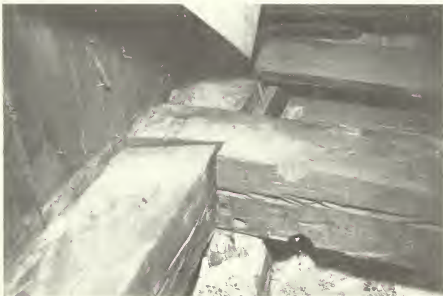
Illustration 19. Antram-Gray House: Dovetail Joints of Wall Plates in Northeast Corner of Attic.
