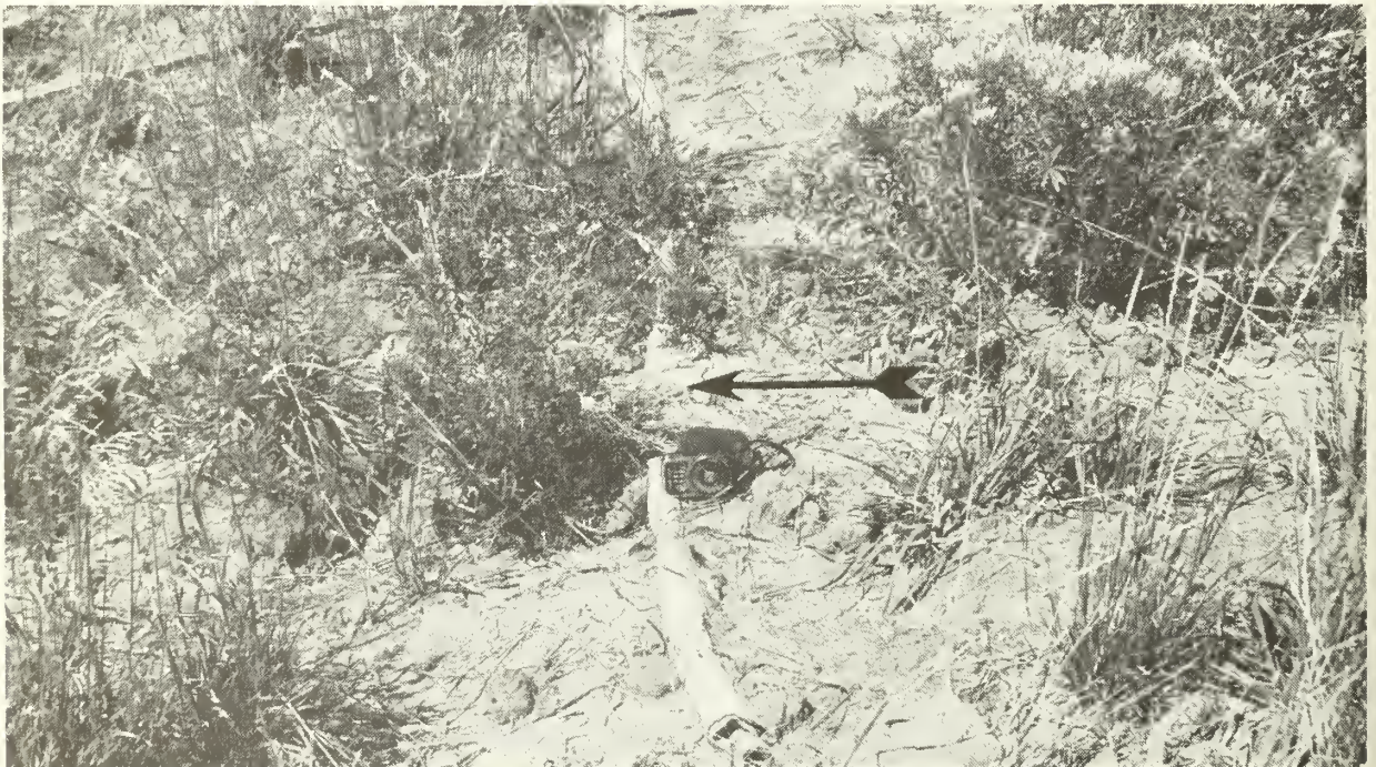
Figure 1.—Looking at a submerged burlap strip installed on waterway No. 6 on Alkali Creek watershed. Arrow indicates the direction of flow.
