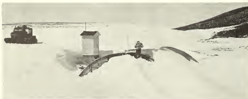
Figure 2.—The arch-covered weir under moderate winter conditions.
