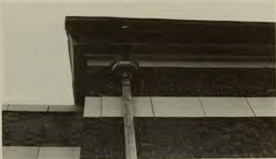
6. Lead-coated copper downspout, top.
