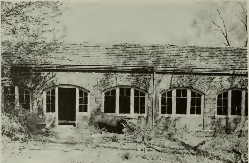
15. Missing sash, east elevation, C-8C.
