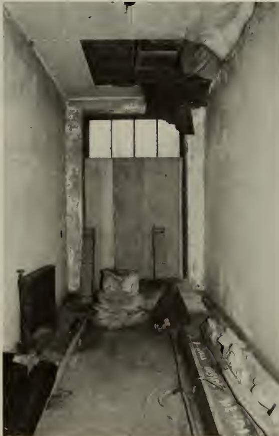
27. Water-damaged acoustical ceiling panels, H106.
