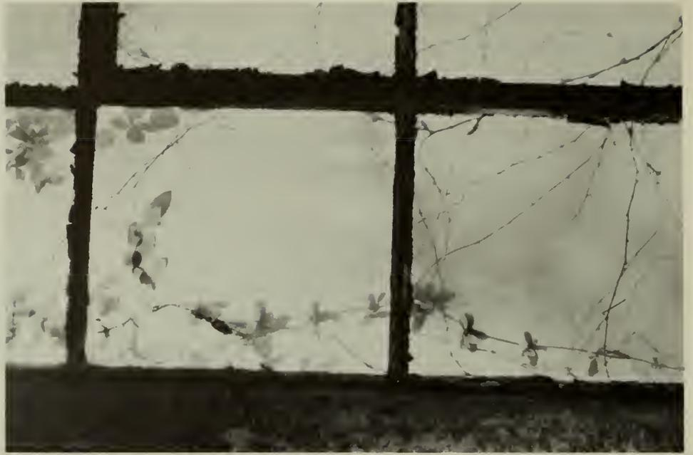
18. Corroded metal sash, C-9D.
