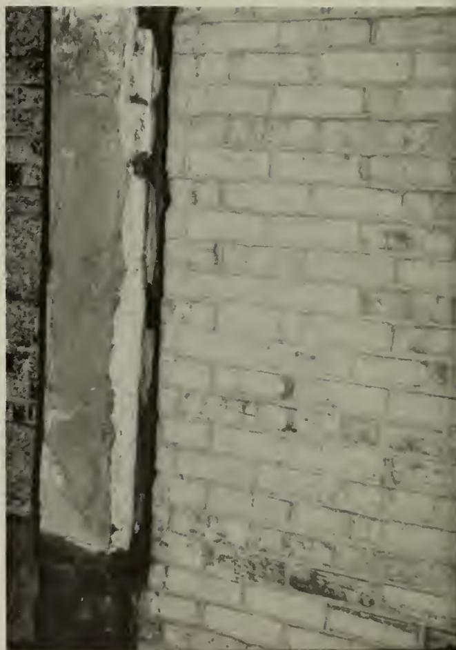
37. Gap at junction between walls of C-8C and C-9A.
