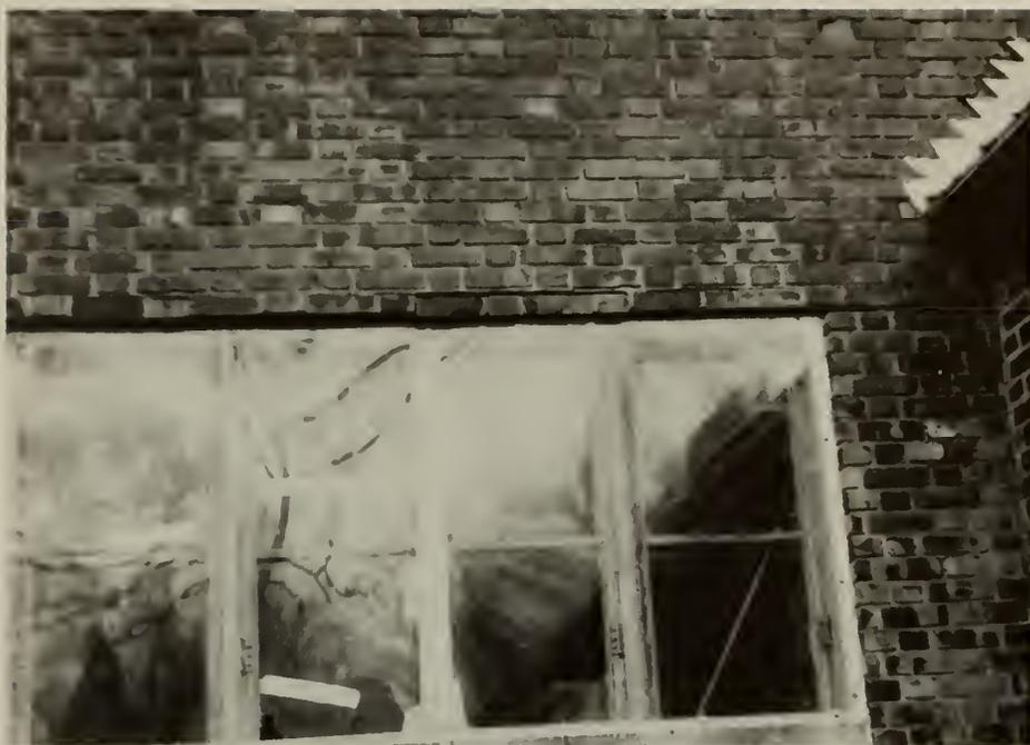
61. Horizontal cracks above lintel, north facade, west link.
