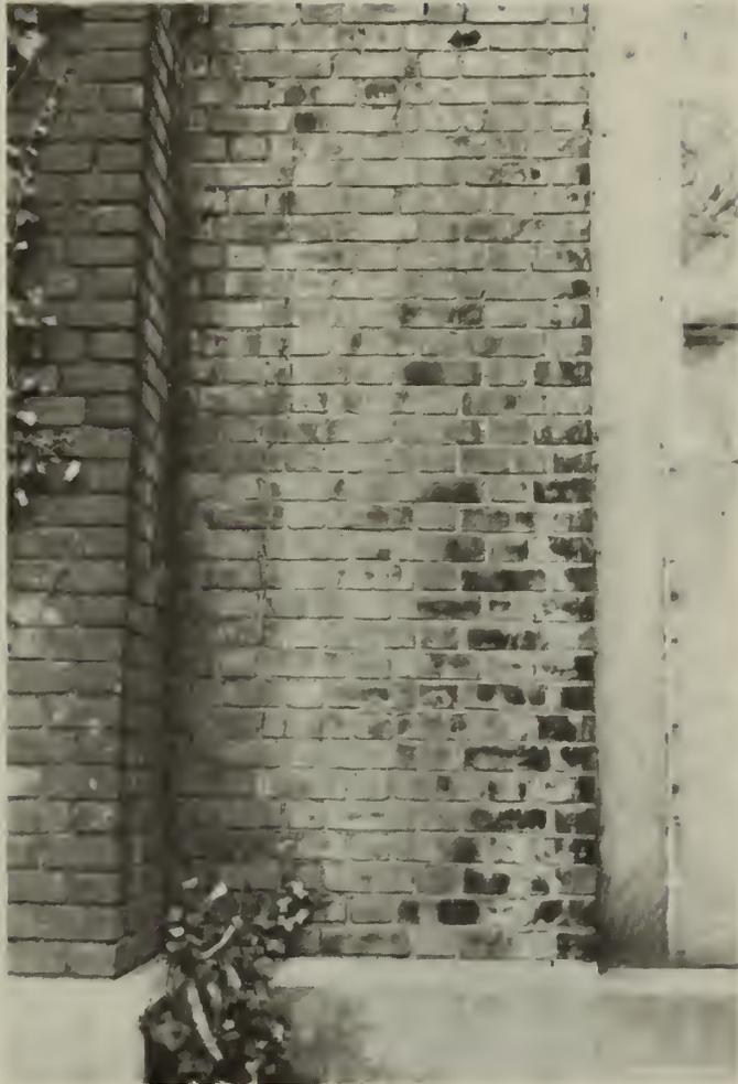
25. Efflorescence, east facade.
