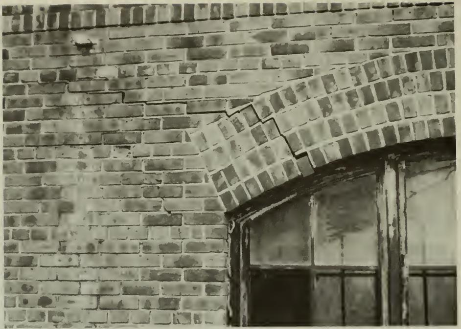
25. Cracking at brick joints, C-7B.
