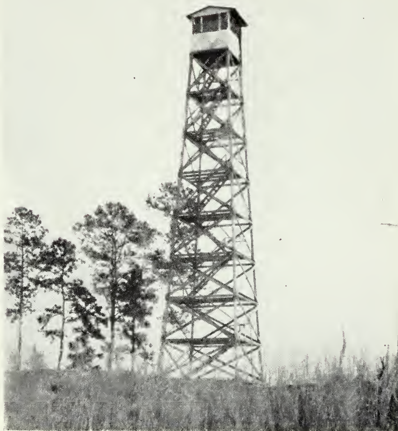
Forest fire lookout tower, built of cypress, on Pine Island Timber Protective Organization, near Albany, Ga.
