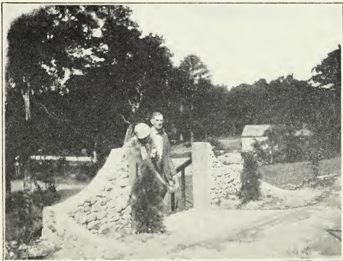
New entrance to the spring basin at Indian Springs Park.
