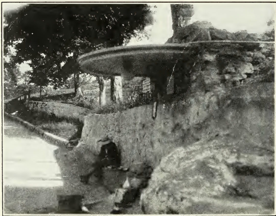
Spring, basin and new superstructure at Indian Springs Park.
