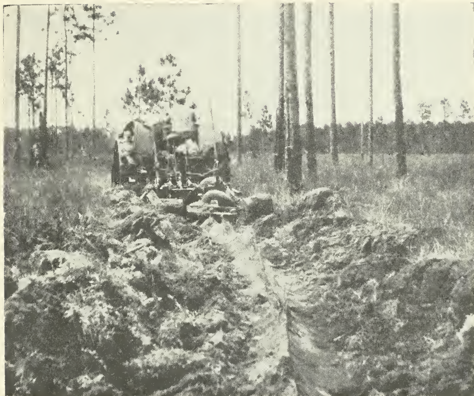
Constructing Firebreak on Timber Protective Organization Land.
