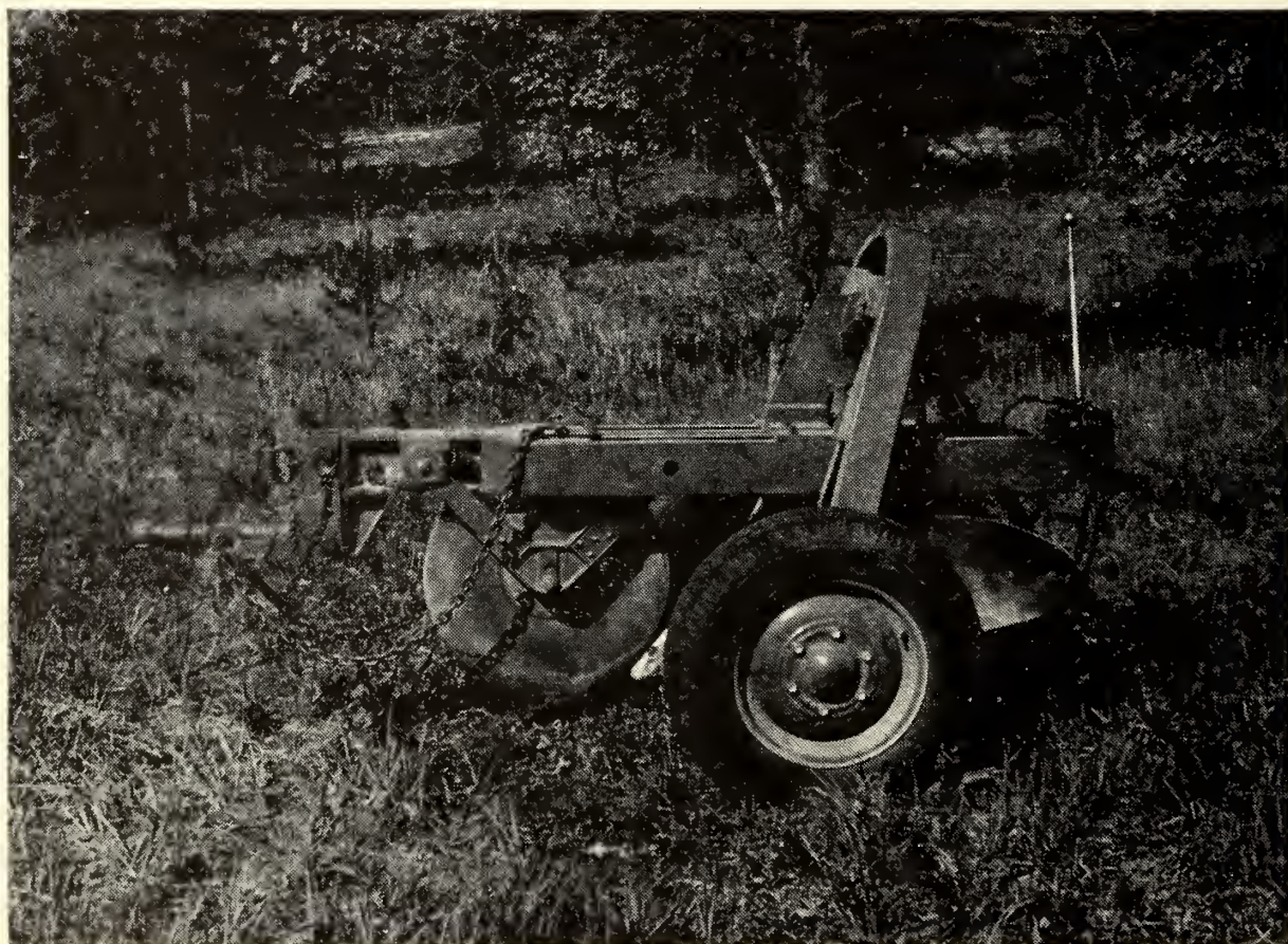
FIGURE 2.—Michigan hydraulic sulky plow in raised position.
