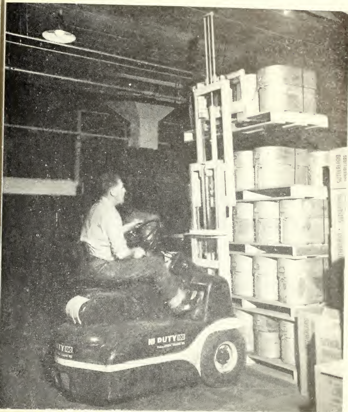
FIGURE 4.—Lift truck handling four 25-man mess outfits on a single pallet.
