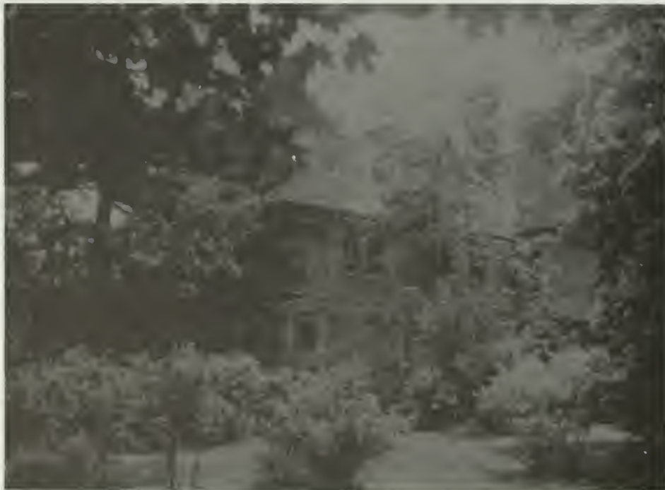
FIGURE 3.8: Northeast side of house, 1950. (SAHINHS, TRA Materials, Box 5, Folder 2, GAIC "F").
