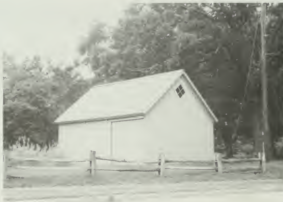
FIGURE 4.14: The north and east facades of the gardener's shed, 1993. (Photograph by author).
