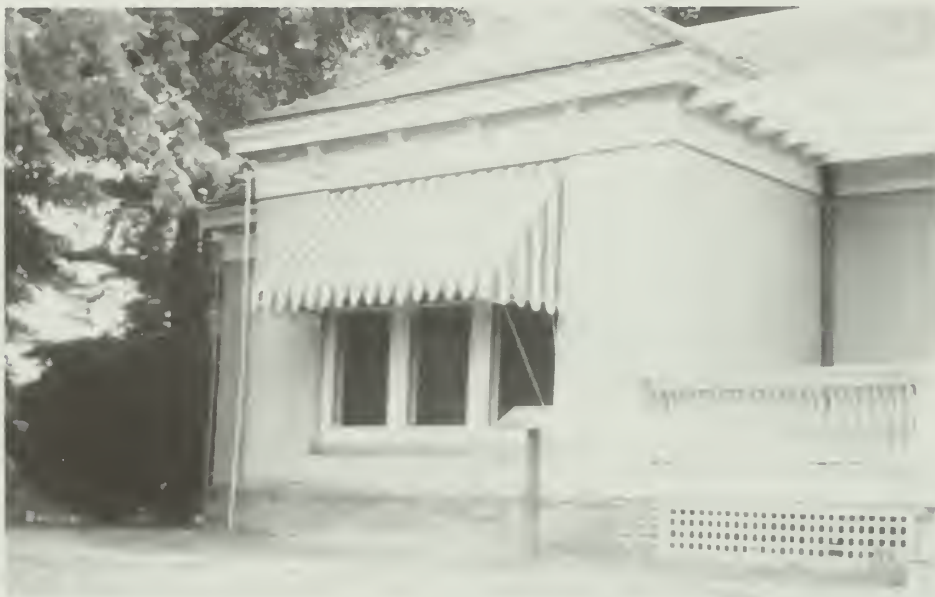
FIGURE 4.29: Poles near corners of North Room, 1993. (Photograph by author).
