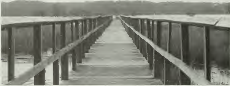
FIGURE 4.8: Bridge at Cold Spring Harbor Beach, 1993. (Photograph by author).
