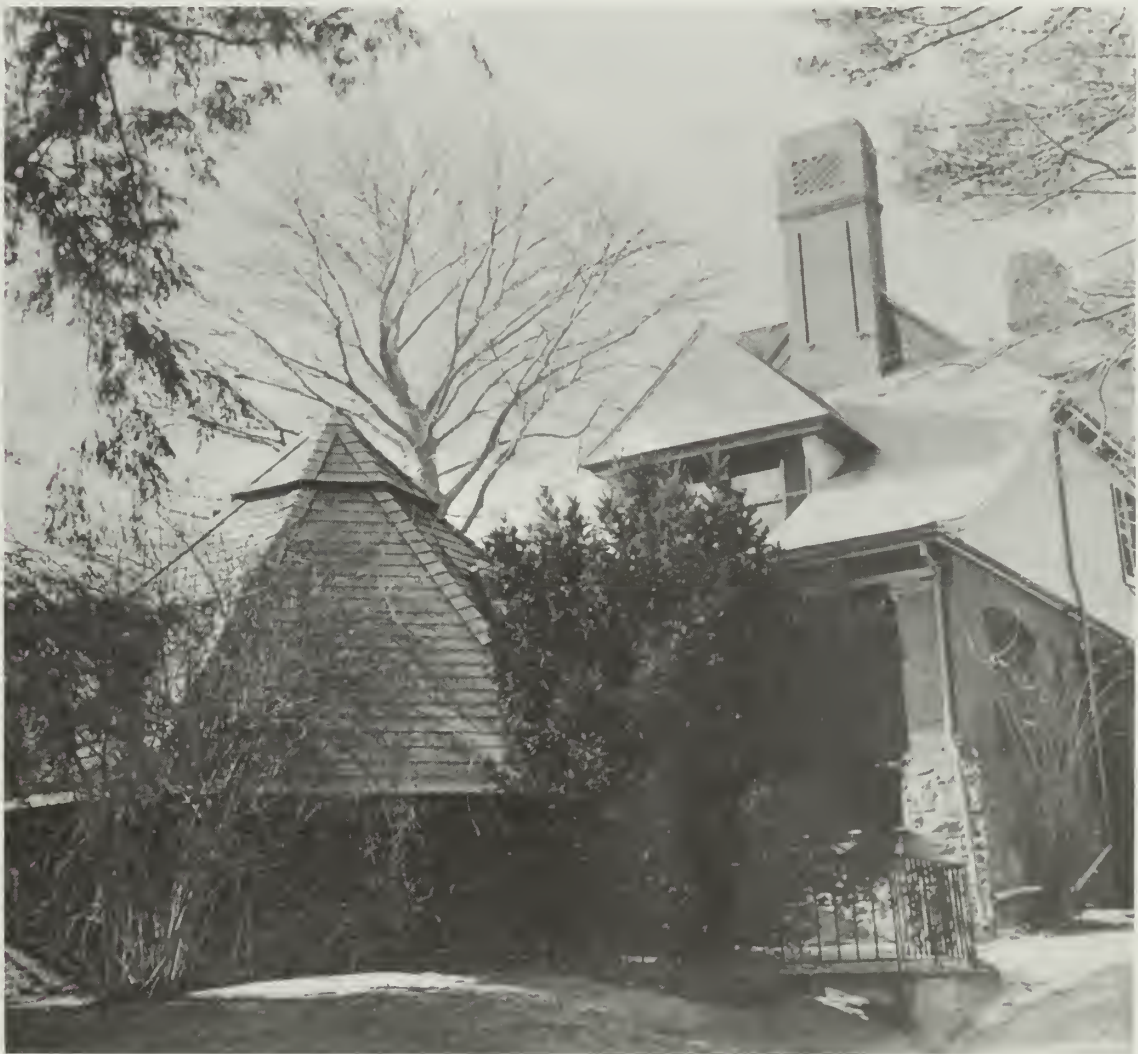
FIGURE 3.12: Wrought iron fence near restrooms, c. 1960. (SAHINHS).
