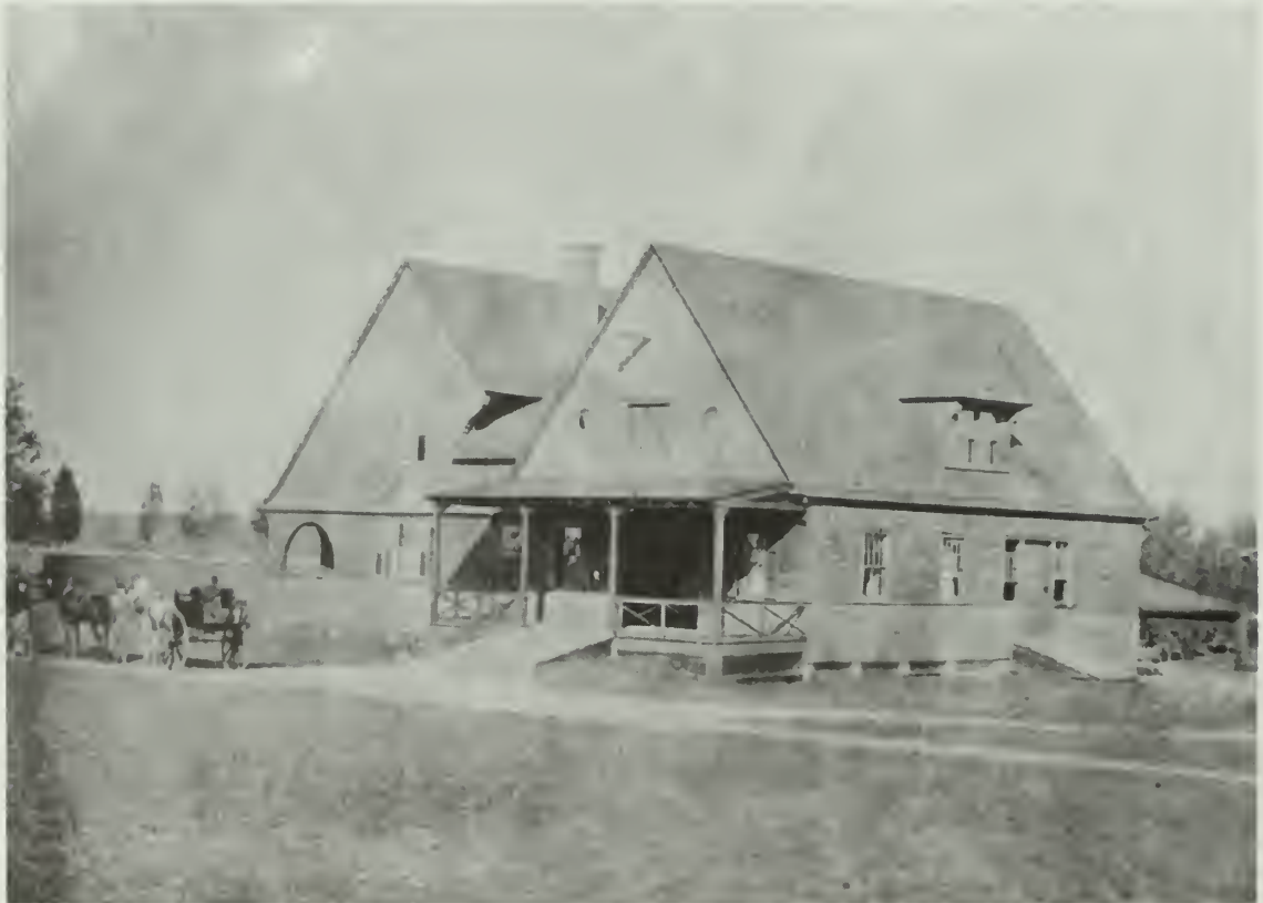
FIGURE 1.16: The west facade of the stable and lodge at Sagamore Hill, 1905. (SAHINHS, no. 1112, Box 6).
