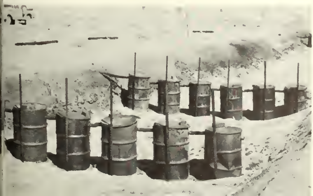
Figure 10.-- Metal drums used for catchment basins.
