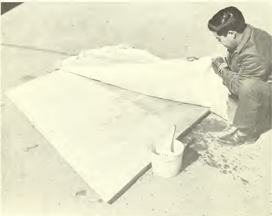
Figure 2.--Fiberglass coating being applied to the plywood.
