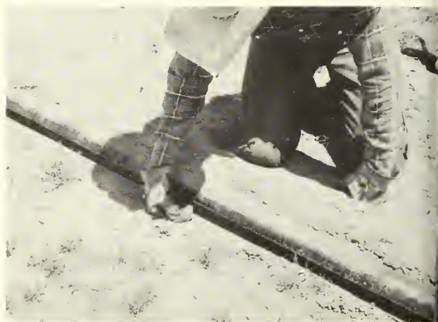
Figure 8.-- Making the collection trough flush with the soil surface.
