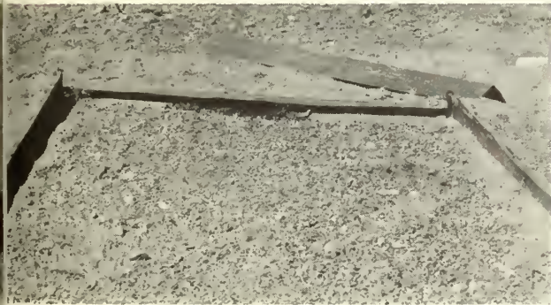
C, roofing valley;
