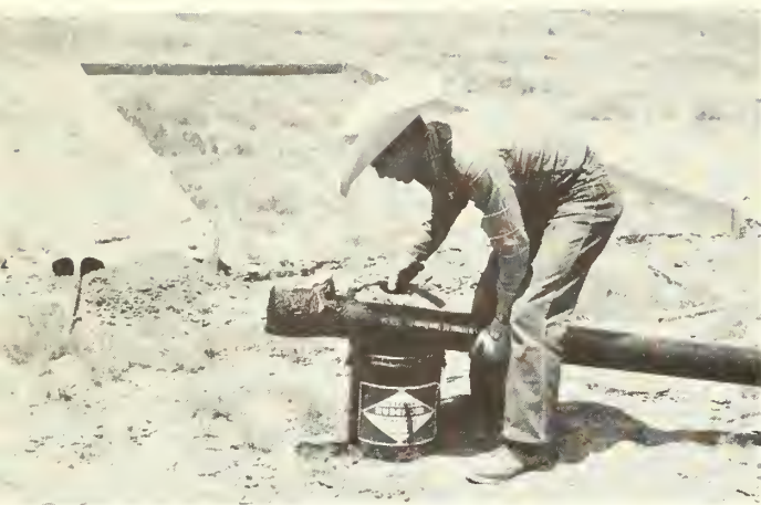
Figure 7.-- Sealing the hose connector to the collection trough.
