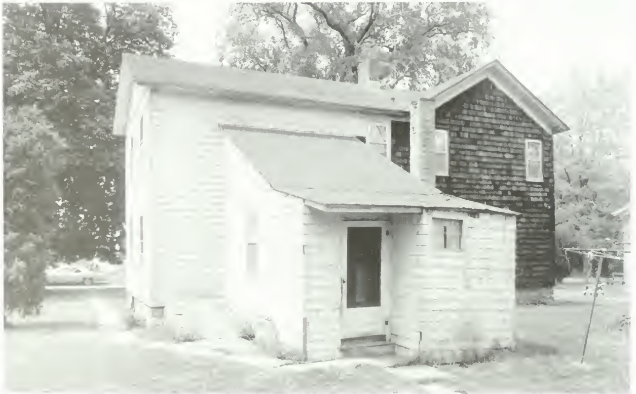
Figure 14. Stanton House: west and east elevations, July 19, 1968.
