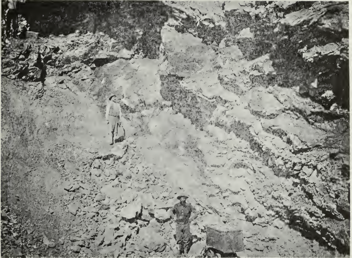
View of one of the working faces of the Keane Wonder Mine, showing the ease of mining. The ore at this point could be stripped directly off the face of the cliff, which saved the company thousands of dollars over the costs of tunneling, shafting, and timbering. From a booklet, "Bullfrog Mining District," published by the Rhyolite Chamber of Commerce, 1909.
