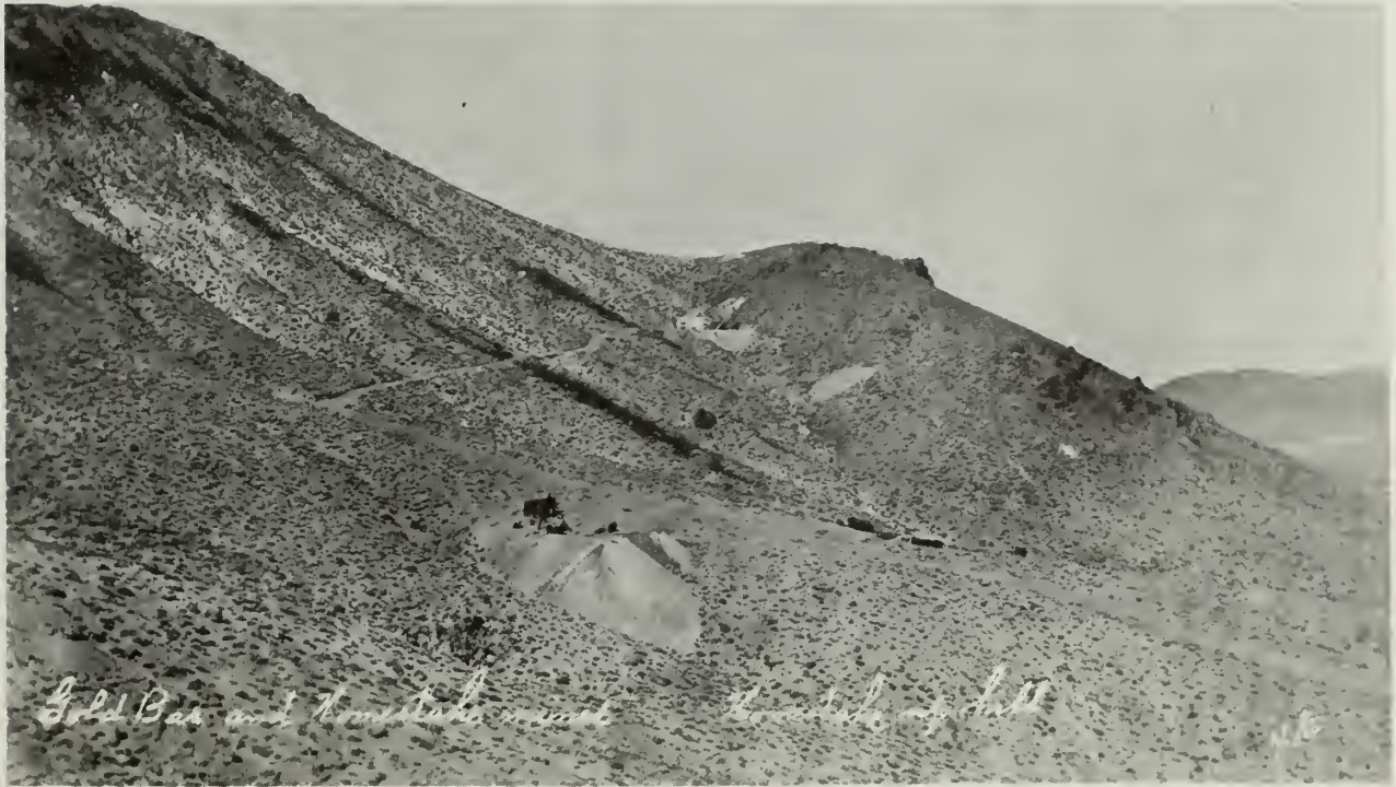
Another view of the Gold Bar-Homestake complex in late 1905, taken up the hill to the northwest of the previous picture. The dump and hoist in the foreground are the main workings of the Gold Bar Company, and the buildings in the center of the picture are also part of the Gold Bar complex. The two dumps and the structure towards the top of the hill belong to the Homestake Company. Photo courtesy of Nevada Historical Society.
