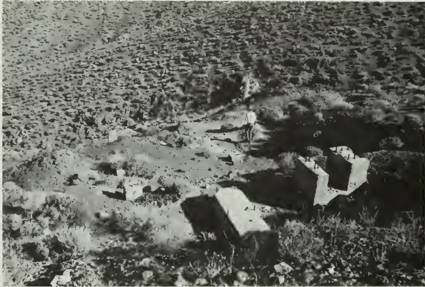
Ruins of the 1916 Lane mill, located just southwest of Chloride City. Photo was taken from the dump above the mill, showing the remnants of several concrete pedestals. The mill tailings are visible to the right front of the person in the photo, and the stone wall built to contain those tailings are just above his head.
