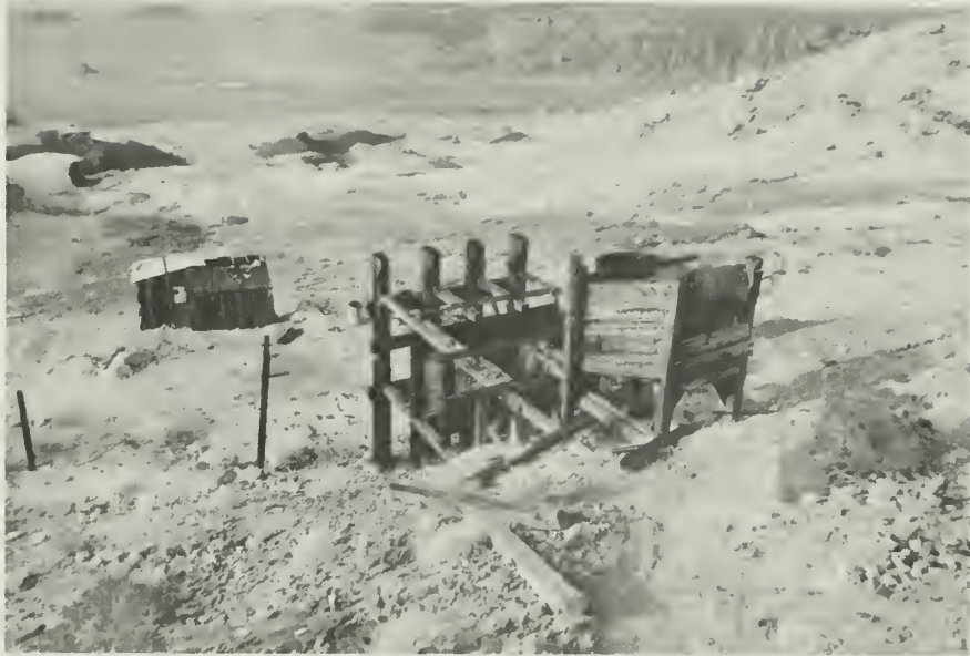
Johnnie Cyty's three-stamp mill, showing the small ore bin above the mill, and his shack below.
