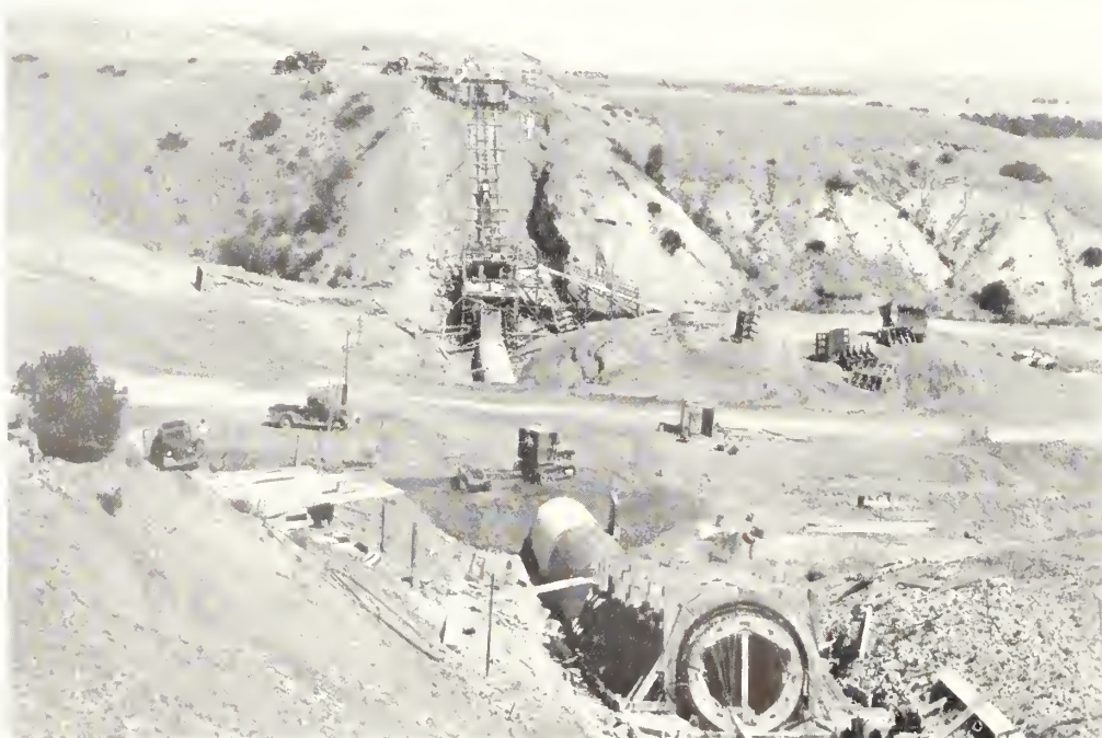
Siphon at main canal station 623+01 from inlet looking toward discharge
