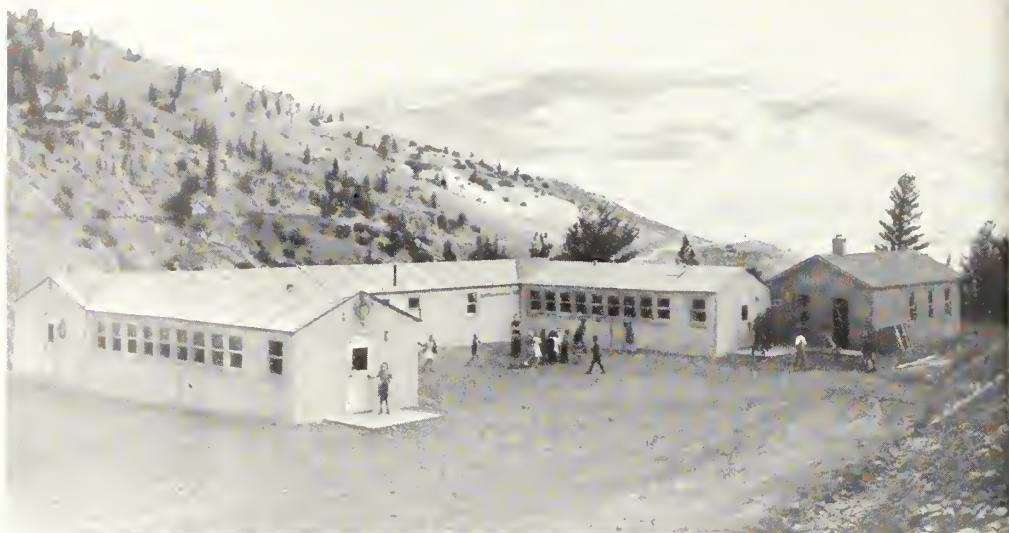
Looking eastward at contractor's recently constructed school buildings. High school is on right
