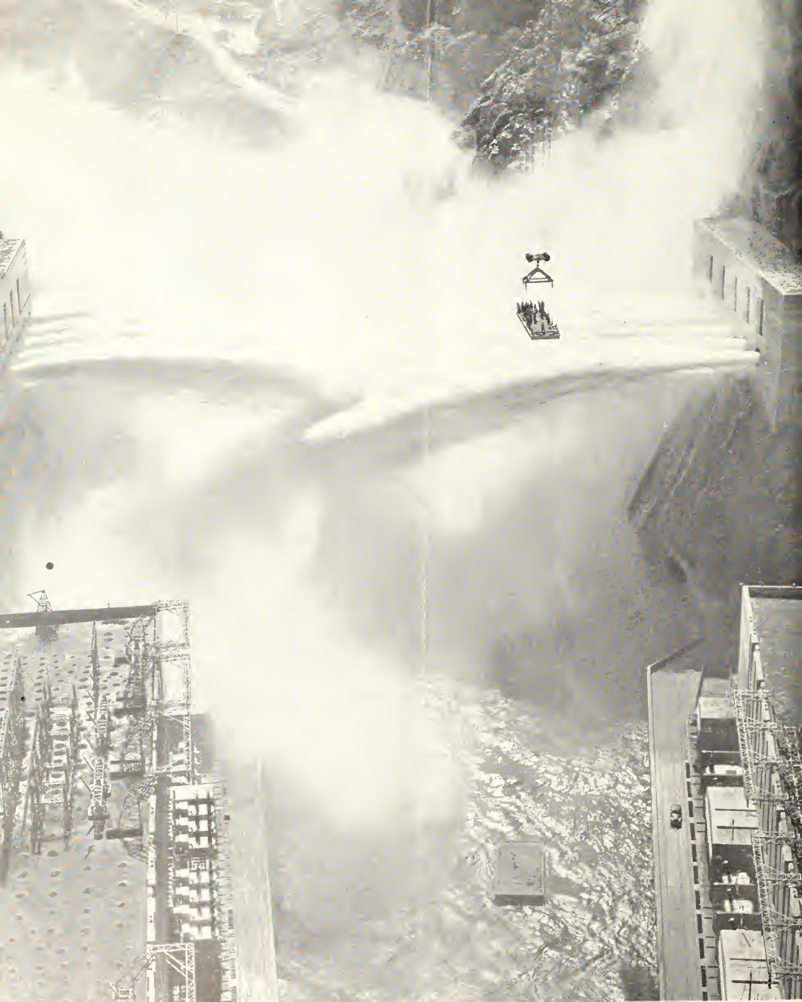
CELEBRATING BOULDER DAM'S FIFTH "BIRTHDAY" BY TESTING ITS NEEDLE VALVES. INSPECTION FROM THE CABLEWAY PLATFORM IS QUITE A THRILL
