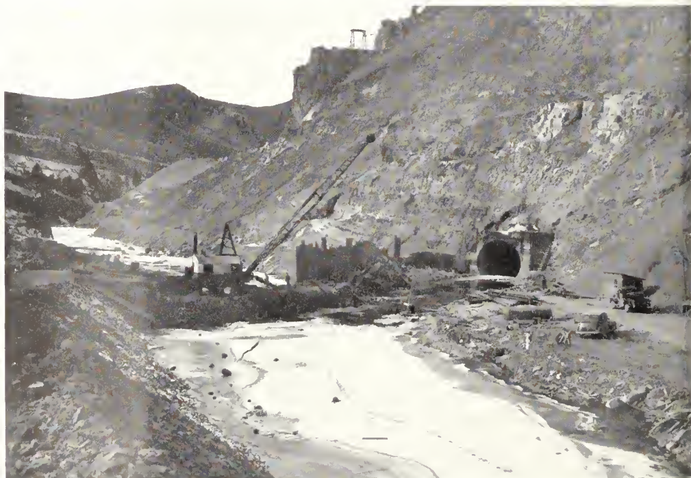
Green Mountain Dam
