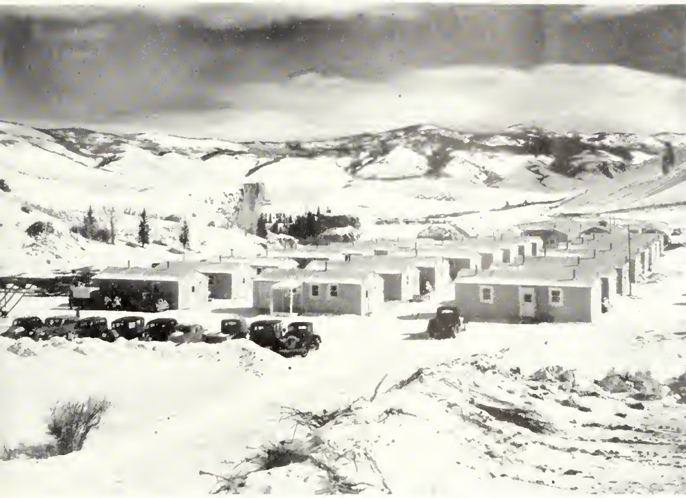
Looking eastward from top of stock pile at contractor's temporary camp
