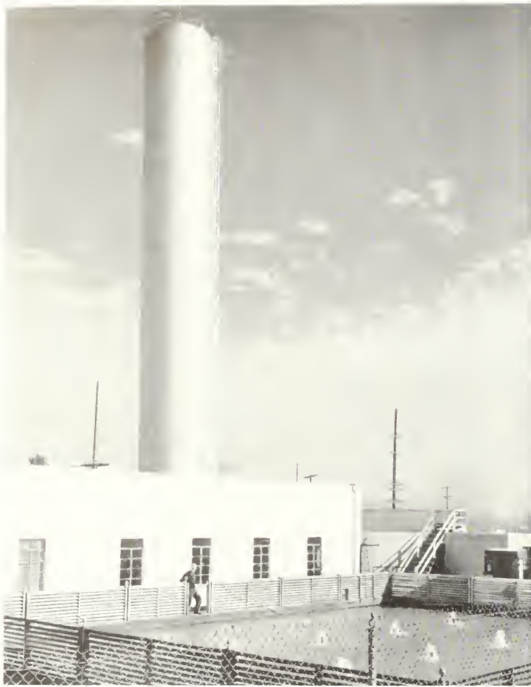
Aerating basin through which fresh water from the Contra Costa Canal is delivered to the city of Pittsburg
