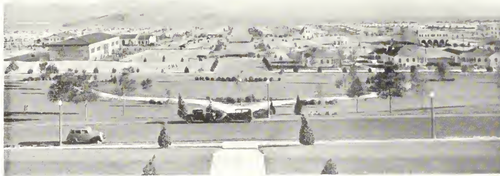
Boulder City, Boulder Canyon project, Nevada
