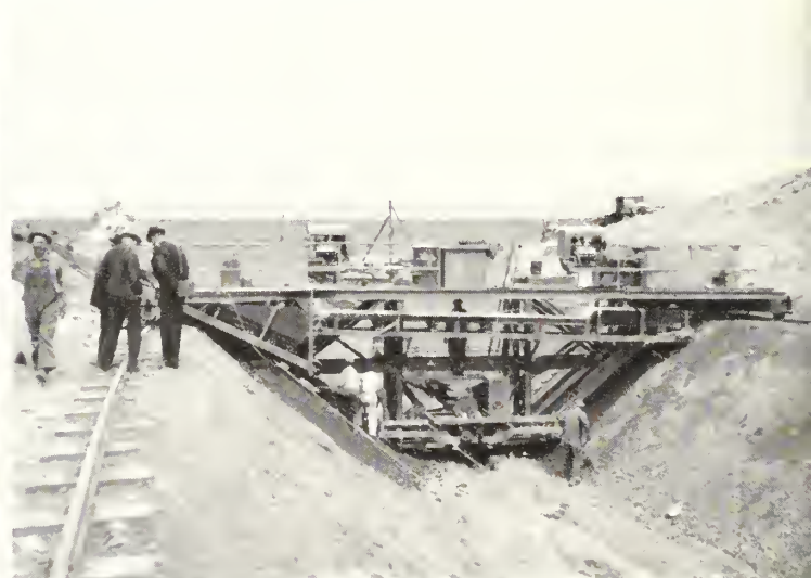
Photo 3: Canal trimming machine at Station 1124.
