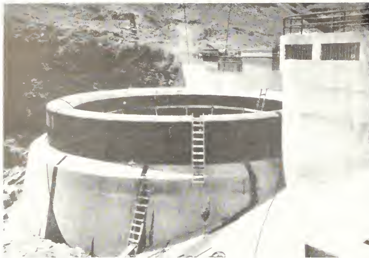
Figure 7. Ring gate floated to raised position during test.
