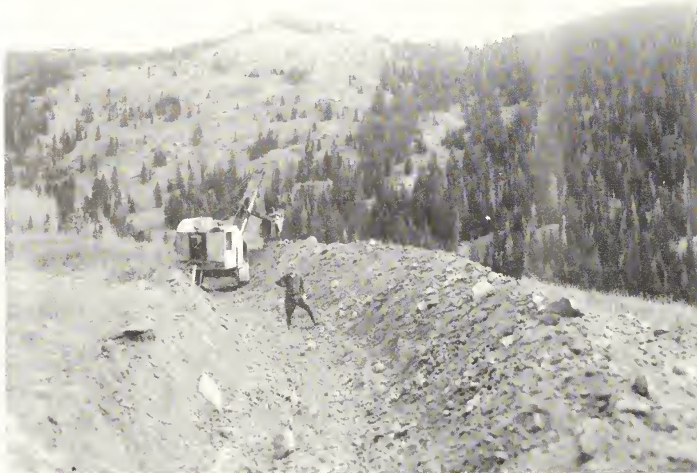
Excavation of Cedar Creek Feeder Canal, tributary to Spring City Tunnel
