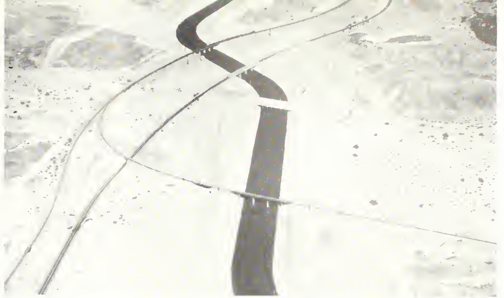
Four bridges span the All-American Canal at this point
