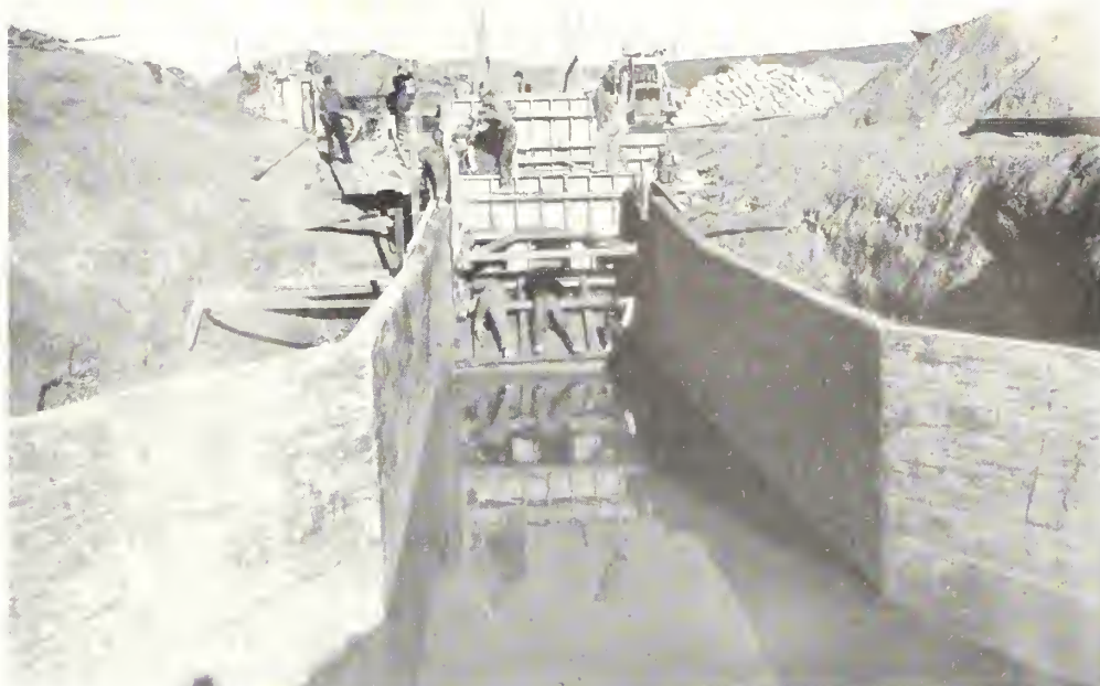
Placing concrete in Crackerbox Wasteway
