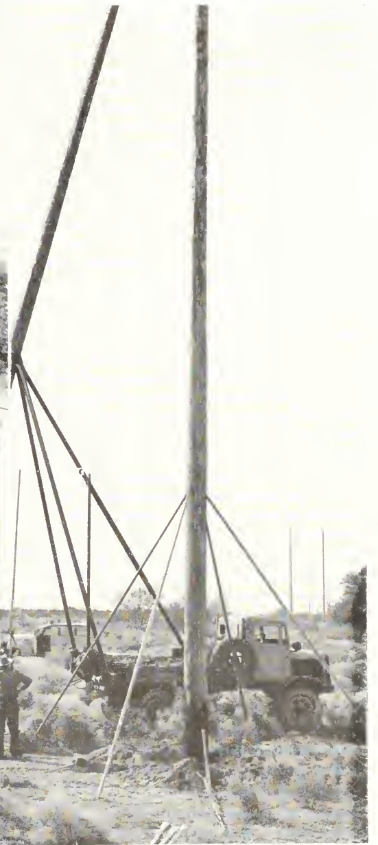
Placing the poles.
