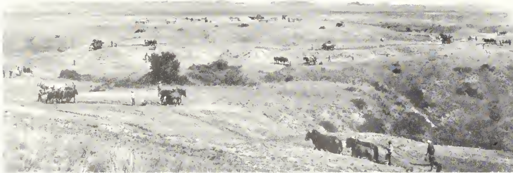
Main canal excavation operations at station 630+00
