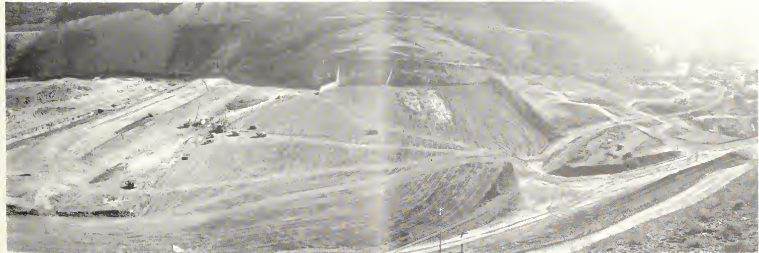
Panorama No. 2. Appearance of embankment December 1, 1939
