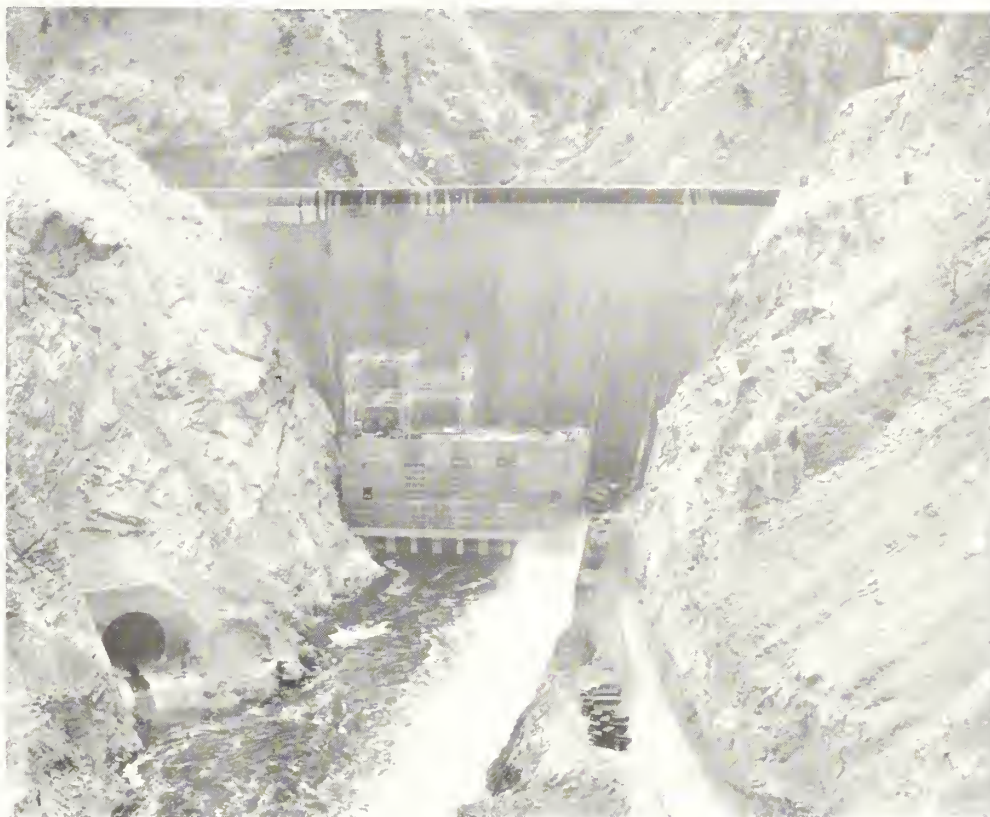
Seminole Dam and power plant, recently completed on the North Platte River
