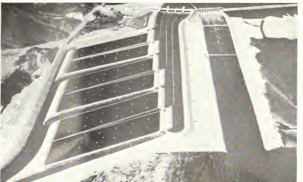
Desilting works, All-American Canal
