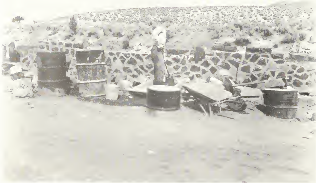
CCC enrollees constructing top course of parapet wall
