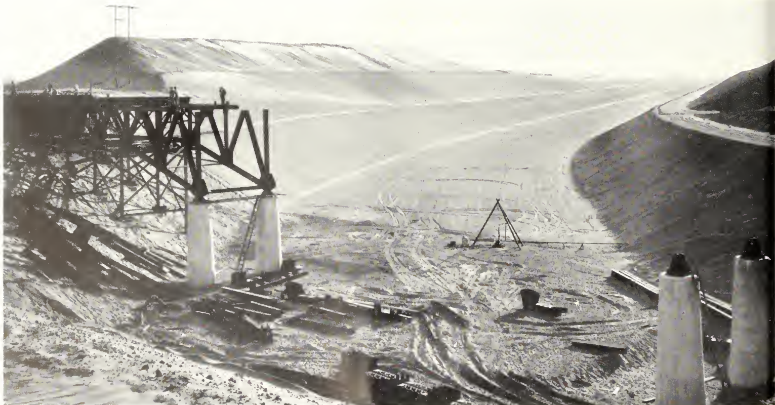
All-American Canal under construction
