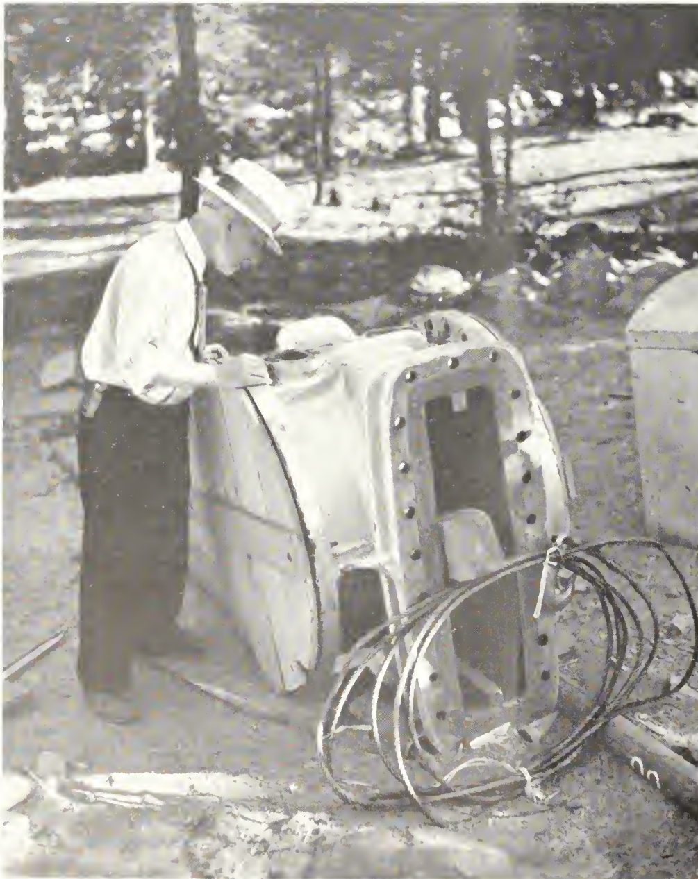
Valve for tunnel control works at Snow Lake, awaiting transportation over 6-mile trail to the lake
