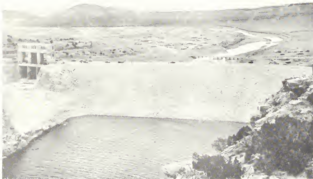
Alcova Diversion Dam, Kendrick project, Wyoming
