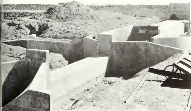
Turn-out and 3-way division structure at Allison Heading, 9 miles east of Calexico
