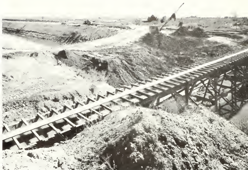
Metal flume carrying Alamitos Canal across All-American, with dragline removing "plug"
