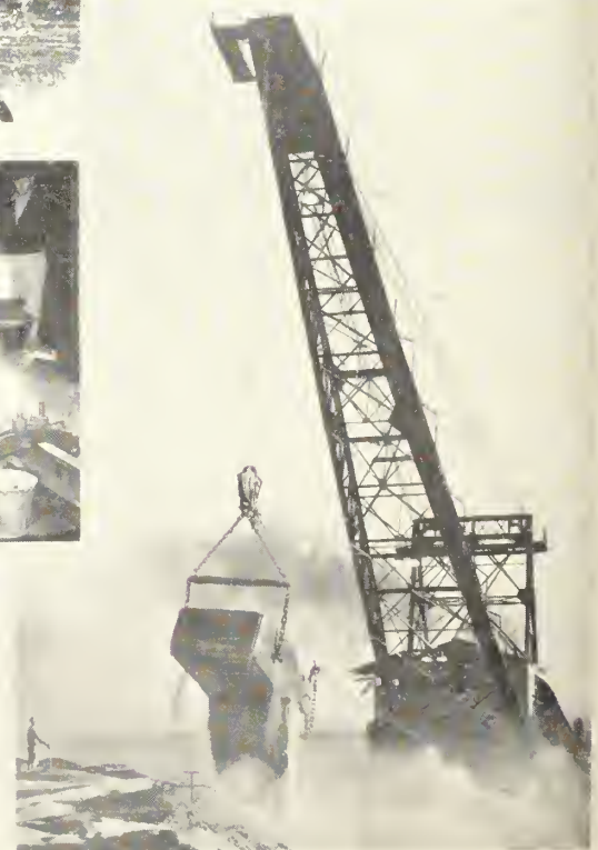
THIRTY-TWO TONS AT A BITE this shovel is digging the 134 mile Coachella branch of the All American Canal, California
