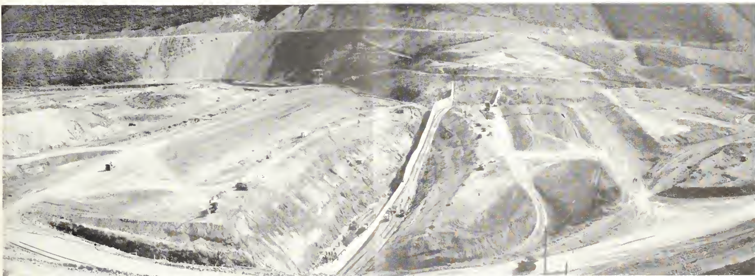
Panorama No. 1. Status of Construction October 26, 1939
