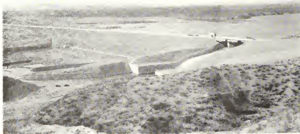
Upper: Elephant Butte Dam and Powerhouse; lower: Caballo Dam. Rio Grande Project, N. Mex.-Tex.
