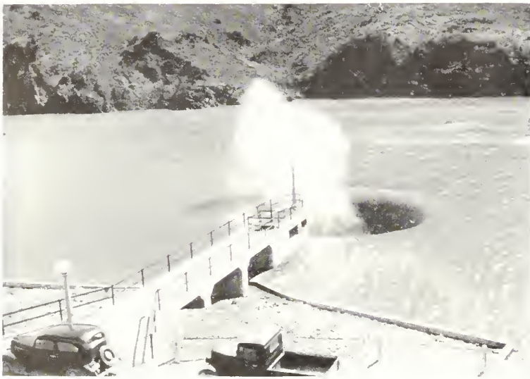
Figure 8. Spillway with 11½-foot depth on crest.
