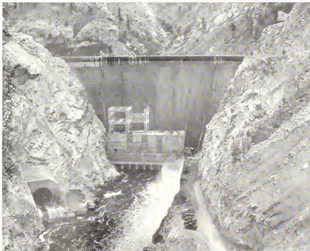
Seminole Dam, Kendrick project, Wyoming
