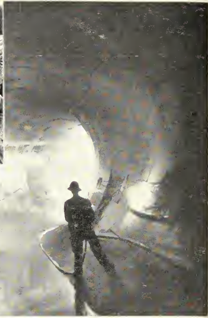
TUNNEL CURVE at Green Mountain Dam site, Colorado
