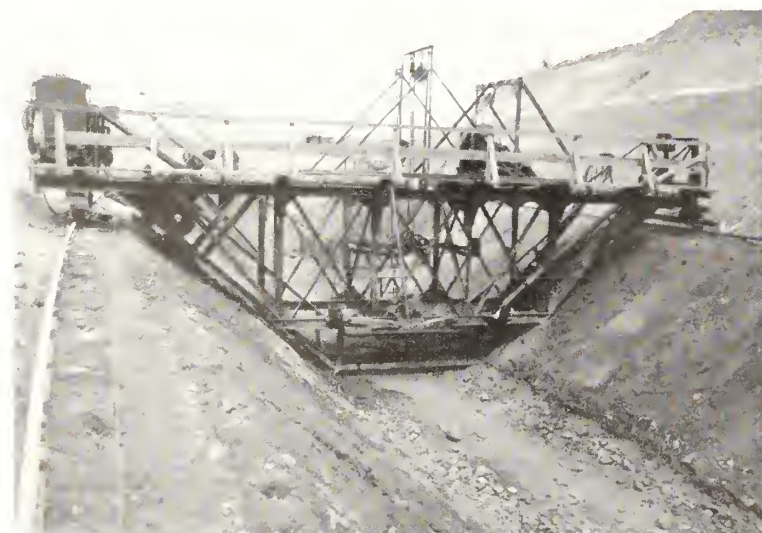
Photo 2: Compacting machine operating at Station 1125, 8 miles east of Yakima. Hammer at left.
