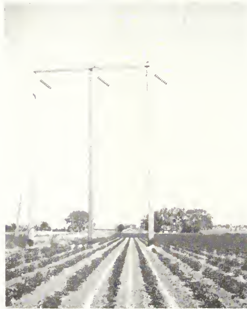
Power being transmitted across an irrigated field to homes on land to be benefited by Seminole Dam and power plant
