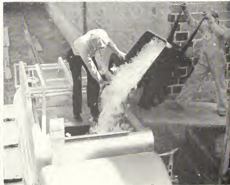
Ice is dumped into compartment of truck for purpose of cooling water in which salmon are placed
