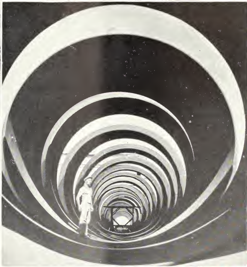
Pipe sections made of 16,000,000 lbs. of steel plate to be stitched together with 83 tons of welding rod, will line the penstock tunnels leading to the Grand Coulee power plant
