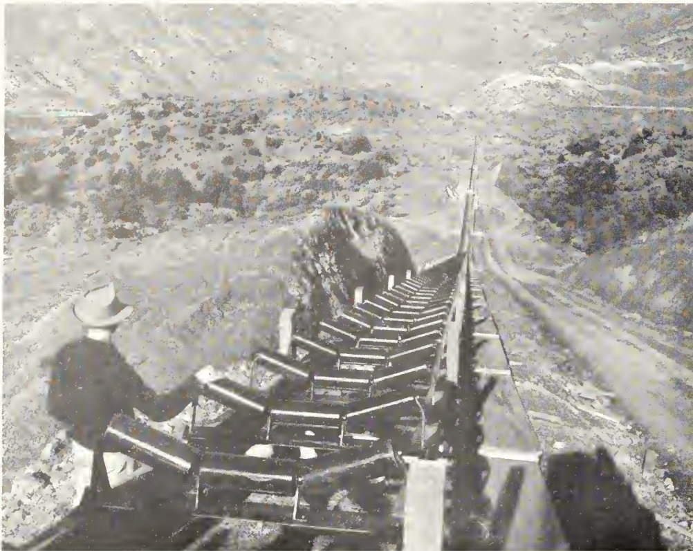
Aggregate conveyor between Redding and Coram, looking down long flight toward Sacramento River
