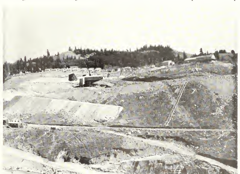
Looking southeast from edge of trash-rack excavation at contractor's permanent camp
