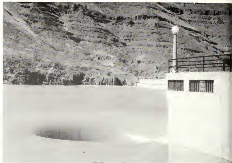
Figure 9. The glassy smoothness of the rapidly flowing water, 21½ feet deep over crest shown in this picture, as it starts its 300-foot plunge, is remarkable.
