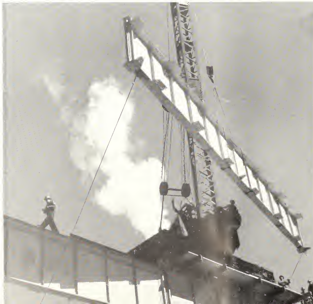
Bridge building for railroad relocation, Central Valley project
