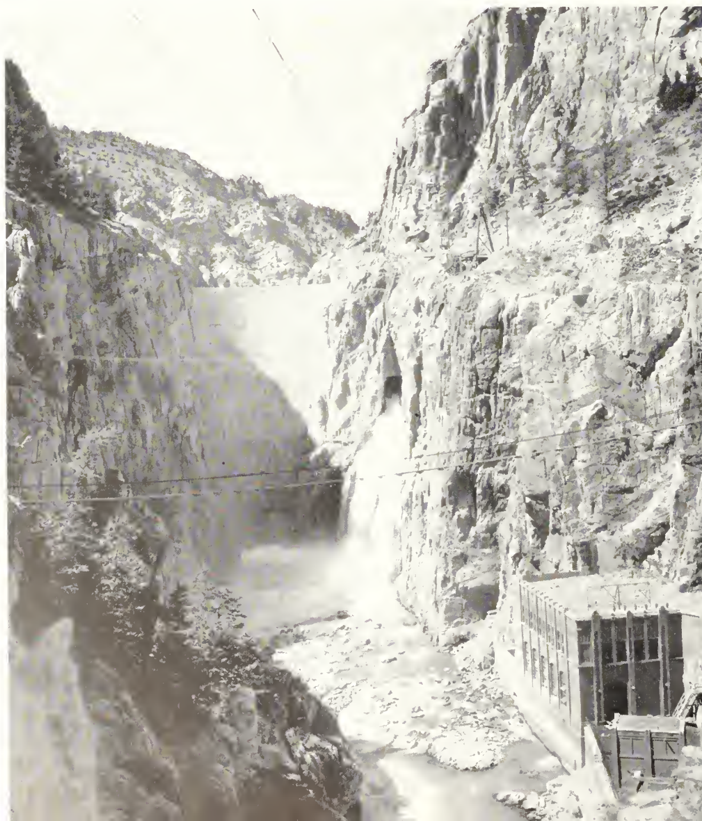
Shoshone Dam and Powerhouse, Shoshone Project, Wyo.
