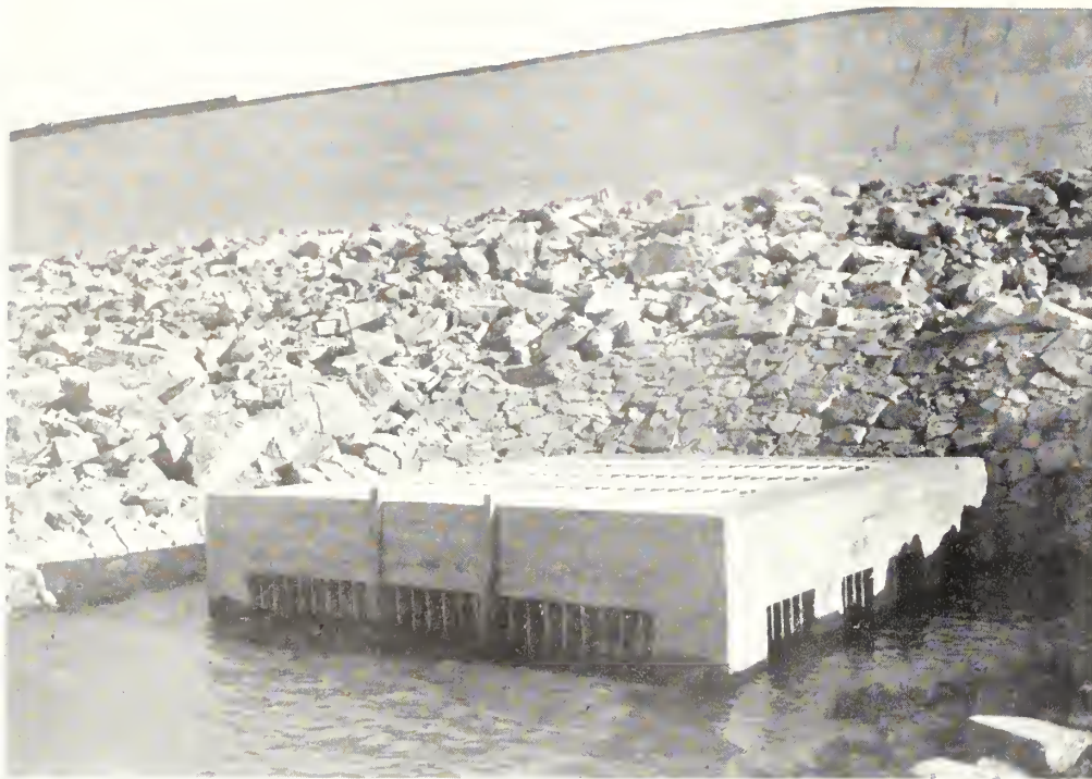
South crib and rock riprap
