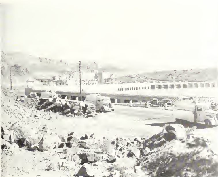
Trucks loaded with salmon leaving Rock Island Dam for Columbia River and tributaries
