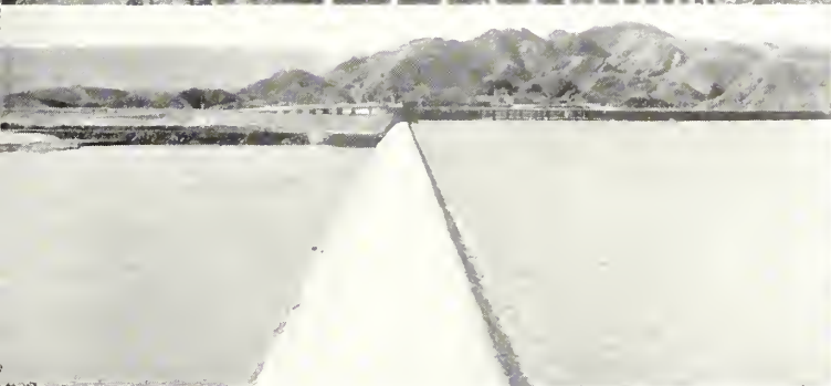
Top: Roosevelt Dam, Salt River project, Arizona Center: Stoney Gorge Dam, Orland project, California Bottom: Imperial Dam, All-American Canal, Arizona-California
