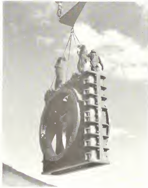
Gate frame section of 102-inch valve.
