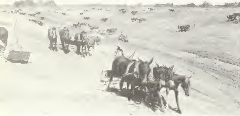
"Four-mule-power" fresno scrapers at work on new canal across Imperial Valley, just north of International boundary
