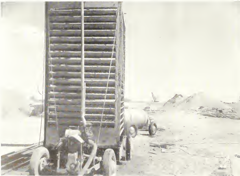
Portable cooling tower used for pre-cooling concrete-mixing water on Coachella Branch of All-American Canal
