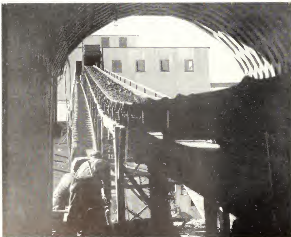
Looking out of recovery tunnel under raw storage pile toward mill building, during first test run
