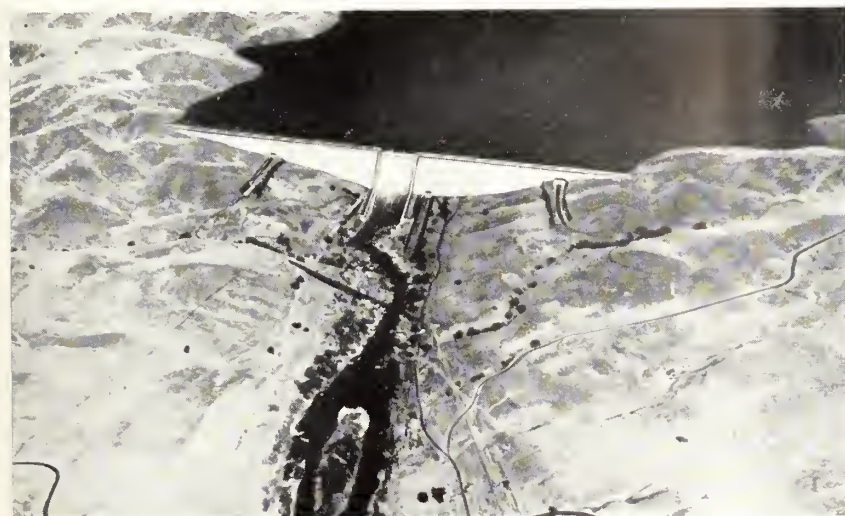
Friant Dam, Central Valley Project, California
