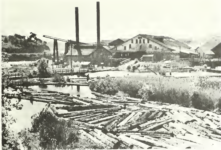
Figure 3.- This is a large sawmill typical of those found on the large timber holdings on the coast. These large mills generally saw 25 or more million board feet of lumber per year. They use principally redwood and Douglas-fir timber. The first sawmill on this site was constructed in 1860 but it burned in 1889. The present mill was built on this same site in 1890. It has operated almost continuously ever since.
