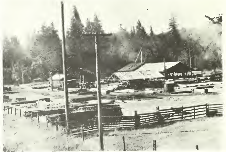
Figure 4. This is a small sawmill typical of some recently constructed by forest industries in this area. These mills produce from 1 to 10 million board feet of lumber per year. They saw redwood and Douglas-fir timber mostly.
