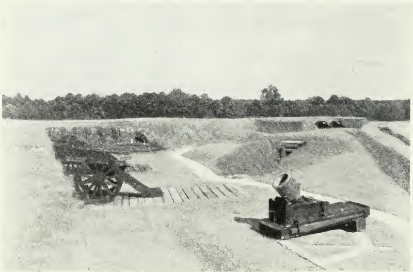
Figure 35. —HISTORICAL EXHIBITS IN PLACE. RESTORED EARTHWORKS, ORIGINAL ORDNANCE IN NEW MOUNTINGS. GRAND FRENCH BATTERY, COLONIAL NATIONAL HISTORICAL PARK, VIRGINIA
