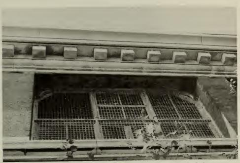
19. Second floor window, exposed riveted spandrel beam, north projection.
