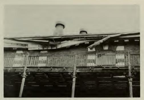
50. Collapsing gutter; missing bracket and extant cast-iron capital, porch; south elevation, view north.
