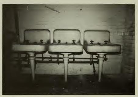
26. Typical pedestal sink installed between 1900-1924, room 204.
