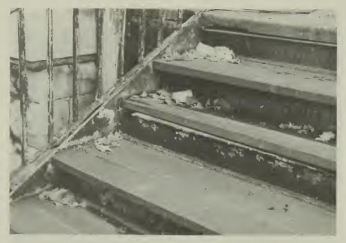
53. Corroded risers, unstable slate treads, porch stairs.
