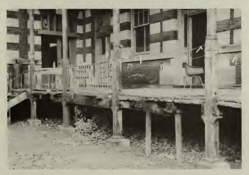
51. Corroded beams, missing railing, temporary shoring. Porch, view northwest.
