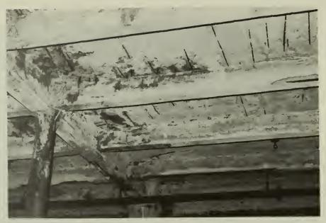
5. Room 209- reinforcing rusting through slab soffit. Spalling of ceiling parging.
