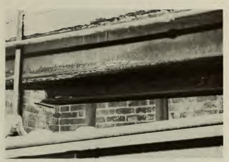
7. Delaminating corrosion of flange of steel beam added under first floor construction.
