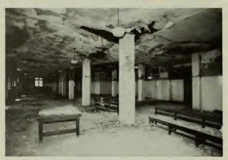
14. Room 212- view southwest- tile wainscot on walls and columns, tile floor, deteriorating plaster on walls and ceiling.
