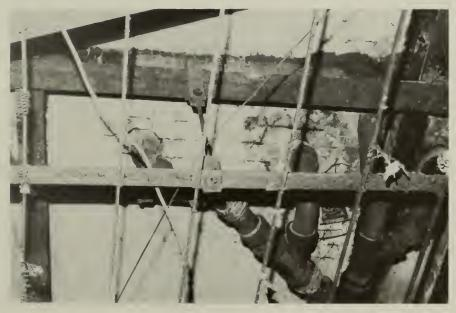
Second floor hung ceiling, corroded beams and exposed metal lath.
