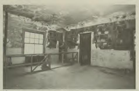
35. Room 201- deteriorating plaster and exposed terracotta block in northeast corner.
