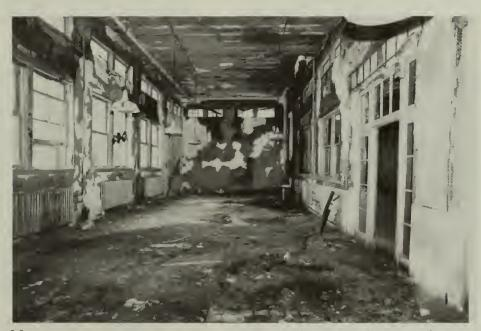
36. Room 119- destroyed plaster finishes and extensive moisture penetration.
