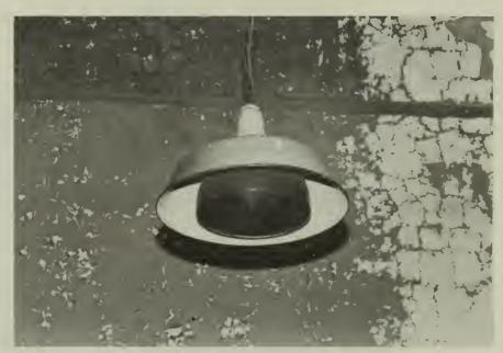
6. Type B- RLM fixture with blue tinted globe lamp, room 125, ca. 1939.
