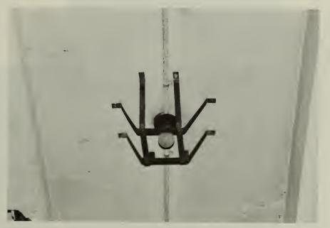
12. Conduit mounted housing with lamp, metal strip guards occur in second floor recreation porchroom 210 and 211
