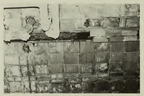
First floor ceiling, corroded beam soffits and missing tile.
