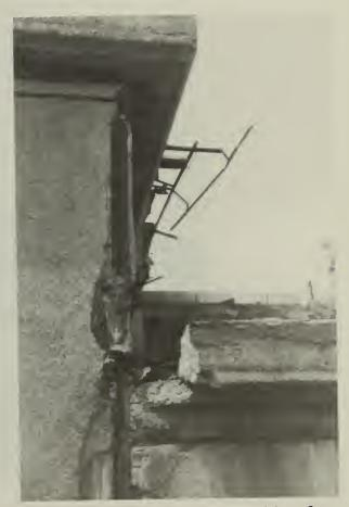
55. Spalling concrete, corridor from the kitchen and laundry to the bakery and carpentry (hall 201).
