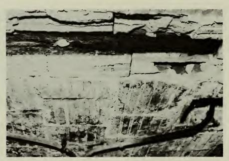
Corroded bottom flange of first floor steel beam in northeast corner of basement ceiling.
