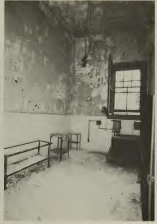
Room 102- tile wainscot, hexagonal tile flooring, plaster walls and ceiling.
