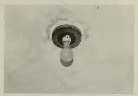
11. CML- bare lamp in porcelain socket set in ceiling mounted metal housing, typical,
