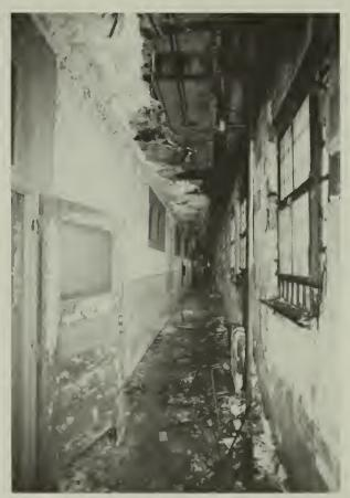
22. Hallway 201- view north, hung ceiling destroyed, severe deterioration of materials on exterior light court wall (right).
