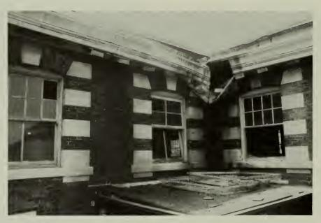
49. Deformed gutter falling off, juncture of east pavilion and north elevation, view southeast.
