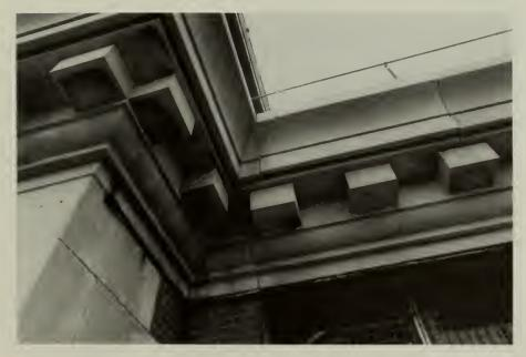
40. Open mortar joints, cornice, east elevation.
