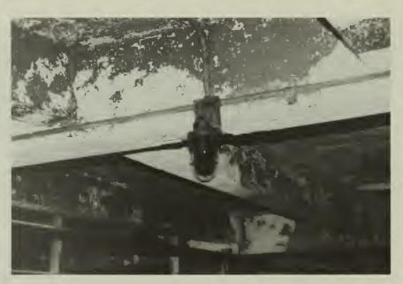
Type C- 'Vaportight' fixture with cast metal guard, room 122, ca. 1935.
