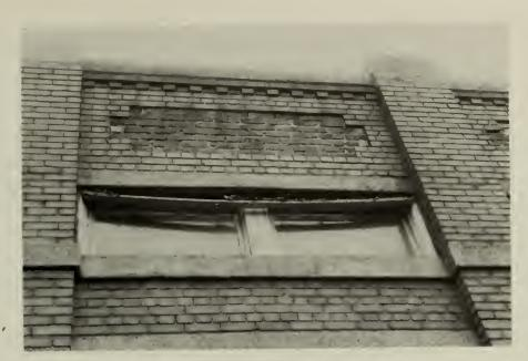
58. Warped and separating window frame, "Ice Plant", north elevation.
