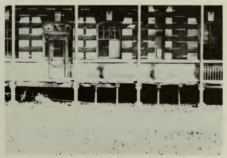
South porch. Decomposition of steel supports and I-beams.
