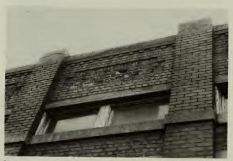
57. Spalling and loss of masonry units. "Ice Plant", north elevation.
