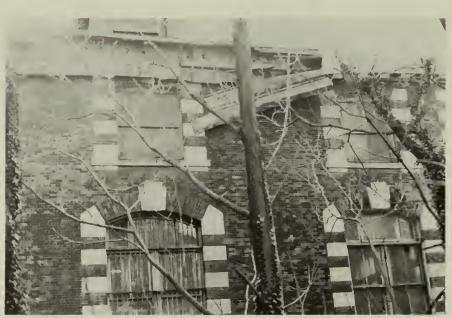
North facade. Collapse of copper cornice and gutter.
