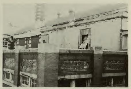
3. North facade, western end. Deterioration and sag of copper cornice.
