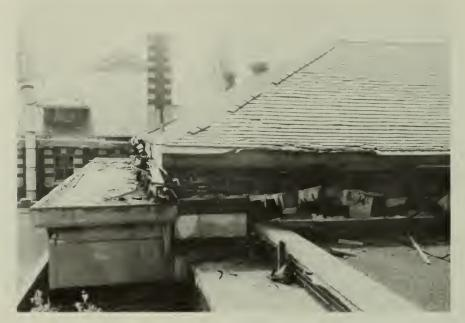
48. Missing, cracked, and spalling roof tile; deformed gutter falling off, west pavilion, northwest corner, view east.
