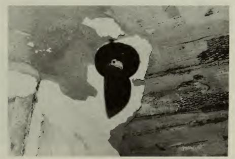
8. Type C- porcelain socket with metal ceiling mounted housing and directional metal shade, (found at perimeter of second and third floor dormitories)
