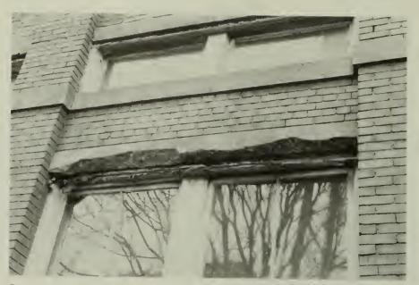
56. Spalling at window lintel, "Ice Plant", north elevation.
