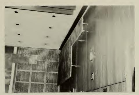
31. The mural is mounted on wood panels that are suspended from the wall on metal brackets.
