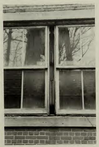
59. Exposed rusted counterweights, "Ice Plant", north elevation.
