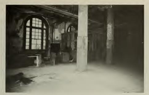
8. Room 114- finishes of concrete flooring, cement plaster wainscot and freestanding columns encased with galvanized iron.
