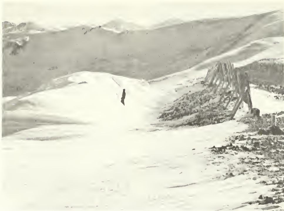
Figure 7. —Natural drifting of snow (foreground) in the alpine can be enhanced by placing fences to put additional snow on top of an already deep snowpack. This is done to increase the runoff during summer months from such areas.
