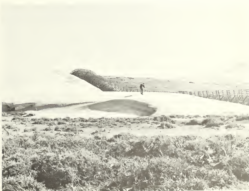
Figure 22.—By trapping snow behind snow fences such as this evaporation of blowing snow is reduced, and snowmelt water is concentrated to enhance its delivery to the stream or ground water recharge.
