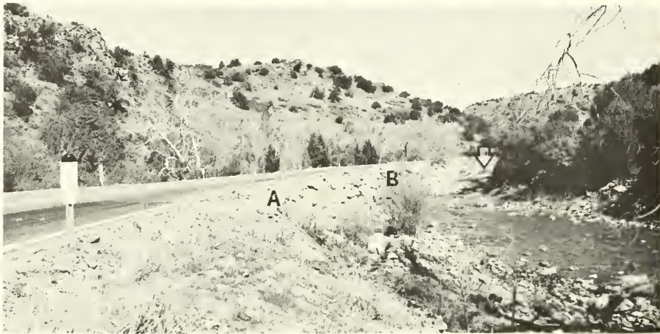
Figure 22.—(a) In mountain country, highway construction often infringes on streams. A relatively large meander bend (A) of Sycamore Creek, central Arizona (flowing from left to right), was cut off and the streambed relocated to the opposite side of the road (B). Thus streamlength was shortened, slope gradient steepened, and a nickpoint introduced at (D) that led to the development of a bedscarp in the volcanic bed rocks. This scarp advanced about 300 feet upstream (C) within approximately 25 years. At (D), the original meander bend connected with a short straight reach still used by the creek. (b) Closeup view of the 8-foot-deep bedscarp (arrow). Adjustment processes not only caused a bedscarp but also tried to reestablish the meander, endangering the road bed by undercutting. (c) Rock riprap bank protection was required between A and B to protect the road. Arrow signifies bedscarp location.
