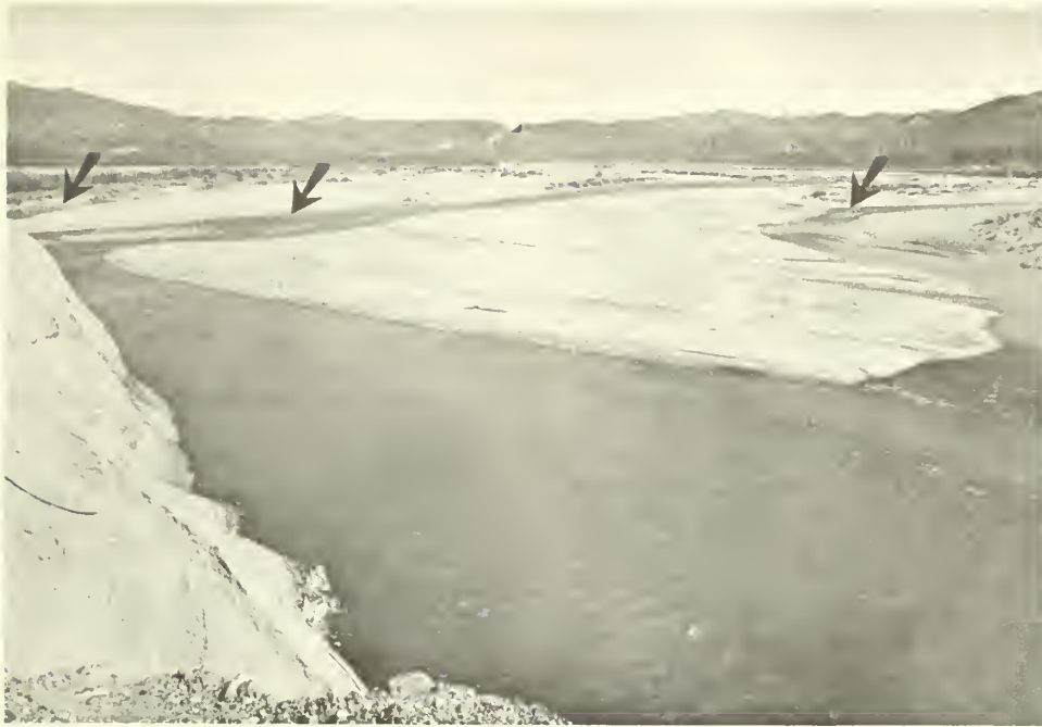
Figure 17.—Heavy sediment loads in this Salt River reach above Roosevelt Reservoir, Arizona, created a wide bed with shallow flow depth. Thus, stream competence (sediment-carrying capacity) was drastically reduced. To increase flow depth (and competence), the flow split into several channels (arrows). Flow in the foreground is from left to right.
