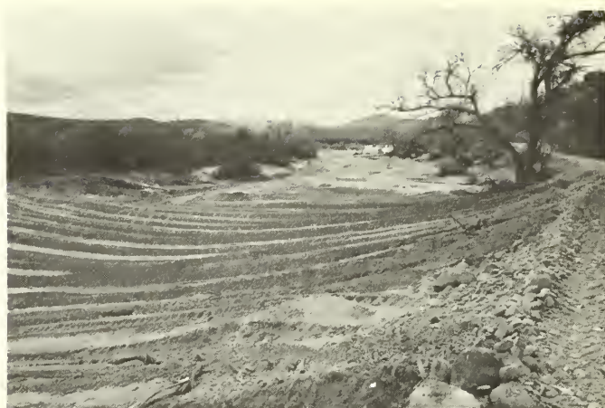
Figure 24.—Tractor excavation of sediment from this streambed was unavoidable because of the road location. Since sediment loads are very high during high flows, as indicated by high frequency of large bars in the river, this branch channel will refill. In the long run, relocation of the road may be less costly than repeated excavations.
