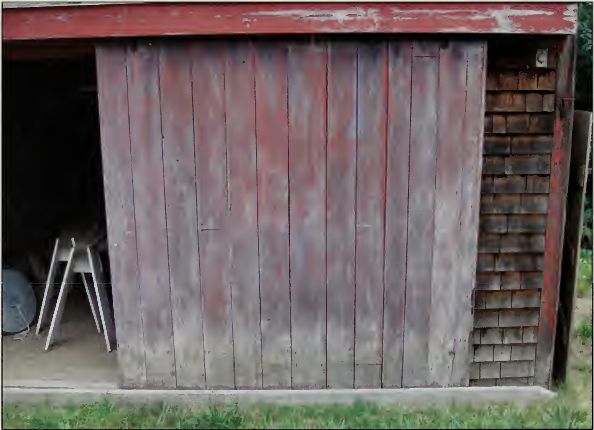
Figure 234. D101 in west elevation, Woodshed (2007).
