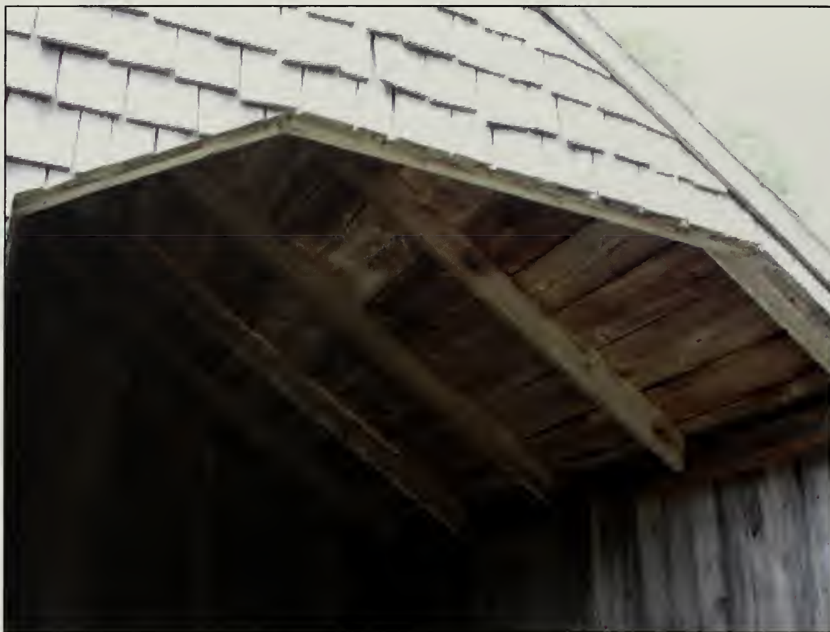
Figure 346. Ceiling of Open Shed, Barn (2007).
