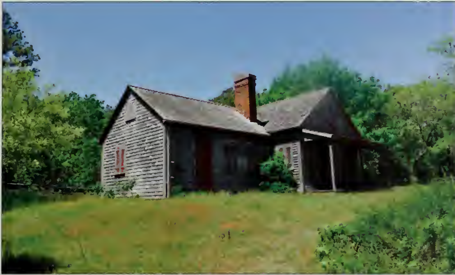
Figure 81. Vegetation south and east of the Country Store. Note the Japanese barberry next to the porch, at center, and the clump of cactus and rose in the foreground (OCLP, June 2010.)
