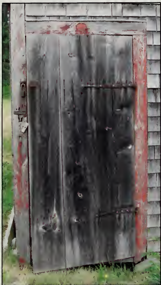
Figure 235. D102 in south elevation, Woodshed (2007).
