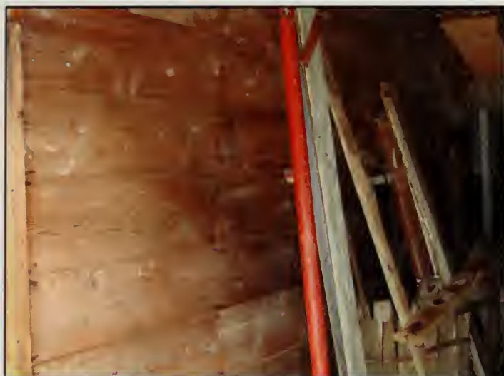
Figure 268. Southeast wall, flush horizontal boards, Room 101, Garage (2007).
