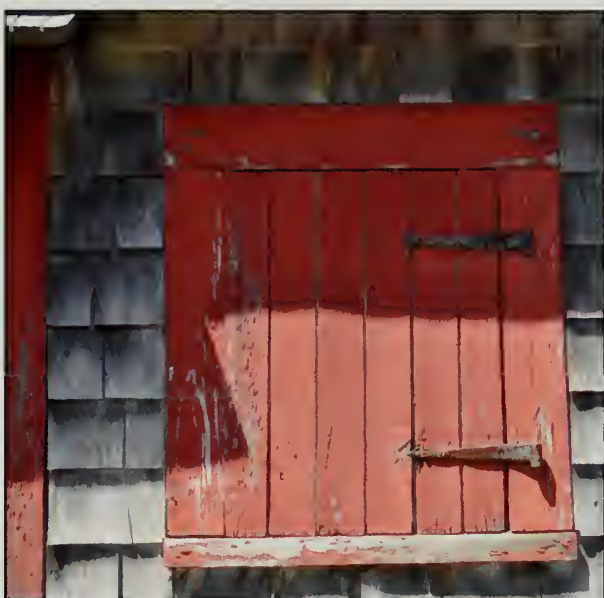
Figure 373. W107 in south elevation, Guest House (OCLP, 2010).
