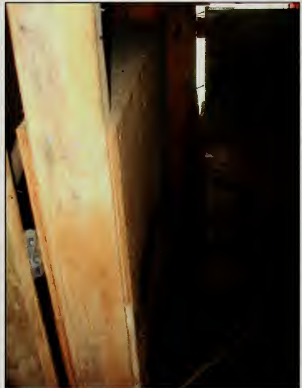
Figure 318. West wall of Box Stall, Barn (2007).
