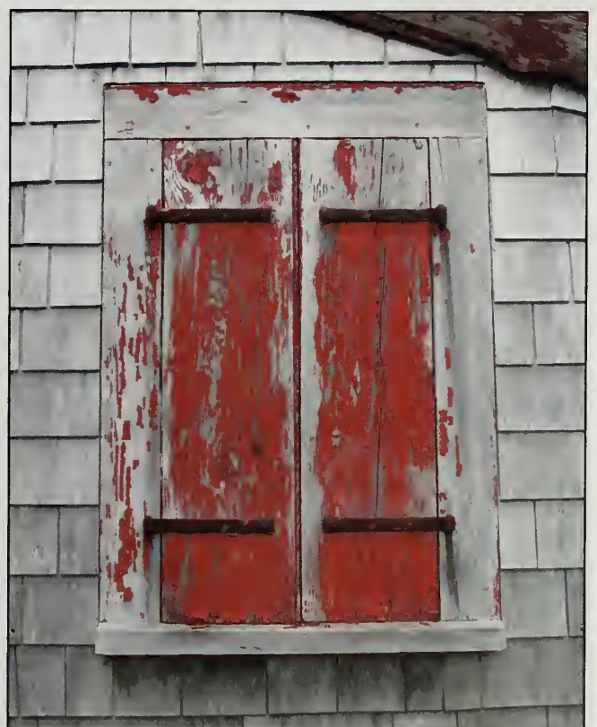
Figure 489. W104 in east elevation, Country Store (2007).
