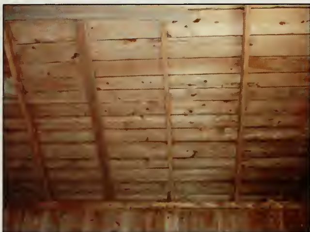
Figure 340. Ceiling of Carriage Room, Barn (2007).
