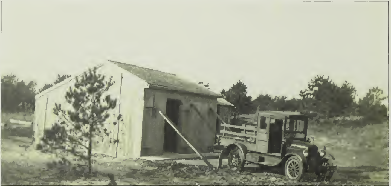
Figure 160. Looking northwest at the new Garage, 1929. Note the sparse vegetation and disturbed soil, likely due in part to grading at this location. (Cape Cod NS archives, H6-187.)
