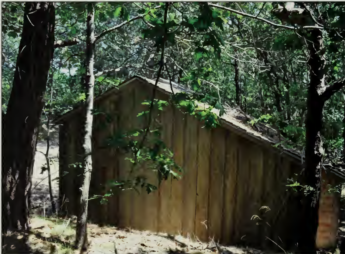
Figure 255. Northwest elevation, Garage (OCLP, 2010).
