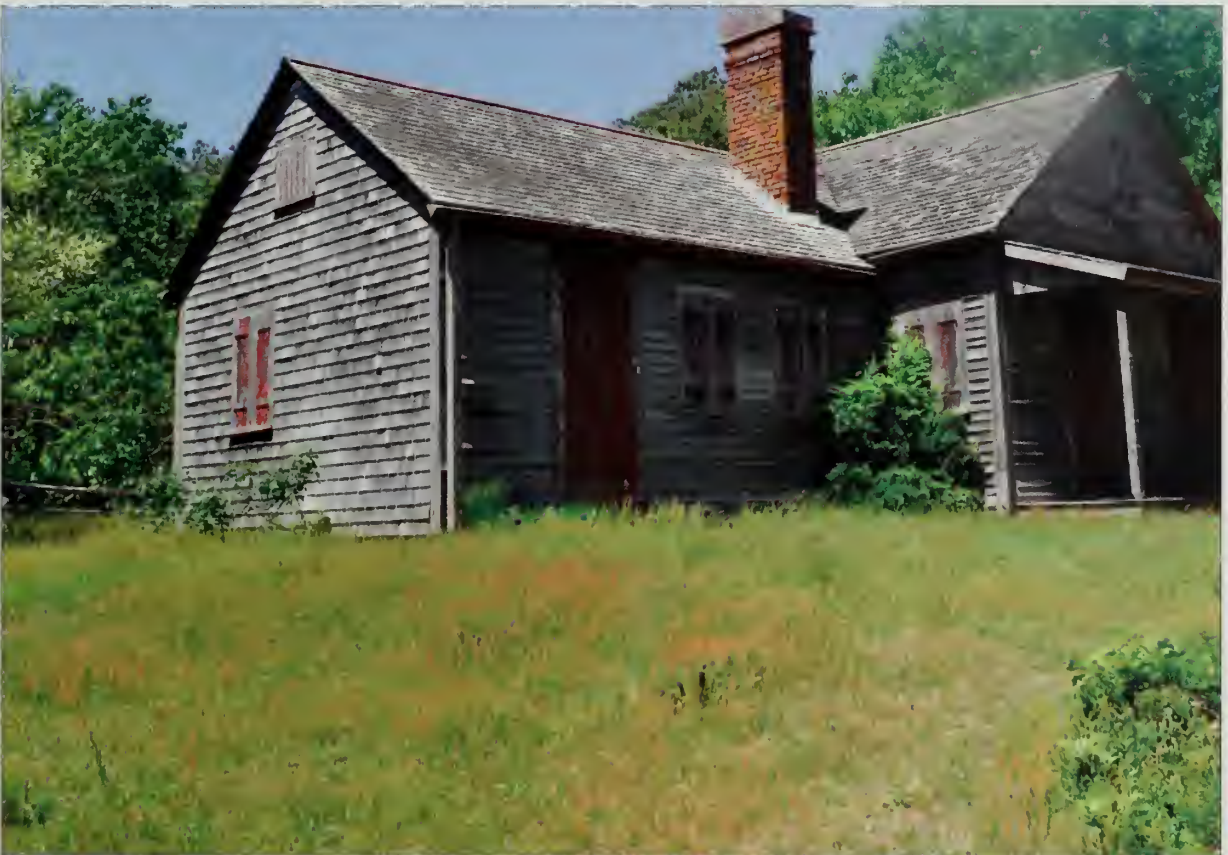
Figure 154. Looking northwest toward the Country Store, May 2010. (OCLP.)
