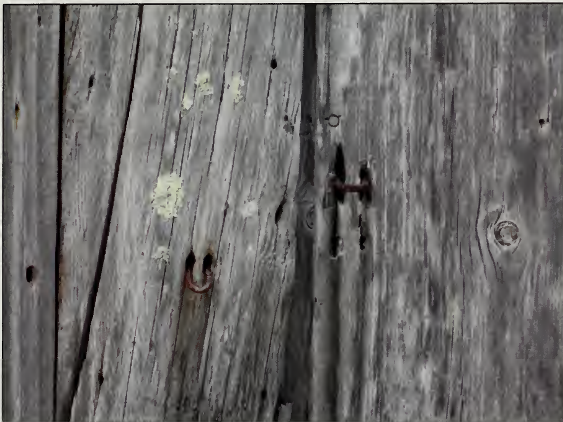
Figure 292. Hardware (two iron eyes) on door within D103, east elevation, Barn (2007).
