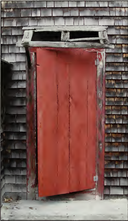
Figure 483. D104 in west elevation, Country Store (2007).
