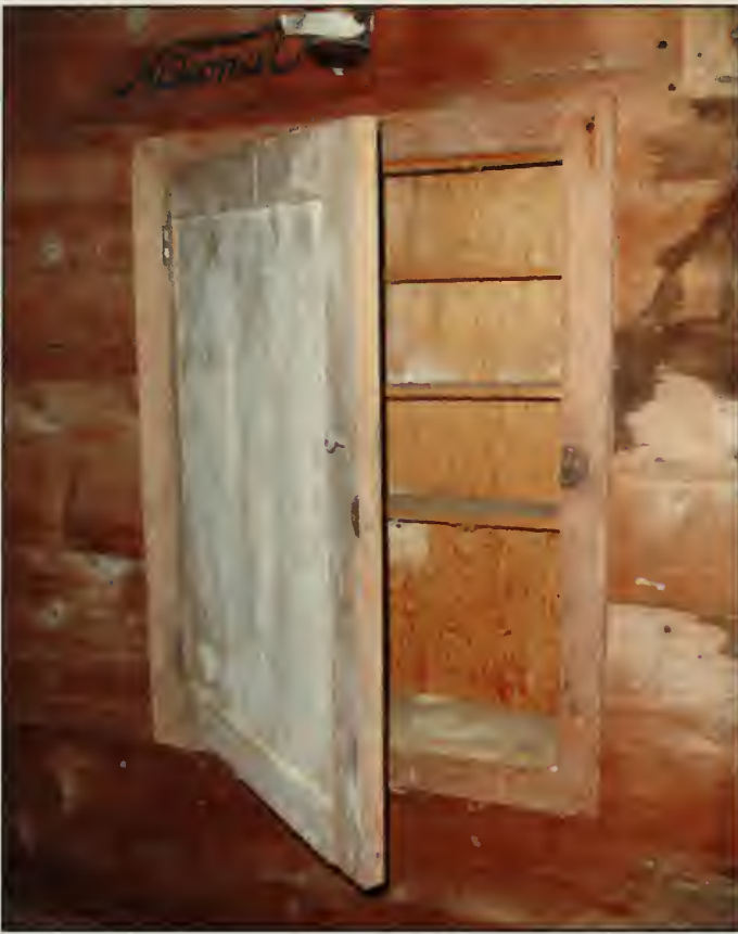
Figure 277. Built-in cabinet, in center of northwest wall, Room 102, Garage (2007).
