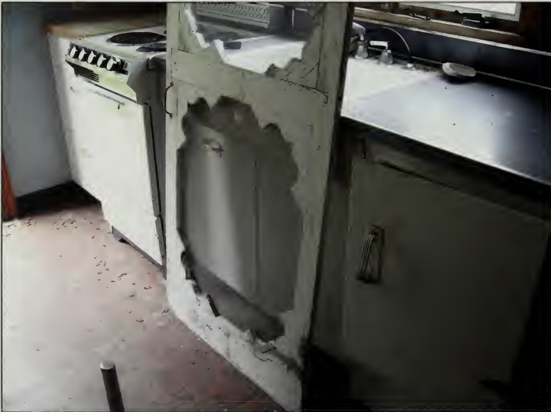
Figure 442. Lower west wall of Kitchen, Guest House (2007).
