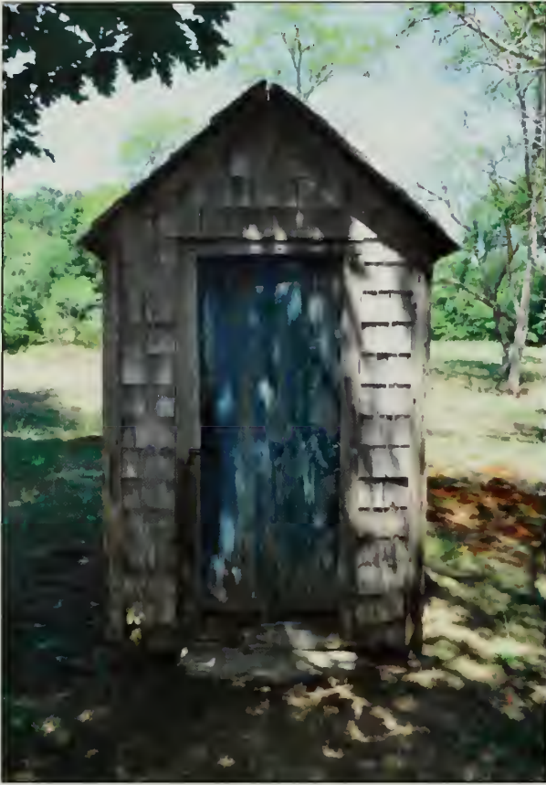
Figure 535. South elevation, Guest House Privy (OCLP, August 2010).
