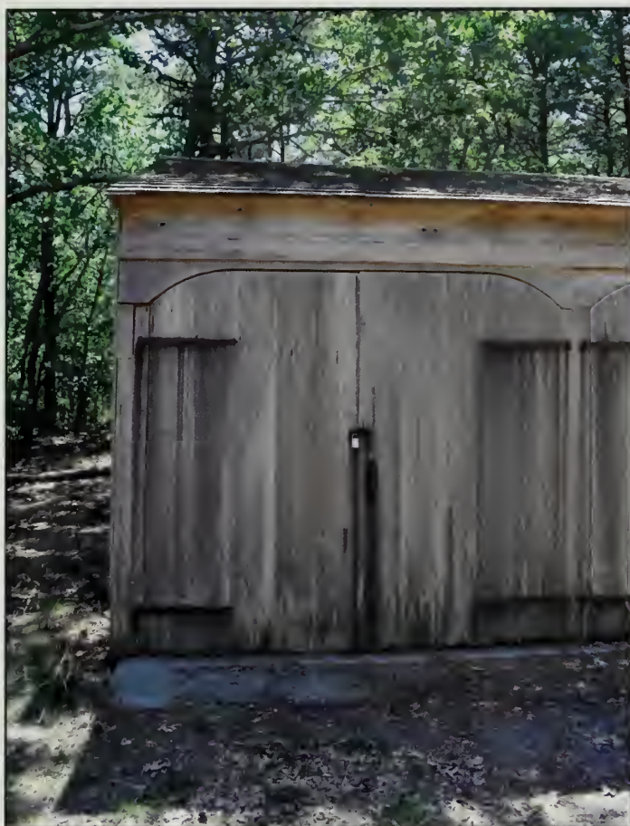
Figure 259. D101 in northeast elevation, Garage (OCLP, 2010).
