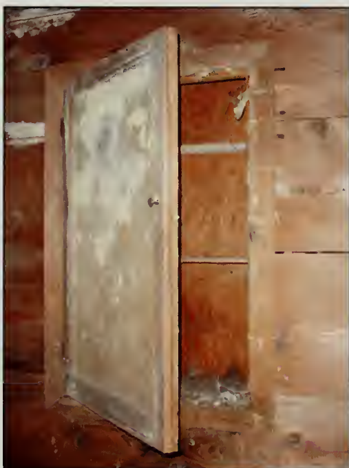
Figure 270. Built-in cabinet, right of D104. Northwest wall, Room 101, Garage (2007).
