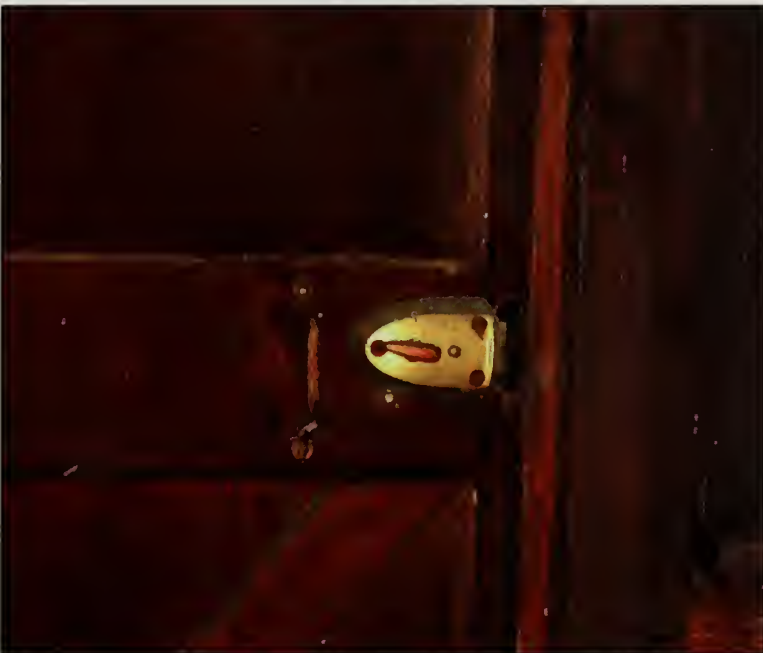
Figure 469. Deadbolt lock and metal door pull on interior of D101, Summer House (2007).
