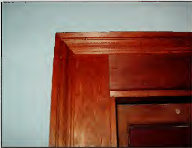
Figure 444. Window trim on W109 on east wall of Kitchen, Guest House (2007).
