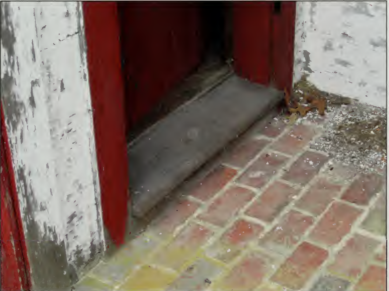
Figure 361. Threshold located within D101, west elevation, Guest House (2007).
