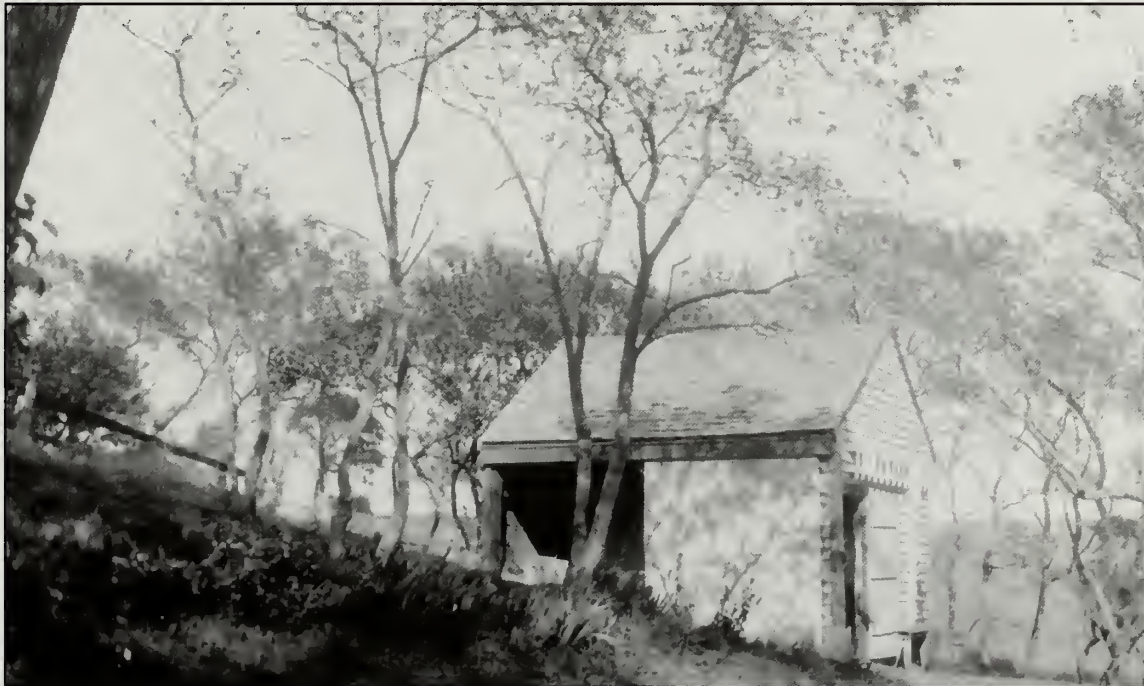
Figure 202. Woodshed in 1921 with newly shingled north and south elevations. (CACO Archives/GKH Journal).
