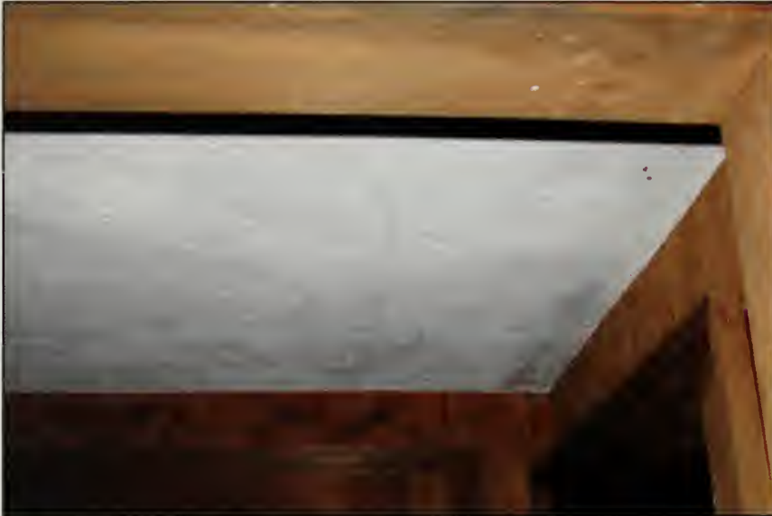
Figure 436. Ceiling of Closet, Guest House (2007).
