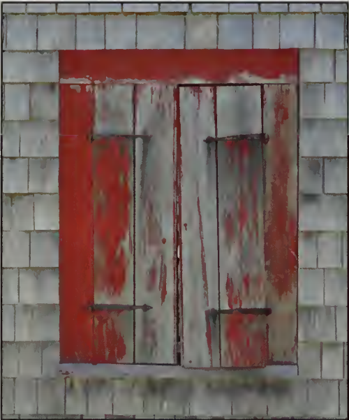
Figure 376. W111 in east elevation, Guest House (OCLP, 2010).
