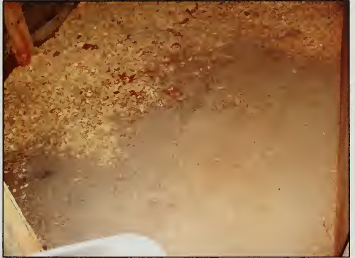
Figure 314. Floor of Box Stall, Barn (2007).
