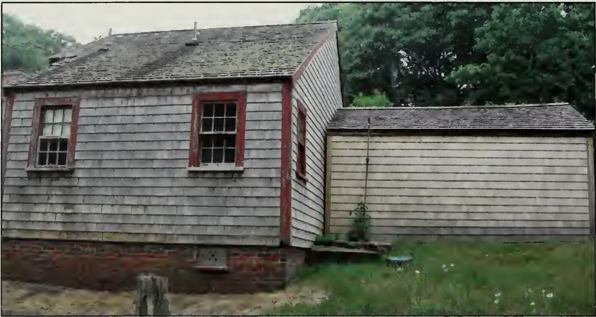
Figure 233. East elevation, Woodshed, showing brick foundation on Laundry/Bath addition (2007).
