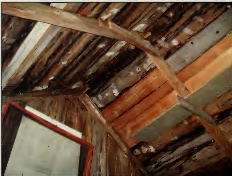
Figure 244. Ceiling of Storage Room, Woodshed (2007).
