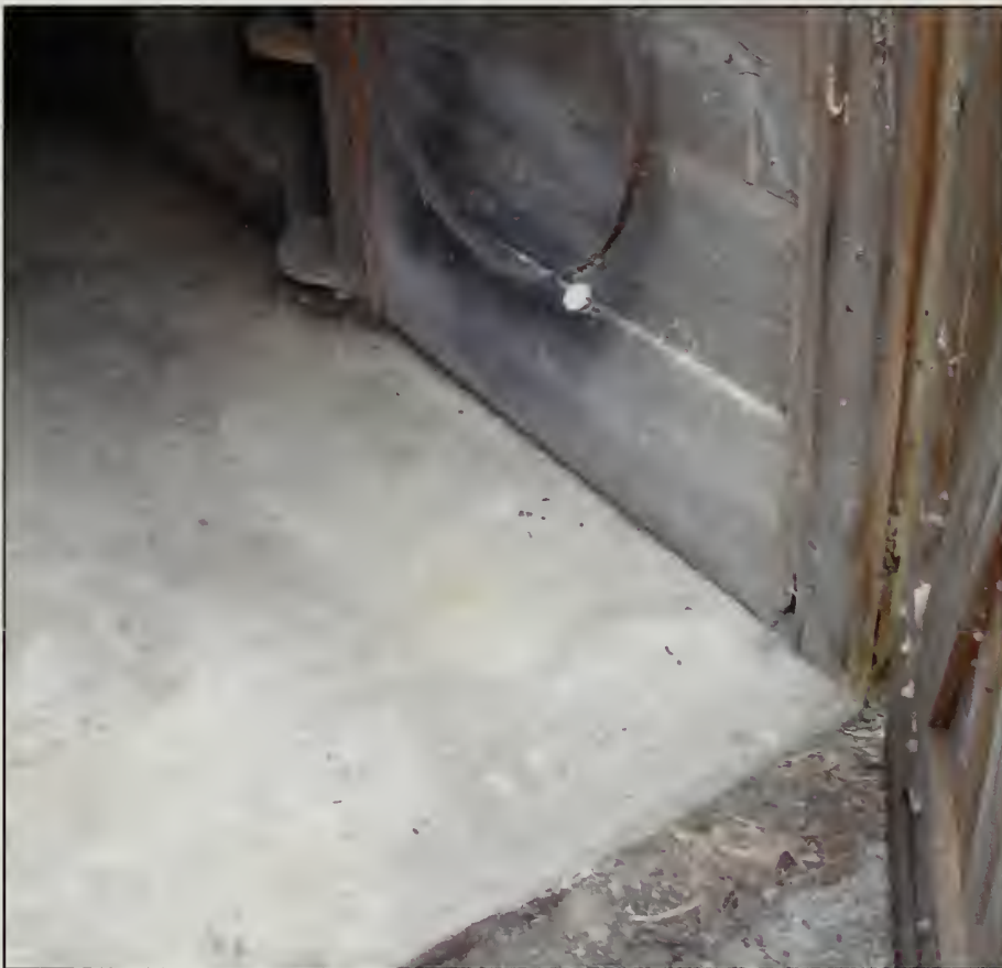
Figure 267. Poured concrete floor of Room 101, Garage (2007).
