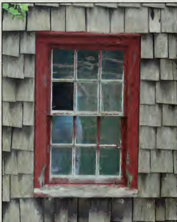
Figure 302. W108 in west elevation, Barn (2007).
