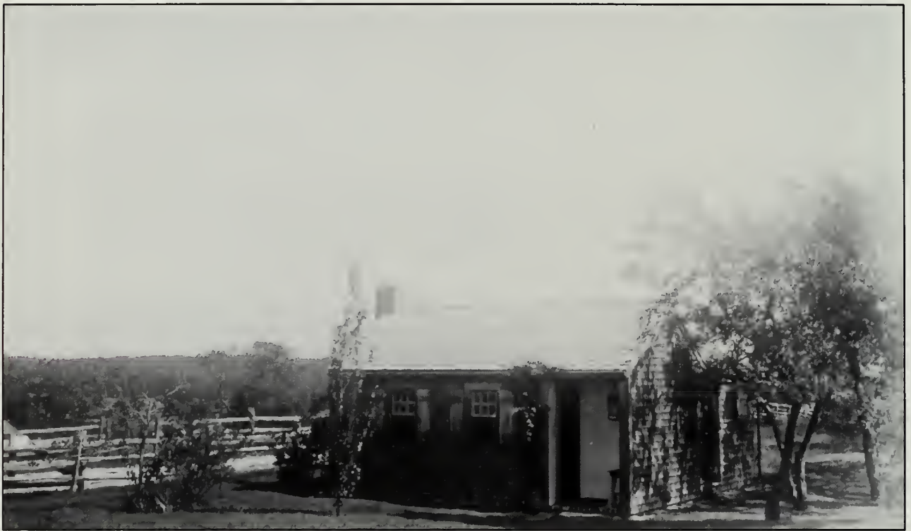
Figure 215. Guest House as originally constructed in 1929 (GKH Journal, p. 77).
