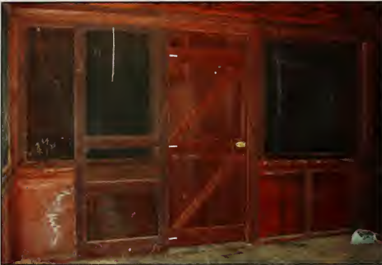
Figure 468. East wall inside Summer House (2007).
