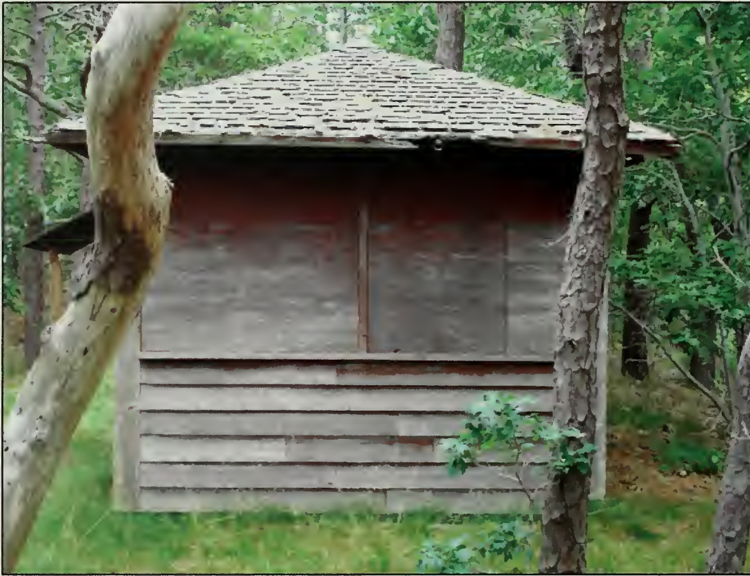
Figure 451. South elevation, Summer House (2007).
