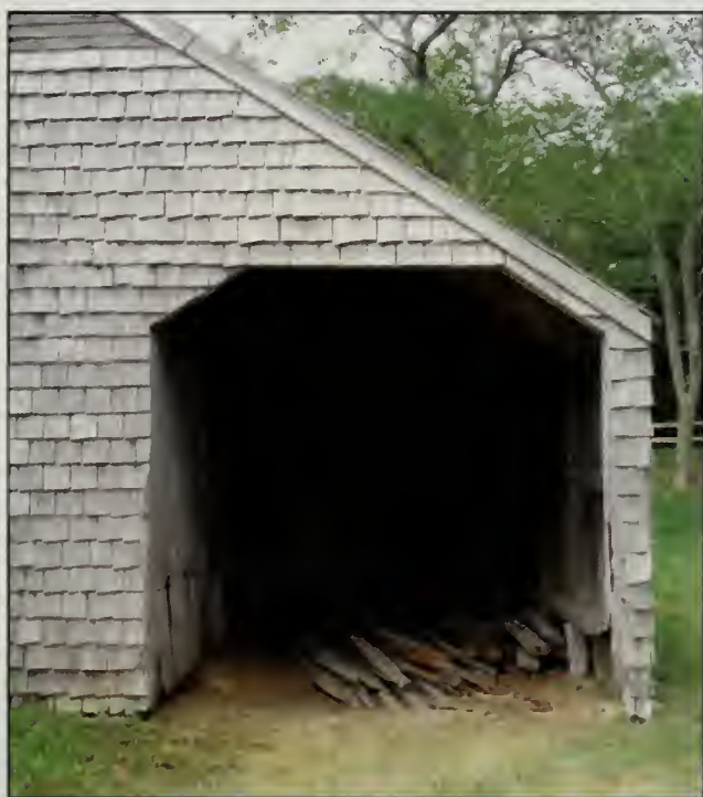
Figure 293. D104 in east elevation, Barn (2007).
