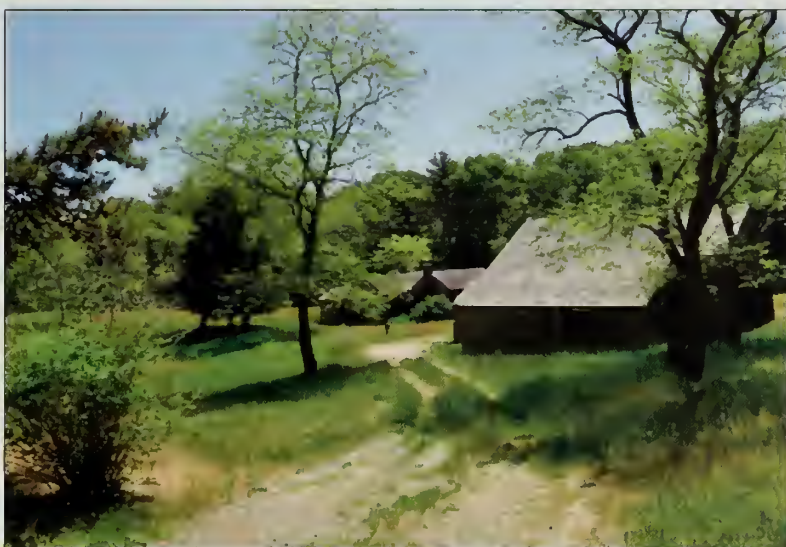
Figure 88. Looking southeast to the Barn with the Guest House and privy beyond, from near the entrance to the building complex. (OCLP, June 2010.)
