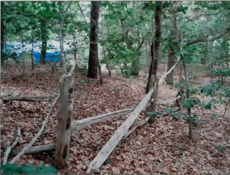
Figure 105. Fence corner turning north to the southwest of the Garage, July 2007 (OCLP).
