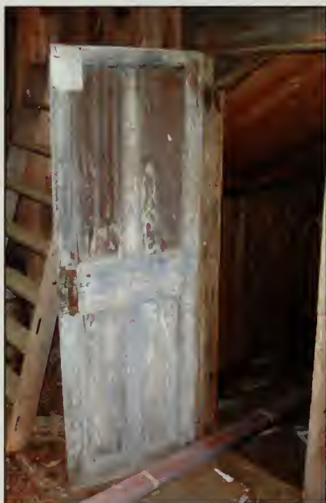
Figure 335. D111 in east wall of Carriage Room (leads to Shed), Barn (2007).
