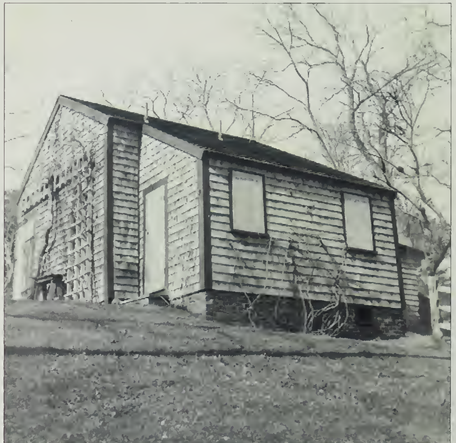
Figure 40. Looking northwest at the Woodshed and fence, in a photo taken for the 1973 Historic Structure Report on the Atwood-Higgins building complex. (Cape Cod NS archives.)
