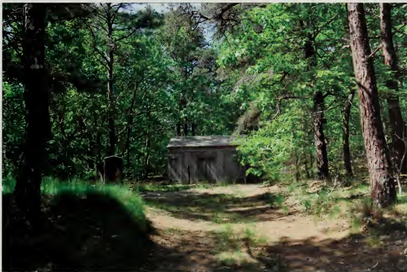
Figure 163. Looking west at the new Garage, May 2010. (OCLP)
