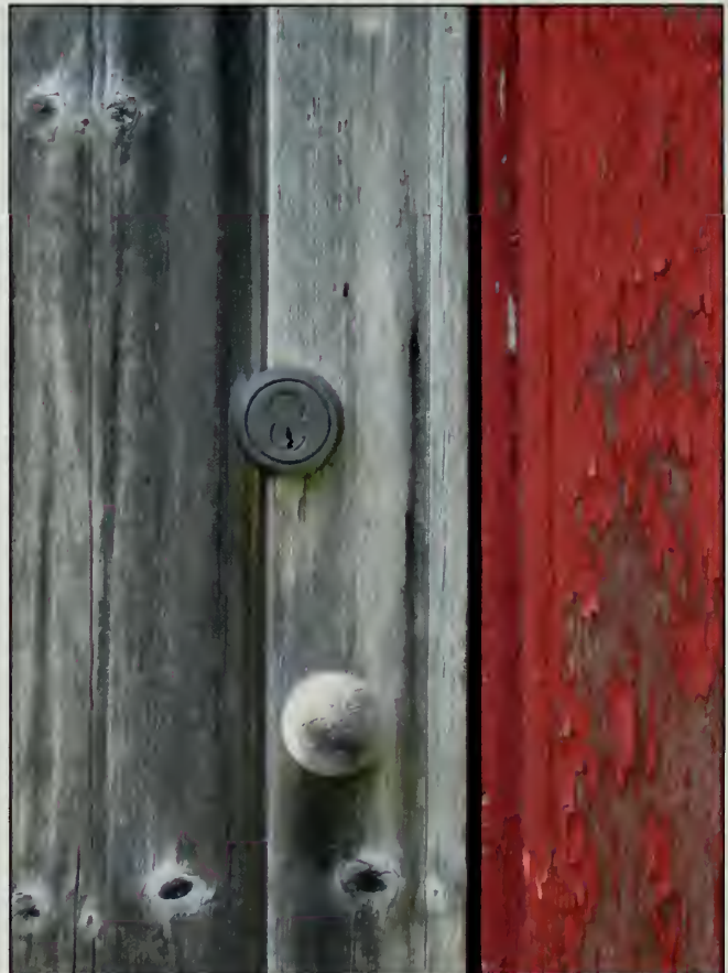
Figure 365. Hardware on door within D103, south elevation, Guest House (2007).
