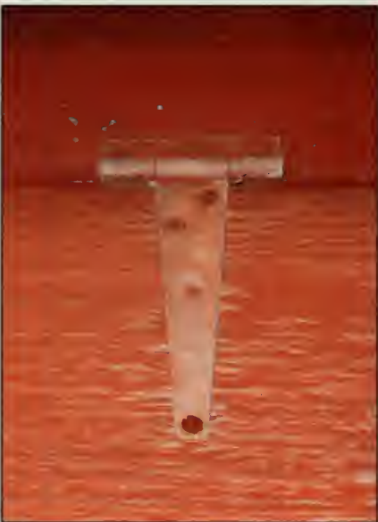
Figure 461. Typical metal strap hinge found on shutter on exterior window, Summer House (2007).
