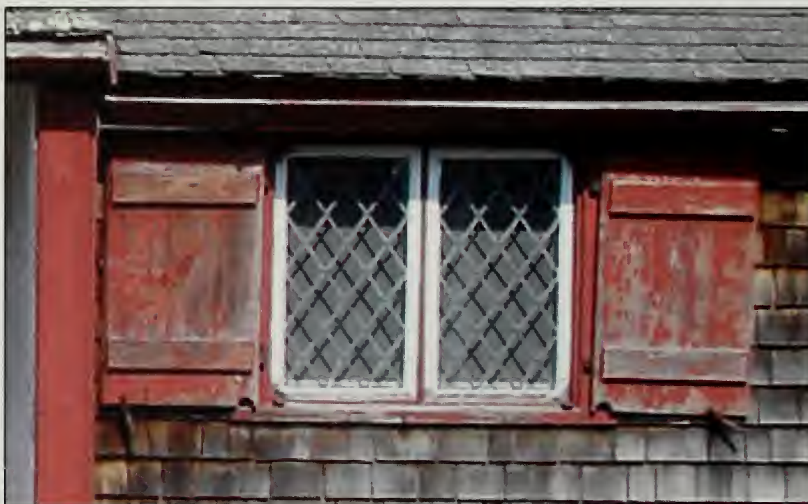
Figure 370. W104 in west elevation, Guest House (2007).
