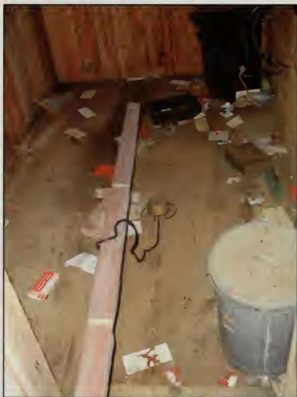
Figure 347. Floor of Shed, Barn (2007).
