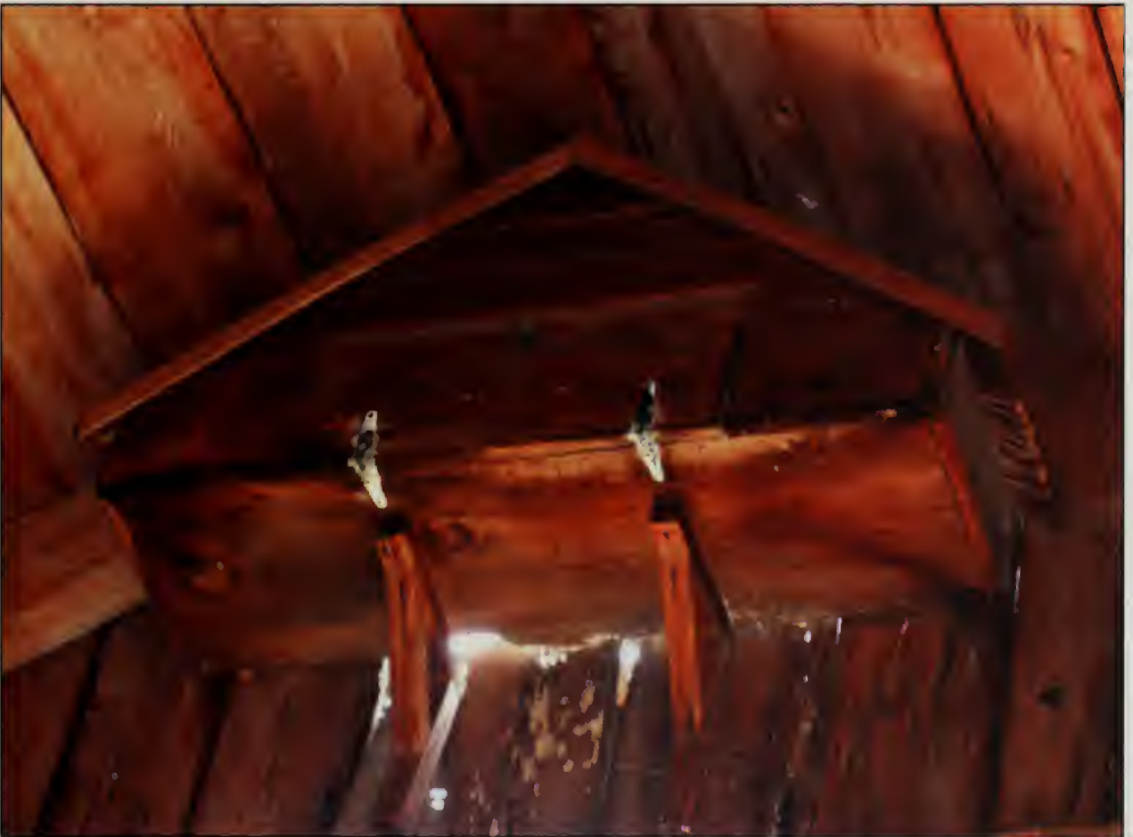
Figure 333. Built-in birdhouse, gable peak of east wall in Carriage Room, Barn (2007).
