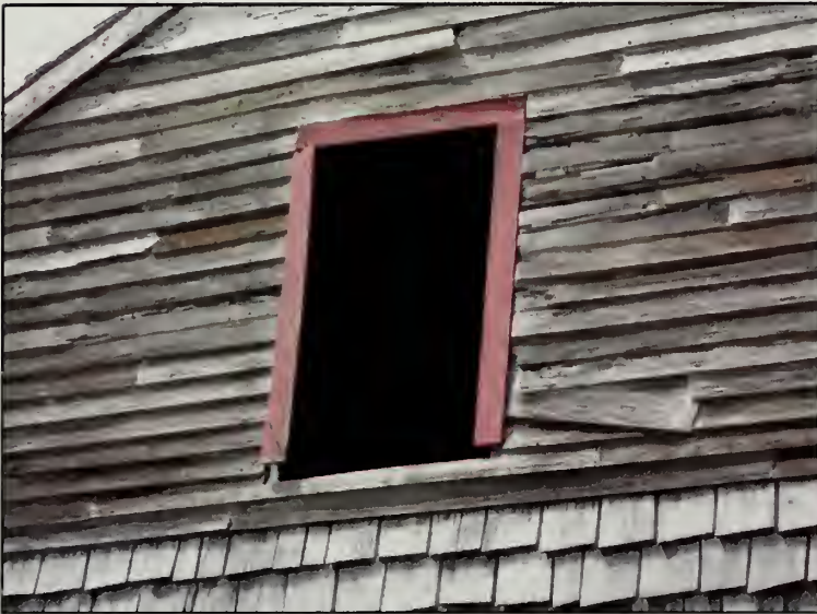
Figure 298. W104 in east elevation, Barn (2007).
