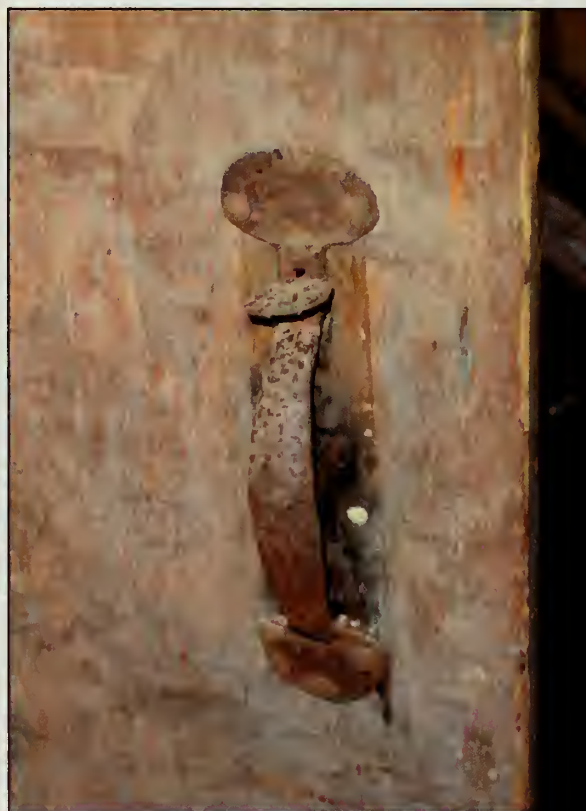
Figure 323. Iron thumb latch of door within D108, Harness, Barn (2007).
