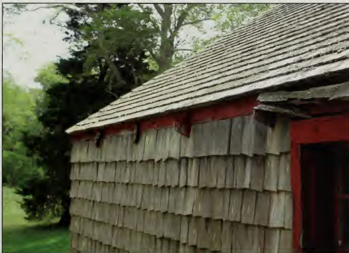
Figure 305. Gutter brackets on eastern end of north elevation, Barn (2007).
