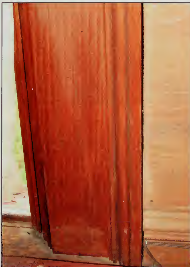
Figure 398. Interior trim surrounding windows in Living Room, Guest House (2007).
