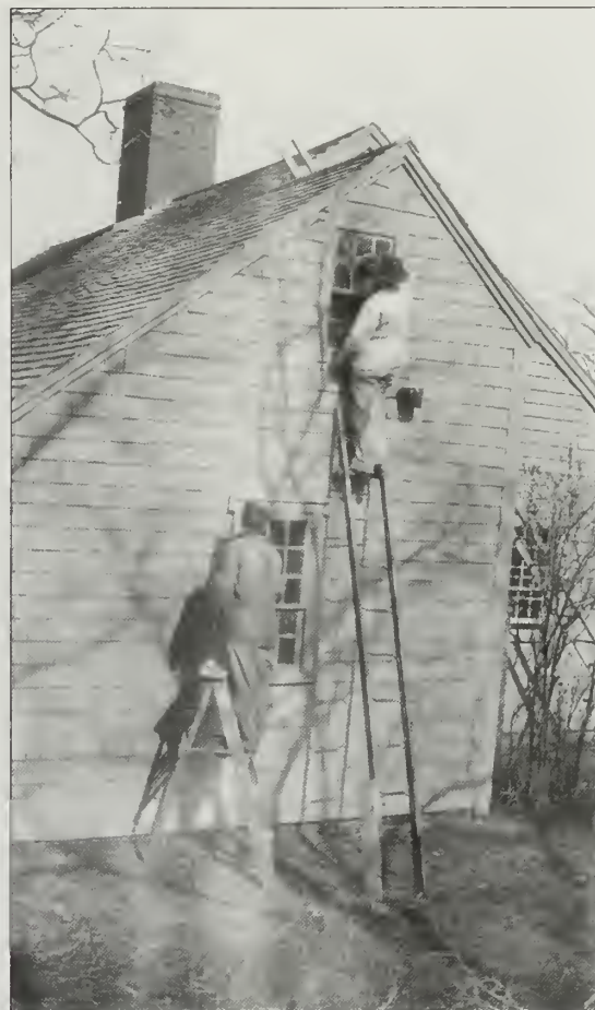
Figure 126. Two workmen applying the first coat of paint to the west side of the Atwood-Higgins House in 1920. Note the lilac at right. (Cape Cod NS archives.)
