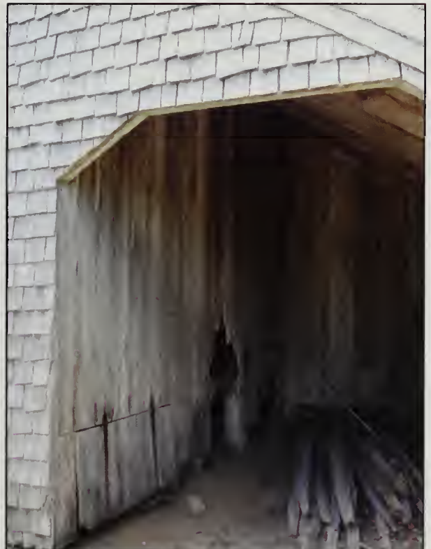
Figure 345. South wall of Open Shed, Barn (2007).
