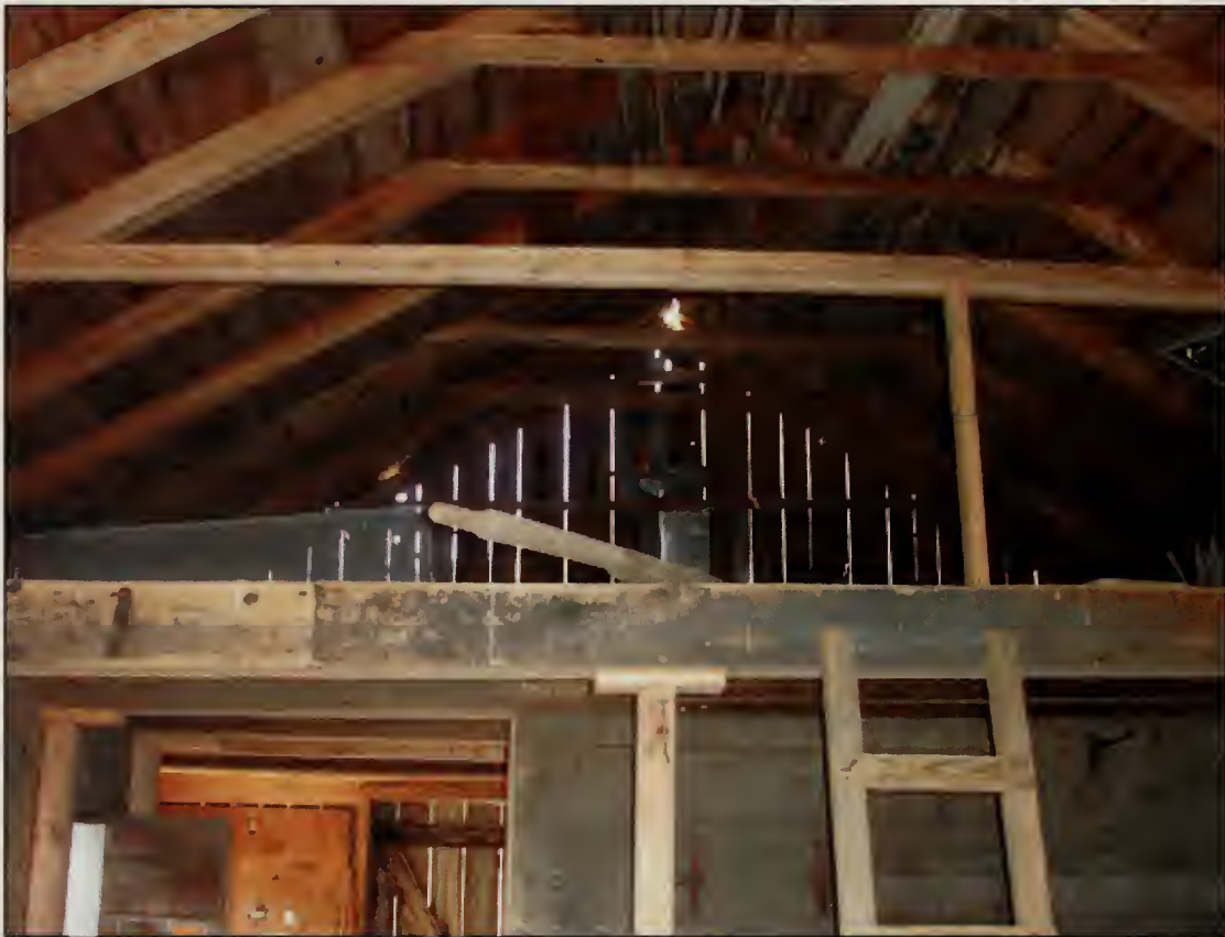
Figure 353. Loft of Barn (2007).
