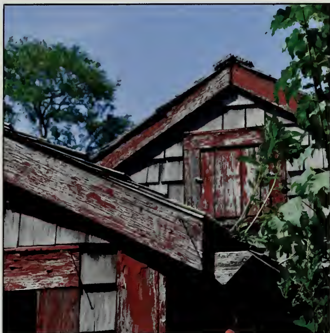
Figure 371. W105 in south elevation, Guest House (OCLP, 2010).
