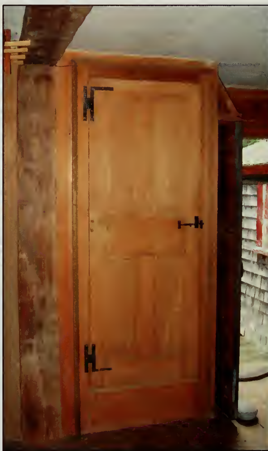
Figure 521. D107 in west wall of Country Store Room, Country Store (2007).
