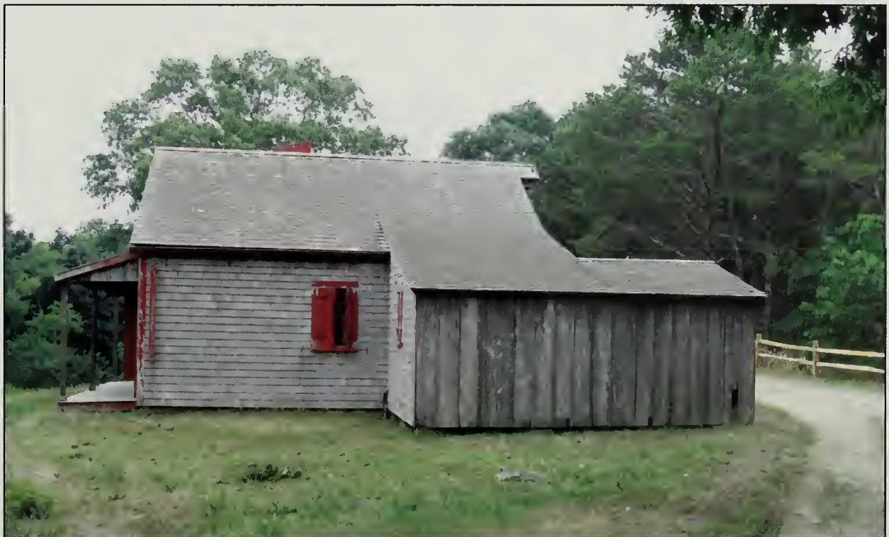
Figure 472. North elevation, Country Store (2007).
