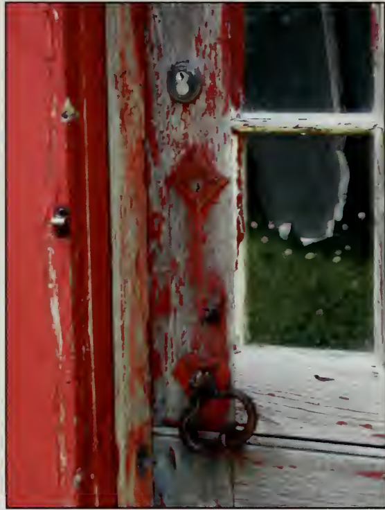
Figure 363. Hardware on door within D102, south elevation, Guest House (2007).
