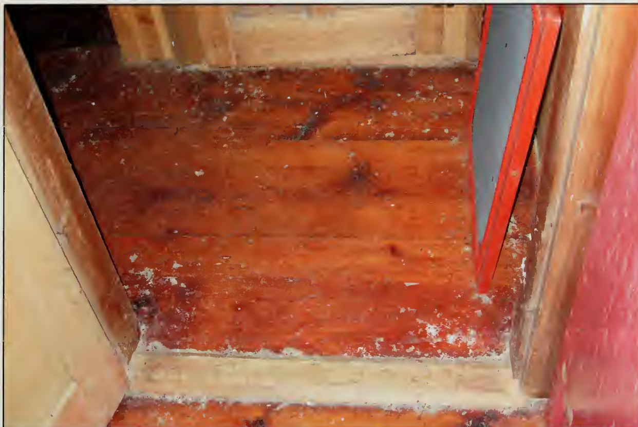
Figure 432. Floor of Closet, Guest House (2007).
