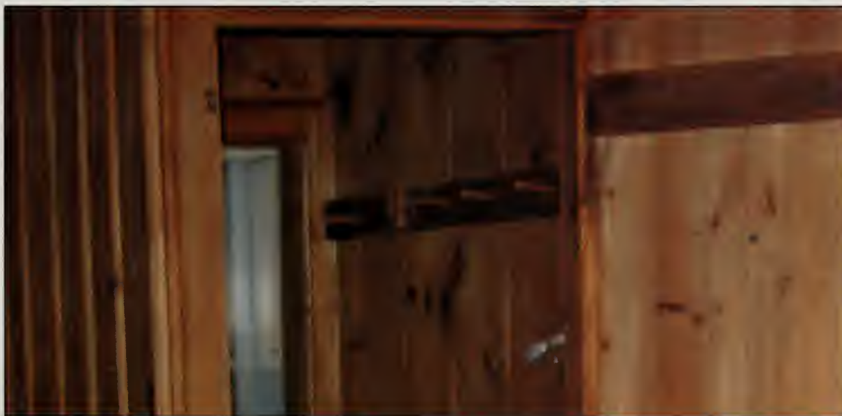
Figure 439. Wooden pegs on west wall of Hallway, Guest House (2007).
