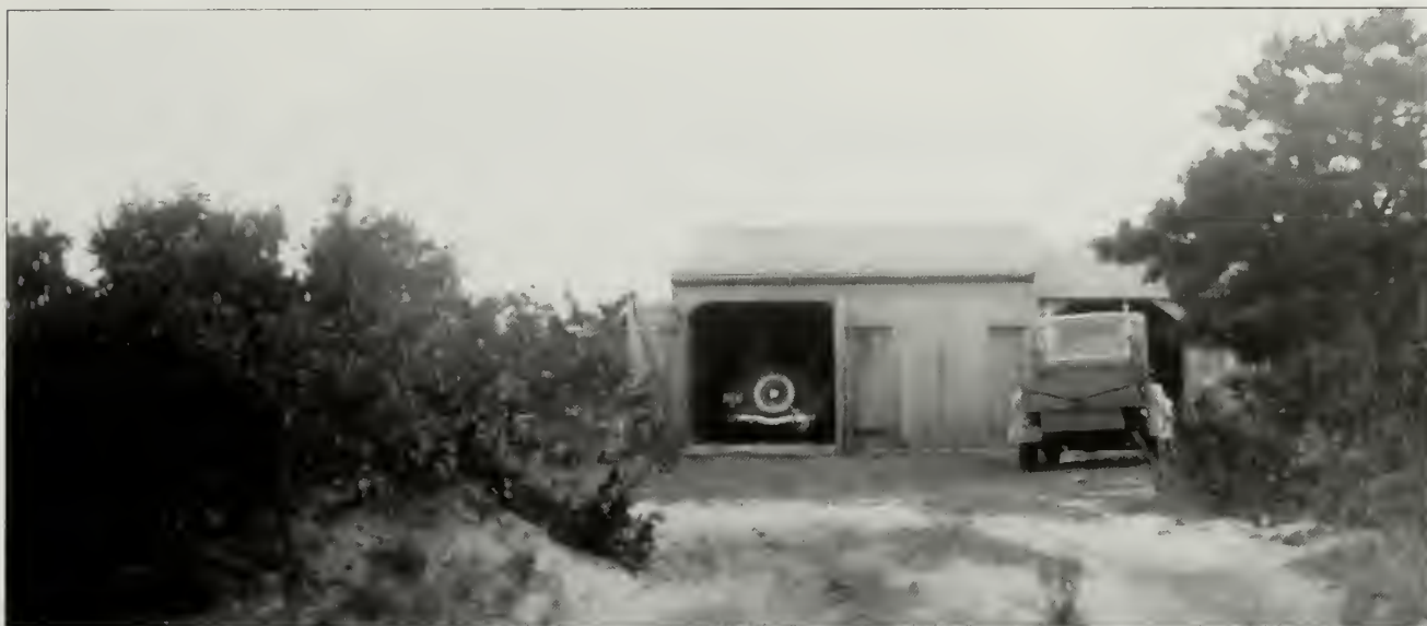
Figure 162. Looking west at the new Garage, 1929. (Cape Cod NS archives.)
