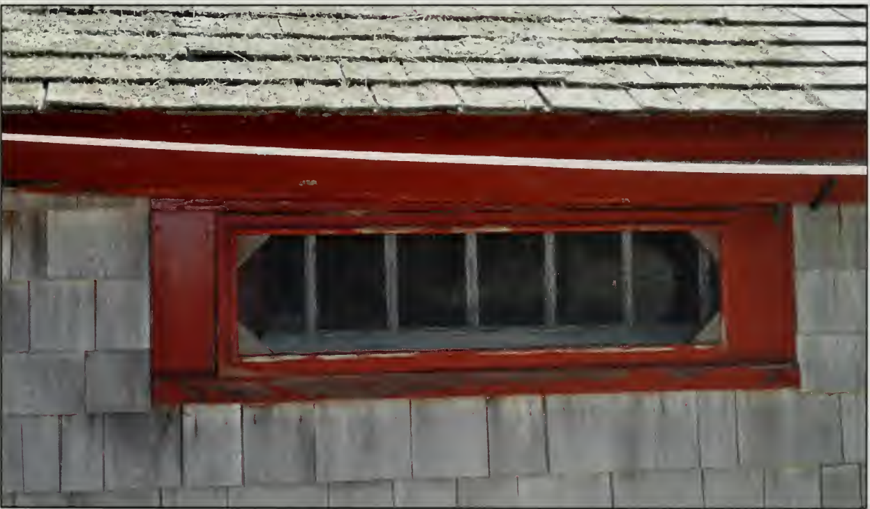
Figure 379. W114 in north elevation, Guest House (OCLP, 2010).
