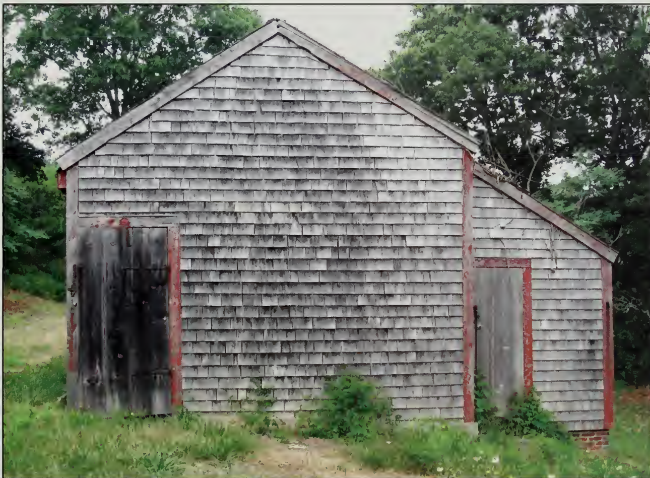
Figure 229. South elevation, Woodshed (2007).
