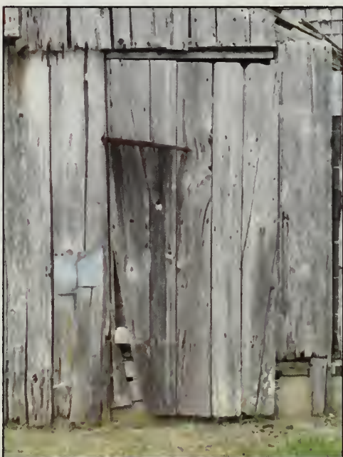
Figure 291. D103 in east elevation, Barn (2007).
