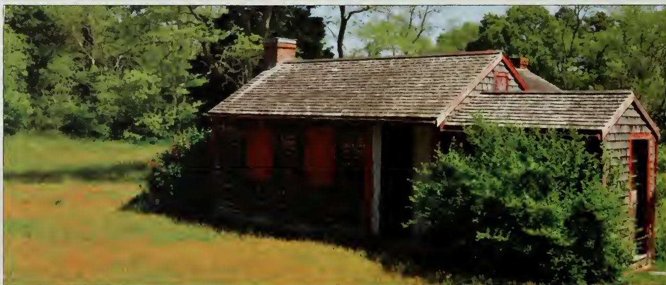
Figure 157. Looking northeast at the Guest House, May 2010. (OCLP)
