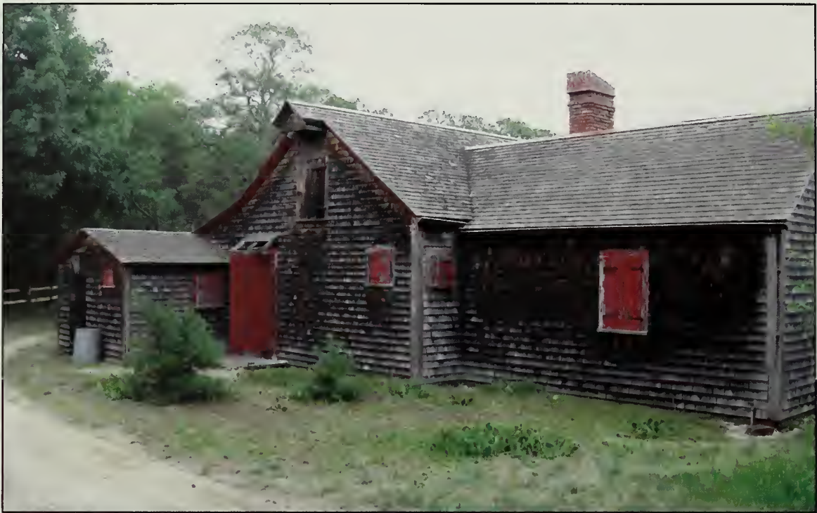
Figure 473. West elevation, Country Store (2007).
