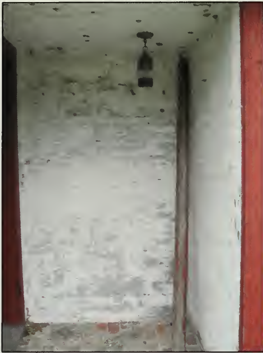
Figure 386. South and east walls of Entry, Guest House (2007).
