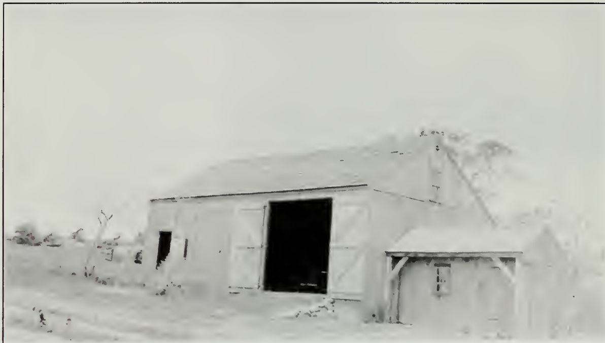
Figure 213. Barn prior to the addition of siding on the east elevation (siding added in 1930). (CACO AH File Drawer).
