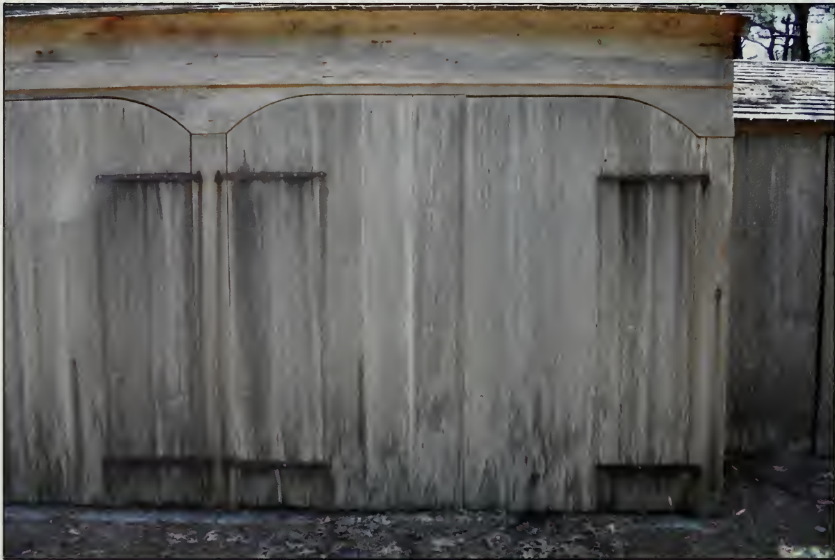
Figure 262. D102 in northeast elevation, Garage (OCLP, 2010).
