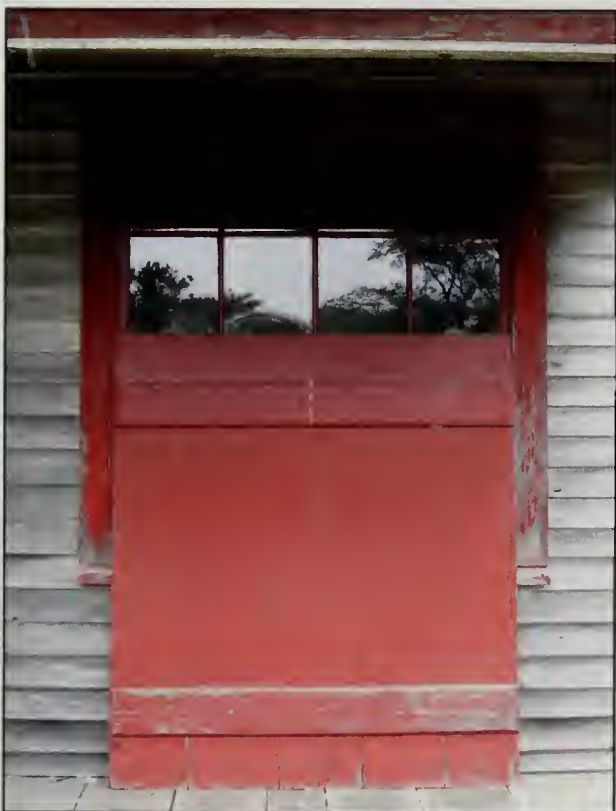
Figure 488. W103 in east elevation, Country Store (2007).
