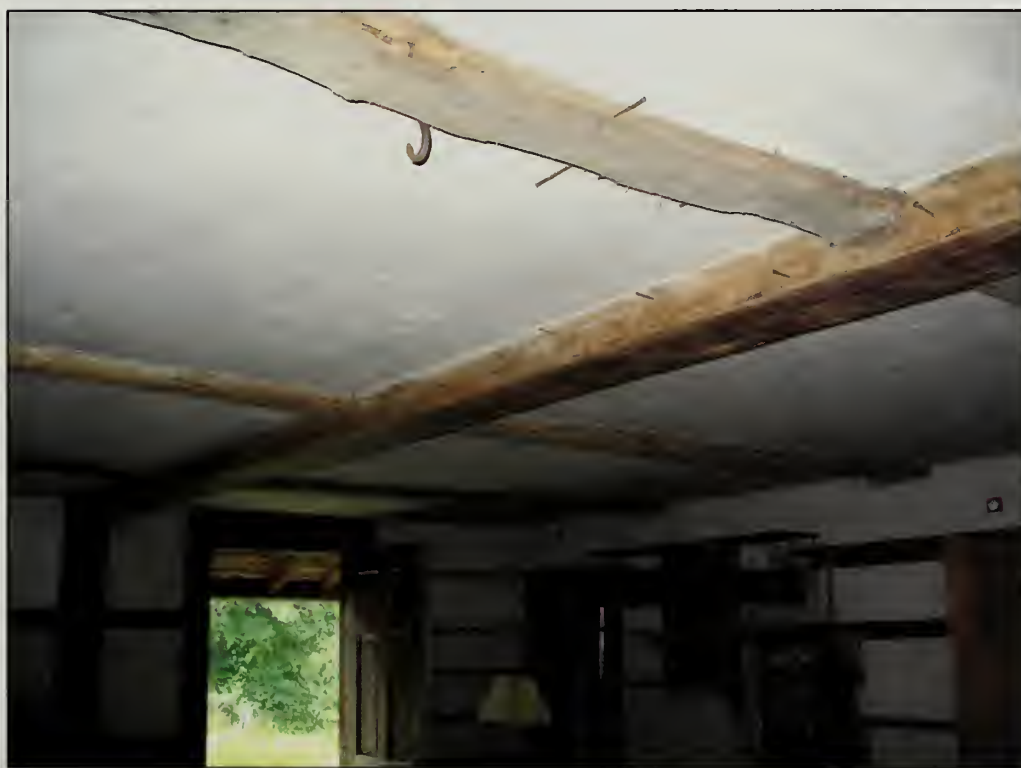
Figure 524. Ceiling of Country Store Room, Country Store (2007).
