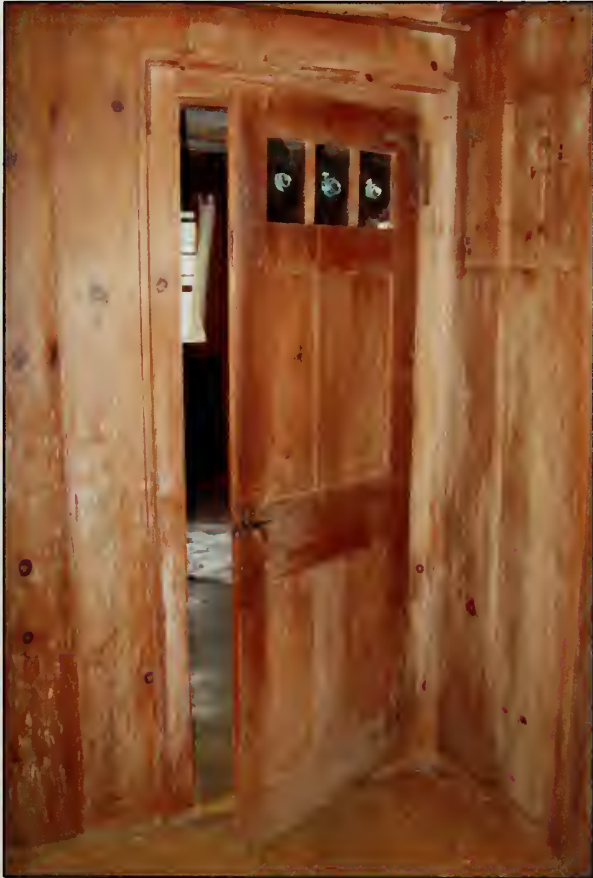
Figure 409. D106 in South Bedroom (leads into Living Room), Guest House (2007).
