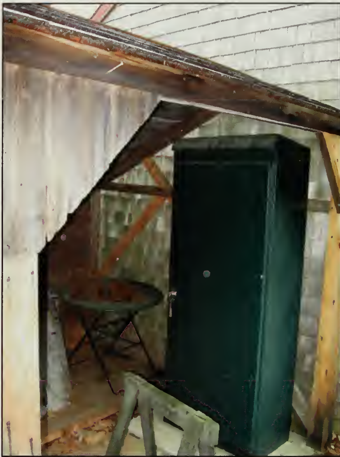
Figure 251. South wall in Woodshed addition, Woodshed (2007).
