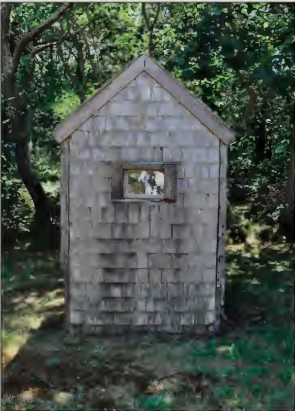
Figure 537. North elevation, Guest House Privy (OCLP, August 2010).
