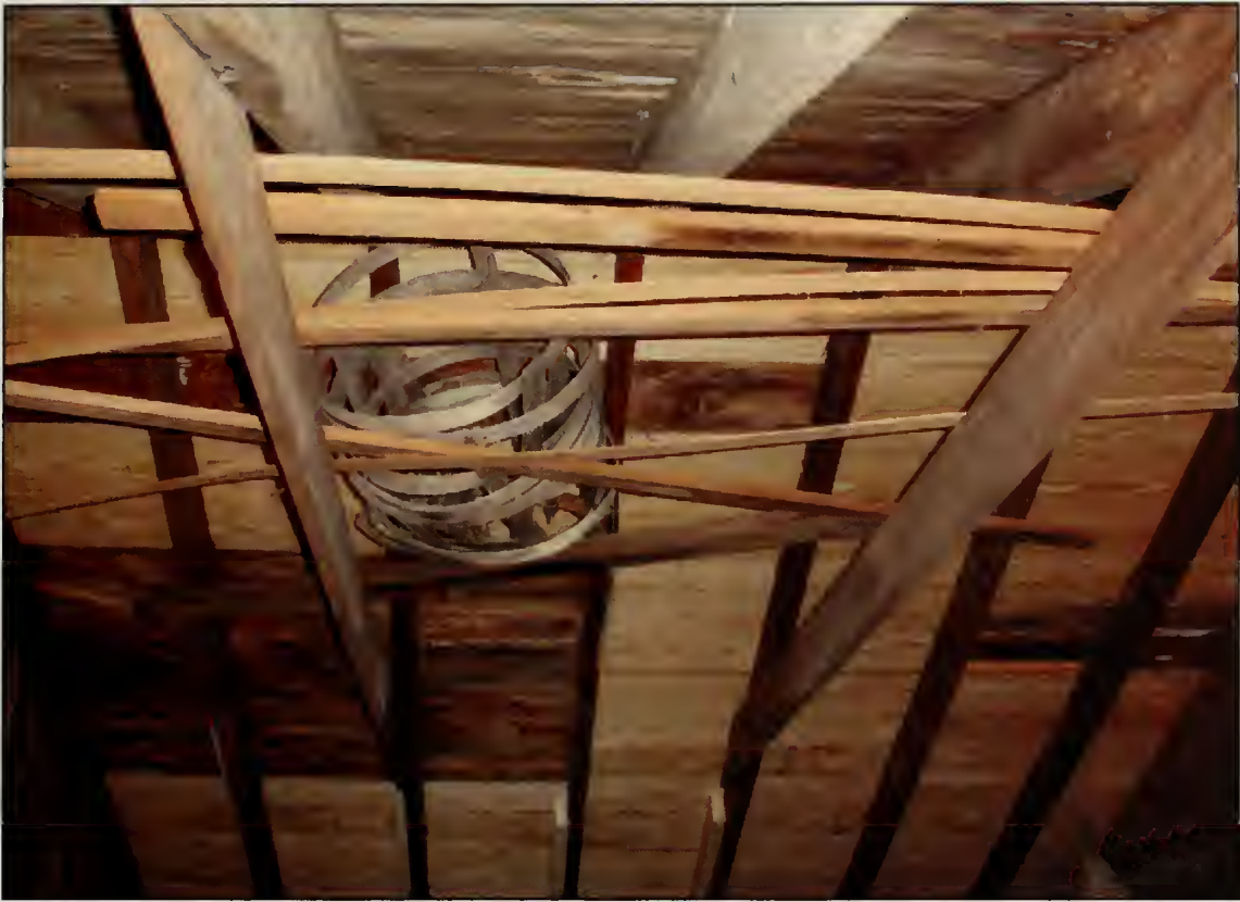
Figure 279. Exposed roofing system of Room 102, Garage (2007).
