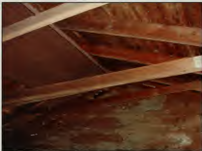
Figure 272. Ceiling of Room 101, Garage (2007).
