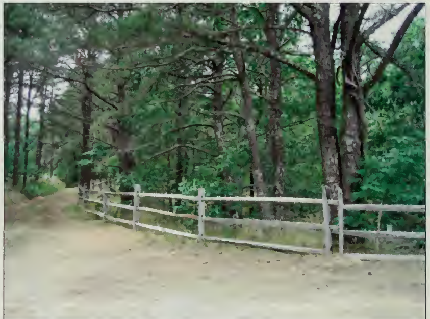
Figure 103. Old Town Road leading away from the building complex, west of the Country Store, to the Garage concealed behind the slope at left. Note the original fence with three rails, which was repaired in June 2007, and the small green pipe at right. (OCLP, July 2007.)
