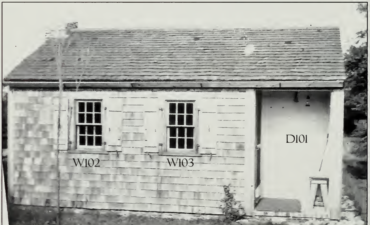
Figure 216. West elevation of Guest House as originally constructed in 1929, showing the locations of W102, W103, and D101 (GKH Scrapbook).
