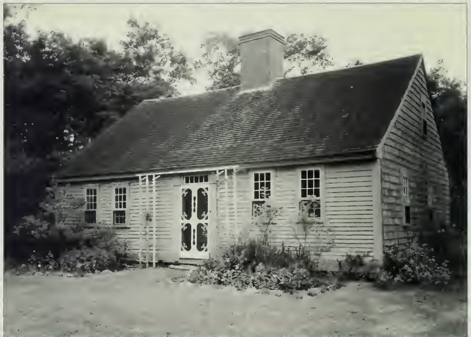
Figure 124. Looking northwest at the Atwood-Higgins House on August 6, 1959. Note the carefully tended flower beds and lawn. The hillside beyond supports several trees. (Cape Cod NS archives, H6-008.)
