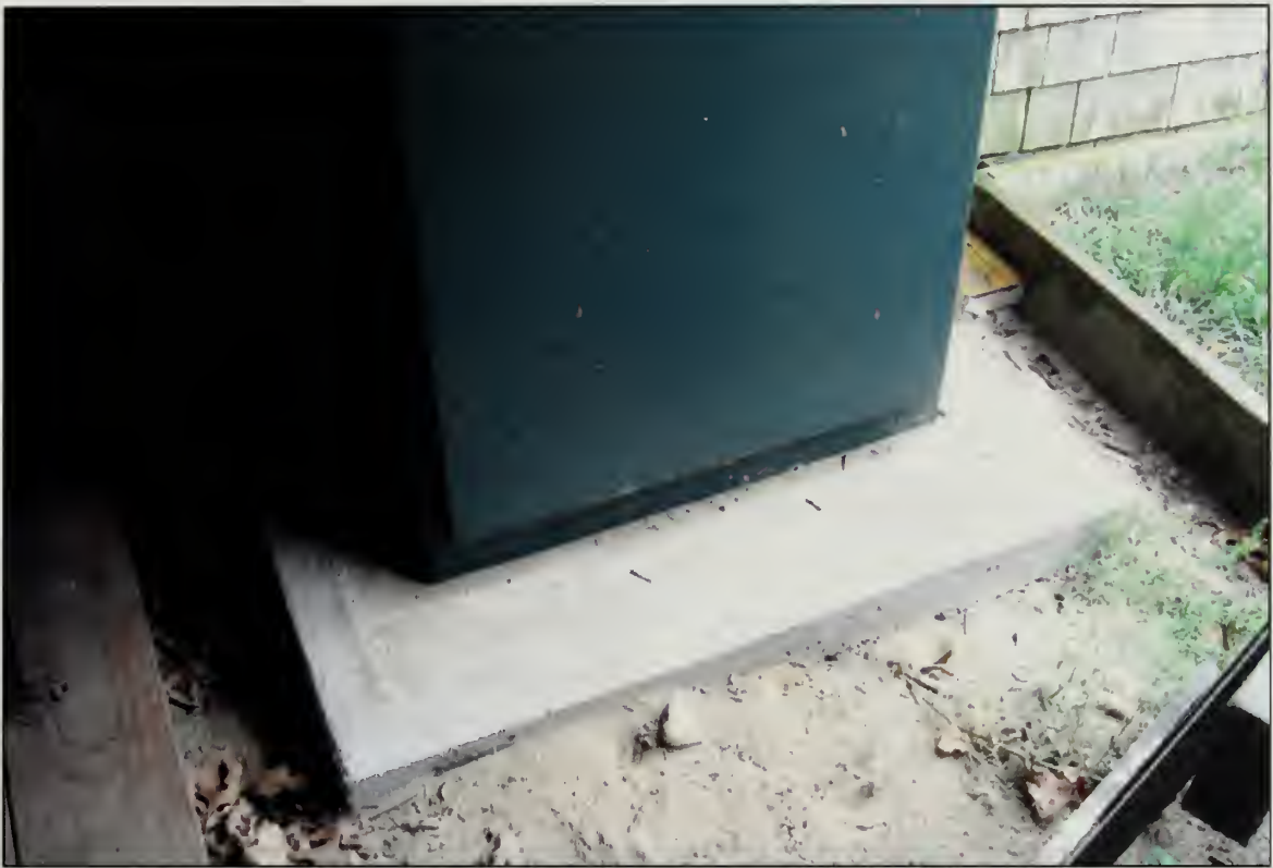
Figure 253. Concrete Slab in Woodshed addition, Woodshed (2007).
