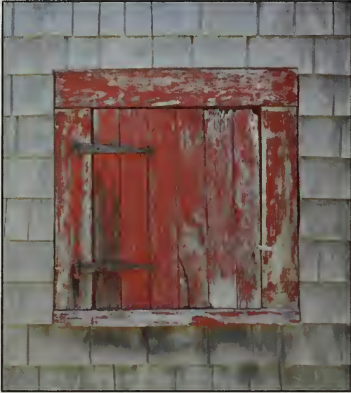
Figure 375. W110 in east elevation, Guest House (OCLP, 2010).
