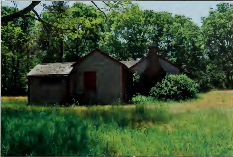
Figure 93. North side of the Guest House. Note the Norway maple, lilac, and day lilies growing along the foundation. (OCLP, June 2010.)
