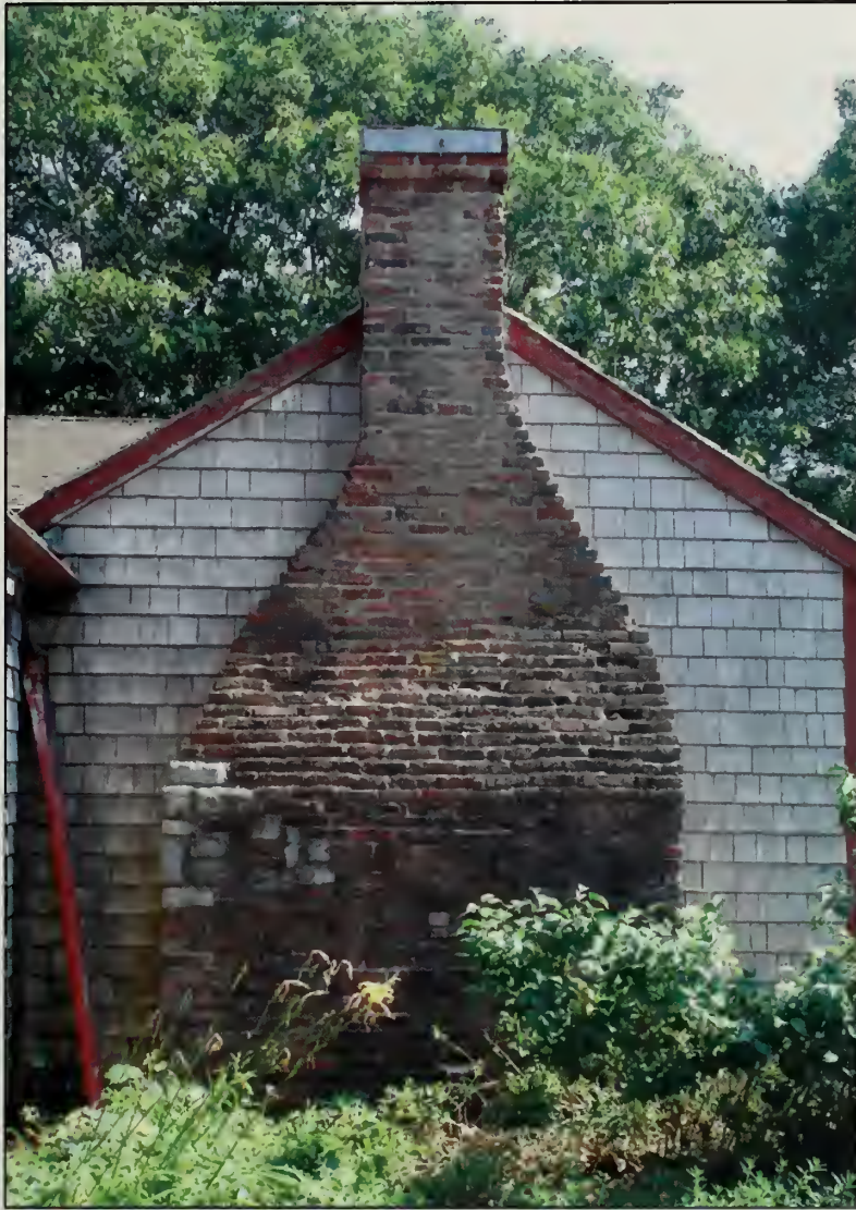
Figure 384. Chimney on north elevation, Guest House (2007).
