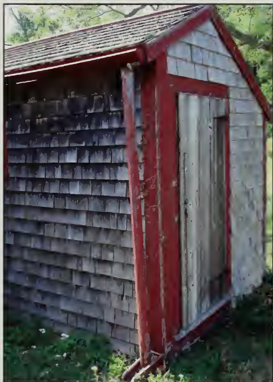
Figure 382. Downspout on exterior northeast corner of the Closet, Guest House (2007).
