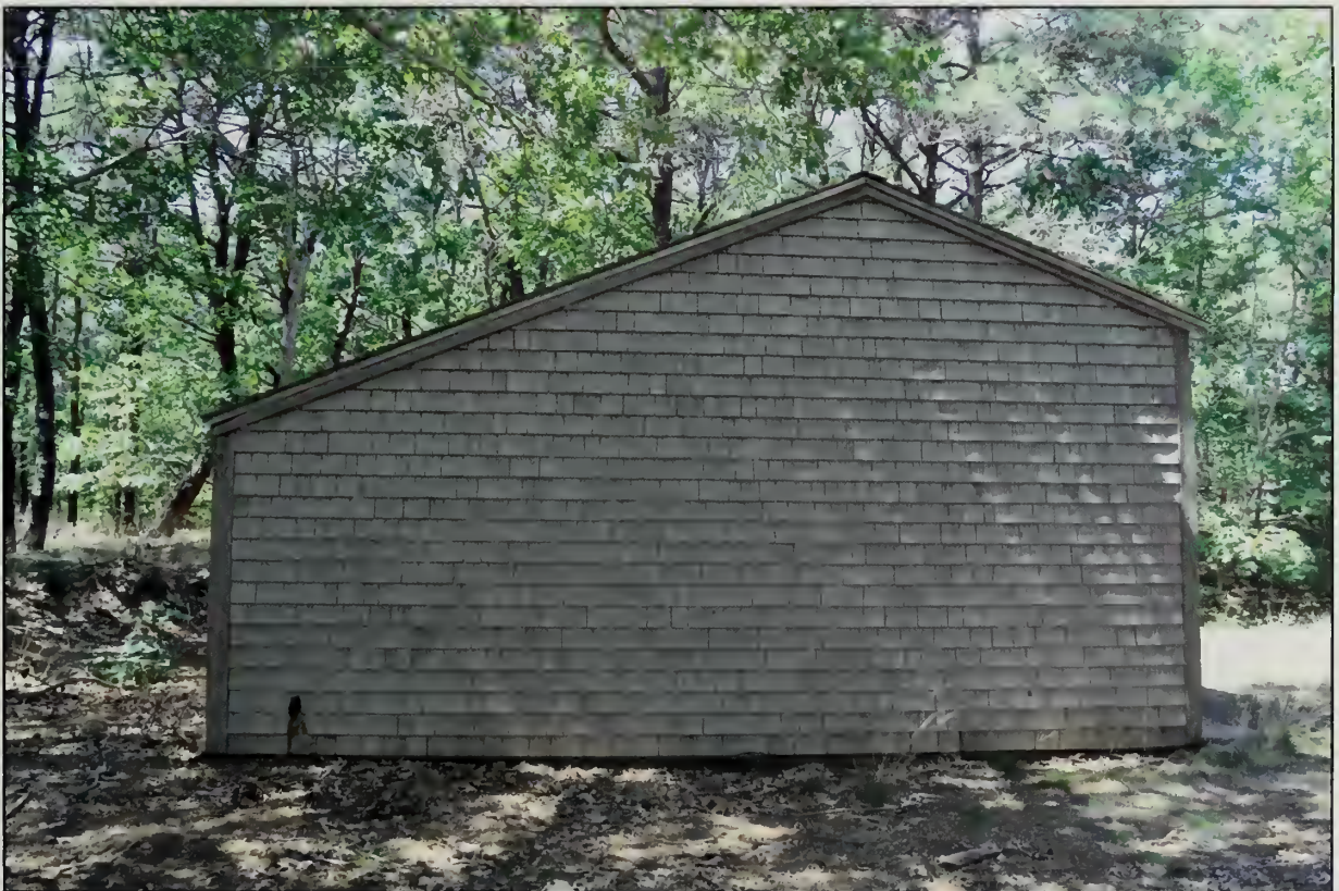
Figure 257. Southeast elevation, Garage (OCLP, 2010).
