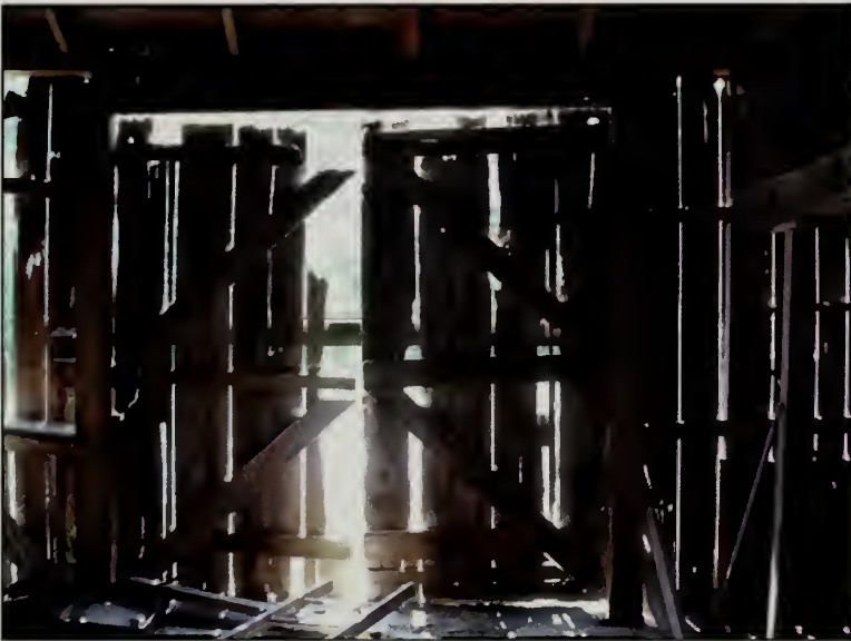
Figure 326. South wall and D102 of Carriage Room, Barn (2007).
