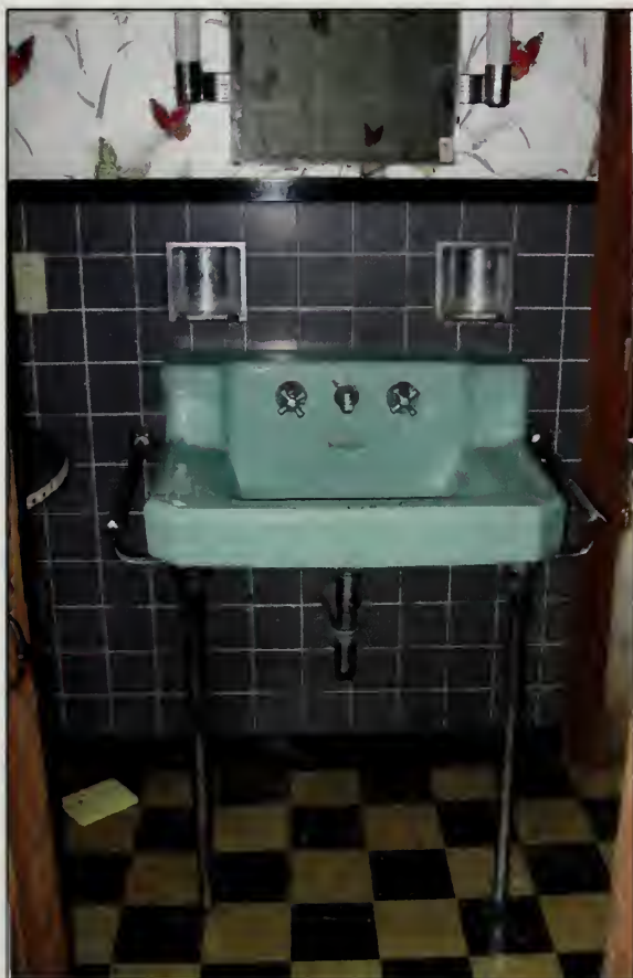
Figure 421. Console table sink on south wall of Bath, Guest House (2007).
