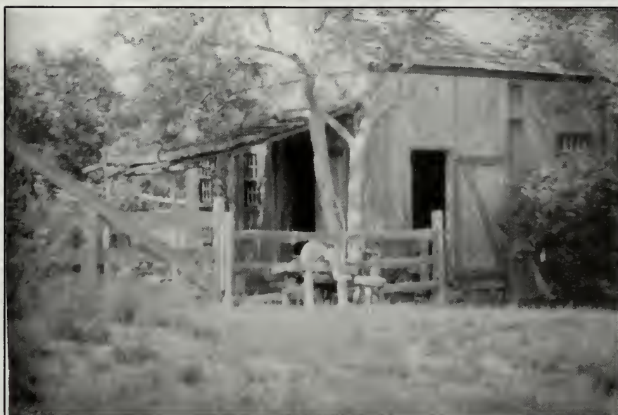
Figure 212. West side elevation of Barn depicting the lean-to open porch roof addition constructed in 1928. (GKH Journal, p. 71).
