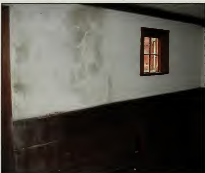
Figure 424. West wall of North Bedroom, Guest House (2007).
