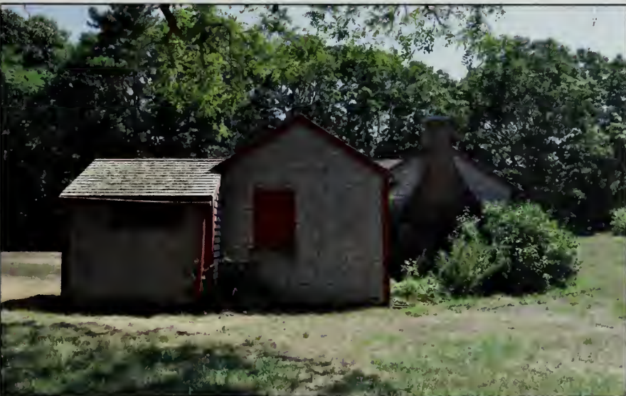
Figure 357. North elevation, Guest House (OCLP, 2010).
