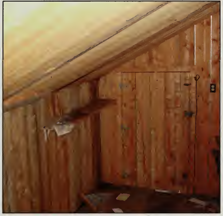
Figure 350. Built-in shelf on north wall of Shed, Barn (2007).
