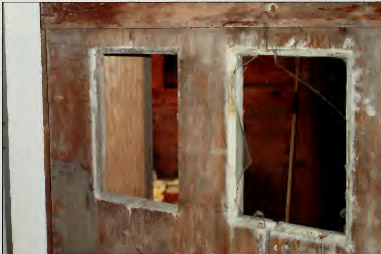
Figure 324. Two windows in door of D108, Harness, Barn (2007).
