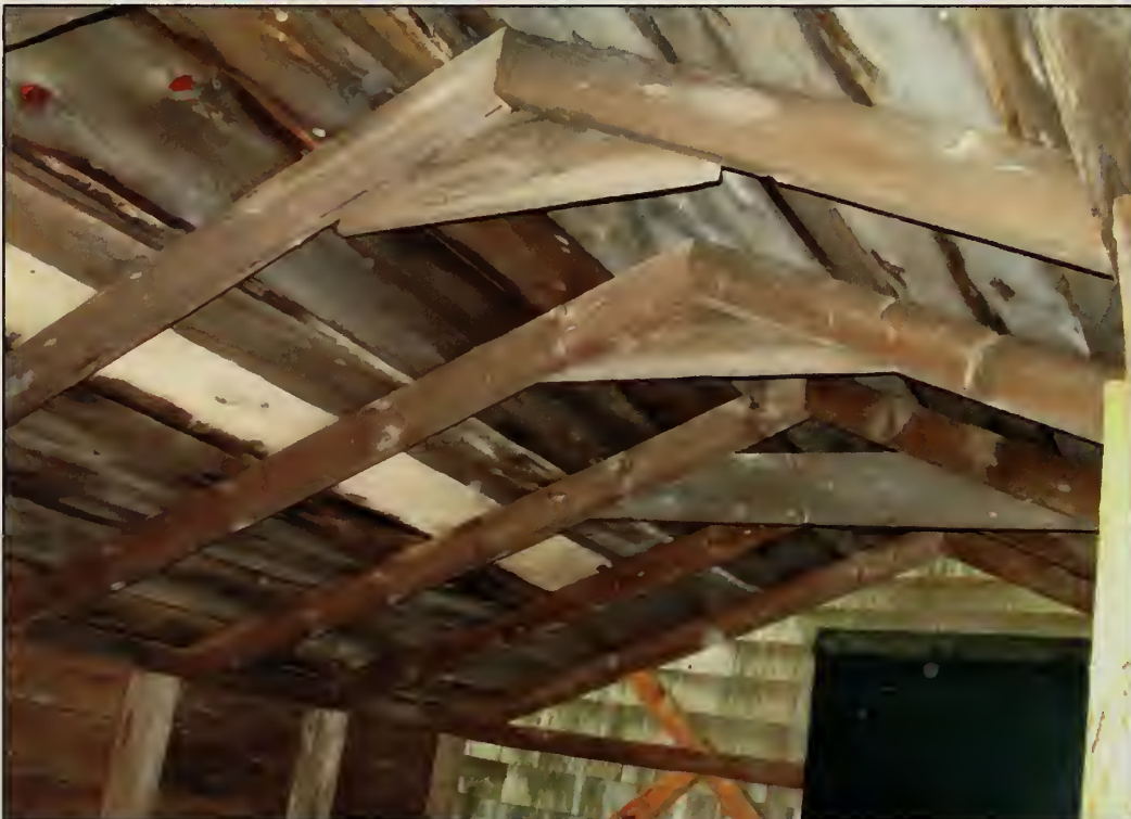
Figure 252. Ceiling in Woodshed addition, Woodshed (2007).
