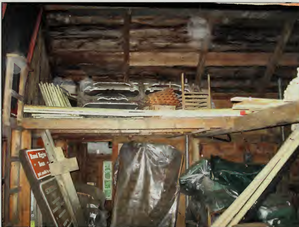
Figure 242. Loft on east wall in the Storage Room, Woodshed (2007).
