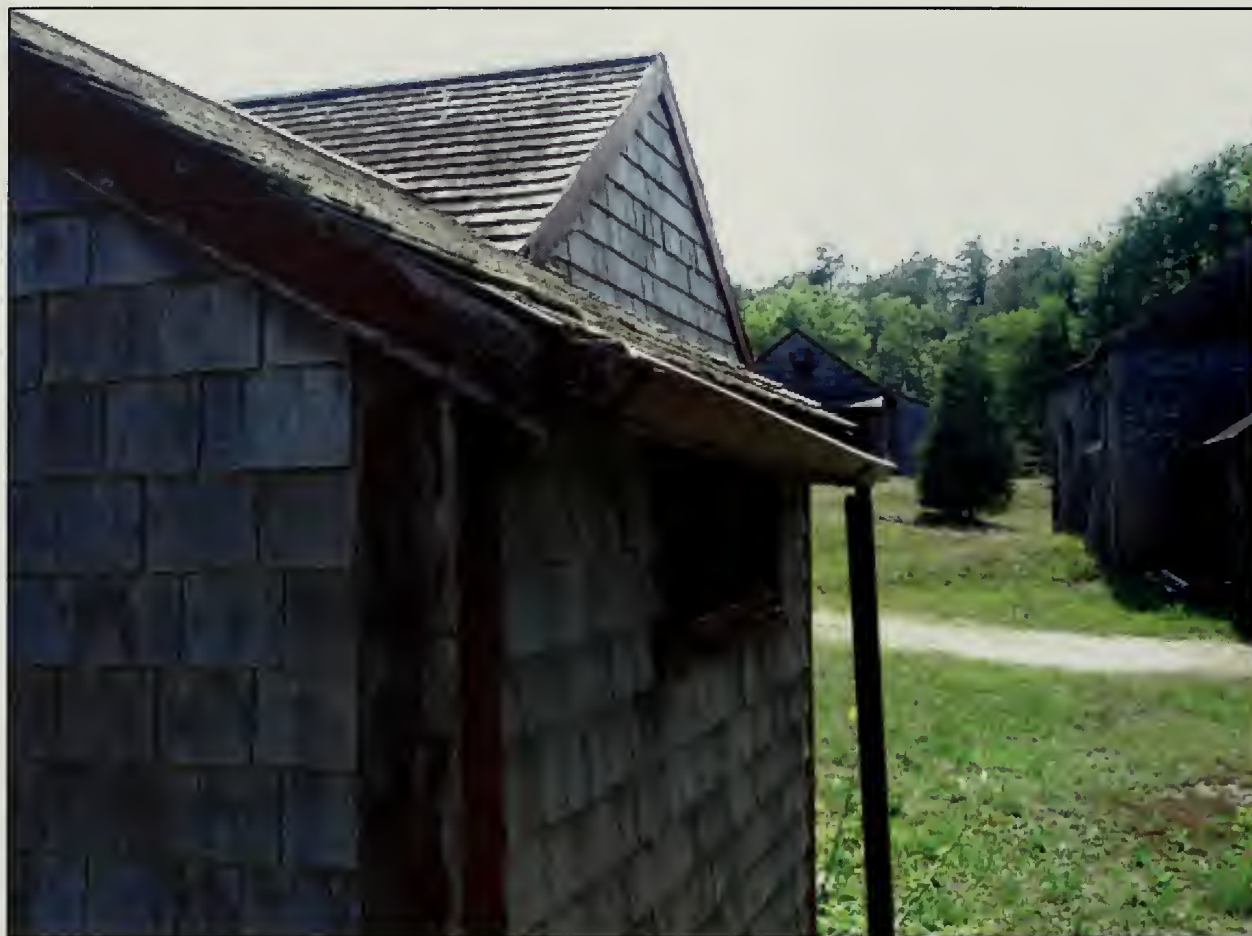
Figure 381. Gutter on north elevation, Guest House (2007).
