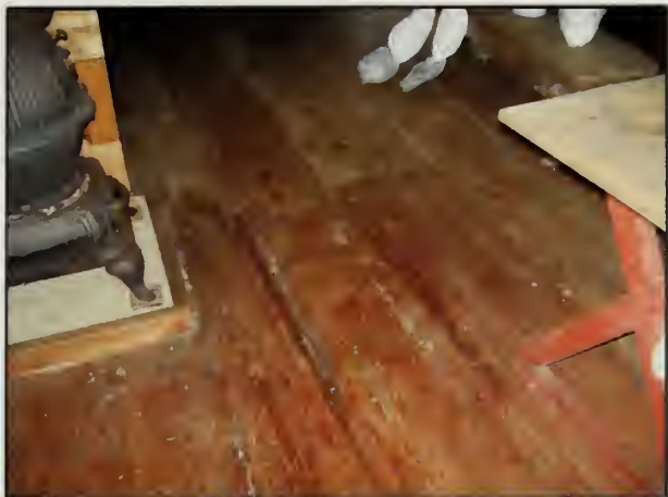
Figure 516. Floor of Country Store Room, Country Store (2007).
