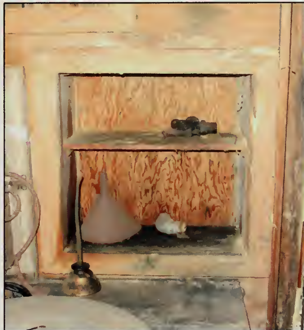
Figure 275. Built-in cabinet, northeast wall of Room 102, Garage (2007).
