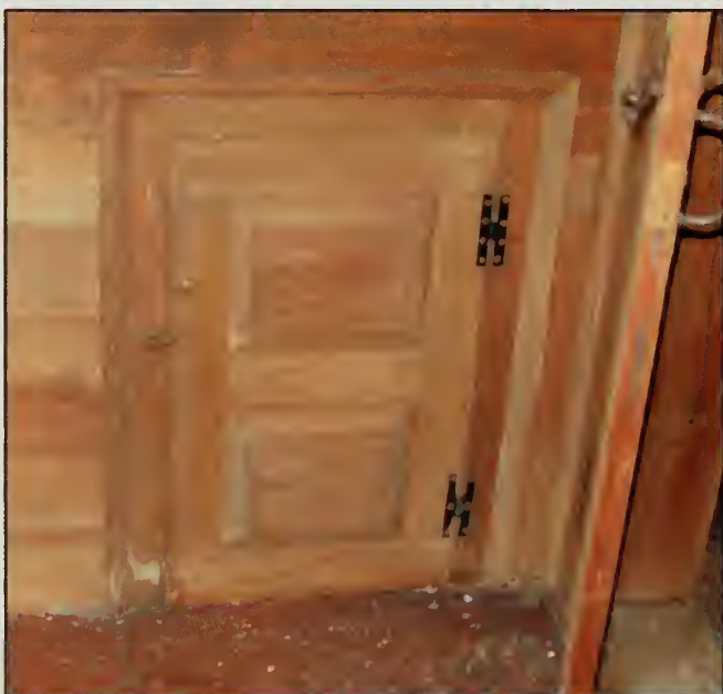
Figure 425. Built-in cabinet in lower half of west end of south wall in North Bedroom, Guest House.
