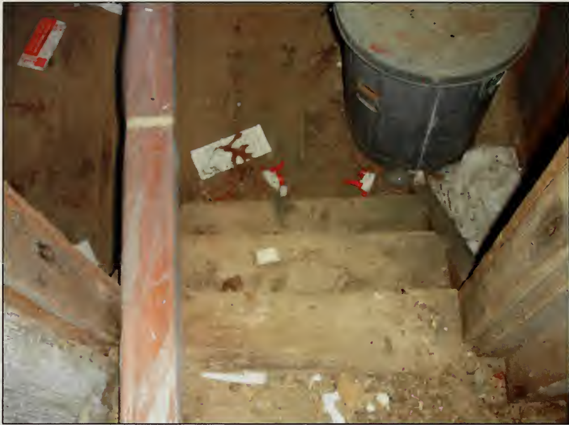
Figure 352. Stairs located below D111 in Shed, Barn (2007).
