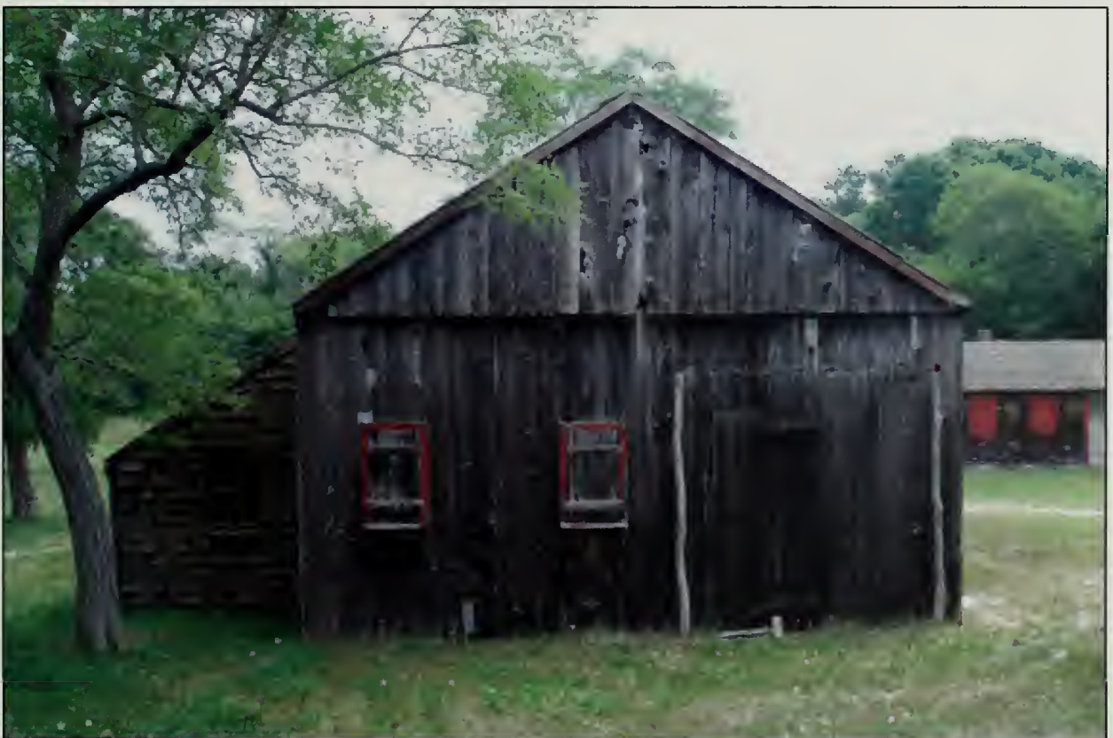
Figure 284. West elevation, Barn (2007).
