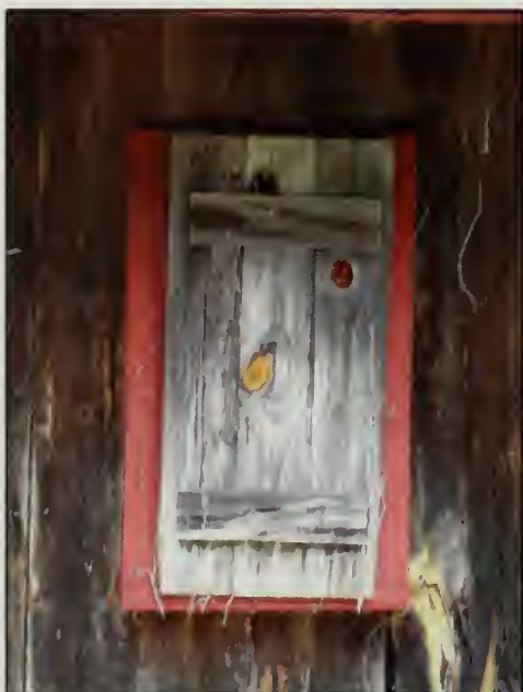
Figure 297. W103 in south elevation, Barn (2007).
