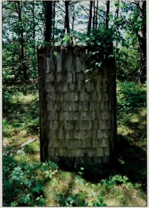
Figure 544. East elevation, Northeast Privy (OCLP, August 2010).
