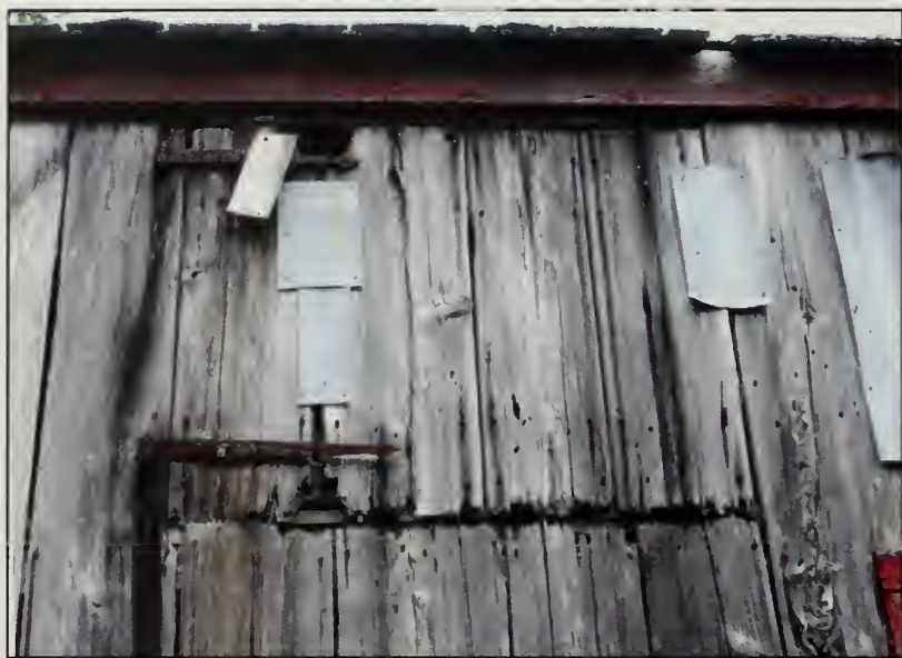
Figure 295. W101 in south elevation, Barn (2007).
