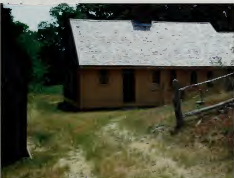
Figure 65. Slope with vegetation north of house at right. Note the post in the foreground, which is made of whalebone. (OCLP, June 2010.)
