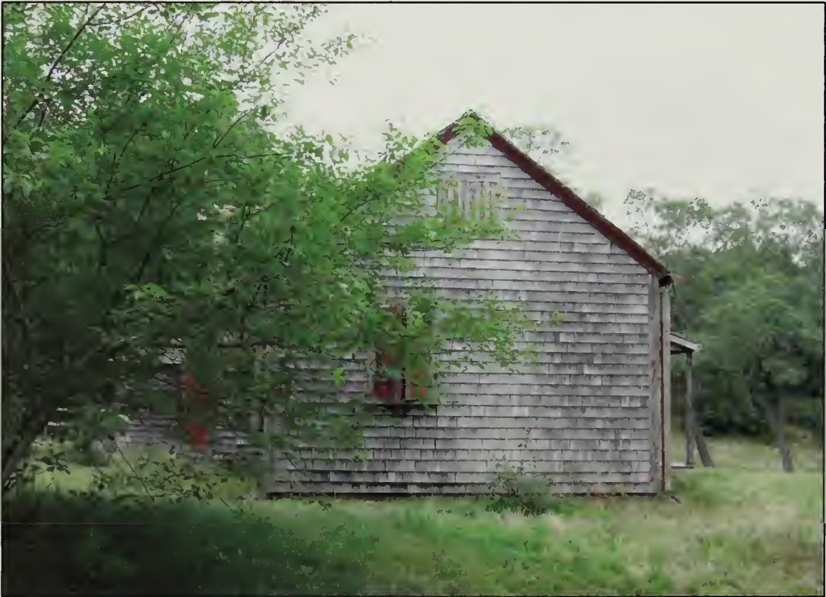
Figure 474. South elevation, Country Store (2007).
