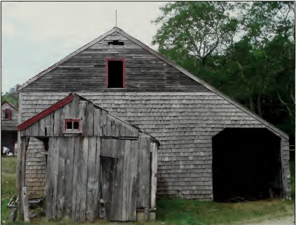
Figure 282. East elevation, Barn (2007).
