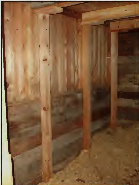
Figure 317. North wall of Box Stall, Barn (2007).
