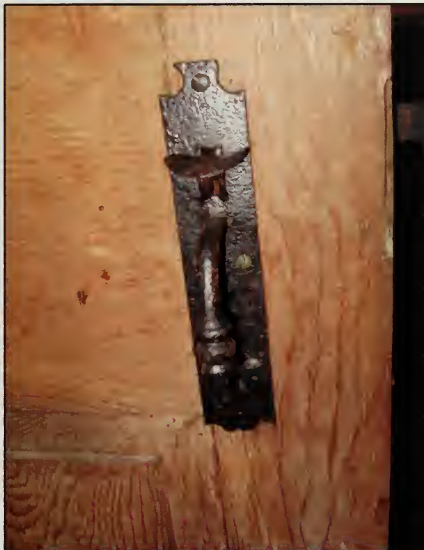
Figure 427. Iron thumb latch on North Bedroom side of door located within D110, Guest House (2007).
