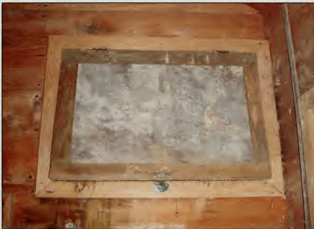
Figure 276. Built-in cabinet, northeast end of northwest wall, Room 102, Garage (2007).
