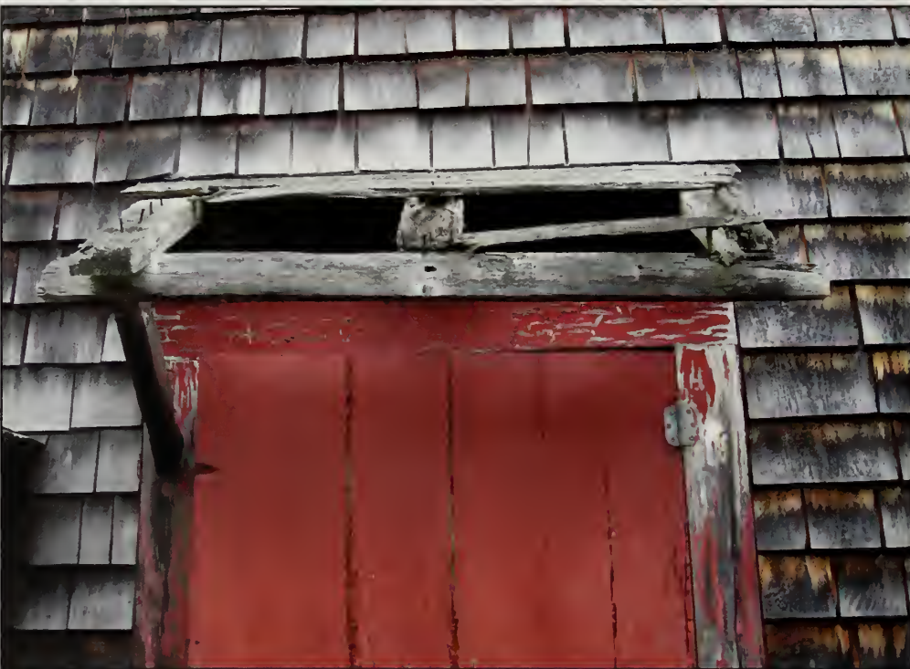
Figure 485. Shed roof over D104 on west elevation, Country Store (2007).
