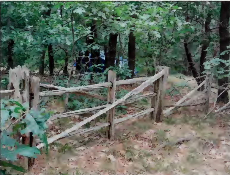
Figure 106. Fence gate to the northwest of the Garage. Note the hurdle-style design of both fences and gate. (OCLP, July 2007.)
