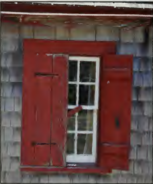
Figure 377. W112 in east elevation, Guest House (OCLP, 2010).
