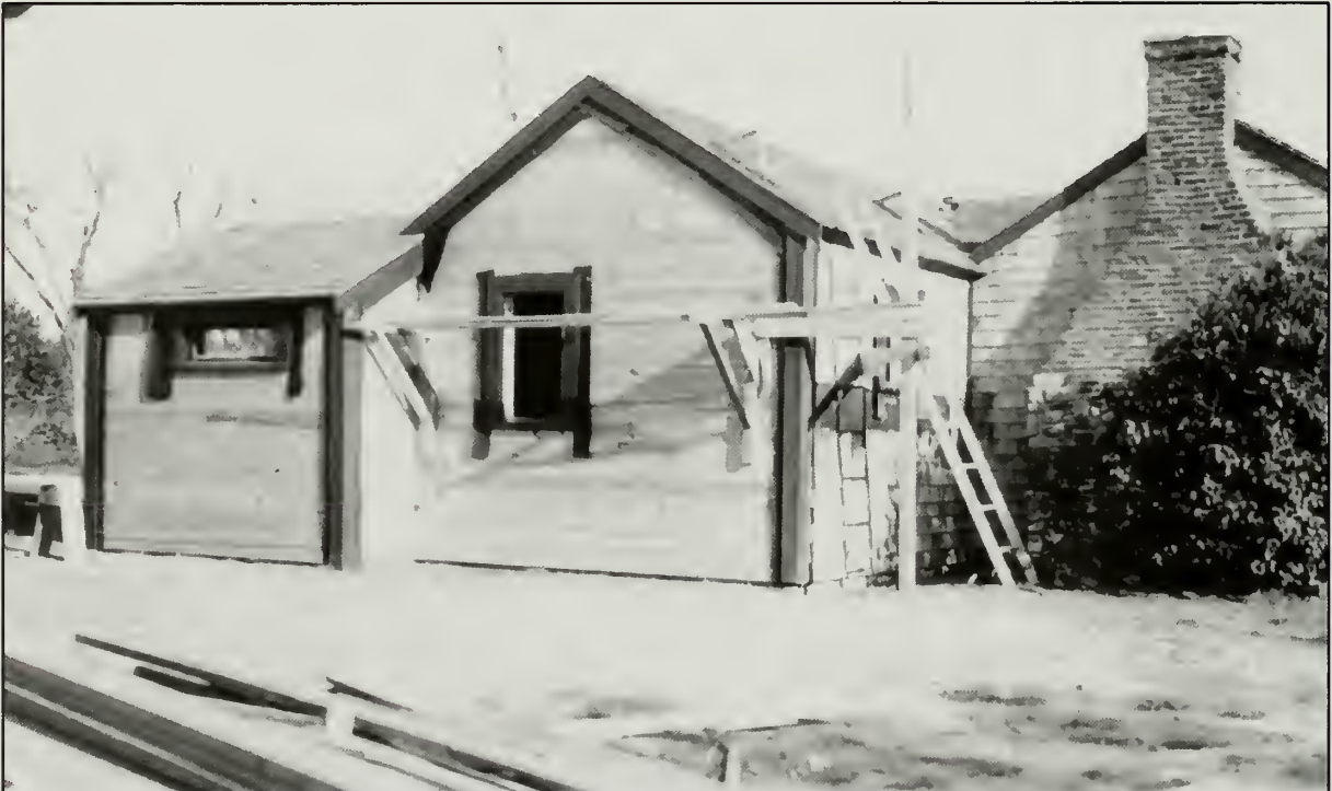
Figure 220. Addition constructed in 1951 on north elevation of Guest House (GKH Journal, p. 129).
