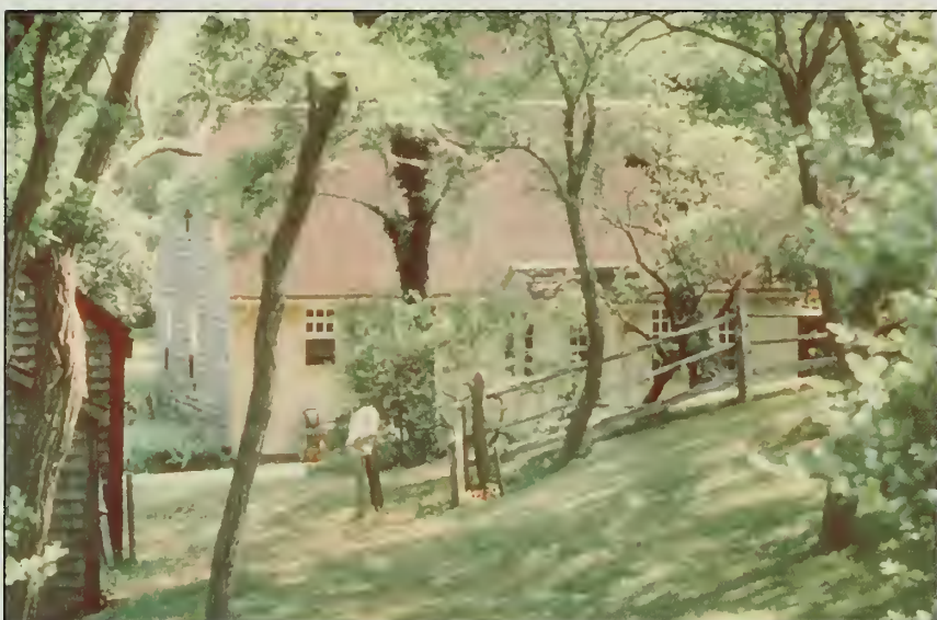
Figure 189. View northeast of the flower beds south and west of the house, 1959. Note the bench under the black locust tree and the mature lilac against the house. (Cape Cod archives, H6-116.)
