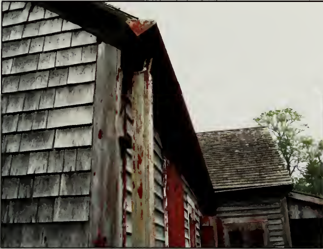
Figure 501. Gutter and downspout on east elevation, Country Store (2007).
