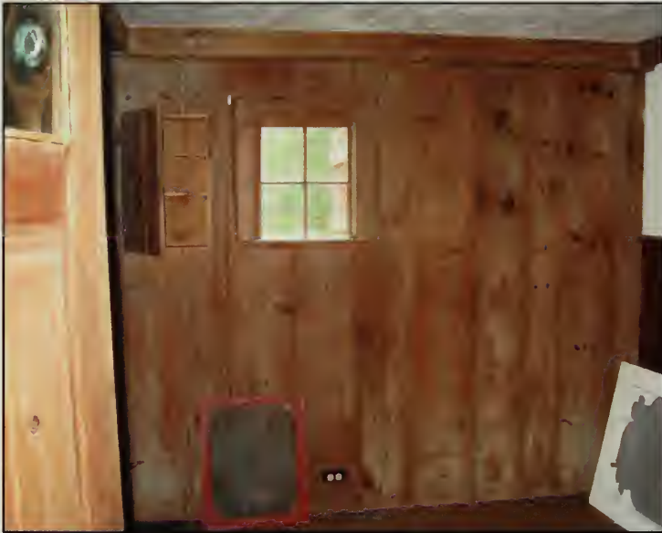
Figure 406. East wall of South Bedroom, Guest House (2007).
