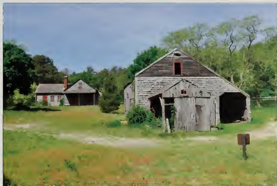
Figure 150. Looking west at the Barn and east side annex, May 2010. (OCLP)
