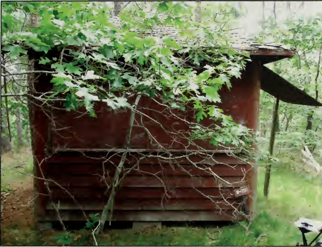
Figure 453. North elevation, Summer House (2007).
