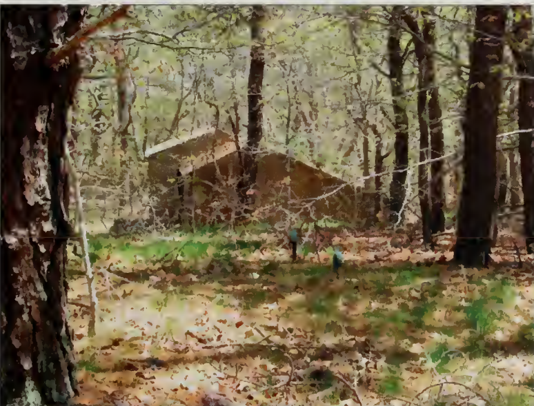
Figure 107. Green pipes north of the Garage as seen from the Old Town Road. (OCLP, May 2007.)
