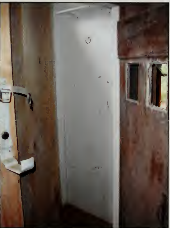
Figure 321. West wall of Harness, Barn (2007).
