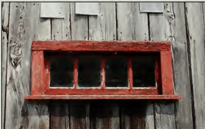
Figure 296. W102 in south elevation, Barn (2007).
