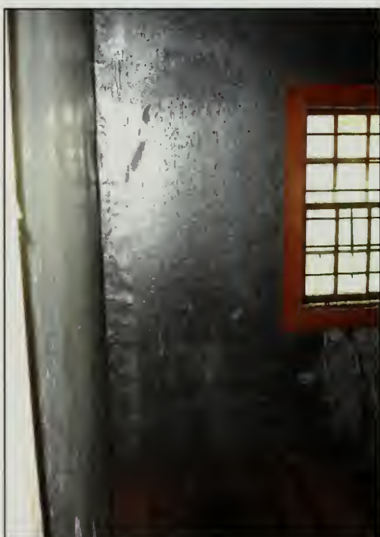
Figure 342. West wall of Bunk Room, Barn (2007).
