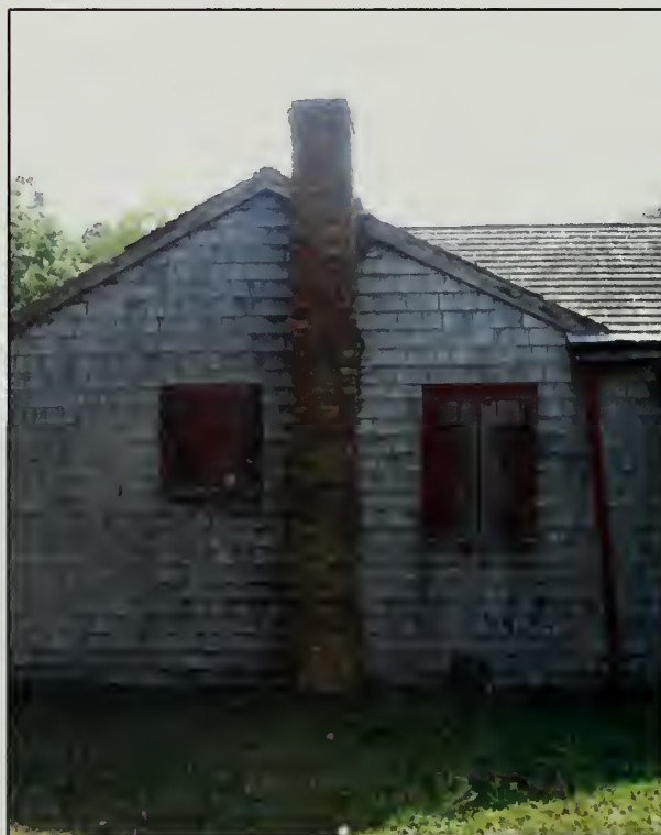
Figure 383. Chimney on southern end of east elevation, Guest House (2007).
