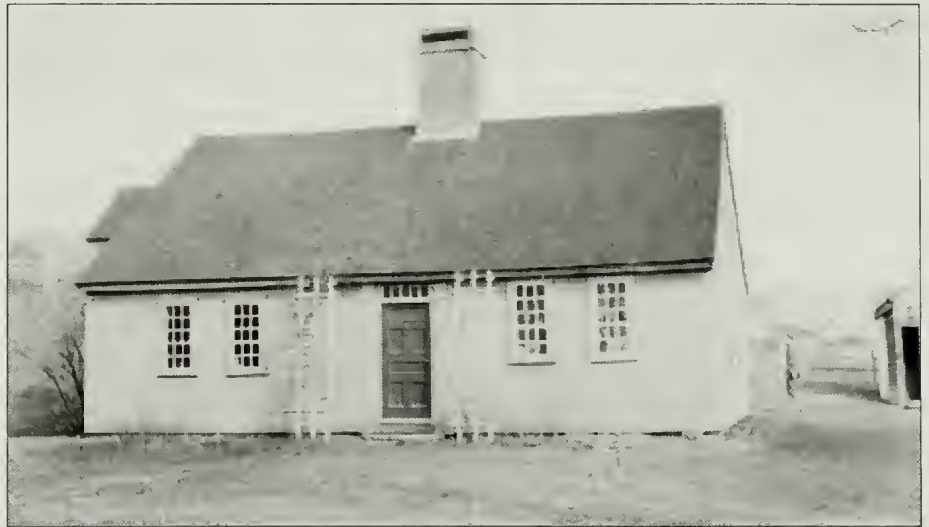
Figure 123. Looking northwest at the newly resingled Atwood-Higgins House, in 1920. (Cape Cod NS archives.)
