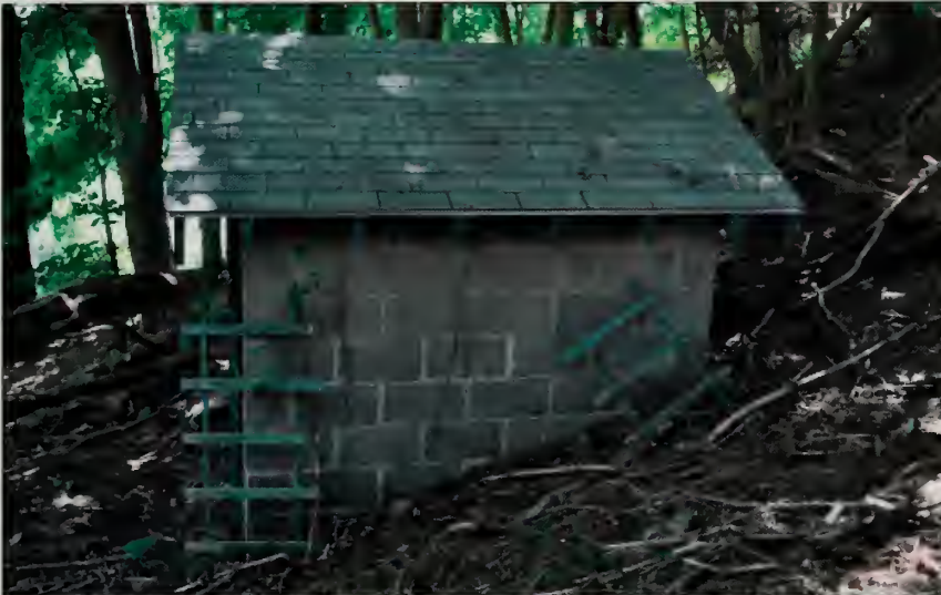
Figure 548. North elevation, Wellhouse (OCLP, August 2010).
