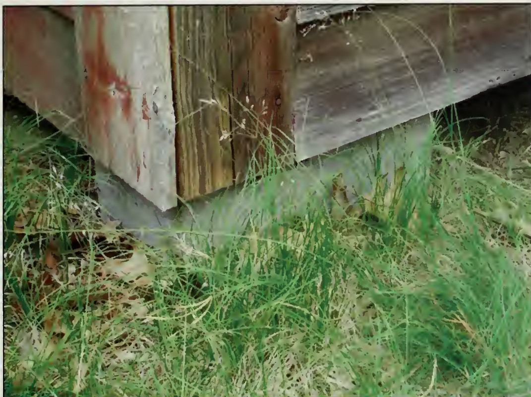
Figure 456. Concrete block foundation, Summer House (2007).
