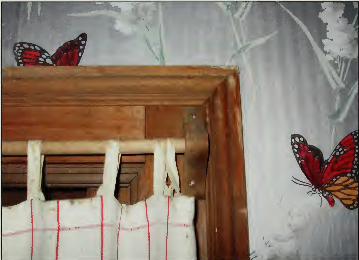
Figure 419. Interior window trim of W111 of Bath, Guest House (2007).
