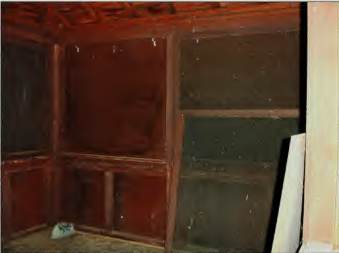
Figure 467. South wall inside Summer House (2007).
