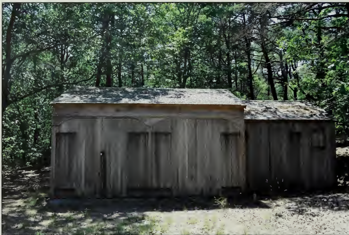
Figure 254. Northeast elevation, Garage (OCLP, 2010).
