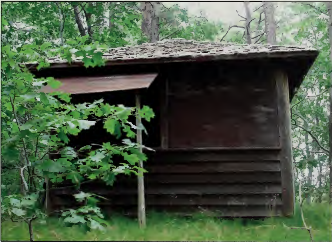
Figure 454. West elevation, Summer House (2007).
