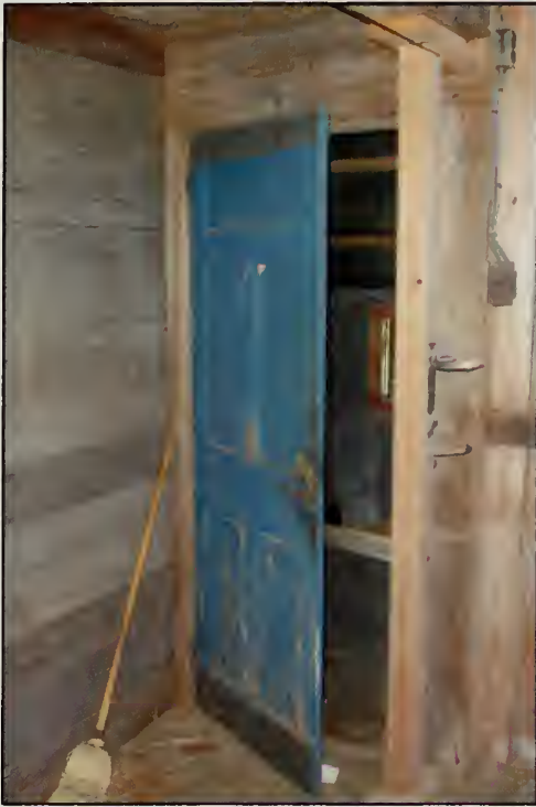
Figure 337. D110 in north wall of Carriage Room, Barn (2007).
