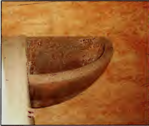
Figure 313. Iron trough in northwest corner of stall, Barn (2007).
