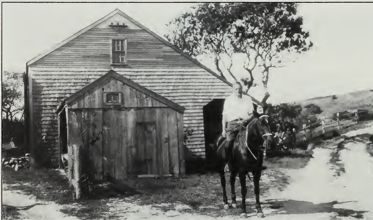
Figure 214. East elevation of Barn. Note the exterior of the bird refuge at the gable peak, constructed in 1930. (Higgins Scrapbook H6-194).
