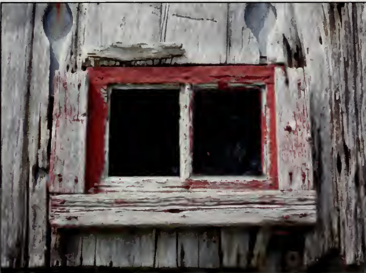
Figure 299. W105 in east elevation, Barn (2007).
