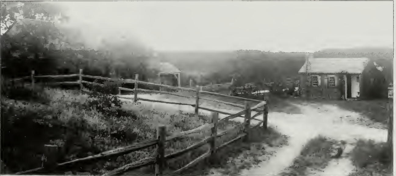
Figure 177. View northwest of the Barn and Guest House with driveway in foreground, 1942. Note the light fixture at the far right. (Cape Cod archives.)
