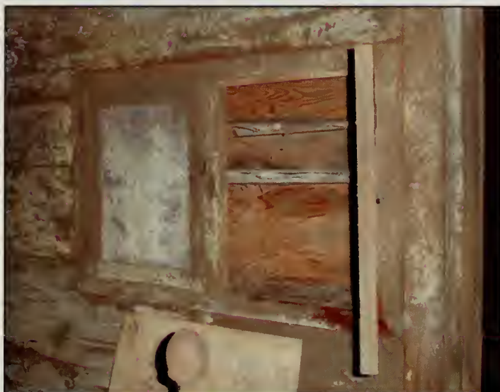
Figure 269. Built-in, cabinet left of D104. Northwest wall, Room 101, Garage (2007).
