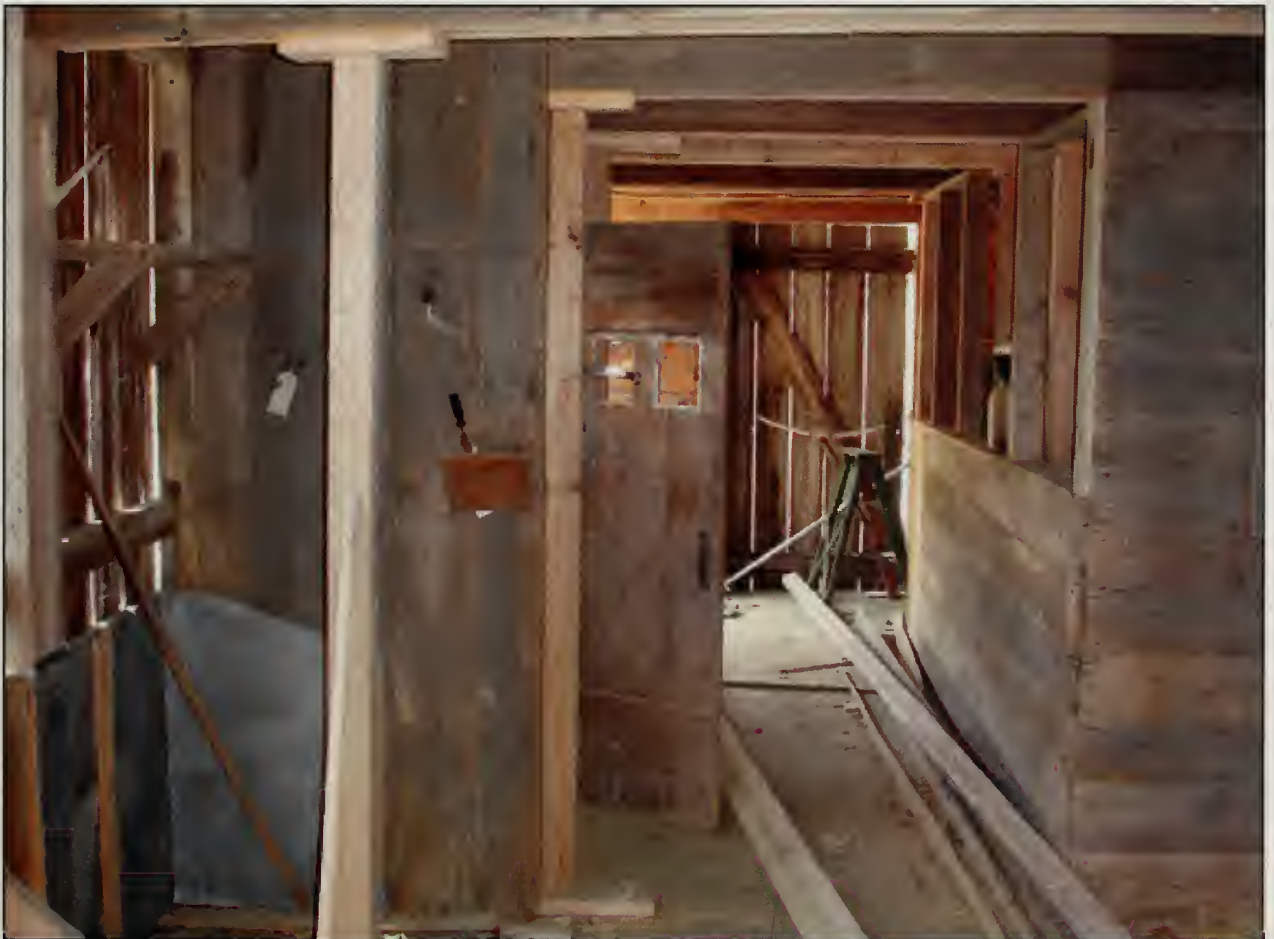
Figure 339. D109 in west wall, of Carriage Room, Barn (2007).
