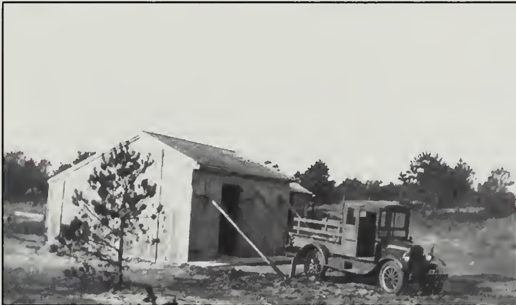
Figure 207. Garage, 1929. Note vertical siding on southeast elevation not yet sided with wooden shingles. (Scrapbook, Photograph H6-187).
