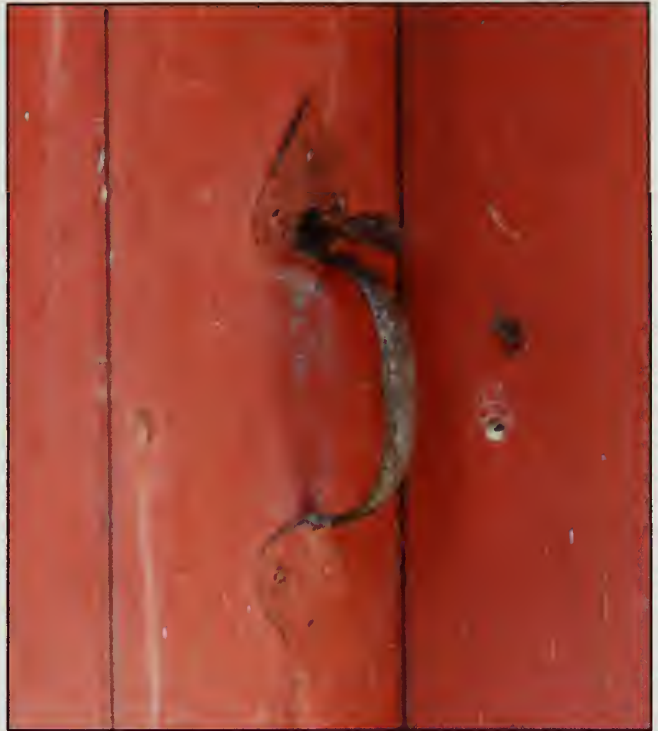
Figure 360. Iron thumb latch on door within D101, west elevation, Guest House (2007).
