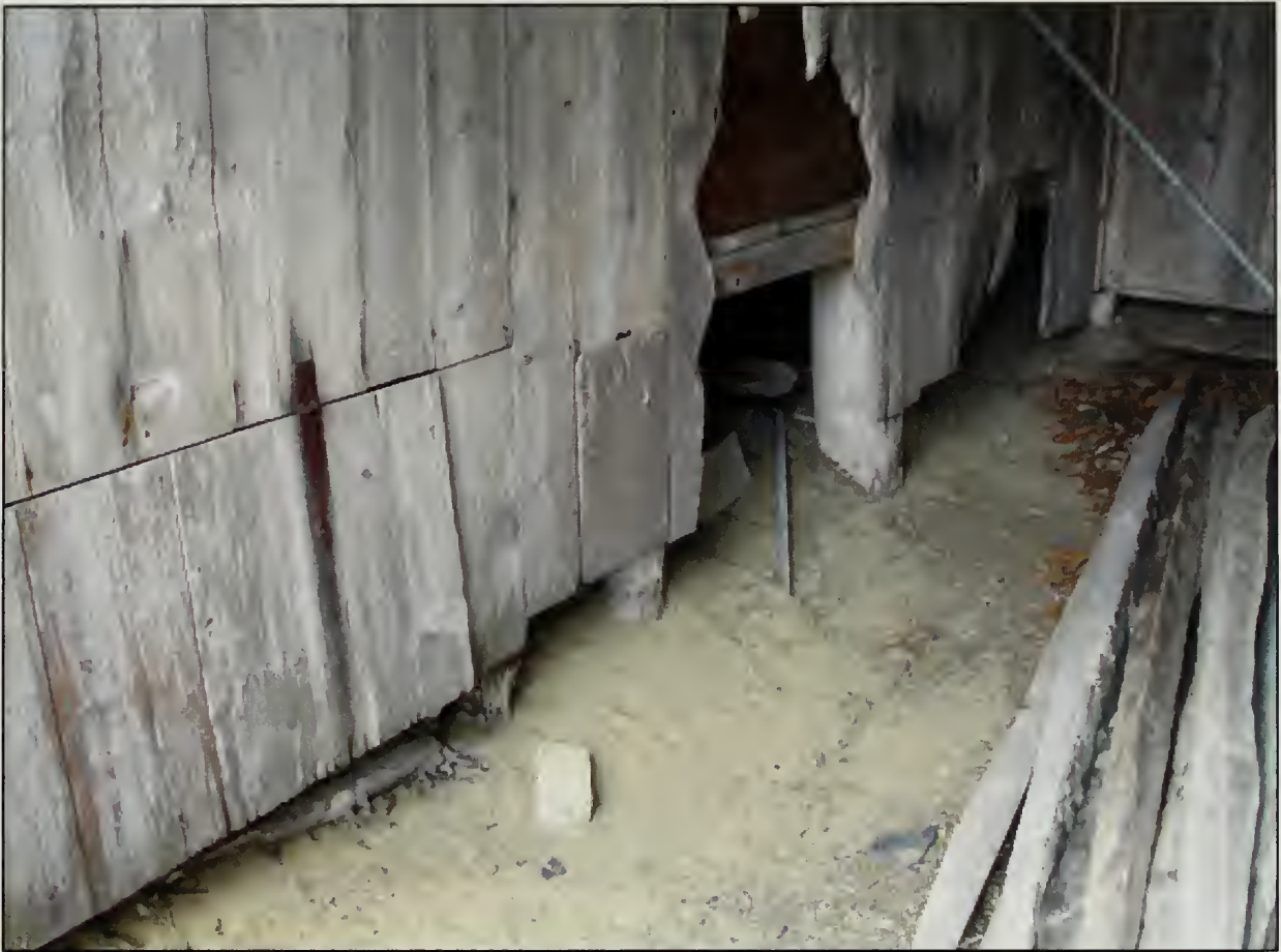
Figure 286. Wooden post foundation, Barn. (Photograph taken in the Open Shed looking at the south wall on the north side of the Barn where wall siding is missing) (2007).
