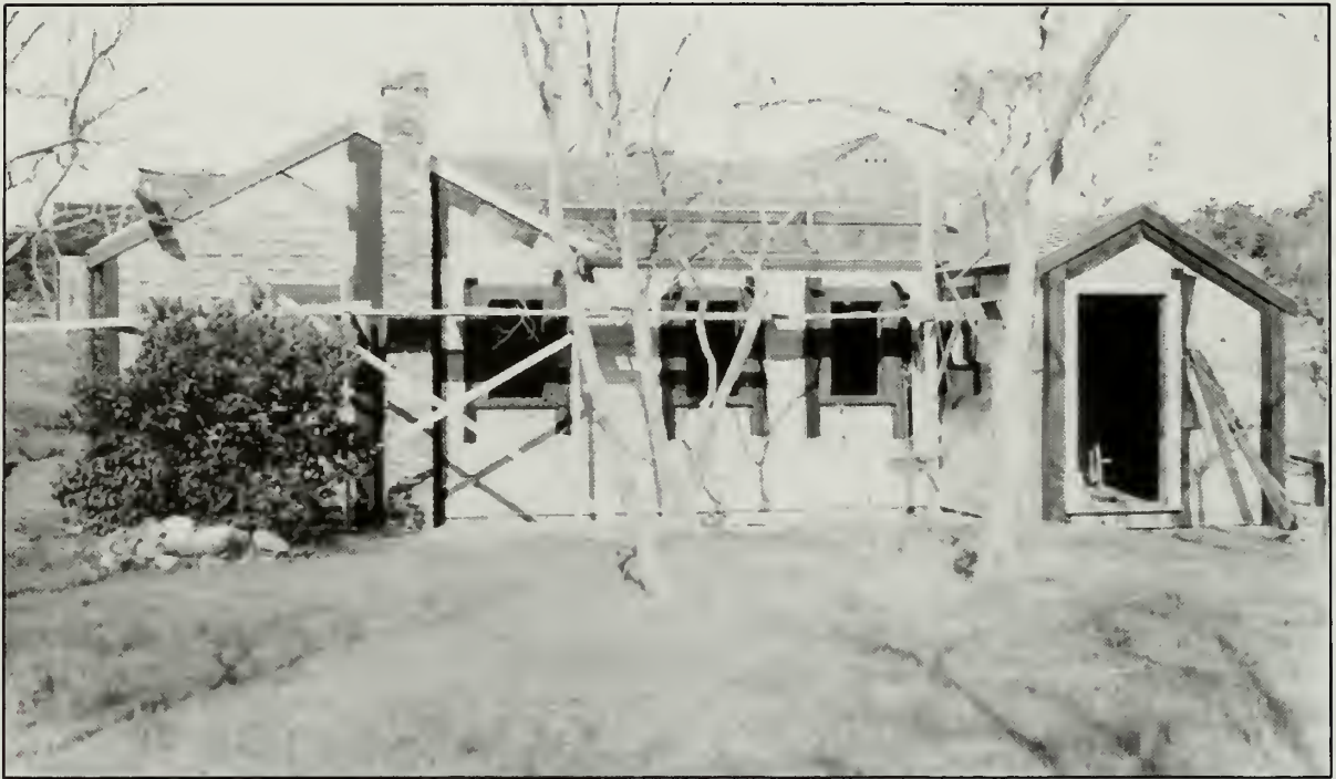
Figure 219. Addition constructed in 1951 on east elevation of Guest House (GKH Journal, p. 129).
