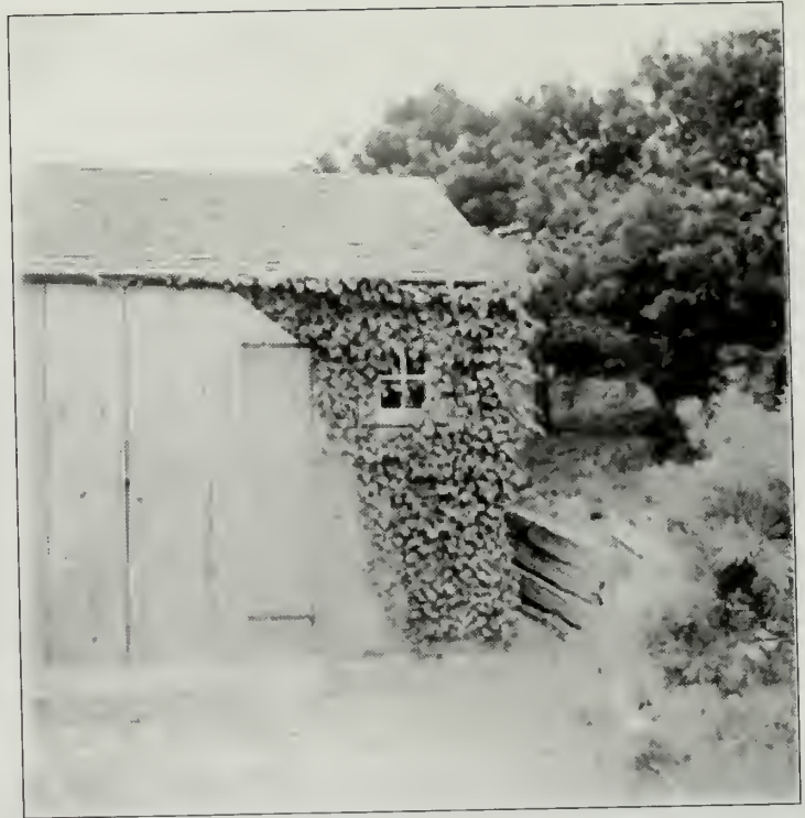
Figure 164. Looking west at the sand bank next to the Garage which was "bulkheaded" with railroad ties, c. 1929. (Cape Cod NS archives.)
