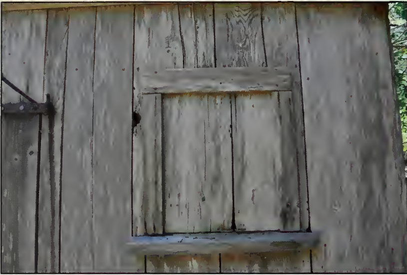
Figure 265. W101 in northeast elevation, Garage (OCLP, 2010).
