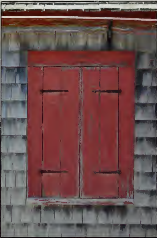
Figure 378. W113 in east elevation, Guest House (OCLP, 2010).
