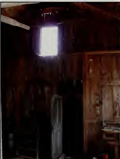
Figure 327. East wall and D11 of Carriage Room, Barn (2007).
