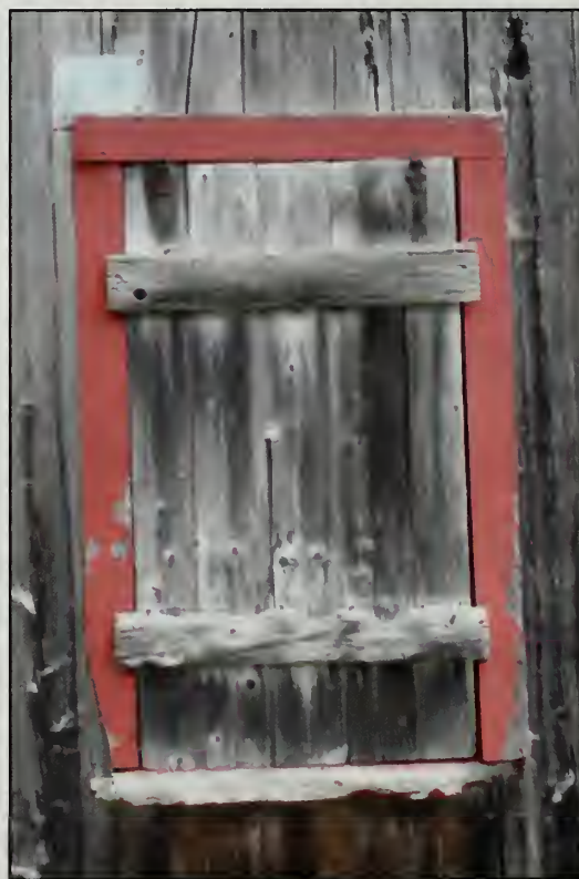
Figure 303. W109 in west elevation, Barn (2007).
