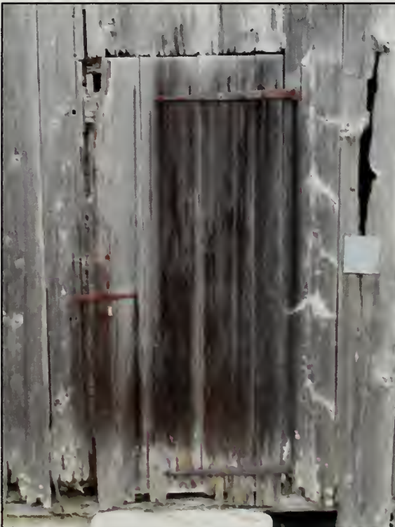
Figure 287. D101 in south elevation, Barn (2007).
