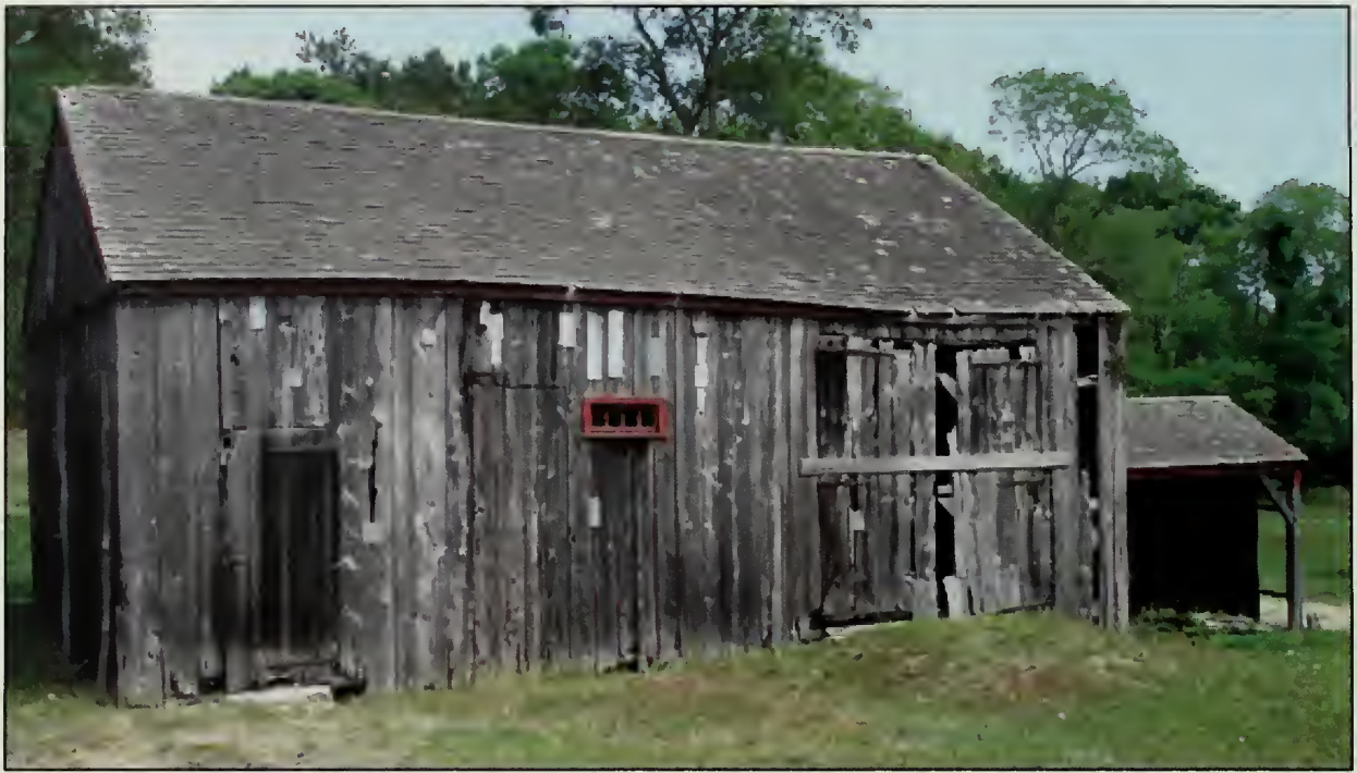
Figure 281. South elevation, Barn (2007).
