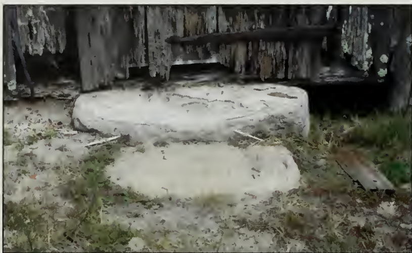
Figure 289. Two large stone steps, under D101 on south elevation, Barn (2007).
