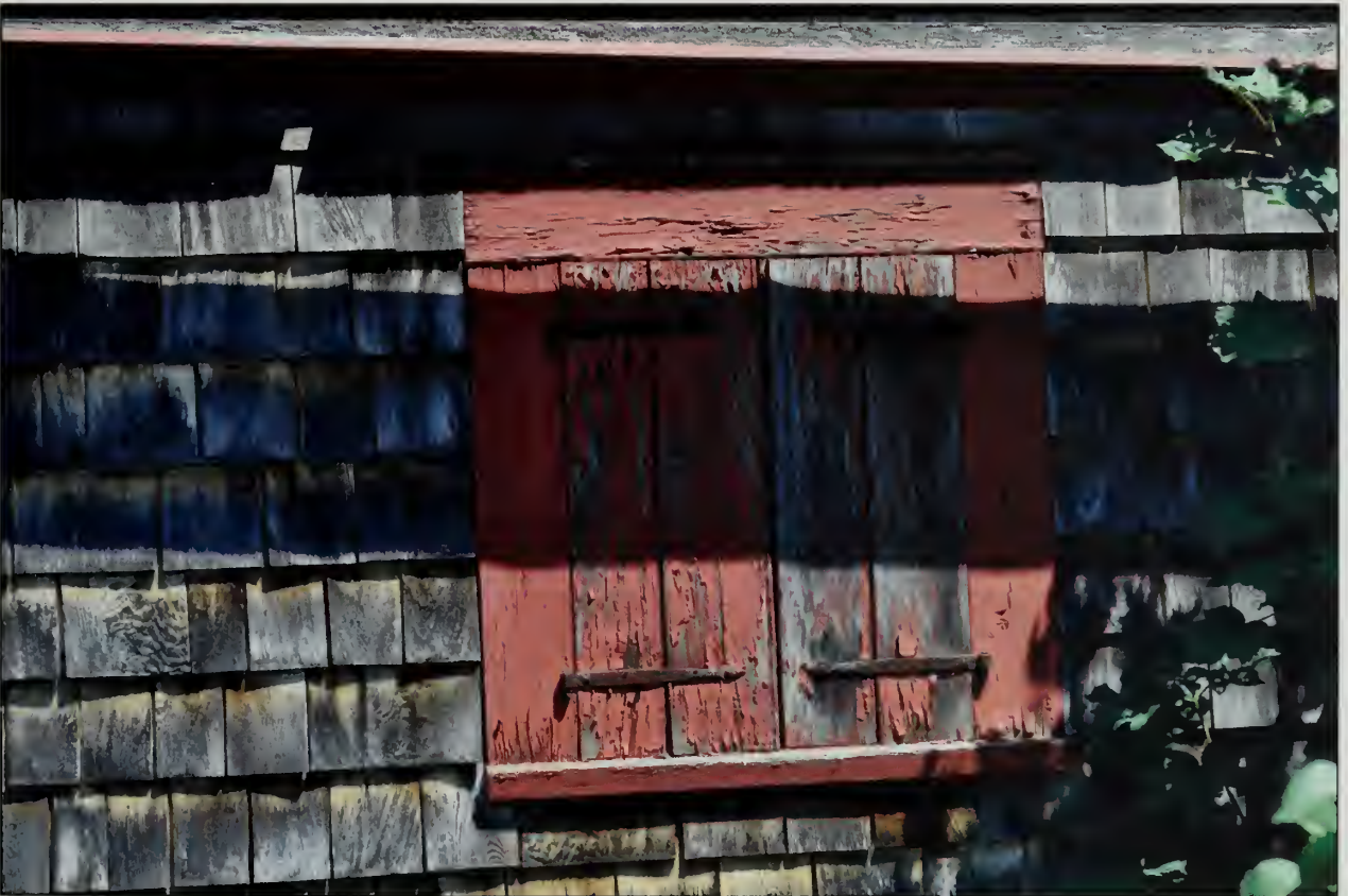
Figure 368. W101 in west elevation, Guest House (OCLP, 2010).
