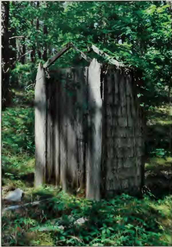
Figure 543. South and east elevations, Northeast Privy (OCLP, August 2010).
