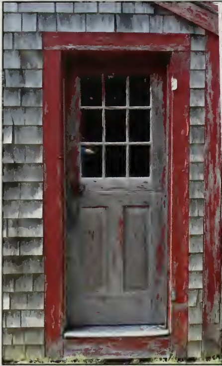
Figure 362. D102 in south elevation, Guest House (2007).
