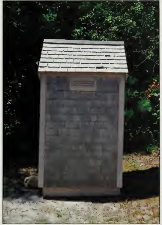
Figure 532. East elevation, Atwood-Higgins House Privy, rebuilt in 2007 (OCLP, August 2010).
