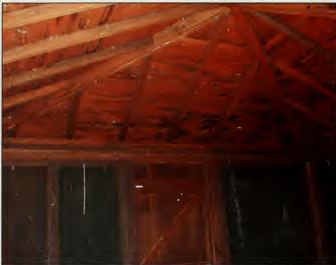
Figure 464. Roofing system, Summer House (2007).
