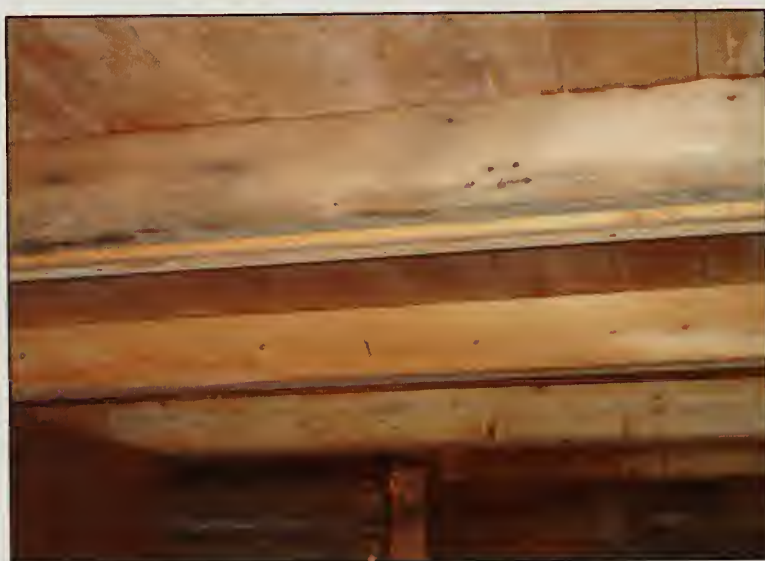
Figure 312. Ceiling of Stall, Barn (2007).
