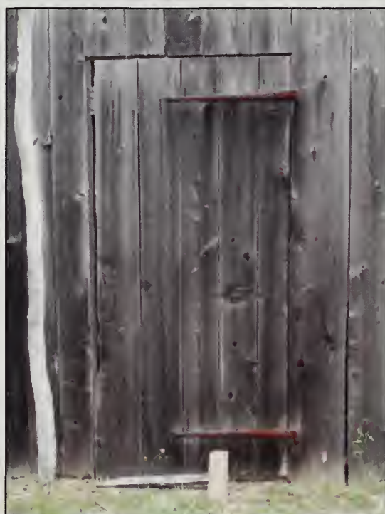
Figure 294. D105 in west elevation, Barn (2007).
