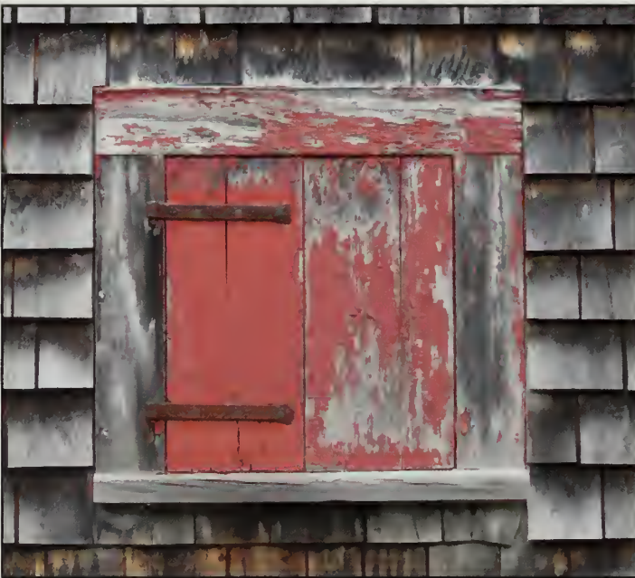
Figure 492. W107 in west elevation, Country Store (2007).
