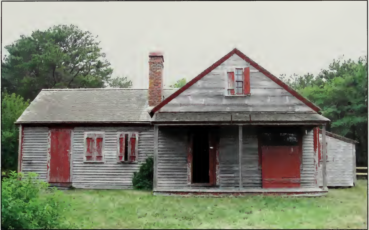
Figure 471. East elevation, Country Store (2007).
