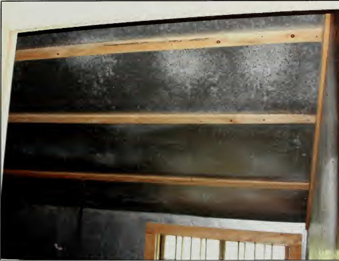
Figure 343. Ceiling of Bunk Room, Barn (2007).
