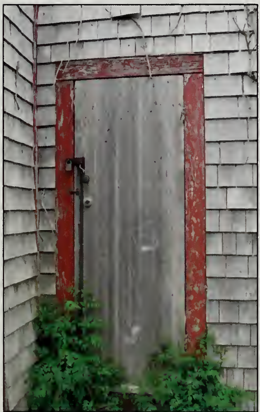
Figure 236. D103 in south elevation, Woodshed (2007).
