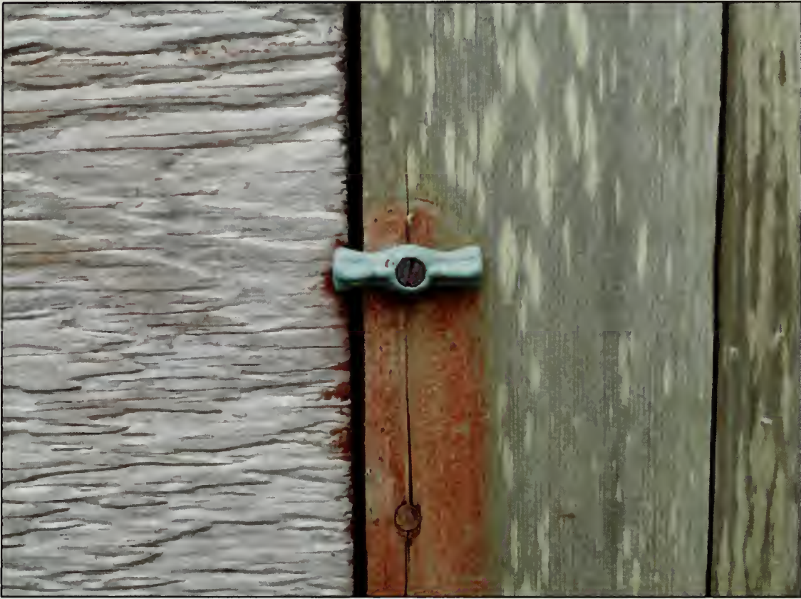
Figure 462. Typical turn lock mechanism for shutters on exterior window, Summer House (2007).
