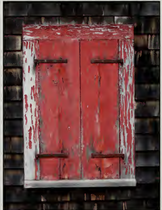
Figure 493. W108 in west elevation, Country Store (2007).
