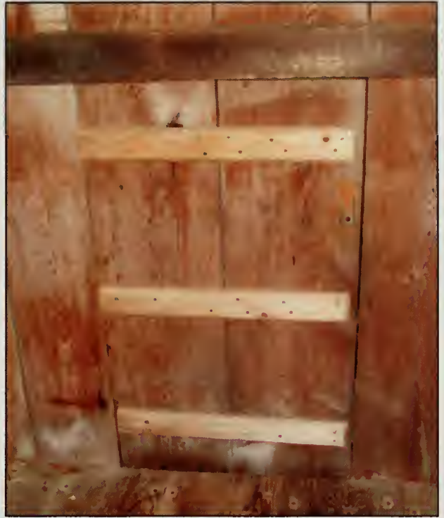
Figure 338. D112 in north wall of Carriage Room, Barn (2007).
