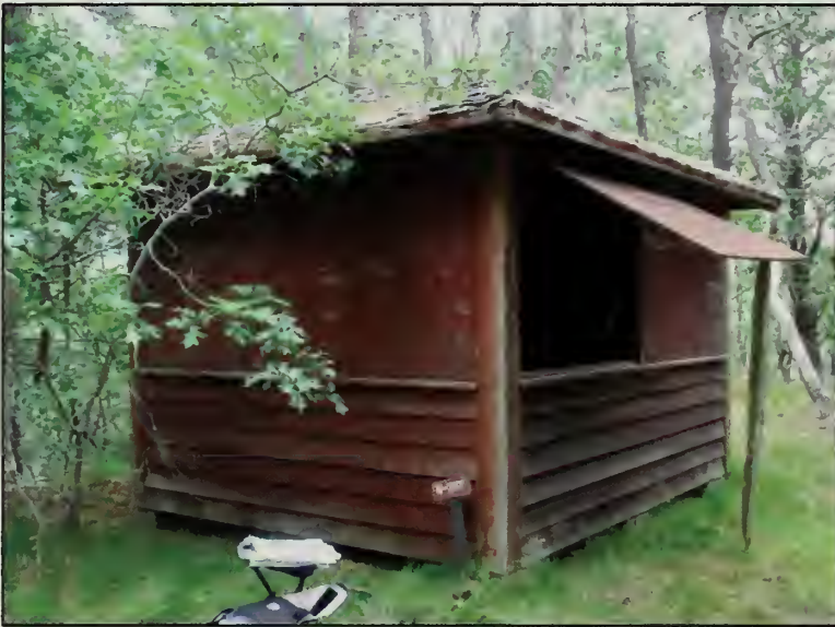
Figure 460. Four windows and shutters in the north and west elevation, Summer House (2007).
