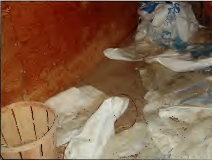
Figure 308. Floor of Stall, Barn (2007).
