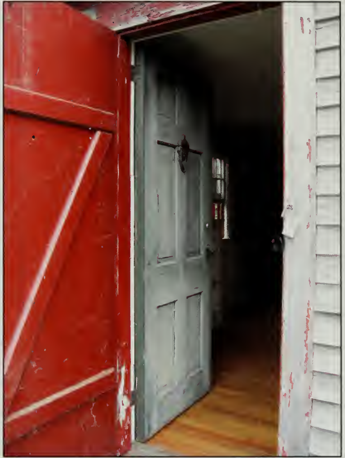
Figure 484. Interior door within D104 in west elevation, Country Store (2007).
