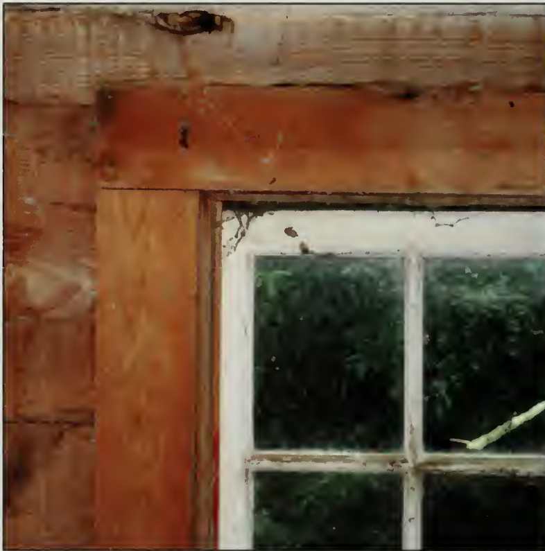
Figure 248. Window trim of W102 in Laundry section of Laundry/Bath addition, Woodshed (2007).
