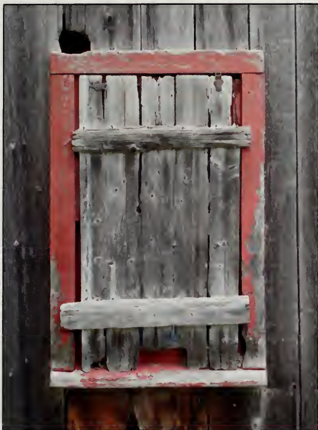
Figure 304. W110 in west elevation, Barn (2007).
