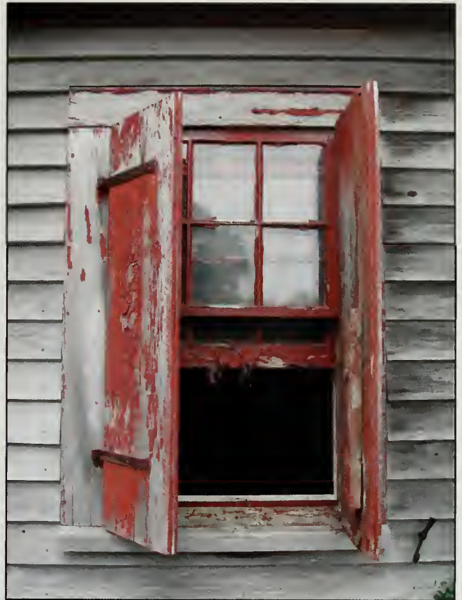
Figure 487. W102 in east elevation, Country Store (2007).
