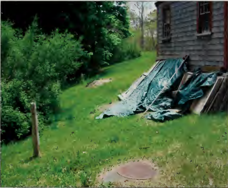
Figure 76. View south of a lone fence post to the east of the Woodshed. The cover for the septic tank is visible in the foreground (OCLP, May, 2007.)
