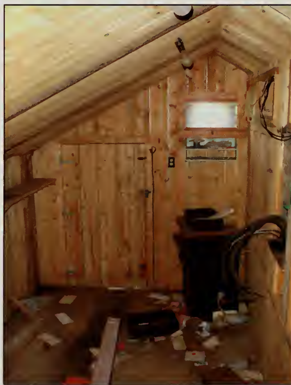
Figure 348. East wall of Shed, Barn (2007).
