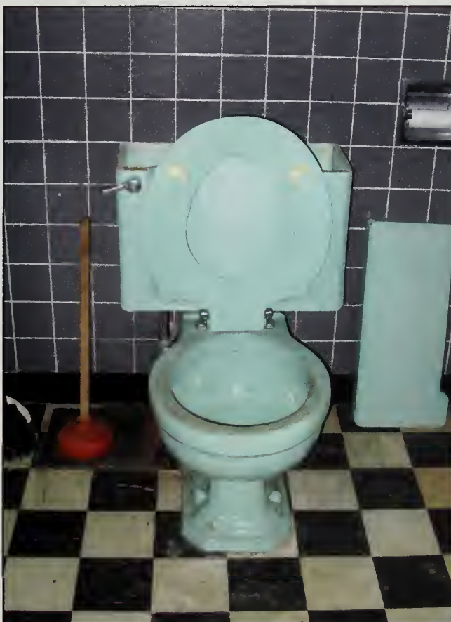
Figure 422. Toilet on north wall of Bath, Guest House (2007).
