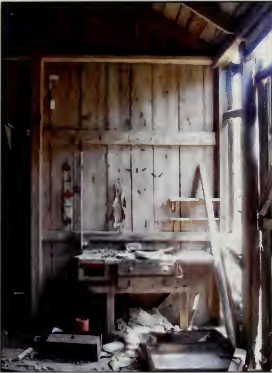
Figure 331. Built-in workbench on east wall of Carriage Room, Barn (2007).
