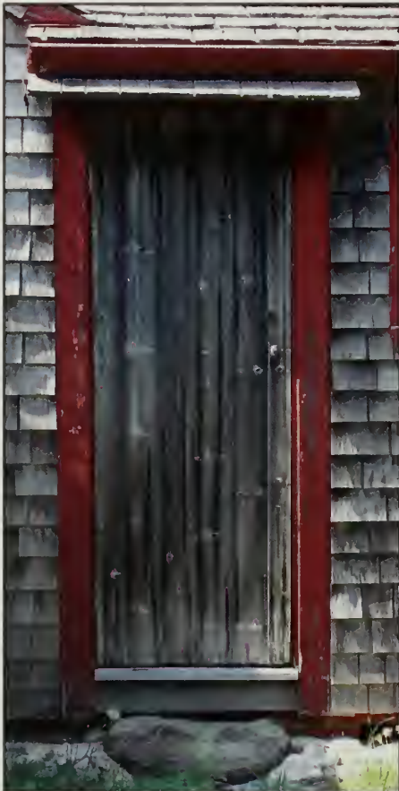
Figure 364. D103 in south elevation, Guest House (2007).
