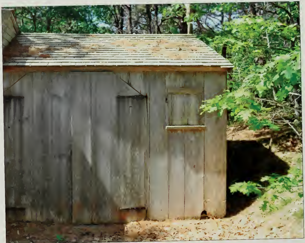
Figure 165. Looking west at the sand bank next to the Garage, May 2010. (OCLP)
