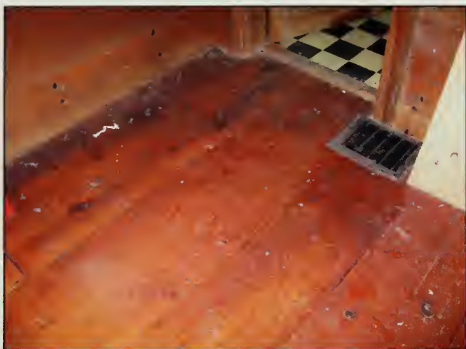
Figure 423. Floor of North Bedroom, Guest House (2007).
