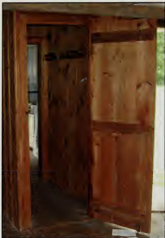
Figure 395. D105 in Living Room (leads into Hallway), Guest House (2007).
