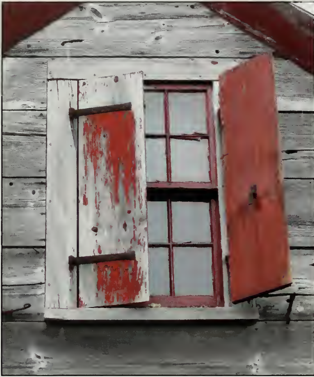
Figure 498. W201 in east elevation, Country Store (2007).
