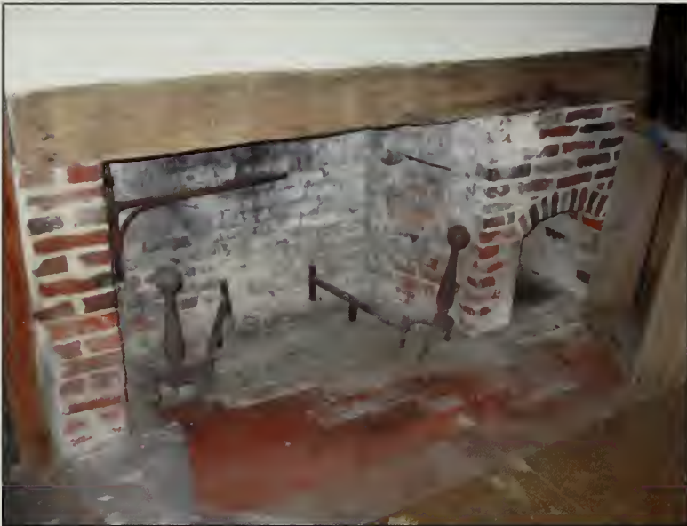
Figure 400. Fireplace in north wall of Living Room, Guest House (2007).
