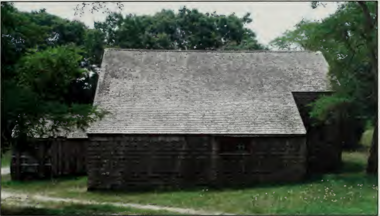
Figure 283. North elevation, Barn (2007).
