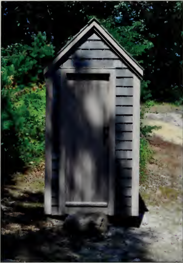
Figure 531. South elevation, Atwood-Higgins House Privy, rebuilt in 2007 (OCLP, August 2010).
