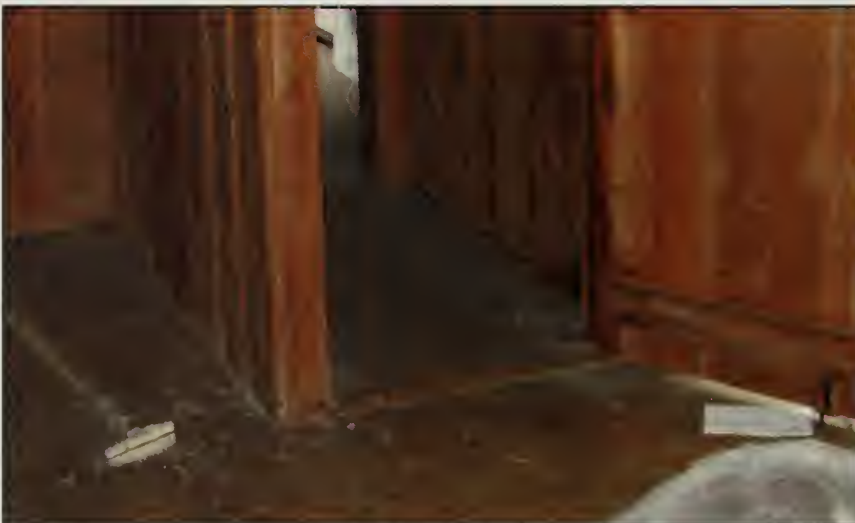
Figure 437. Floor of Hallway, Guest House (2007).
