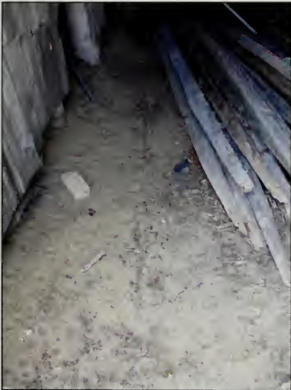
Figure 344. Floor of Open Shed, Barn (2007).
