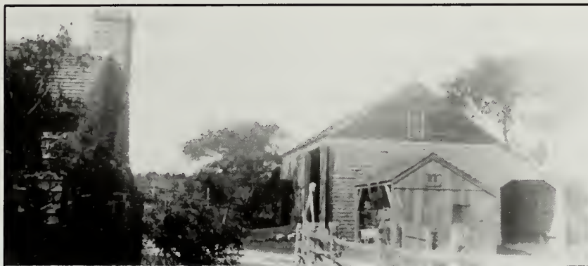
Figure 210. East elevation of Barn depicting east side annex constructed in 1927. (GKH Journal, p. 69)
