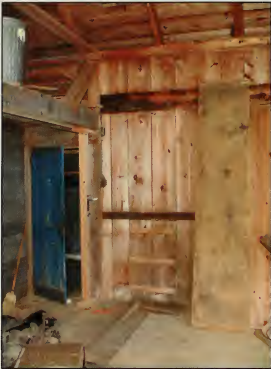
Figure 328. North wall and D110 of Carriage Room, Barn (2007).
