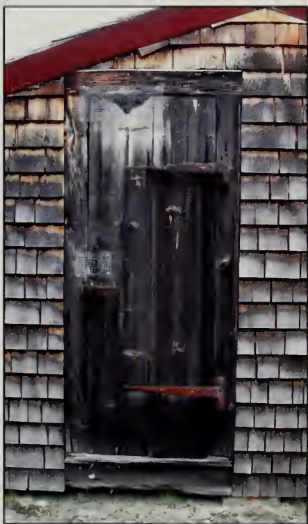
Figure 481. D103 in west elevation, Country Store (2007).
