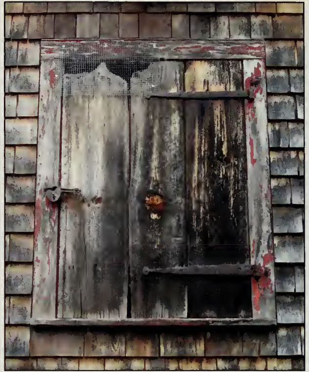
Figure 499. W202 in west elevation, Country Store (2007).
