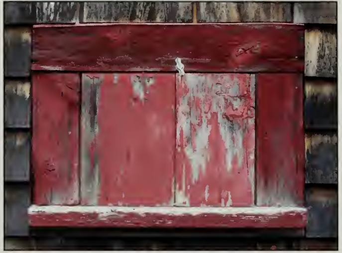
Figure 491. W106 in west elevation, Country Store (2007).
