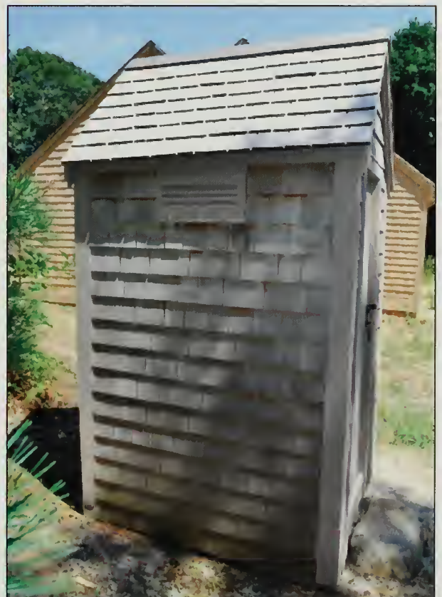
Figure 534. West elevation, Atwood-Higgins House Privy, rebuilt in 2007 (OCLP, August 2010).
