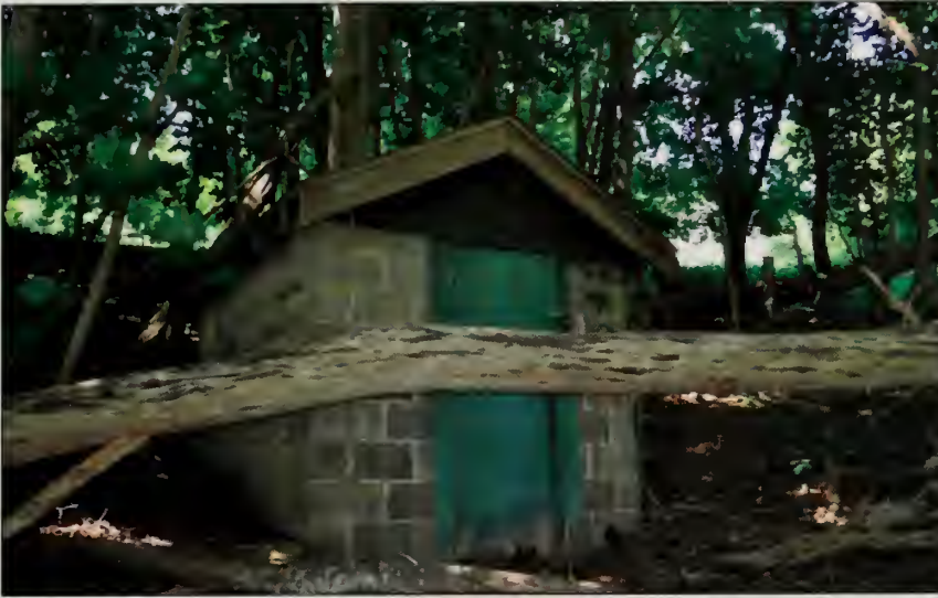
Figure 547. South and east elevations, Wellhouse (OCLP, August 2010).
