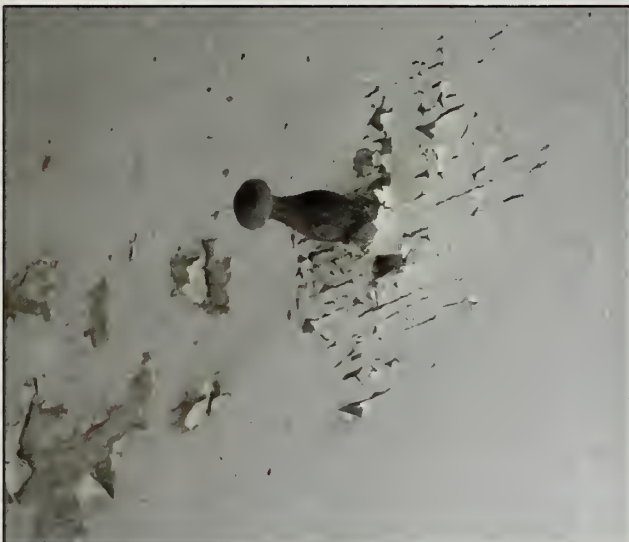
Figure 388. Wooden peg seen on south and east walls of Entry, Guest House (2007).
