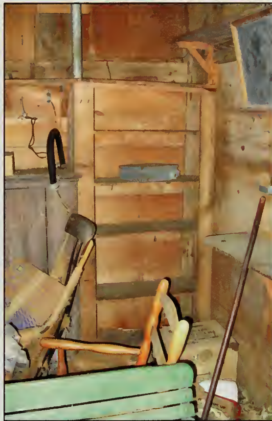
Figure 241. Shelving unit on east wall in the Storage Room, Woodshed (2007).
