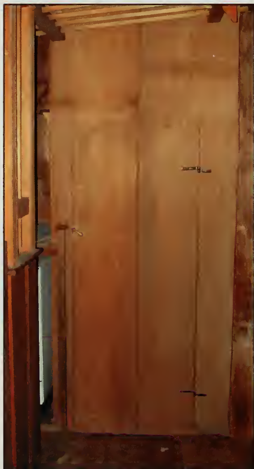
Figure 520. D106 in west wall of Country Store Room, Country Store (2007).
