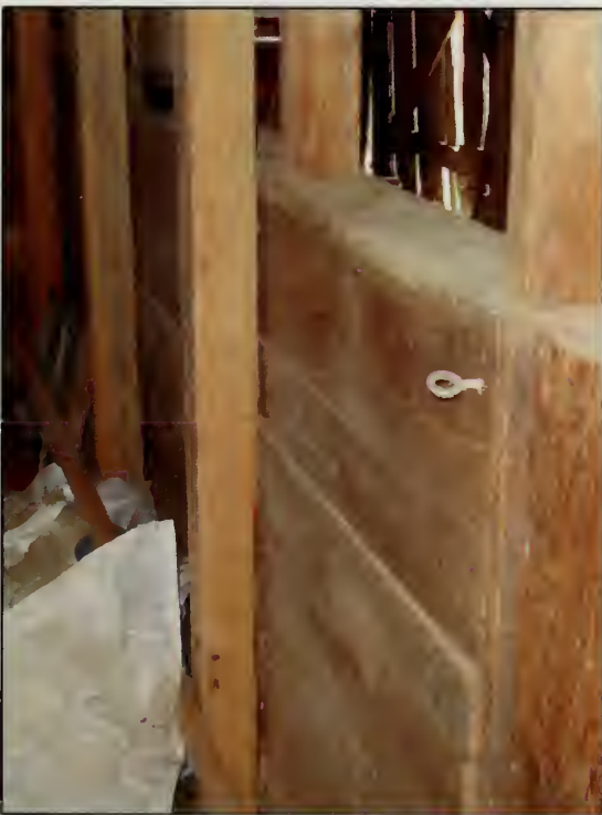
Figure 309. South wall of Stall, Barn (2007).
