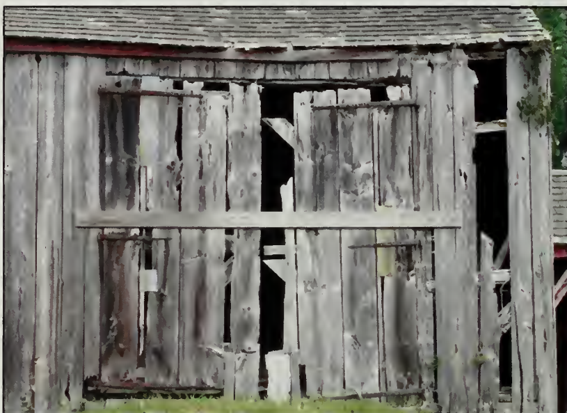
Figure 290. D102 in south elevation, Barn (2007).
