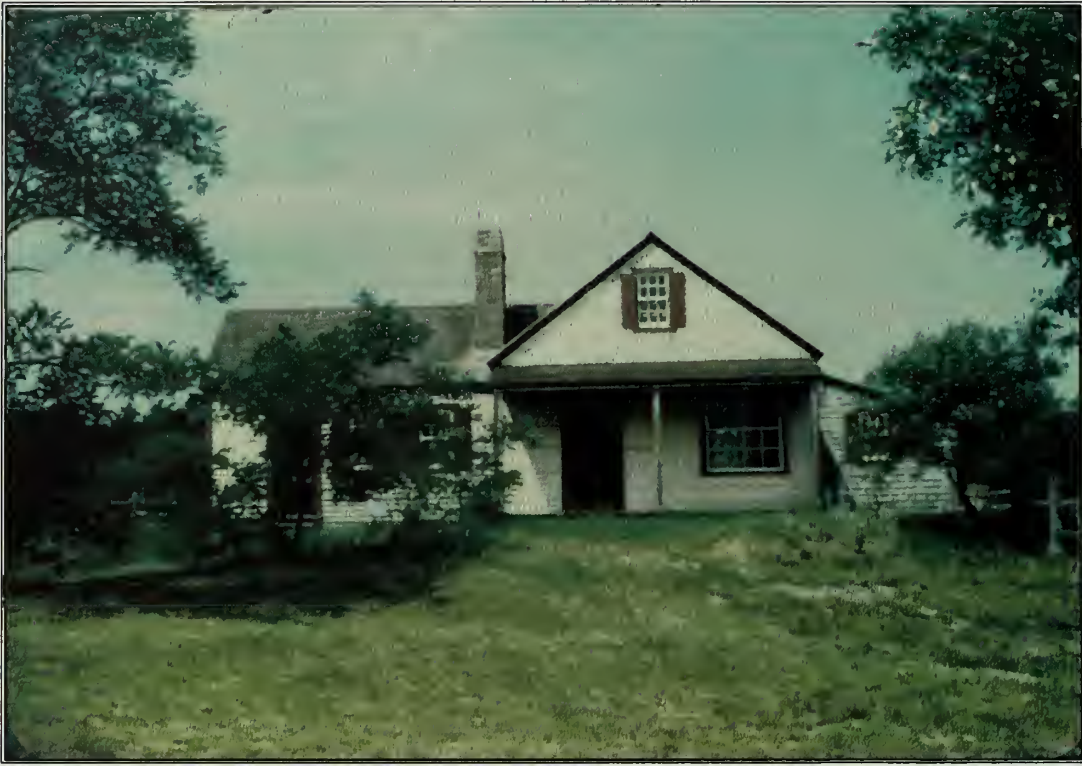
Figure 226. Photograph of the east elevation of the Country Store in 1948 upon completion. (GKH Journal, p. 118).
