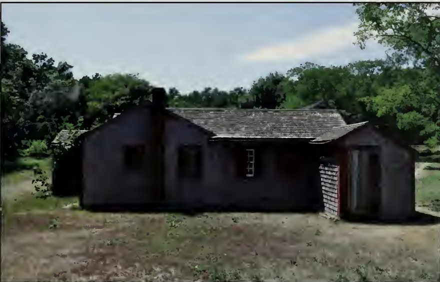
Figure 356. East elevation, Guest House (OCLP, 2010).
