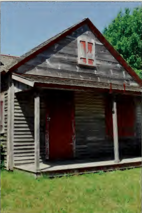
Figure 175. Looking west toward the Country Store porch, May 2010. (OCLP)
