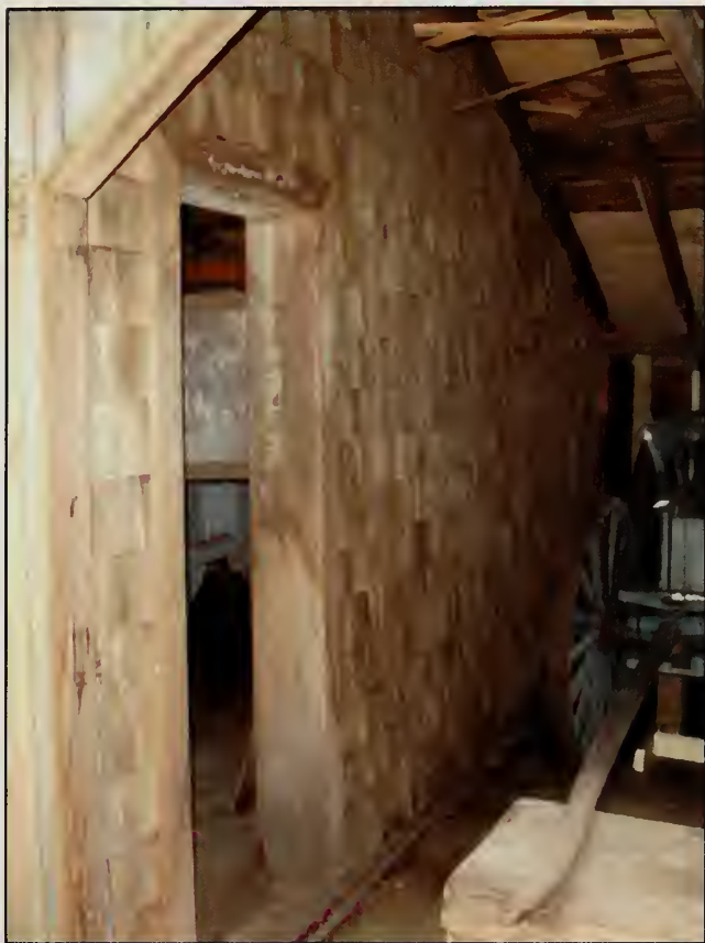
Figure 274. Southeast wall of Room 102, Garage. Note siding is exterior wooden shingles (2007).
