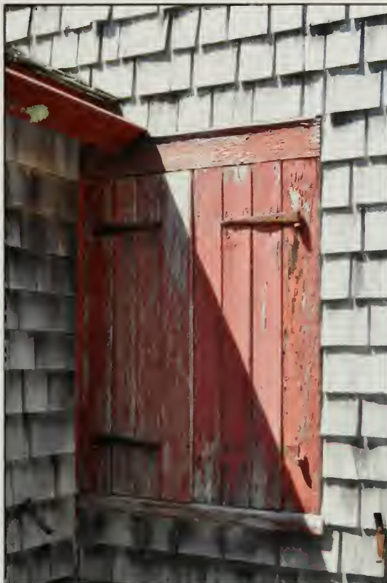
Figure 372. W106 in south elevation, Guest House (OCLP, 2010).
