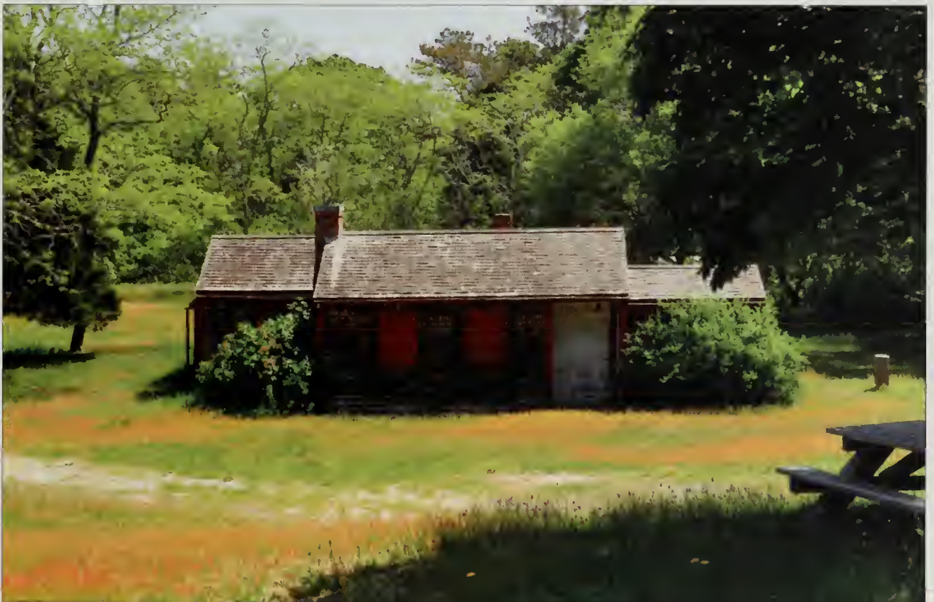
Figure 159. Looking east at the Guest House, May 2010 (OCLP).
