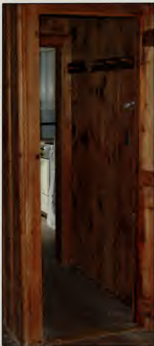
Figure 438. West wall of Hallway, Guest House (2007).
