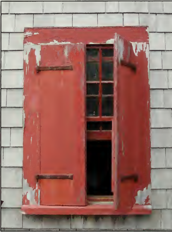
Figure 490. W105 in north elevation, Country Store (2007).
