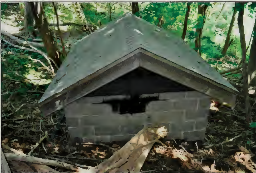
Figure 549. West elevation, Wellhouse (OCLP, August 2010).
