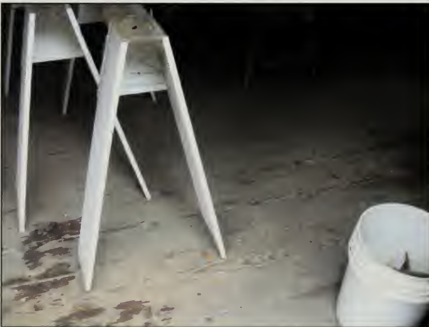
Figure 239. Floor of Storage Room, Woodshed (2007).
