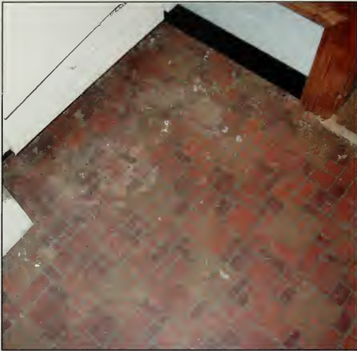
Figure 440. Floor of Kitchen, Guest House (2007).
