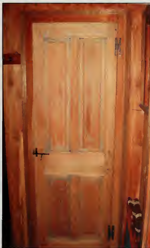
Figure 434. D112 in east wall of Closet, Guest House (2007).
