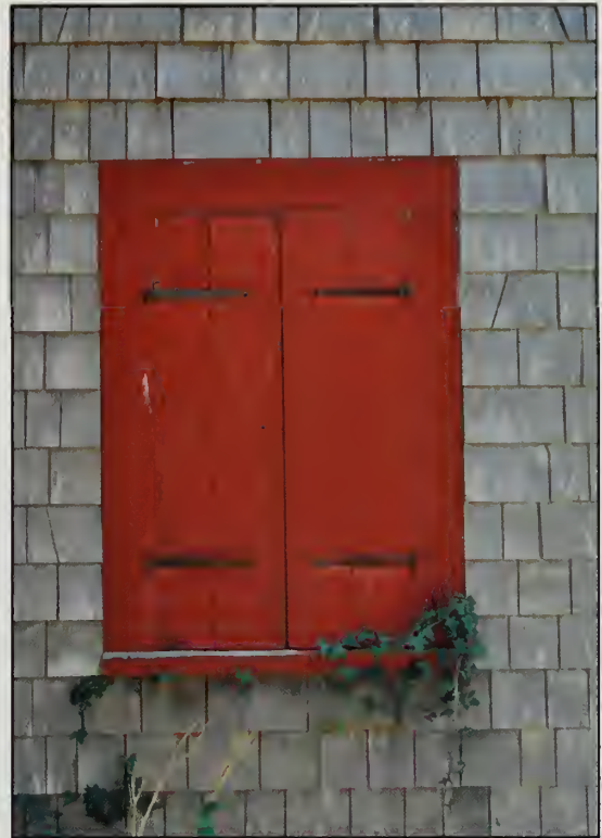
Figure 380. W115 located in north elevation, Guest House (OCLP, 2010).
