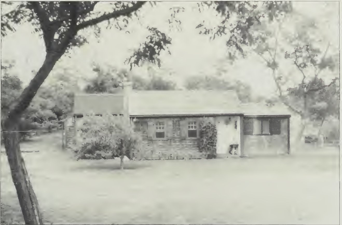
Figure 158. Looking east at the Guest House, complete with 1951 and 1952 additions, likely in the 1950s. Note the granite sun dial base, at right, and the additions of an extra bedroom and bathroom (at left) and Pullman kitchen (at right) to the building (Cape Cod NS archives, H6-267).
