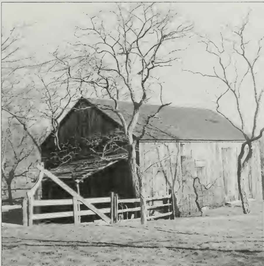
Figure 38. Looking northeast at the Barn and open lean-to, in a photo taken for the 1973 Historic Structure Report on the Atwood-Higgins building complex. (Cape Cod NS archives, H6-298.)
