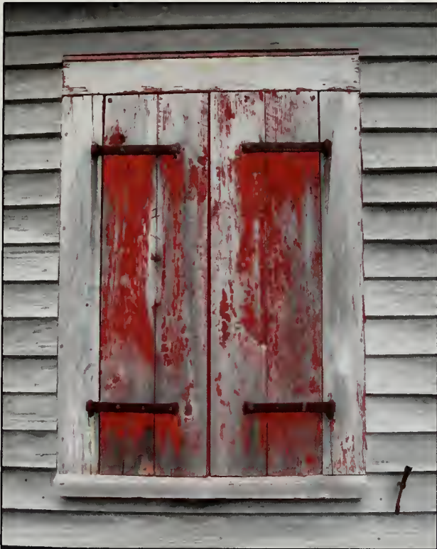
Figure 486. W101 in east elevation, Country Store (2007).
