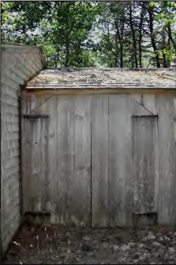
Figure 263. D103 in northeast elevation, Garage (OCLP, 2010).
