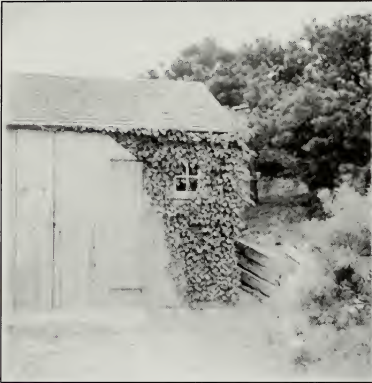
Figure 206. Northeast elevation of Garage, northwest end. Note two-over two casement window located in W101, and railroad ties used for the bulk heading of the sandbank (right). (GKH Journal, p. 75, 1929).
