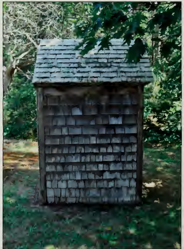
Figure 538. West elevation, Guest House Privy, rebuilt in 2007 (OCLP, August 2010).
