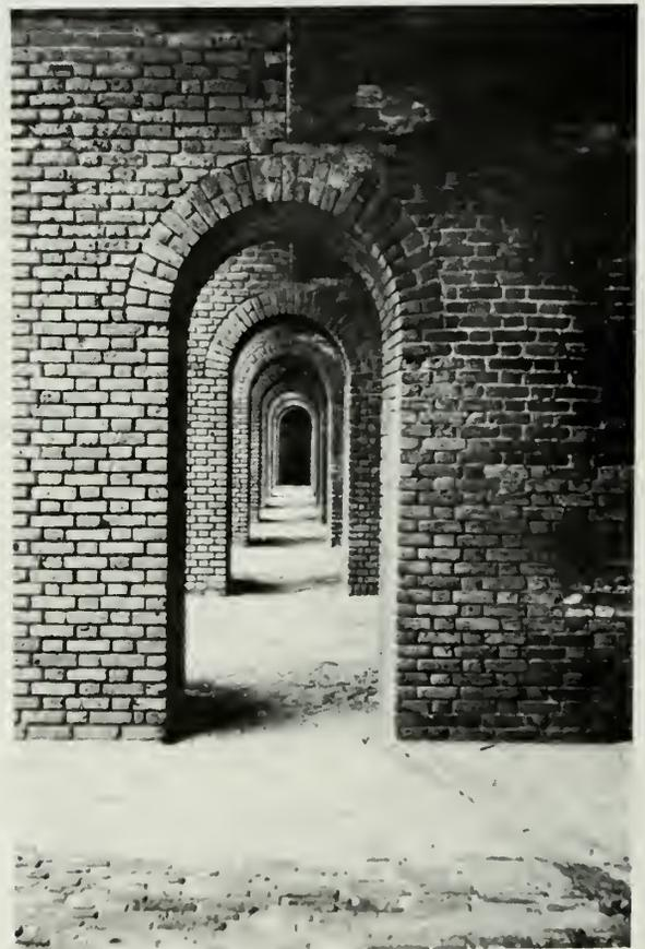
**Plate 8.4.** Example of second tier brickwork in the communication passage. NPS photo by Randy Jonsson.
