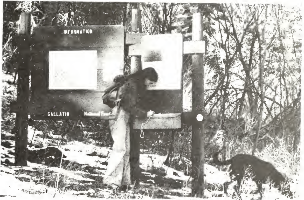
Figure 1.--Double-panel trailhead information center used at major trailheads.
