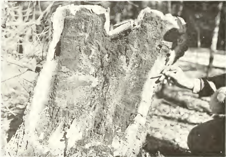
Figure 19. —About 83 percent of the wood in a cross section of this oak trunk had been destroyed by decay, equivalent to about 65 percent reduction in mechanical strength. The tree would be rated as potentially hazardous. (National Park Service photo.)
