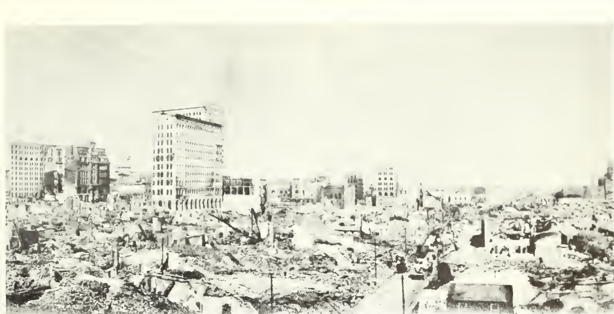
Figure 20.—Baltimore after the fire, looking down Lombard Street. Brick buildings crumbled. Fireproof buildings were gutted. The Continental Trust Building is behind the large structure at left center. (Reproduced from Baltimore Afire , published and copyrighted by Schneidereich & Sons, Baltimore, Maryland.)
