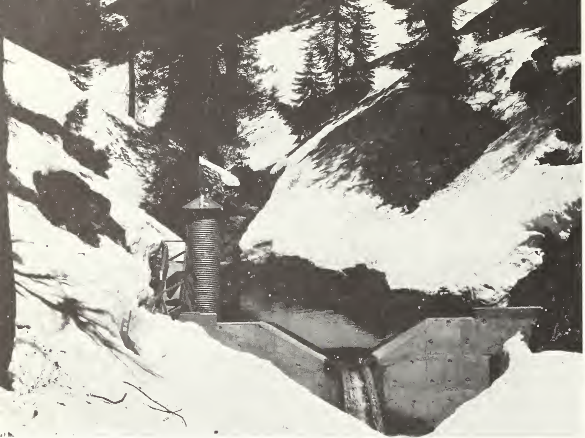
Figure 13.—Water yield resulting from application of alternative management techniques will be tested on a dozen small watersheds with weirs.
