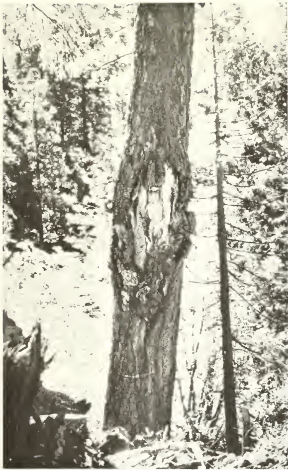
Figure 11. —An old dwarfmistletoe trunk swelling that has developed into an open, dead-faced canker on a white fir. This one would be rated as marginally hazardous.
