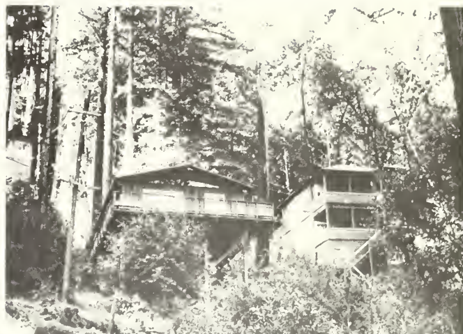
Figure 17. — Houses in young-growth redwood stands effectively remove the land from timber use.
