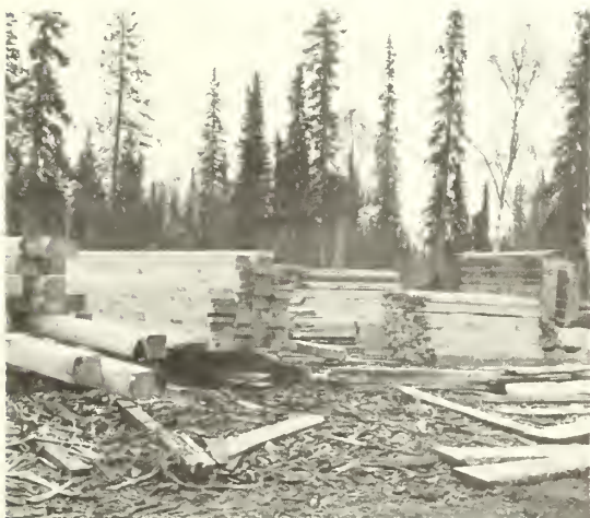
Figure 19.--Because of availability, cost, and good insulation value many homes in the Aniak area are built of these three-sided logs.
