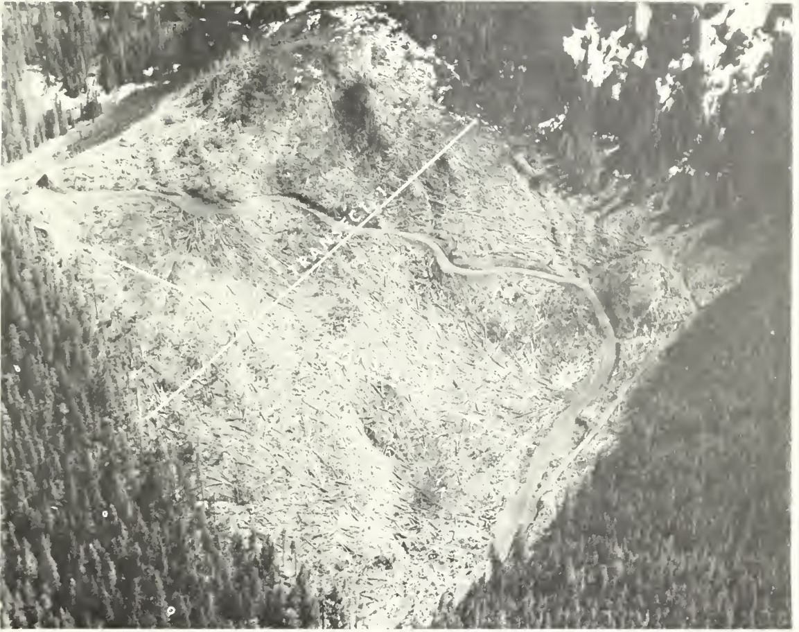
Figure 2.—On 16 of the 30 clearcuts sampled, two transect lines crossing at right angles (as shown above) were located in the units. This is the 100-acre Upper Wash Creek Unit, Mount Hood National Forest. It contained 14,390 cubic feet of residues per acre, with 7,472 cubic feet per acre of material which could be chipped if it could be removed. The unit had 191 tons of residues per acre.
