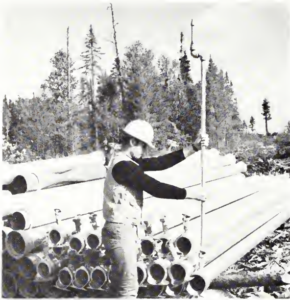
Figure 6.—Aluminum riser installed in quick couplers on a section of lateral pipe.
