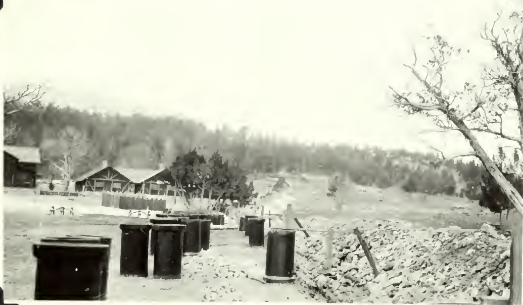
11045-6. Mammoth Sewer, Project #492. Closeup of ditch in Camp Ground. Material in right foreground typical of 65% of excavation.
