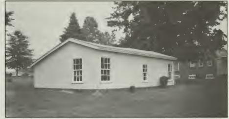
Figure 20 Poultry house, originally used as temporary house, with original board-and-batten siding, Circle 4. Photographer: David Ames, HABS.
