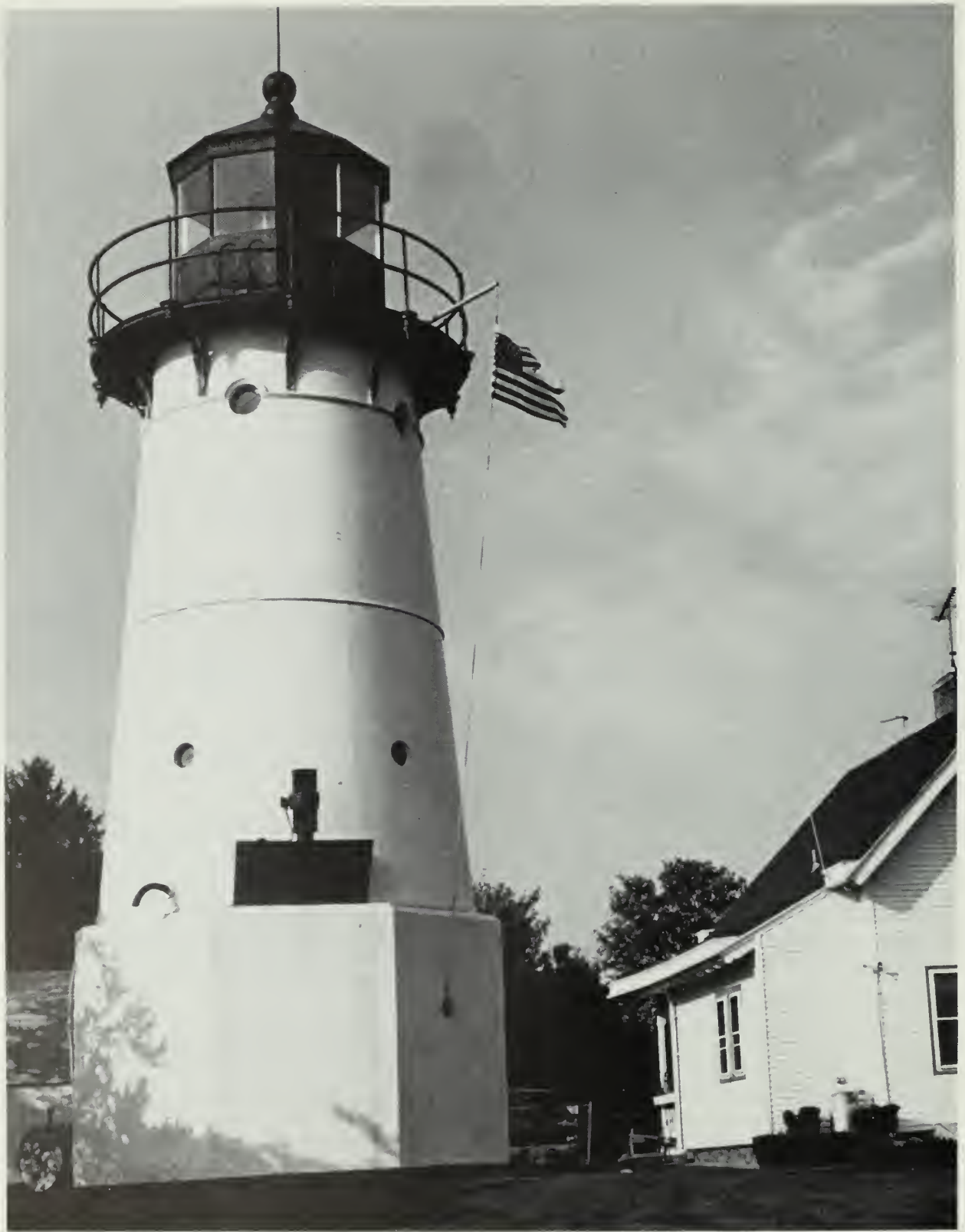
Warwick Lighthouse, Warwick, RI. This lighthouse (1932), owned by the U.S. Coast Guard which is the largest single owner of American lighthouses, was constructed of cast iron pre-fabricated components in use since the 1880s and described in the documents of the U.S. Lighthouse Service. Photo: Eugene Wick York, Rhode Island Historic Preservation Commission.
