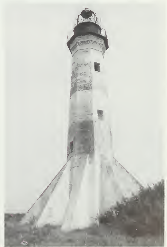
Sabine Pass Lighthouse, Cameron Parish, LA. This octagonal brick lighthouse tower (1856), owned by the State, was constructed with flared buttresses at the base to distribute the concentrated bearing load in this predominantly marshy, unstable soil. The State has received a grant from the Bicentennial Lighthouse Fund for stabilization of all exterior metal work. Photo: Louisiana Division of Historic Preservation.
