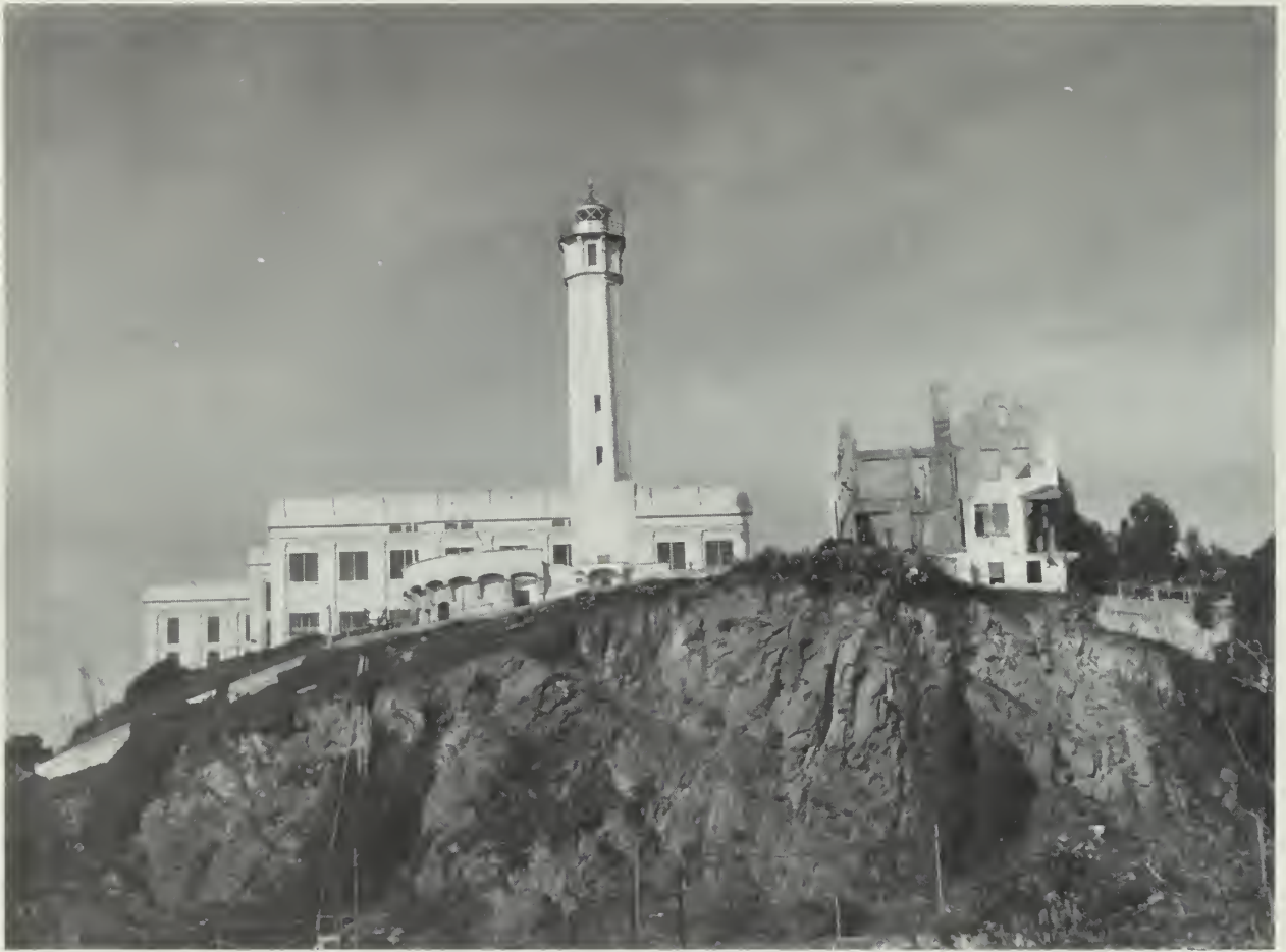
Alcatraz Lighthouse, San Francisco, CA. This reinforced concrete lighthouse (1909), a six-sided tower, is located on Alcatraz Island, and is part of the Golden Gate National Recreation Area, a unit of the National Park System. It was built near the site of the first U.S. lighthouse on the West Coast, which was demolished in 1909. Photo: National Park Service files.
