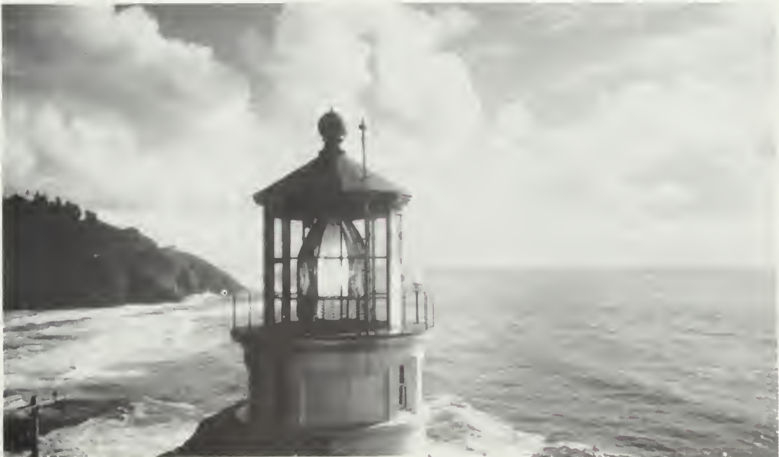
Heceta Head Lighthouse, Heceta Head, OR. This rare first order lens, installed in 1893 at the time of construction of this U.S. Coast Guard owned lighthouse, was manufactured by the Chance Brothers, England. Now automated, this million candlepower light can be seen 21 miles off shore. Photo: Lee H. Nelson, FAIA.
