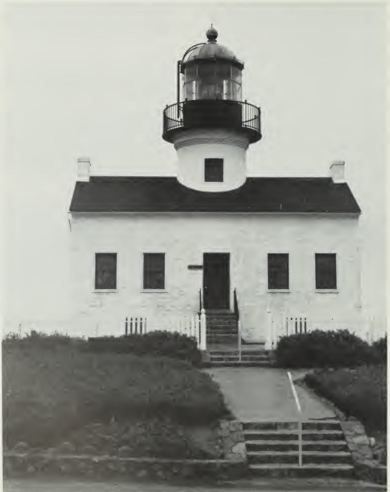
Old Point Loma Lighthouse, Cabrillo National Monument, San Diego, CA. This Cape Cod style masonry lighthouse (1854), owned by the National Park Service, was one of the first eight lighthouses constructed on the West Coast, and may be the sole remaining lighthouse of that type and vintage. It has been preserved by the National Park Service as a museum interpreting the life of 19th century lighthouse keepers and their families. Photo: Camille M. Martone.
