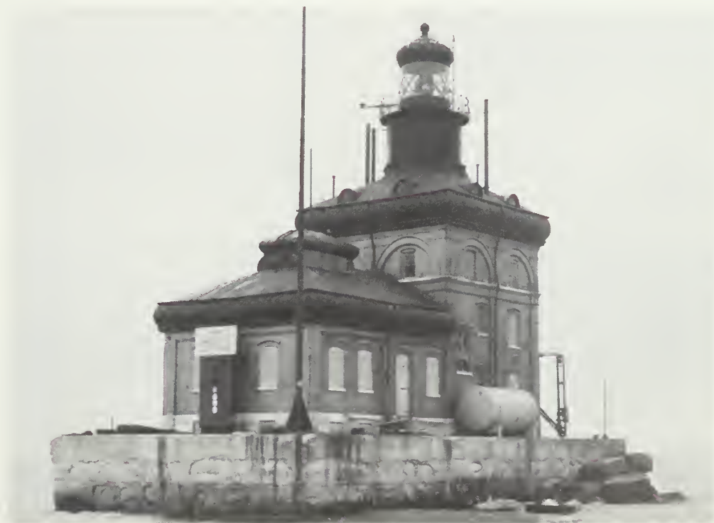
Toledo Harbor Lighthouse, Toledo, OH. This buff-colored brick lighthouse (1904), owned by the U.S. Coast Guard, was important in the development of Toledo as a port. The structural steel frame of the lighthouse sits on a concrete superstructure anchored onto a stone and gravel cribbage foundation. The original 3 1/2-order Fresnel lens is still in use and the lighthouse remains relatively unchanged since its construction. Photo: Carol Poh Miller.
