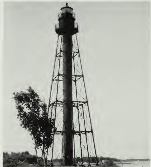
Marblehead Light, Marblehead, MA. This iron skeletal tower (1895), owned by the U.S. Coast Guard, represents an important phase in technology as lighter weight structures reached greater heights. Photo: Massachusetts Historical Commission.
