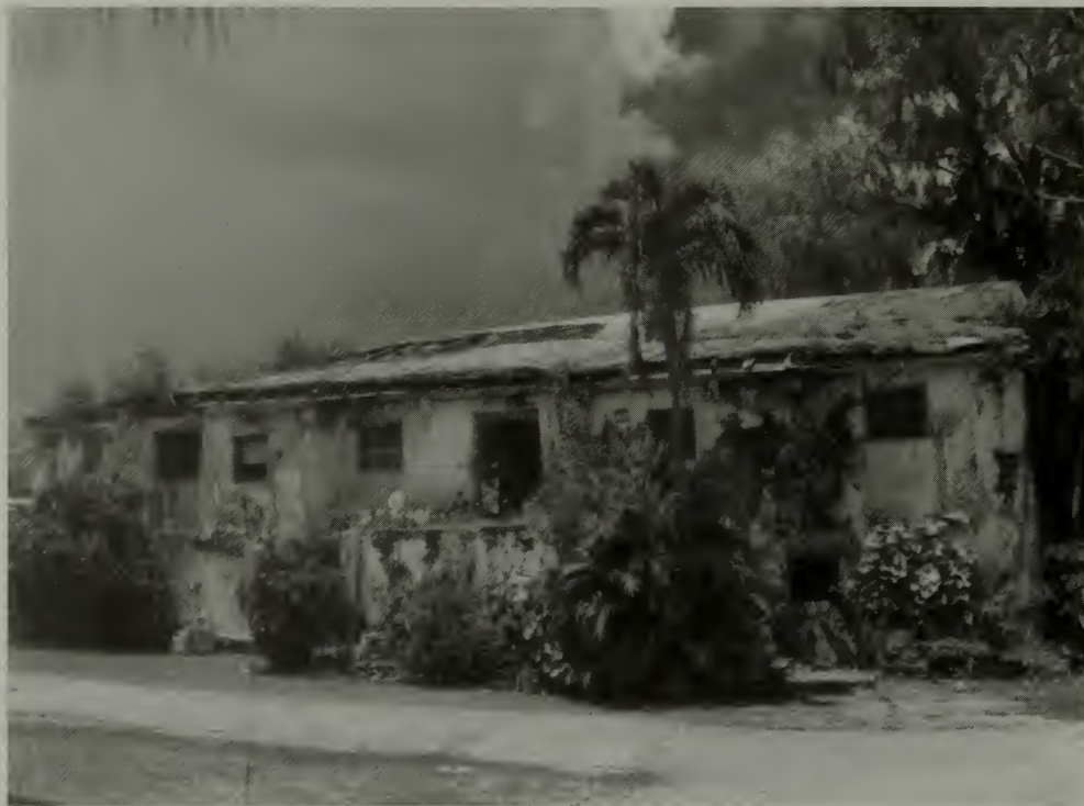
Figure 6.3. Mission Kampanayun Malessu at Merizio, Guam, severely damaged by an earthquake which occurred during Typhoon Ross in September 1992. The lack of funding to restore the structure and the wind-damaged roof saw the continued decay of a historically significant building. (Photo: Dirk Spennemann 1994).
