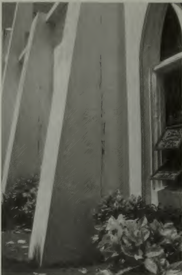
Figure 7.3. St. John's Church, Inarajan, Guam. The earthquake revealed an earlier attempt at seismic retrofitting the buttresses through reinforcement. (Photo: Dirk Spennemann 1994).
