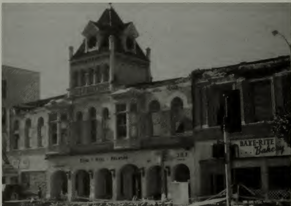
Figure 24.2. A case of retribution. The Oddfellows Fraternal Hall, Watsonville, CA, was damaged during the 1989 Loma Prieta earthquake, the falling parapet masonry killing a pedestrian. Although repairable, the building was quickly demolished a few days after the disaster. The tower is a wood frame construction with metal covering and did not fail during the earthquake event. (Photo: Steade Craig 1989).
