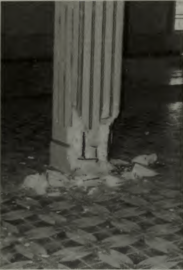
Figure 7.2. St. John's Church, Inarajan, Guam. Minor damage to reinforced concrete column. This damage is repairable and should not result in the loss of a historically significant structure. (Photo: Dirk Spennemann 1994).
