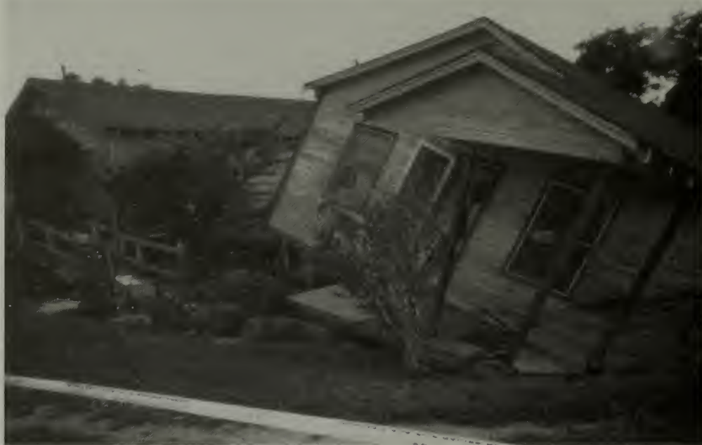
Figure 20.3. Historic home in Albany, Georgia, following Tropical Storm Alberto in July 1994. The flood waters washed out part of the foundation all causing the collapse of the wooden structure (Photo: Jim Lockhart 1996).
