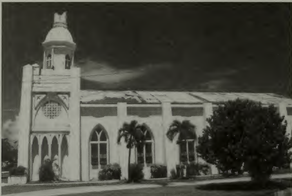
Figure 7.1. St. John's Church, Inarajan, Guam, severely damaged in September 1992 by the dual effects of Typhoon Ross and an earthquake which occurred at the same time. This church is one of the few buildings surviving from the pre-World War II period of Guam and has a very high cultural and historic significance. Note toppled spire ornament and missing roof sections. (Photo: Dirk Spennemann 1994).
