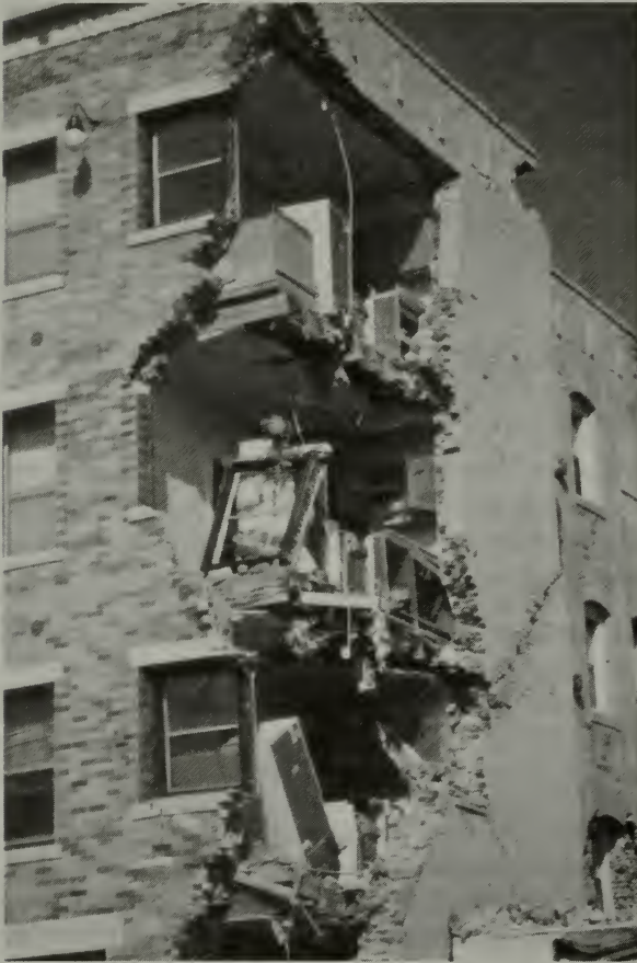
Figure 3.1. Unreinforced masonry apartment building in Hollywood (CA) showing typical earthquake damage at the corner. A completed seismic retrofit would have prevented such heavy damage. Northridge Earthquake 1994. (Photo: Steade Craigo 1994).
