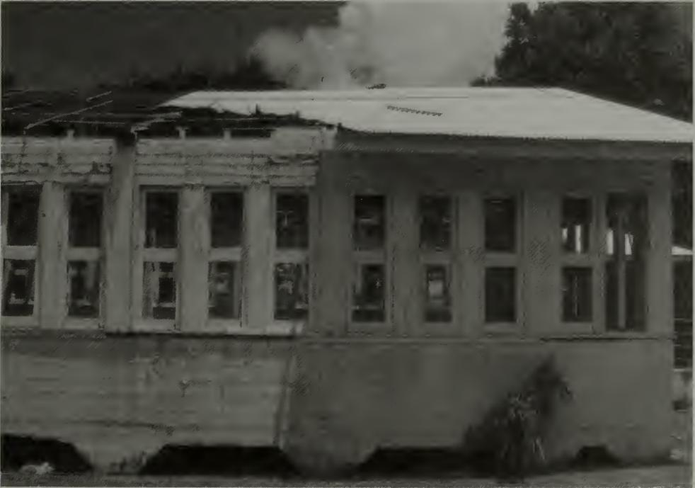
Figure 6.2. The historic school building at Merizio, Guam, severely damaged during Typhoon Ross in September 1992. Note the decay at left brought about by the loss of the roof and subsequent exposure to tropical sun and rain. (Photo: Dirk Spennemann 1994).
