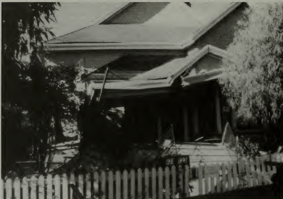
Figure 17.3. A private residence in Santa Cruz, CA., following the 1994 Northridge Earthquake. Wood frame residential structures were commonly damaged when the foundation cripple walls collapsed. (Photo: Steade Craigo 1994).
