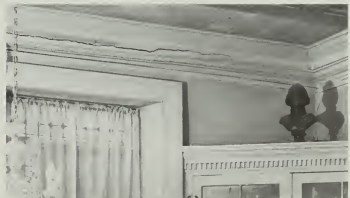
Figure 18. The major crack along this cornice indicates that there has been long-term moisture problem in this room. Restoring the plaster work and repainting should be done only after the water problem is solved. Photo: Jack E. Boucher for HABS.
