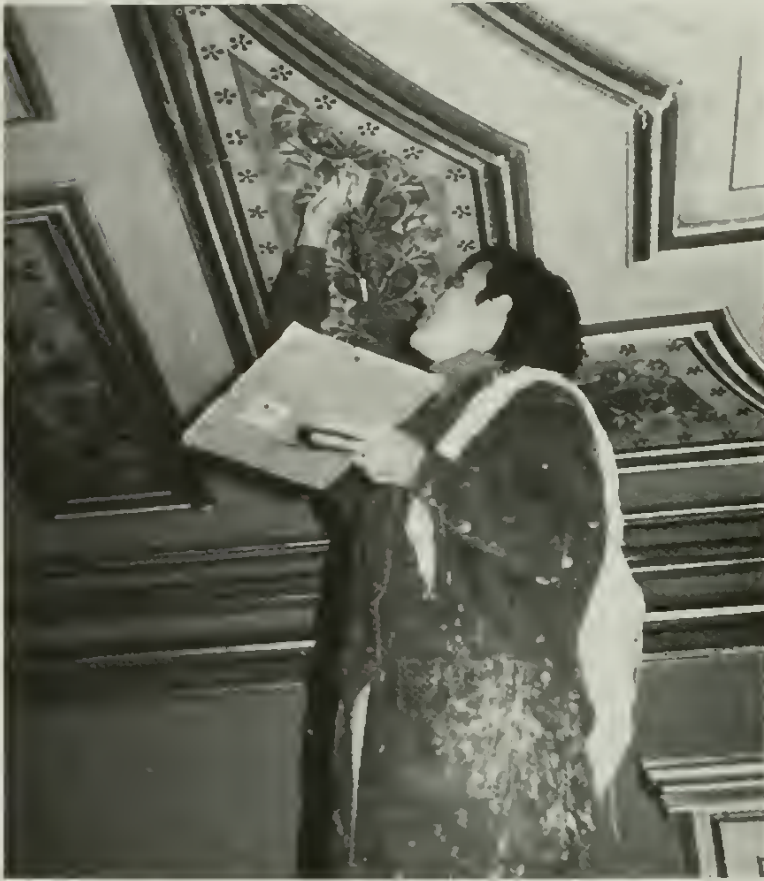
Figure 22. Traditional water-based paint and artists' brushes are being used to reproduce historic finishes within a restoration project. Photo: Courtesy, Alexis Elza.
