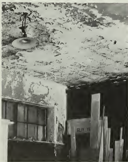
Figure 13. Part of a historic freight depot, this is not a high-style room and its painted surfaces are obviously in poor condition from long-term neglect. Interior spaces that are being converted for a new use in rehabilitation projects can benefit from being repainted in historic period colors rather than a neutral off-white. Photo: National Park Service files.
