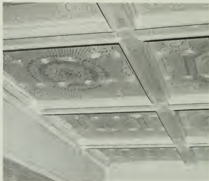
Figure 14. Holes left by insertion of toggle bolts used in the structural strengthening of this ceiling can be seen in the decorative plaster work. Without great expense, a skilled painter can now clean and touch up the damaged areas. This type of targeted repair work can benefit both public and private buildings. Photo: National Park Service files.
