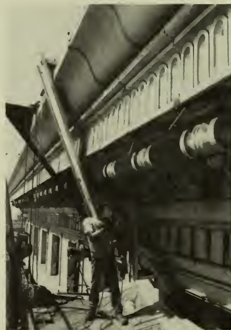
Figure 9. Drilling 6' long vertical holes through the cornice, in a variety of materials, was a delicate operation requiring great skill and specialized drilling equipment. The aluminum drilling jig provided the precise alignment needed to drill the holes for the vertical and angled bracket anchors. Drilling of a vertical anchor is shown. To create an angled outer scroll anchor hole, the drill was mounted on the angled portion of the jig, which passed directly in front of the bracket. Hand-drilled holes could be completed in 15-30 minutes, depending on the depth of the hole and the type of backup material encountered (e.g., brick, terra cotta, light-weight concrete, steel). Holes drilled with the jig required more time, 30-60 minutes, as alignment was more critical and it took time to set the jig in the proper position. Photo by Jeffrey S. Levine.
