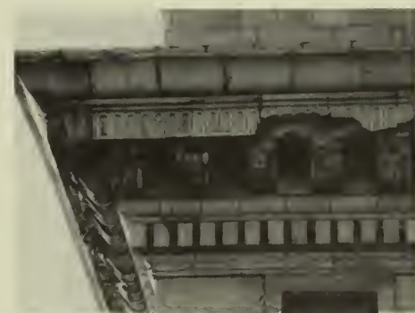
Figure 4. Extreme loss of material was noted in the scalloped fascia above the brackets at the south end of the east elevation of the cornice. This deterioration and corresponding cracking in other fascia units was due to rusting of the structural steel angle iron which supports the fascia units at their center webs (see figure 1). A likely point of water entry was a large open joint located immediately above the fascia, at the bed joint of the cyma recta units. Photo by Jeffrey S. Levine.
