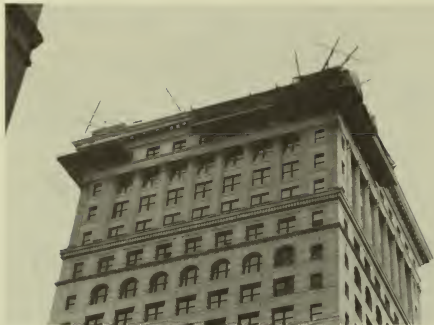
Figure 8. Access to the cornice was provided by cantilevered aerial scaffolds at the southeast and southwest corners of the cornice. All other locations were accessed by hanging two swing stages, side by side. The inner swing was hung off of a V-shaped bracket (shown) while the outer swing was hung from a steel deadman which projected horizontally across the cornice roof. Both the V-shaped bracket and the deadman were designed to transfer the weight of the swings vertically down through the center of the cornice. No load was placed on the outer edge of the cornice. Photos by Jeffrey S. Levine.
