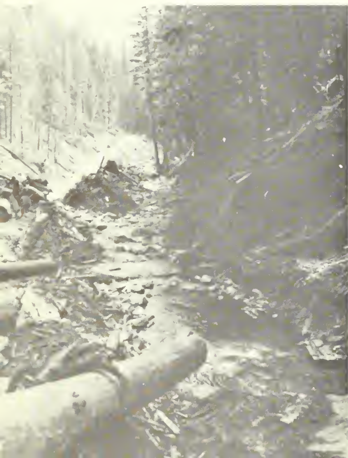
Figure 7.--This road was built too close to the stream channel. It reduced channel capacity and created a direct source of sediment for the stream.
