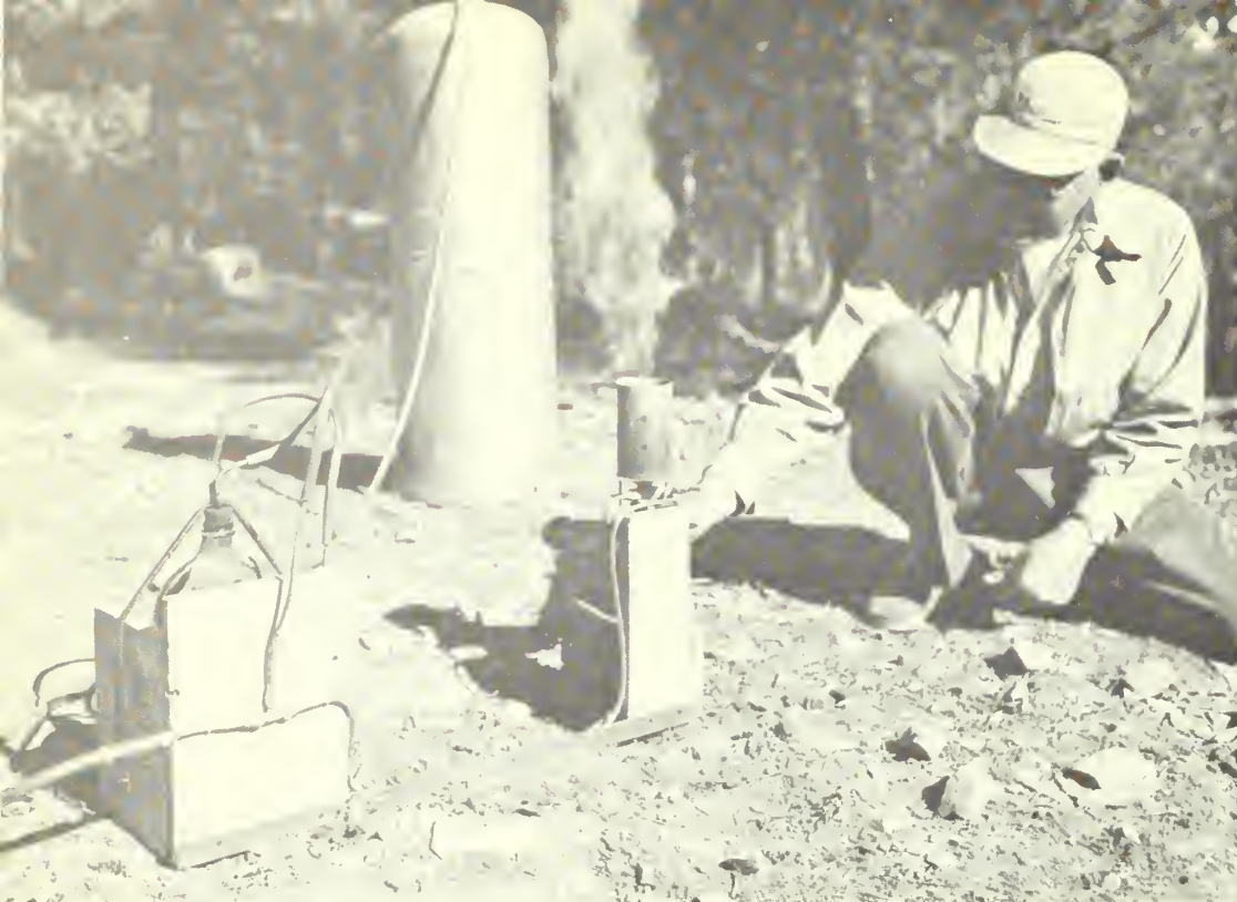
Figure 1.--Acetone-burning silver iodide generator.
