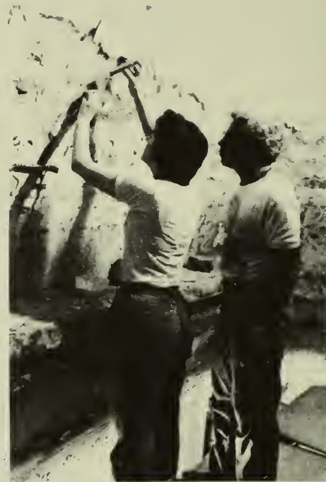
Carole Perrault (left), architectural conservator, North Atlantic Historic Preservation Center, and Paul Schwartzbaum (right), conservator from the International Center for the Preservation and Restoration of Cultural Properties, are shown reattaching gypsum wash to the interior surface of the mission church's dome.
