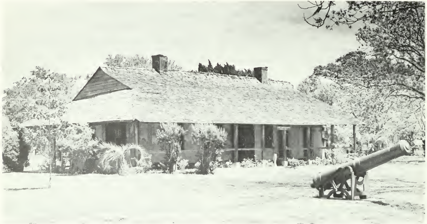
Old Spanish Fort (Old French Fort), Pascagoula, Jackson County, Mississippi. Built c. 1721, this building is frame construction with plastered oyster shell concrete fill. Originally part of an early French land grant, this building is believed to have been part of a palisaded complex built for the defense of early settlers. (Photo by: Hinman Advertisers).
