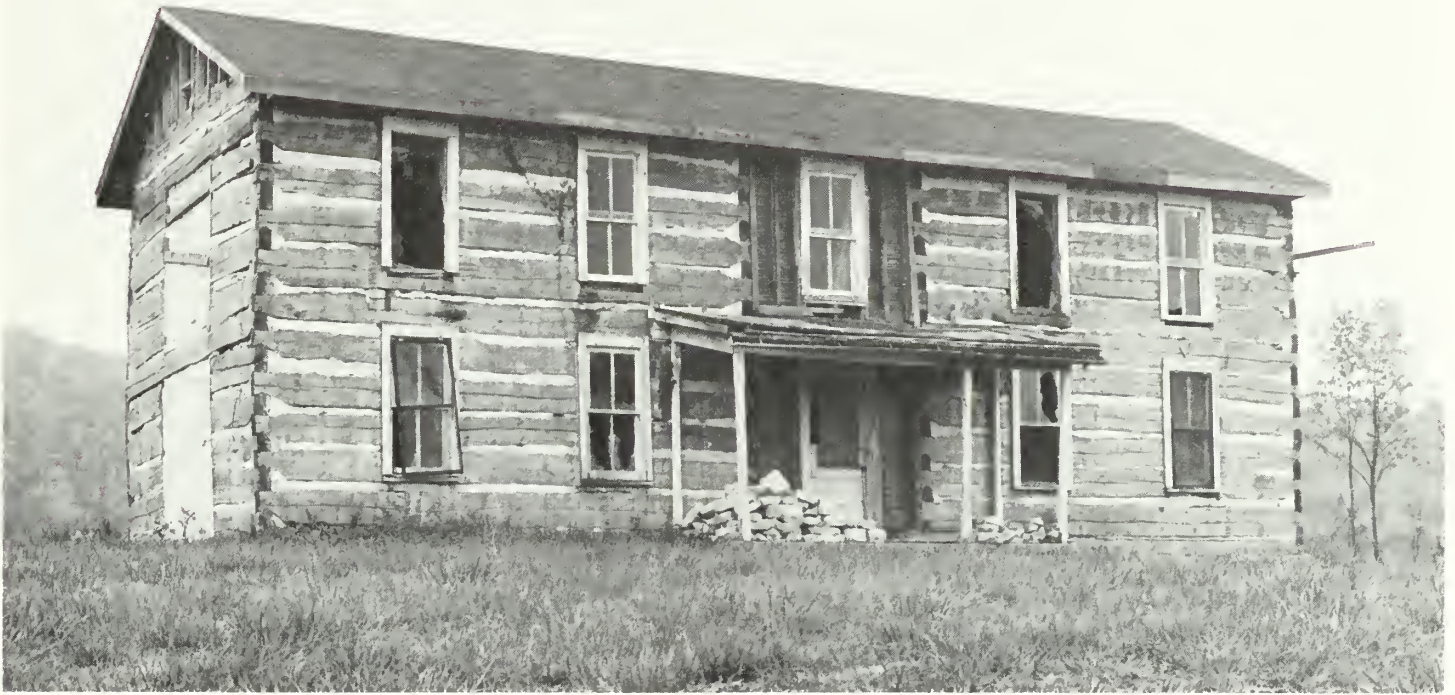
The Andrew Trumbo Log House, Frankfort, Franklin County, Kentucky. This two story dogtrot type log house, constructed c. 1810, is an example of an important vernacular type of early residential construction in Kentucky. (Photo by: Don Snively).
