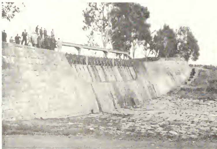
Below left: Grotticelli Dam, Sicily. Lower part built by the Arabs in the 12th Century; remodeled and raised in 1563; remodeled in 1926; silted up but still useful for irrigation diversion. Below right: Small bunches of straw used to prevent wind erosion, east of Zapponita.
