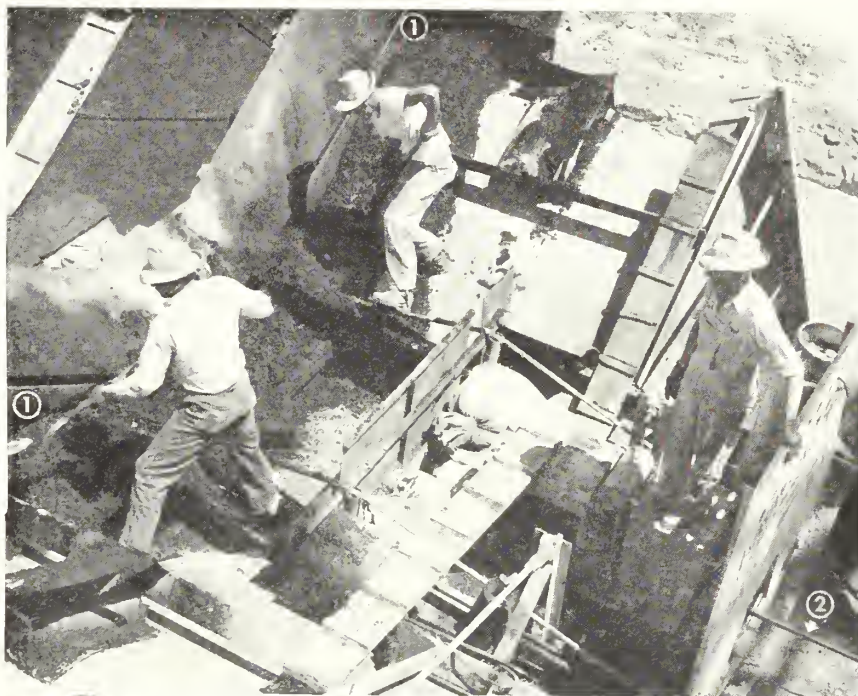
Above: Inside the asphalt lining machine, showing operators guiding the asphalt mix into the pan below the strike-off blades (1). The cable (2) is also shown. At left: In the wake of the paver, showing the other side of the screeds, or strike-off blades (1), and the hot irons (2) used to give a surface seal. Both photos by A. F. Swanson, Columbia Basin project.
