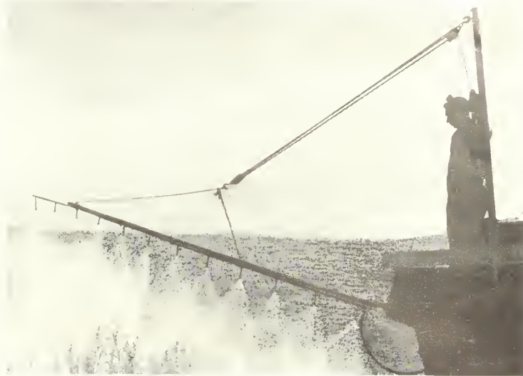
A spraying machine in operation along one of the canals of the Black Canyon Division of the Boise project near Notus, Idaho, using a 2,4-D mixture of weed killer. Photo by Philip Merritt, Region 1.
