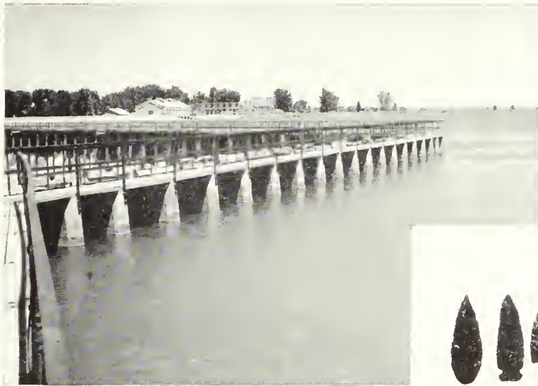
Above: Minidoka Dam on the Minidoka project located on the Snake River in Idaho was constructed in 1909. Dam is of rock-fill, faced on upstream side with impervious earth-fill, and creates reservoir known as Lake Walcott, with storage capacity of 107,240 acre feet. The power plant has 7 generators with a kilowatt rating of 13,400.
