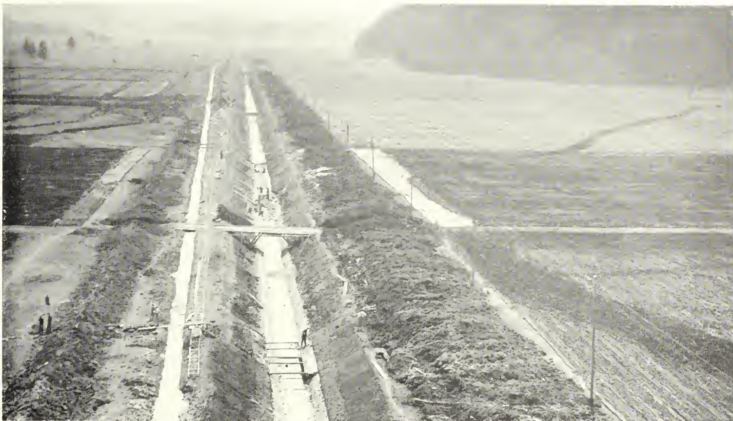
Rapid procedure of Switzerland's reclamation program. Background—excavation of main drainage canal; middle—tile drainage; foreground—cultivation of drained land.
