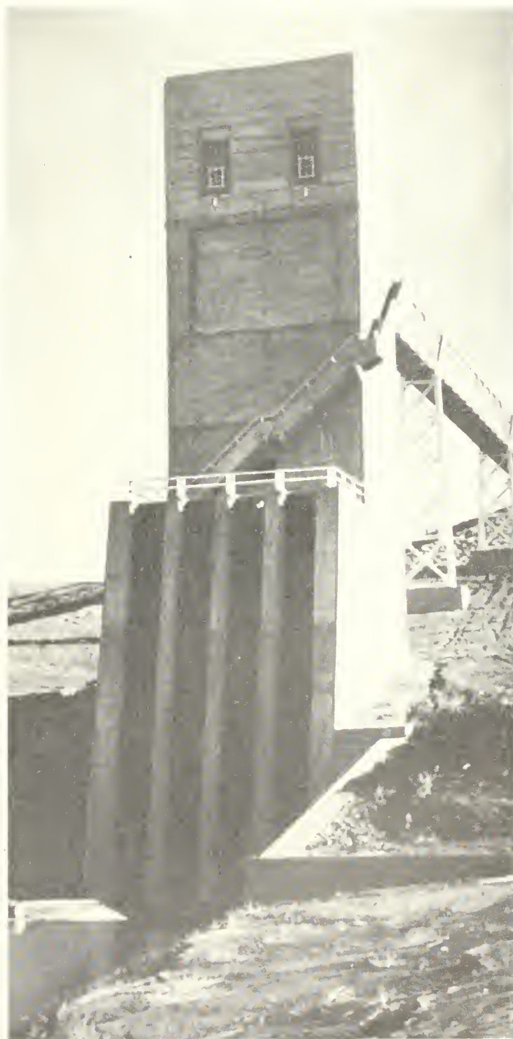
Intake tower, Kanopolis Dam, Kans., now under construction by the Corps of Engineers.
