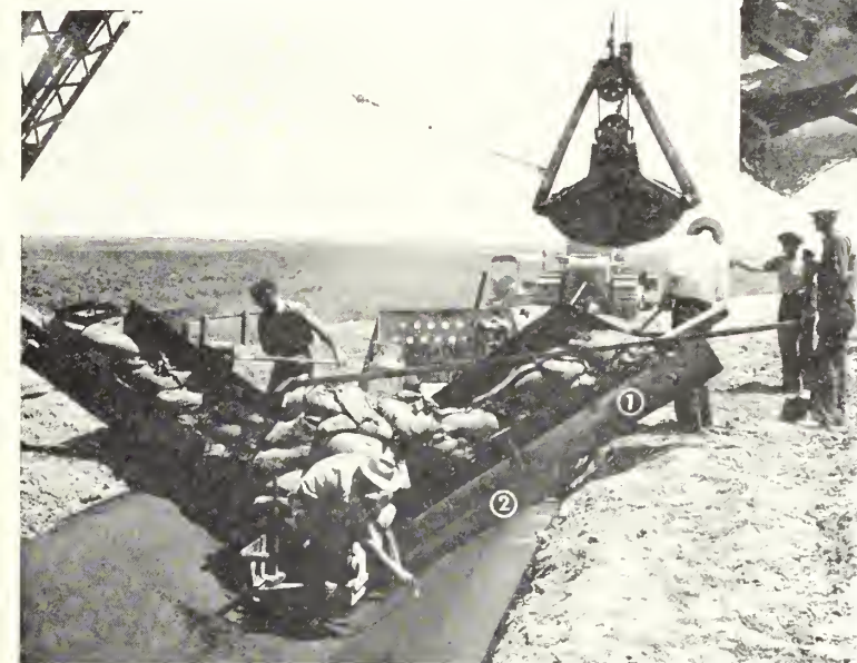
Above: Inside the asphalt lining machine, showing operators guiding the asphalt mix into the pan below the strike-off blades (1). The cable (2) is also shown. At left: In the wake of the paver, showing the other side of the screeds, or strike-off blades (1), and the hot irons (2) used to give a surface seal. Both photos by A. F. Swanson, Columbia Basin project.
