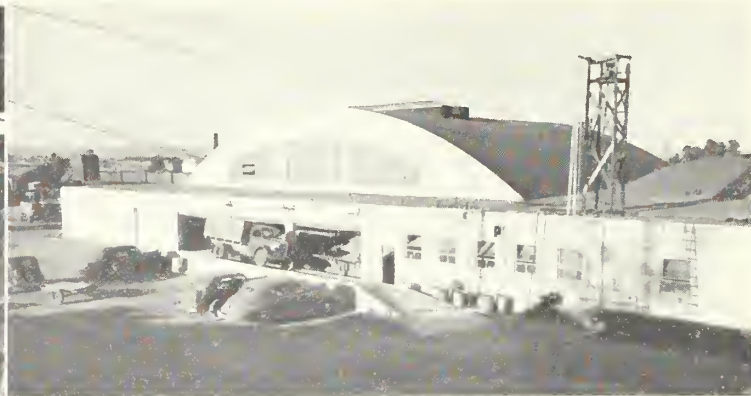
Left, interior of new packing plant at Yuma. In center foreground is sorting table and left, roller stamping machine which trade-marks fruit. Above photo shows exterior of packing shed with conveyor belt handy to trucks, left bodyside of which is unhinged, creating shoot direct to belt. Photos by Harry W. Myers and Samuel B. Watkins, Region III.
