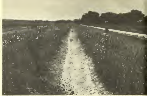
Left, view of an irrigation lateral in the Bostwick Irrigation District near Superior, Nebr., which is choked up with grass type weeds. Right, view of an irrigation lateral in the Bostwick Irrigation District near Superior, Nebr., taken at the end of the season to show effects of the wetted perimeter having been treated with soil sterilant. Photo by G. C. Lynn.
