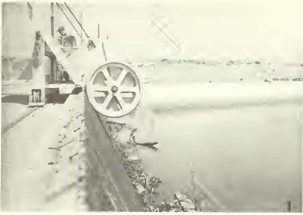
DELTA-MENDOTA CANAL —Side view of trash rake on trash rack structure.—All photos in this article, except otherwise noted, by J. L. Brown, Region 2.
