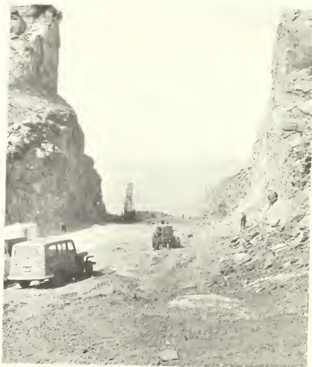
Most spectacular part of all road construction for the Glen Canyon Dam is this 300-foot cut through the Echo Cliffs near Bitter Springs, Ariz.—Photo by Fred S. Finch, Region 4.
