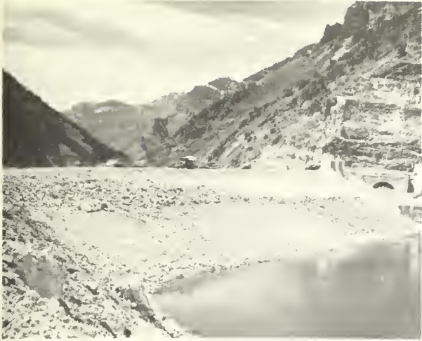
ENLARGEMENT of Pineview Dam—Weber Basin—Utah. Highway tunnel near the right margin of the picture, now filled with rock identifies the original height of Pineview Dam—Photo by Stan Rasmussen.
