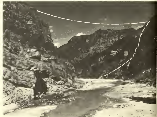
Diversion tunnel outlet, Flaming Gorge Dam. Outline is sketched on picture.
