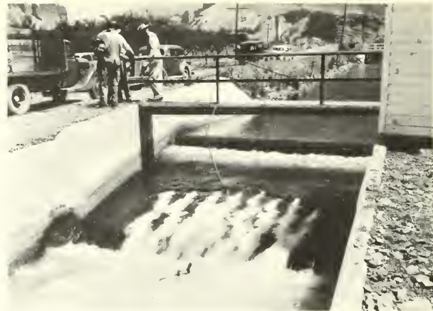
Treating aquatic weeds by admitting a commercial weed killer within a Parshall flume.
