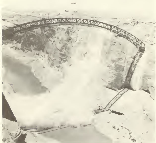
Completed arch. Billow of smoke resulted from blast set off to signal the closure of the two half arches.
