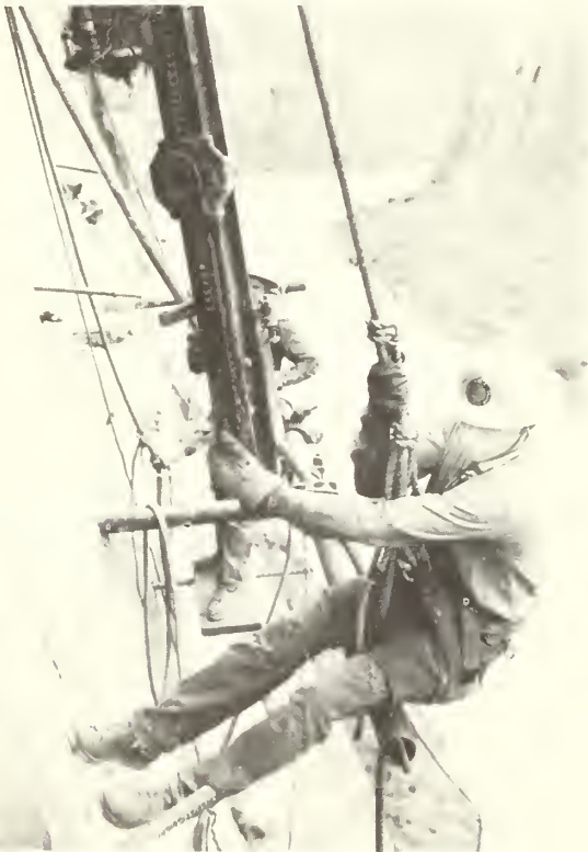
High-scaling brothers, W. D. Jackson, front, and J. R. Jackson, of Mesa, Ariz., drill out the skewbacks for the Colorado River bridge at Glen Canyon. They work some 200 feet down the canyon wall suspended by cables.—Photo by F. S. Finch, Region 4.
