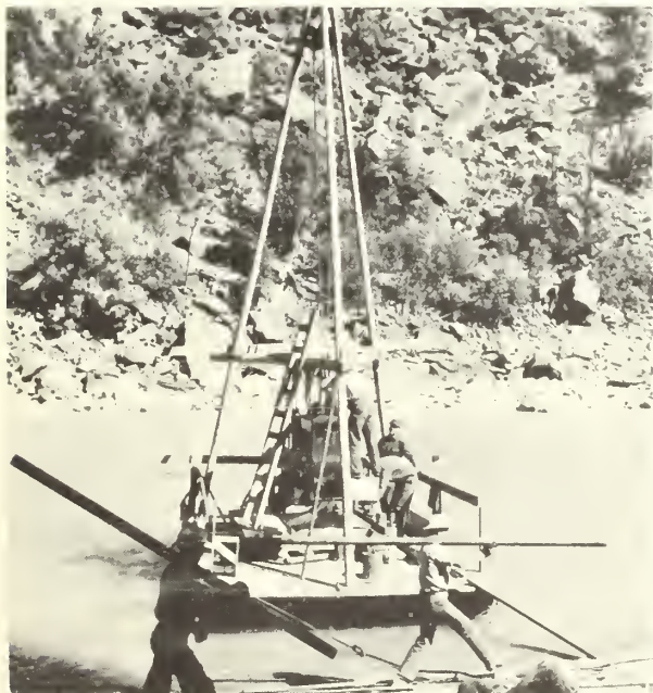
Diamond core drill operating near axis of Flaming Gorge Dam site. Photo by F. H. Anderson, Region 4.
