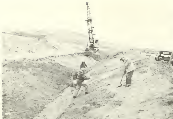
Preparation of the subgrade for lining.
