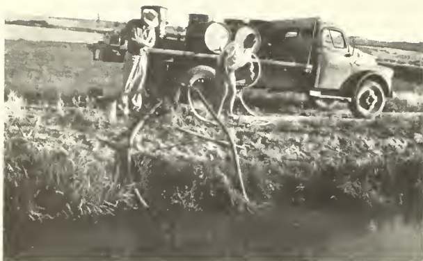
Left, application of experimental herbicide, F98, for pond-weed control, Notus Canal, Black Canyon irrigation district, Notus, Idaho. Right, cutting and removal of pond-weeds by hand.
