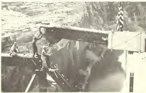
Key chord being lowered into position. Photo by J. L. Digby, Region 4.
