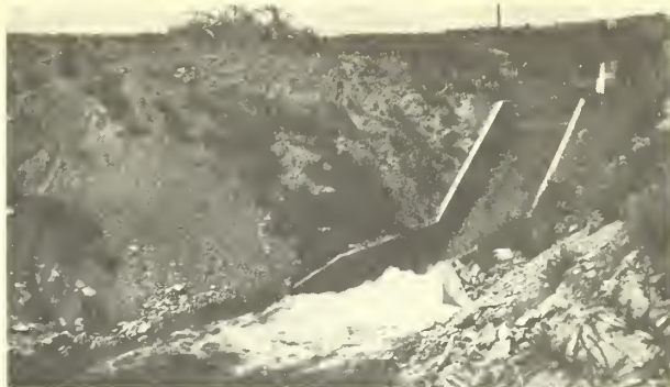
Figure 4.—View of new concrete chute installed spring of 1955. This structure replaced the old drop. The discharge of 125 cfs is one-half the design discharge.
