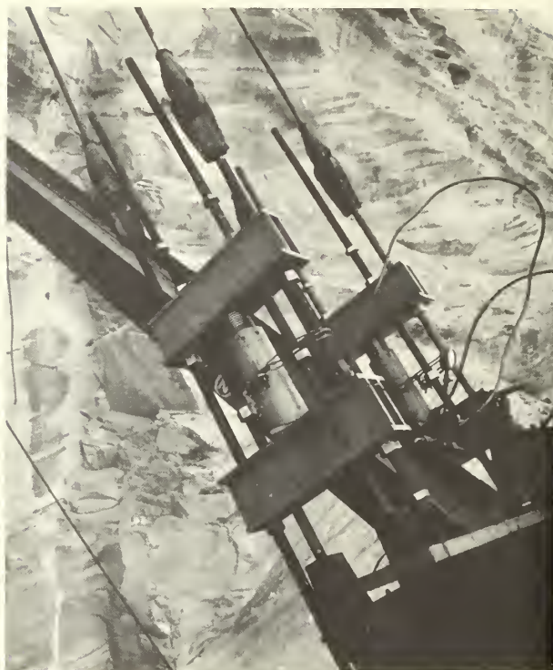
Picture shows detail of the tiebacks with the sections for distributing tension in place.
