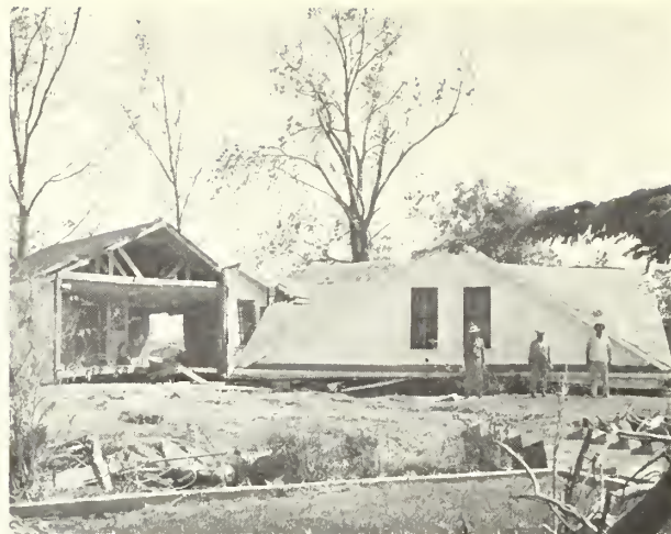
A BREAK OF THE STORM —This fully gabled roof settled relatively undamaged on the ground after losing its ground floor.
