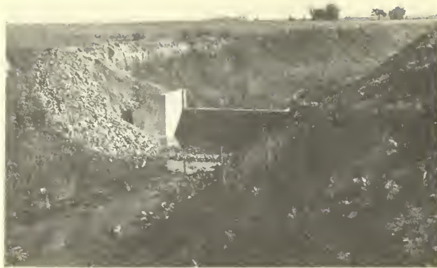
Figure 6.—View of Overall Drop Structure No. 2 shortly after construction in 1955. Energy is dissipated by the pre-formed gravel-armor-plated scour hole. Notice, however, that the coarse portion of the specified armorplating material was not installed.
