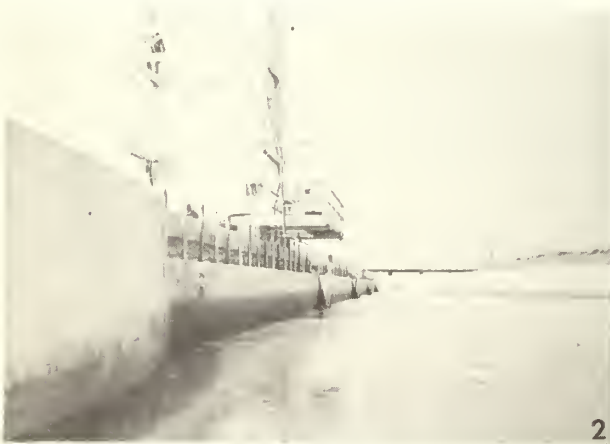
View of primary louver looking downstream. Hoist is used to raise louvers.
