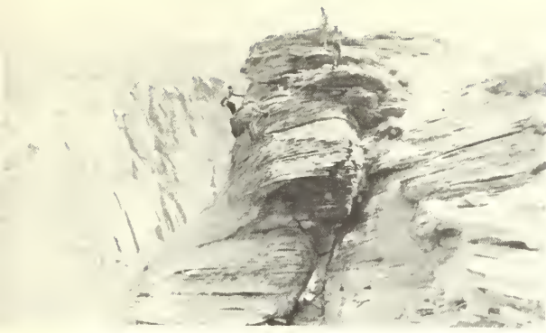
HIGH SCALERS going over the top of right abutment—Glen Canyon Dam site.
