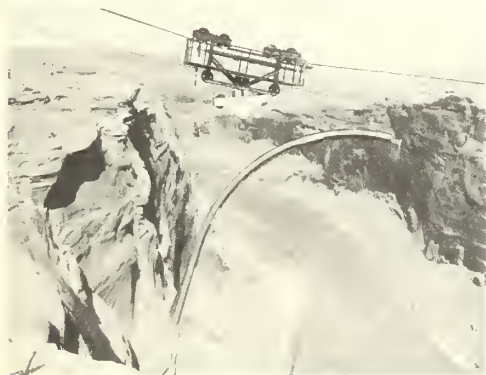
Steel ribbing being lowered 700 feet to bottom of canyon for use in right diversion tunnel. Photo by F. S. Finch, Region 4.
