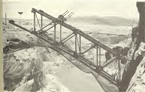
First 4 panels of steel being set on the right bank or east side of Glen Canyon.
