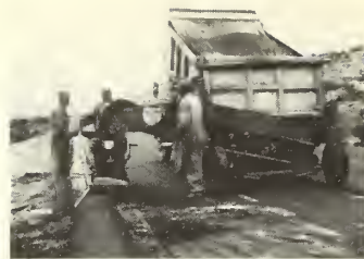
Installing curbing on Bitter Springs—Page access road.
