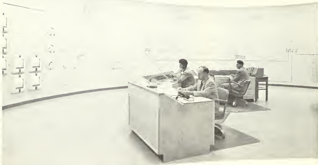
Parker-Davis System Dispatchers' Office—View of the "system diagram board," which pictures the major segments of the entire system with Hoover powerplant at the upper right and the Yuma-El Centro area at the lower left of the diagram.
