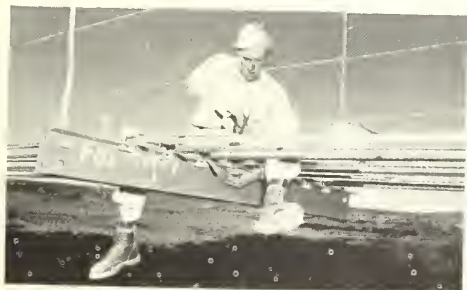
Steel rigger Bill Wilds bolts floor cable locks in place on the foot- bridge spanning Glen Canyon of the Colorado River—Photo by A. E. Turner, Jr., Region 4.
