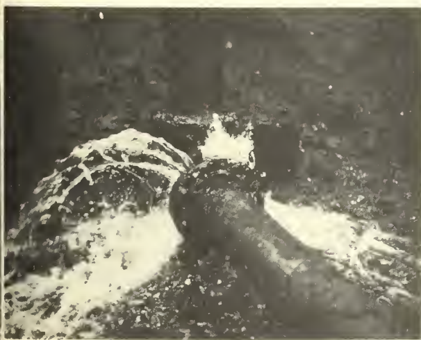
Ogden City Artesian Well No. 36 showing water gushing from break at tee.
