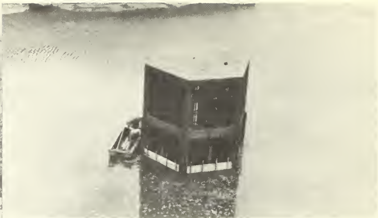
At left: Trashrack structure at Alamogordo Dam during original construction in 1937. Above: Shows method of bulkheading off flow through trashrack.
