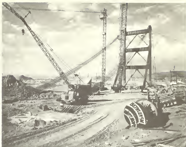
L. to R.: Truck crane servicing job, head tower of 12 ½-ton cableway, tail tower of 25-ton cableway, and tieback tower.
