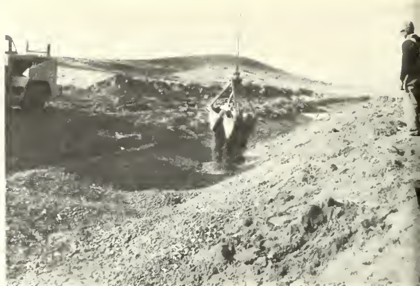
Gravel cover is hauled to site and removed from truck with clam shell bucket and placed in the canal section in one operation.
