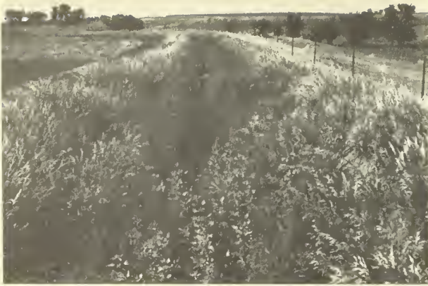
Left, view of an irrigation lateral in the Bostwick Irrigation District near Superior, Nebr., which is choked up with grass type weeds. Right, view of an irrigation lateral in the Bostwick Irrigation District near Superior, Nebr., taken at the end of the season to show effects of the wetted perimeter having been treated with soil sterilant. Photo by G. C. Lynn.
