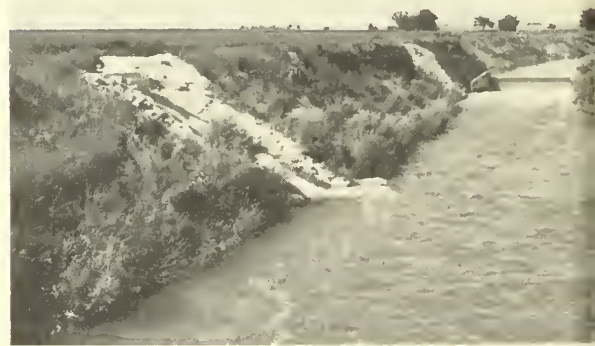
Figure 7.—View of Drop No. 2 in operation two years after construction. The discharge shown is 184 cfs. Notice the rock-plastered spillway for discharging wastewater into the channel from adjacent fields.
