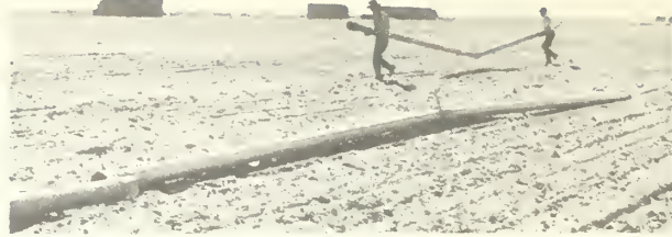
Six-inch aluminum pipe in 20-foot lengths is used for sprinkler line. Two men move one-half mile of pipe from one setup to another in approximately 50 minutes, moving two joints at a time.
