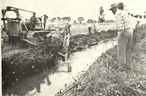
Demonstration of a Briscoe sloper, shown sloping the banks and clearing weeds on a lateral on Garland division.
