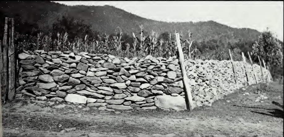
Poles were used at John Oliver's Cades Cove farm to line up the wall as it was built.
