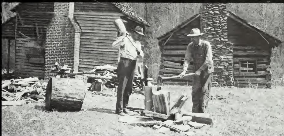
With a mallet and ax, Tom and Jerry Hearon split logs into bolts from which to make shingles.
