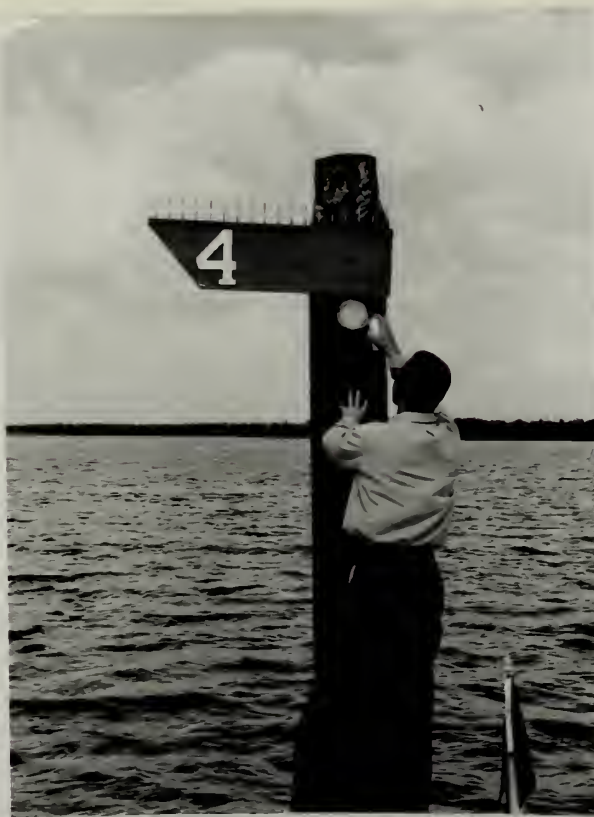
Fig. 6 Installation of new channel markers and pointers in North channel going into Lostman's River.
