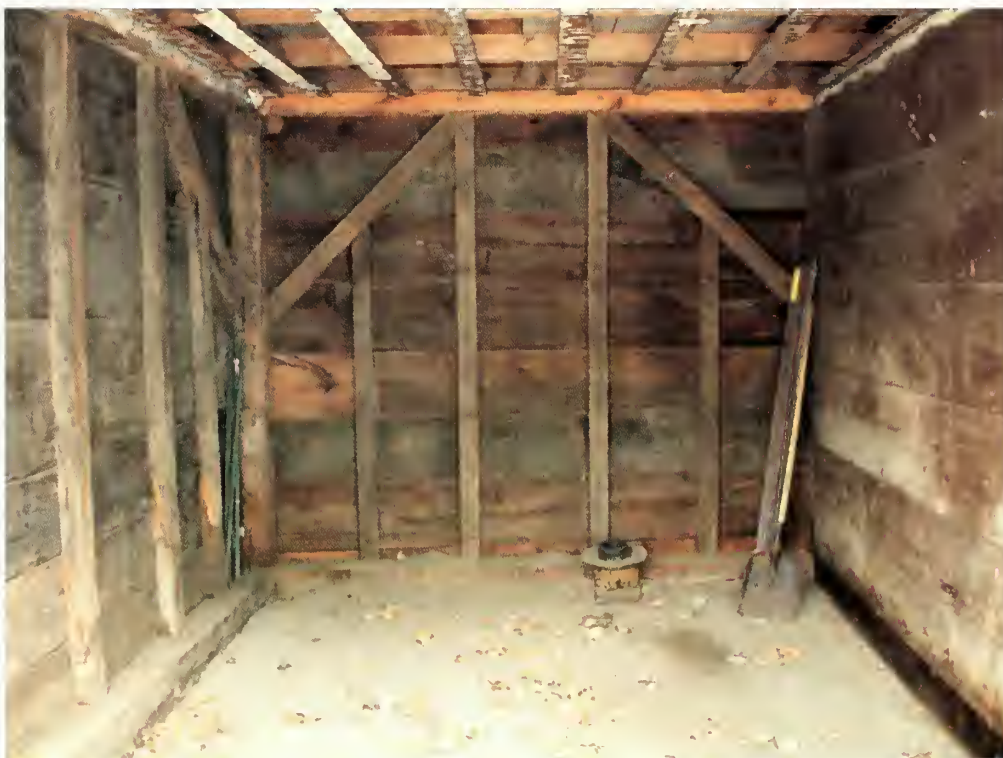
Figure 63. Elisha Jones Shed: Chaise stall, north and east walls, exposed framing including 1974 replacement sill and east girt, spliced studding and corner post, and bracing (2006).
