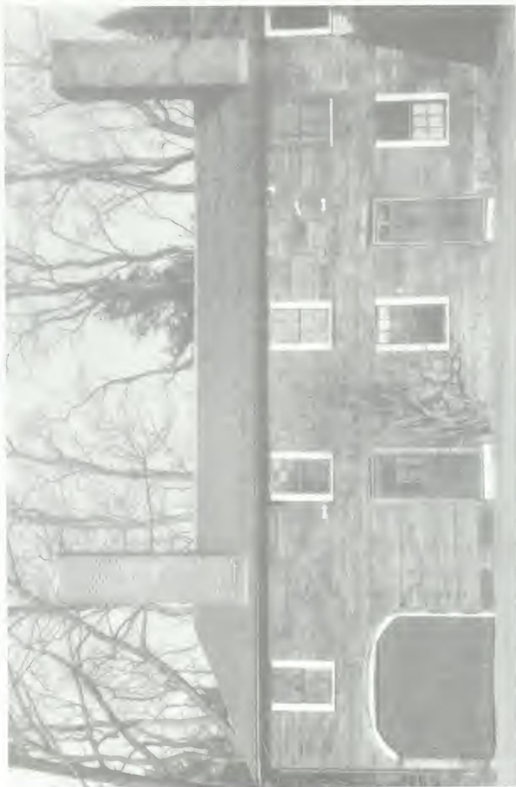
Figure 18. Elisha Jones Shed: West elevation, with arrows indicating evidence of original window openings. The left window (W/224) was reused by John Keyes, and the right one was boarded over in 1865.
