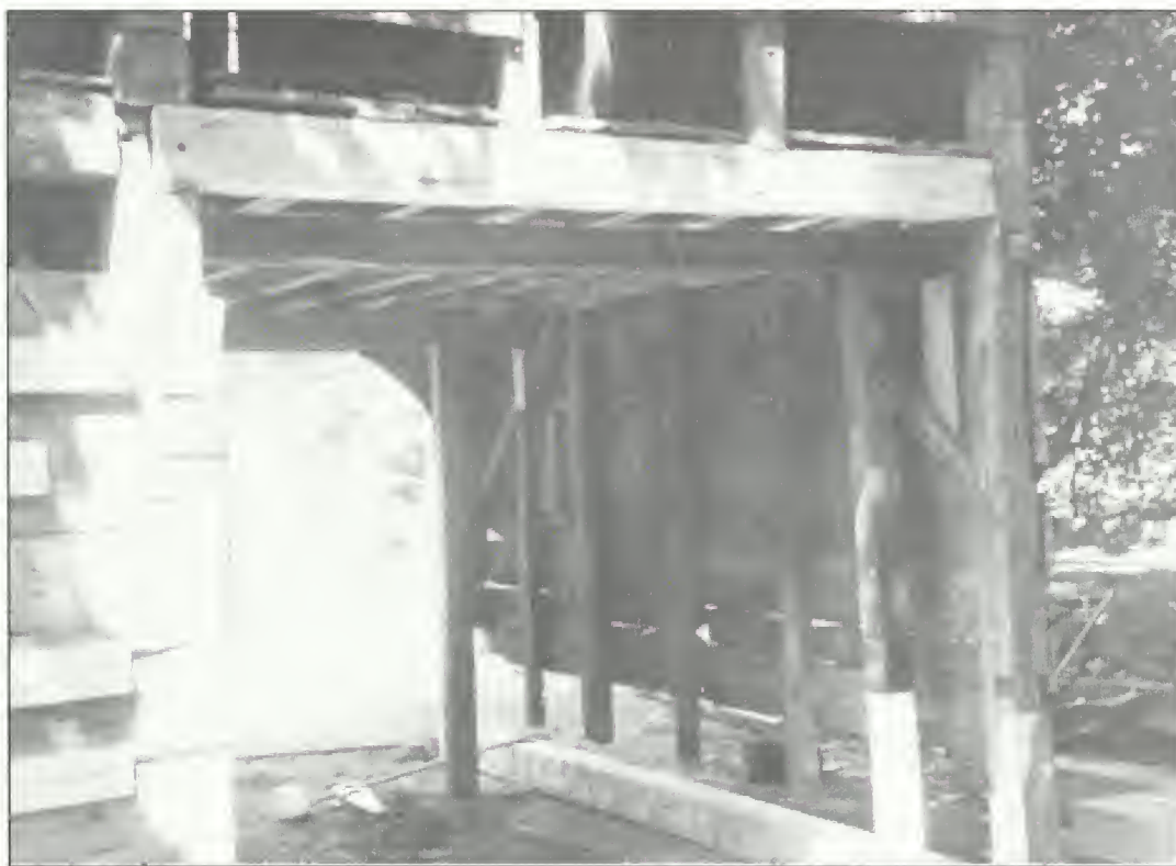
Figure 35. Elisha Jones Shed: East and north wall repairs, including replacement of east- wall girt and north- wall sill, and splicing of posts and studs, 1974.
