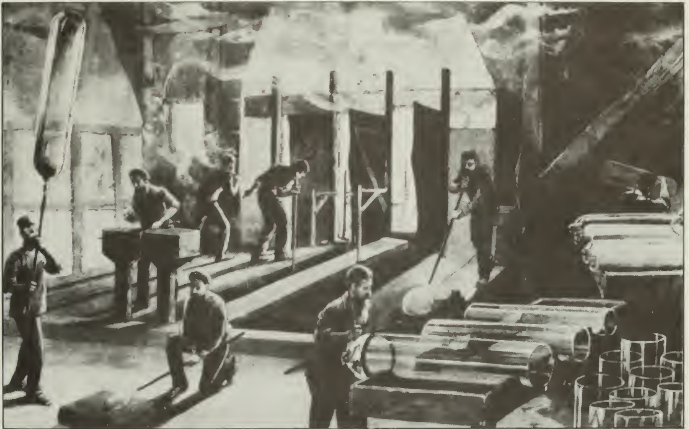
Figure 121. Cylinder or Broad Glass Manufacture. (Wood engraving from "Scenes in a Glass Foundry," by Theo. R. Davis, Harpers Weekly, January, 1884. Reproduced in Wilson 1976:151.)
