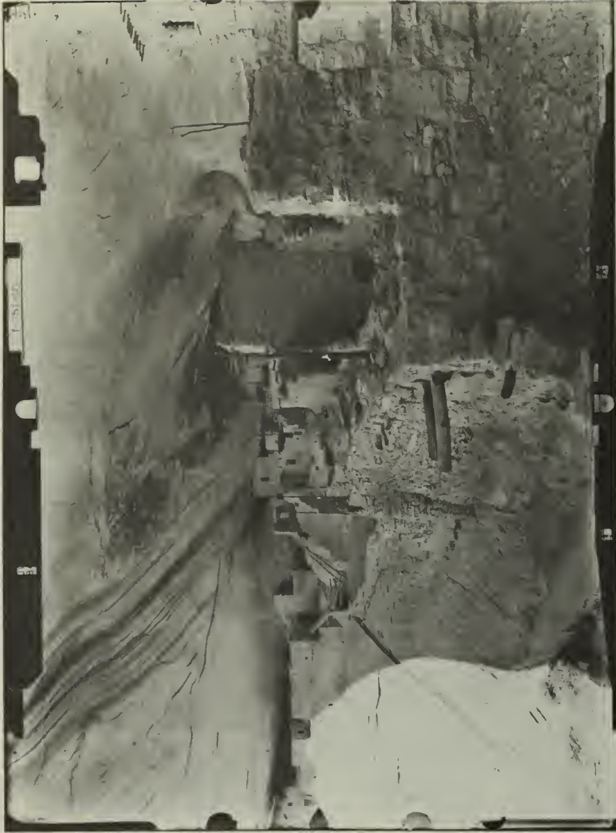
Figure 69 - Right photograph of photogrammetric stereopair within Keet Seel ruin. Taken with Galileo-Santoni phototheodolite, focal length elongated to 151.66 mm, 13 x 18 cm format. Base distance to left camera station 5.42 ft. Camera axis level. Left camera station is the basis for survey control horizon markings of tape. Photograph by Perry E. Borchers.
