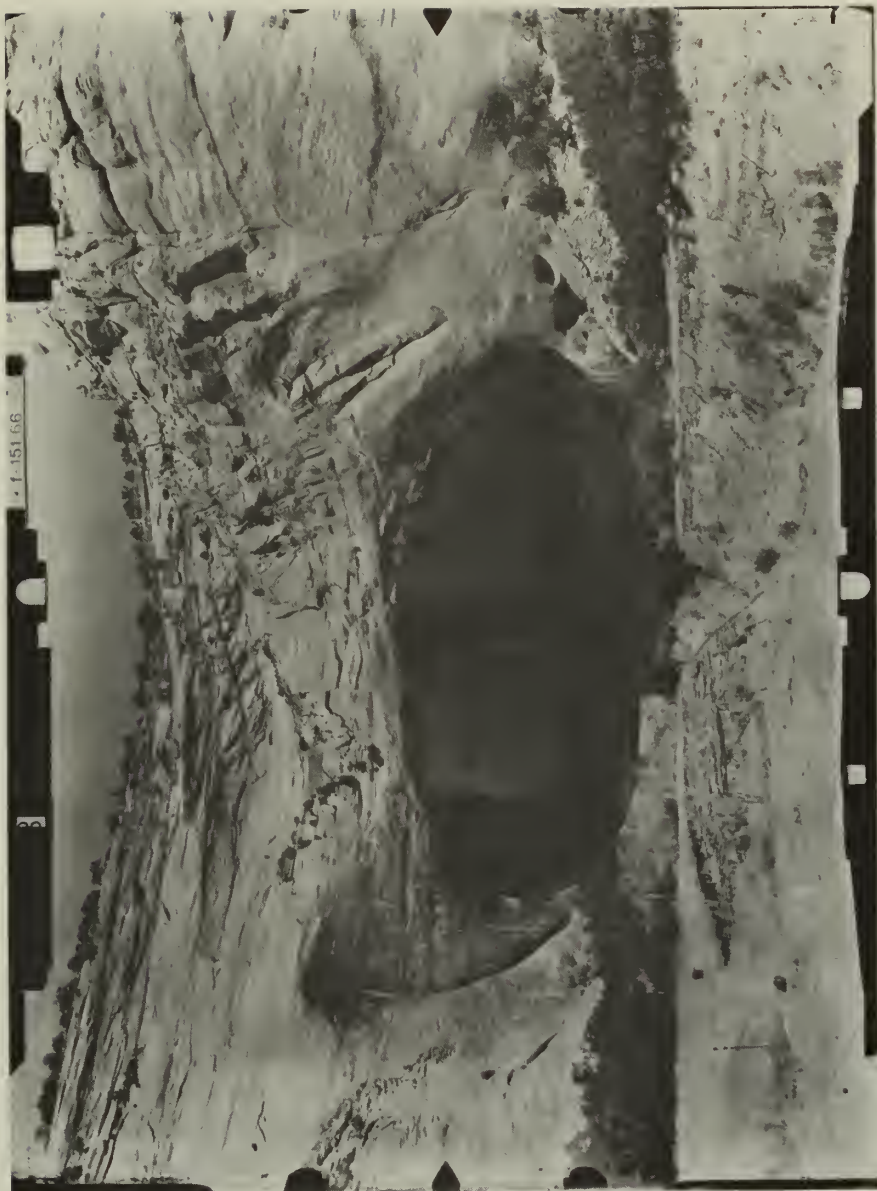
Figure 70 - Right photograph of photogrammetric stereopair of Keet Seel from valley floor approximately 650 ft. in front of cliff opening. Taken with Galileo-Santoni phototheodolite, focal length 151.66 mm, 13 x 18 cm format. Base distance to left camera station 57.21 ft. Camera axis angled upward 15°. Photograph by Perry E. Borchers.
