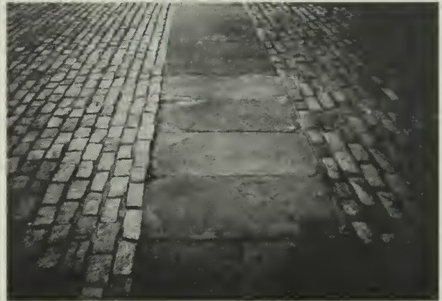
Figure 146: Flagstone panels used in crosswalk, 1997.
