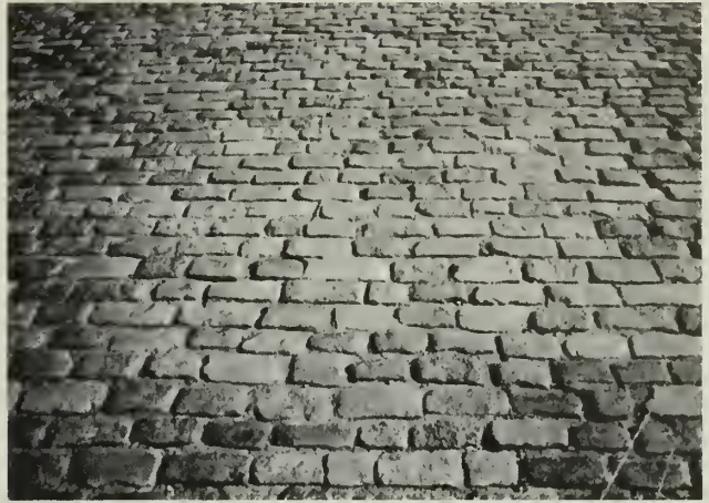
Figure 140: Typical roadbed paving pattern in the park, using Belgian block, 1997.
