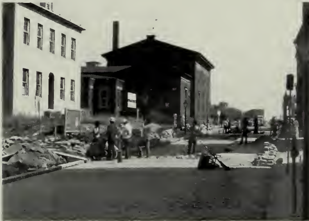
Figure 128: Repaving North Second Street, 1978. A Community Development Block Grant enabled the reinstallation of Belgian block paving on the streets of the Waterfront Historic District between 1975 and 1978.
