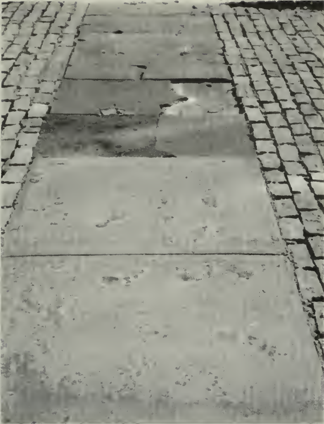
Figure 147: Concrete formed to resemble flagstone paving, 1997.
