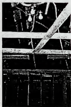
Slave Quarters/Garage, south room, hand-hewn sill on west wall
