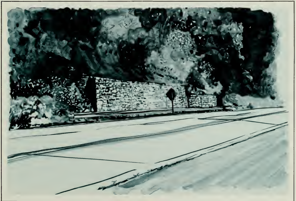
Retaining wall with guide rail near Mt. Union
