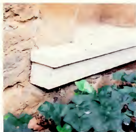
Figure 25. North elevation skirtboard replaced in the 1960s, does not match the original profile as found on the South Dependency.
