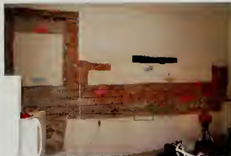
North Dependency, East Room: The location of the lower kitchen's ceiling is preserved as a line of plaster and finishes on the west elevation.
