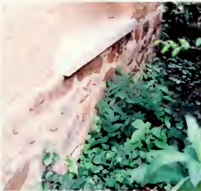
Figure 22. East elevation, vegetation provides a high moisture environment for the wood trim.
