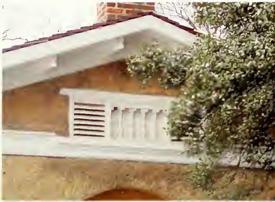
Figure 21. East elevation, horizontal frieze boards running just below the attic vent, balusters and vent elements date to the period of significance.
