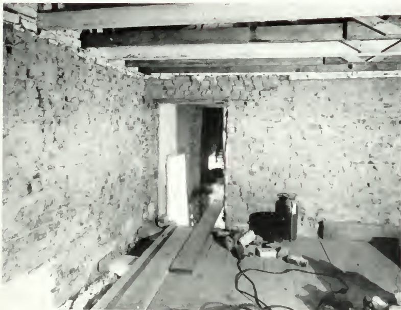
Figure 38. Looking west from east room upper-level into center room through the doorway, 1964 photo showing NPS removal of QMC upper-level floors in progress, and additional joists (those unpainted) inserted between the older joists.
