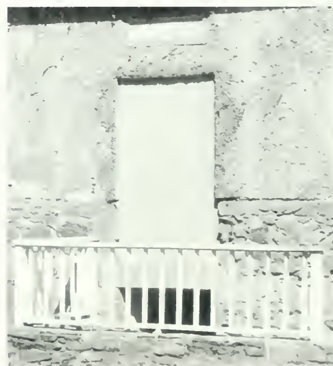
Figure 33. South elevation, closeup of below-grade entrance to summer kitchen and infilled historic door opening following QMC restoration. The upper two feet of the stone foundation wall was exposed and the infilled door area was raised into the area where a cornice had been located historically.
