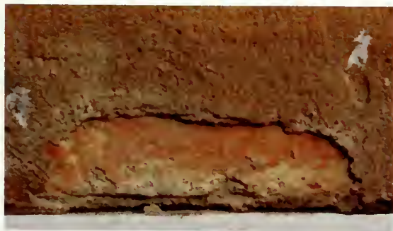
Figure 9: Layers of smooth stucco finish.
