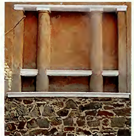
Figure 20. West elevation, ponding water on horizontal trim surface.
