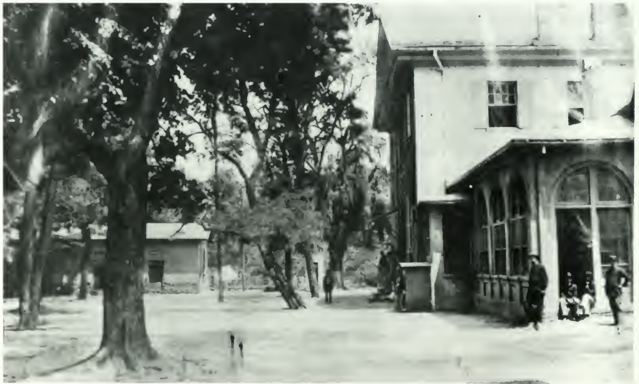
Figure 8. South elevation, 1864 photo by Andrew Russell showing center and east doors of the North Dependency. This image confirms that the door openings were near grade during the Civil War period. Other features seen on this elevation (the rough cast stucco, panel doors, exposed stone foundation, painted panels, and cornices above the door) correspond to the building's current appearance.
