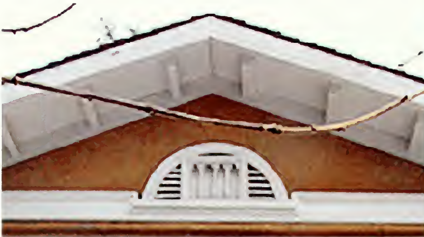
Figure 19. West elevation, fascia board is deteriorated.
