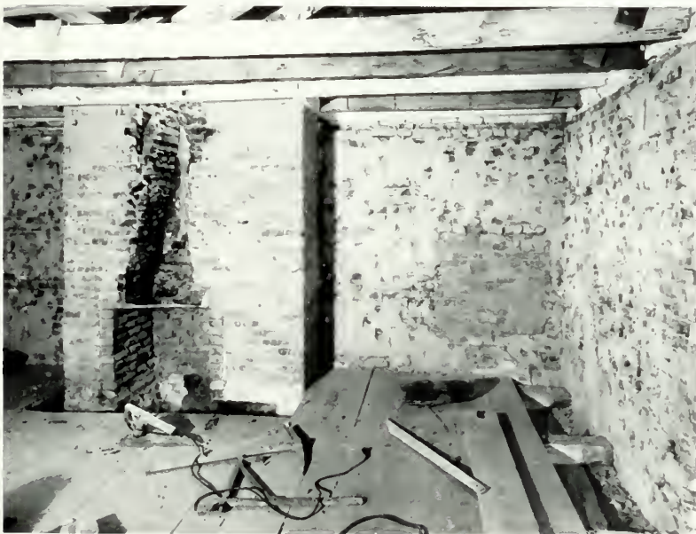
Figure 39. East room upper-level looking east, 1964, showing NPS investigation of fireplace and removal of upper-level floor in progress.
