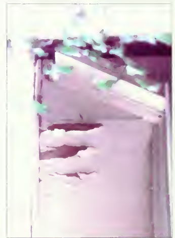
Figure 8: Paint failure and wood rot at NW corner of the eave.
