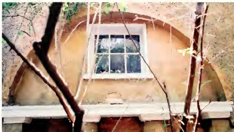
Figure 24. North elevation, many wood elements in the niche (e.g. the column capitals, upper skirt board) were reused from other locations. Early paint layers including a layer of purple were identified in the paint stratification.
