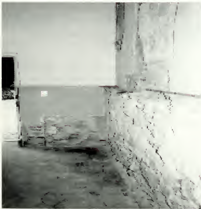
Figure 30. North wall, west end of the center room showing exposed masonry and window hung with the Army's L strap hinges.
