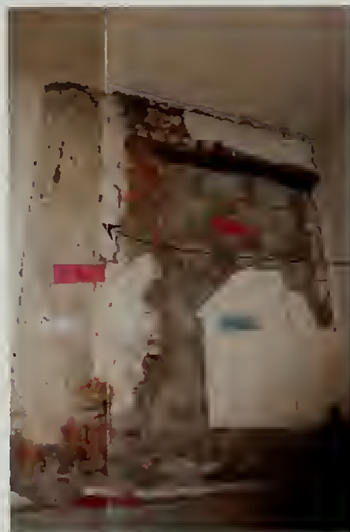
Plank wall location. The wall was installed before the plaster was applied to the walls, and later removed. The patching plaster appears to be a lime-sand mix with a lime wash finish.
