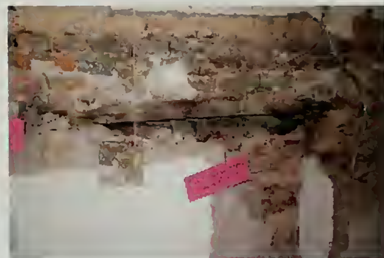
North Dependency, East Room: The location of the lower kitchen's ceiling is preserved as a line of plaster and debris on the north elevation, east window.
