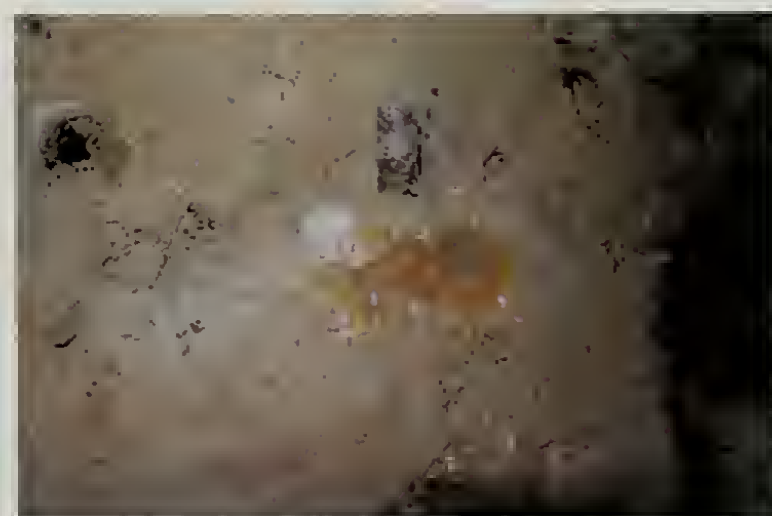
North Dependency, East Room: Small remnants of the plaster finishes survive beneath the later cement plaster. This example was found on the east elevation at the upper room level to the north of the hearth. Its surface area is less than one inch across. The first finish was a brush applied whitewash. The last finish applied to the walls was a yellow distemper paint.
