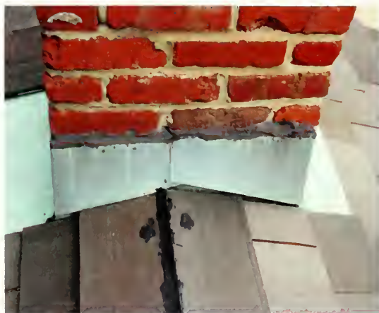
Figure 6: improper installation of flashing.
