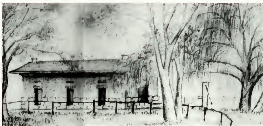
Figure 2. South elevation, A c.1850 drawing that shows three doors at grade, cornices and painted panels above the doors, two chimneys, an exposed masonry foundation bisecting the door openings, and a recessed arched niche on the east elevation. The building probably changed little between its original construction and its appearance in the drawing.
