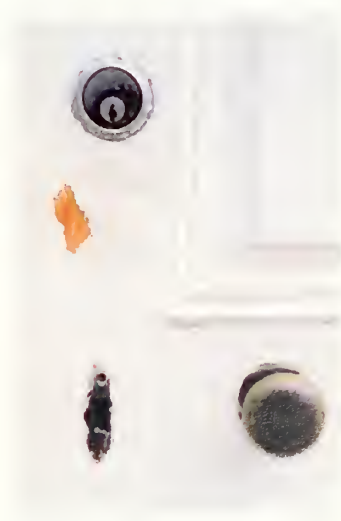
Figure 18. Door hardware needs to be tightened.
