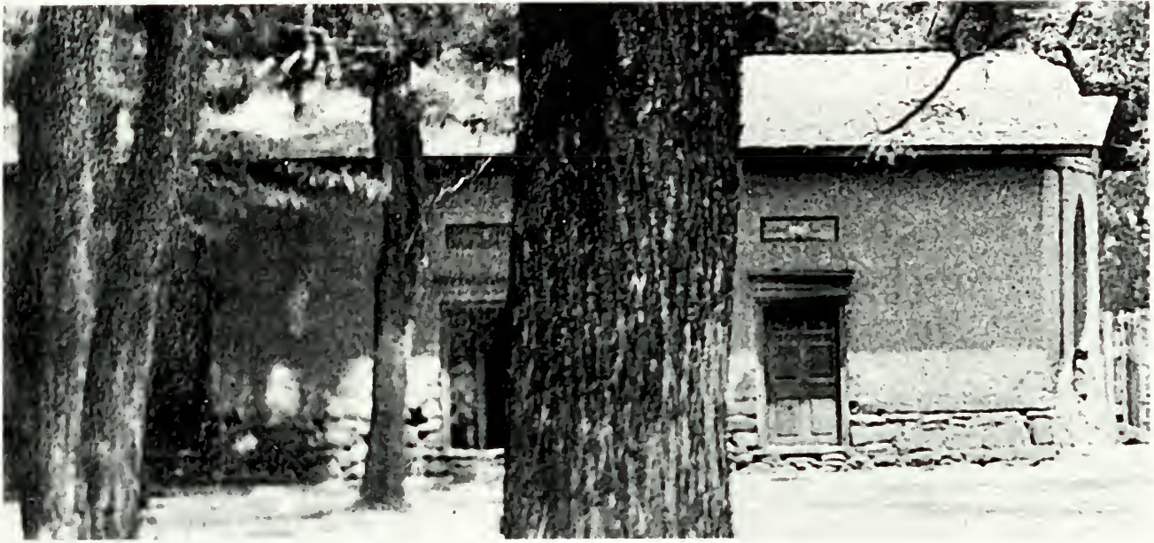
Figure 9. South elevation. Close-up of Andrew Russell photograph, 1864. A light-colored horse or sheep is visible on the painted panel above the east room door. Note that gutters and downspouts were not present on the building at this time. Also note the missing skirt board in the lower portion of the east elevation arch.
