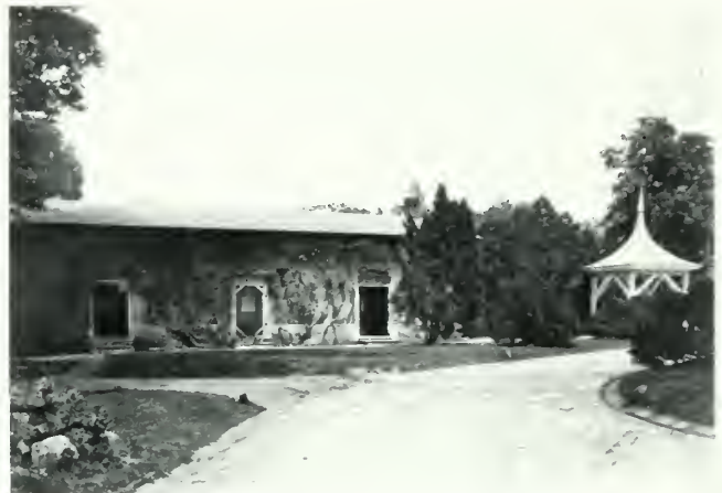
Figures 25 and 26. Photographs of south elevation, circa 1900. The photos show the replacement doors and the foundation with its stucco finish (in the 1860s the foundation was exposed masonry). More importantly, the open door to the east room reveals an exposed shoulder where the original upper-level floor joists once sat. This is consistent with the space being used after the Civil War as a single-level open room with a floor at-grade.
