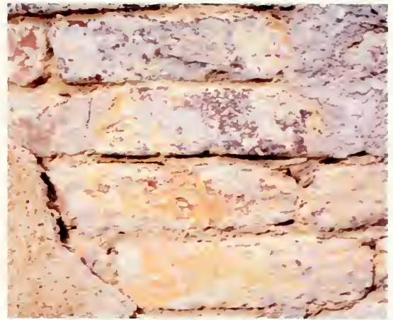
Figure 5: Paint on brick gave the building a more finished appearance in the early years before stucco had been applied to certain wall sections.
