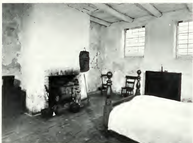
Figure 34 (top left). East room lower-level, 1959 photo showing conditions after 1930 QMC restoration of summer kitchen. Note reconstructed fireplace and exposed joists for upper-level floor
