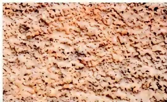
Figure 11. Rough cast finish, closeup showing a render of the aggregate mixed into the matrix.
