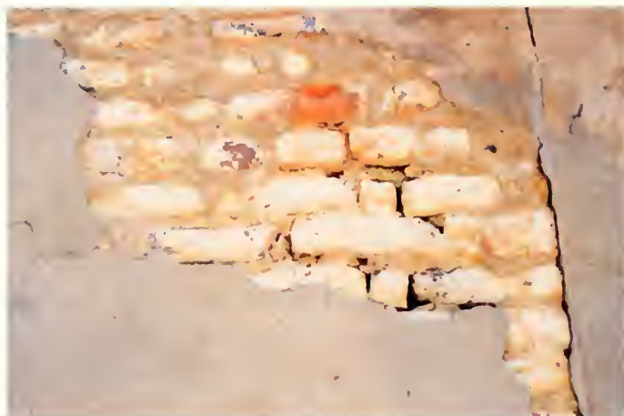
Figure 4. North elevation, 2003, showing painted brick beneath later smooth stucco finish in the recessed arch.
