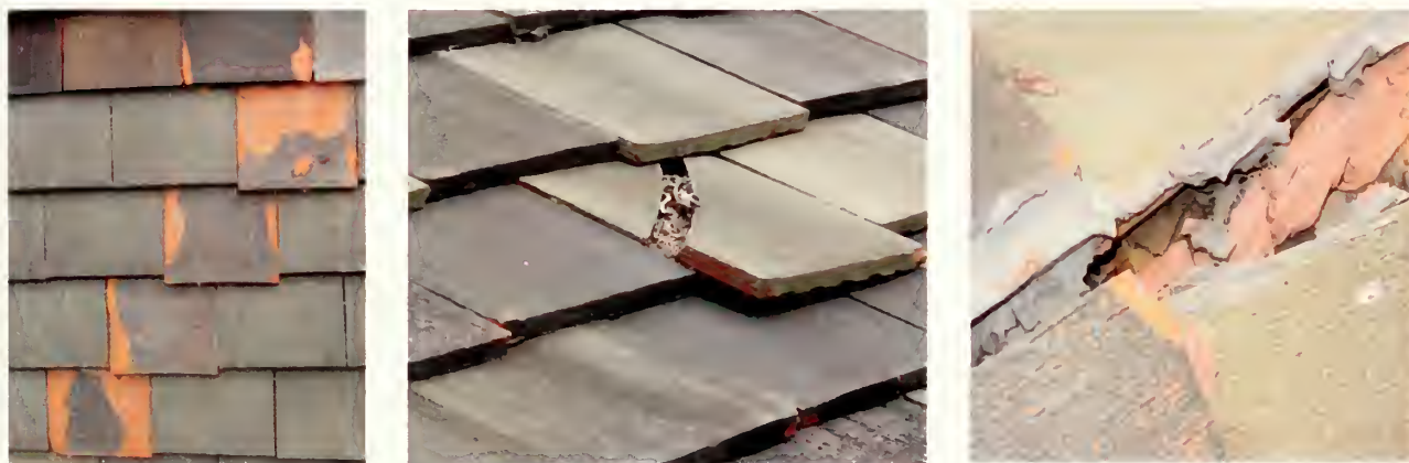
Figure 7: Delamination, chipping, crazing, and structural failure of tile shingles
