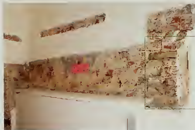
North Dependency, East Room: The location of the upper room's floor level is preserved as a line of plaster and finishes on the south elevation.
