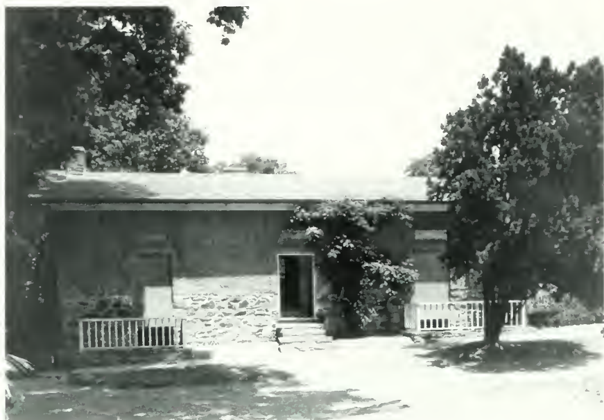
Figure 32. South elevation, 1933 photo. Shows building after QMC restoration. Changes include insertion of a reproduction vestibule partition in the center room; infill of the east and west room historic door openings; the shift upward of all three door openings (obliterating the door cornices) in order to accommodate the two below-grade entrances to the end rooms; and removal of approximately 2' wide band of rough cast finish to align it with the midpoint of the raised door openings.
