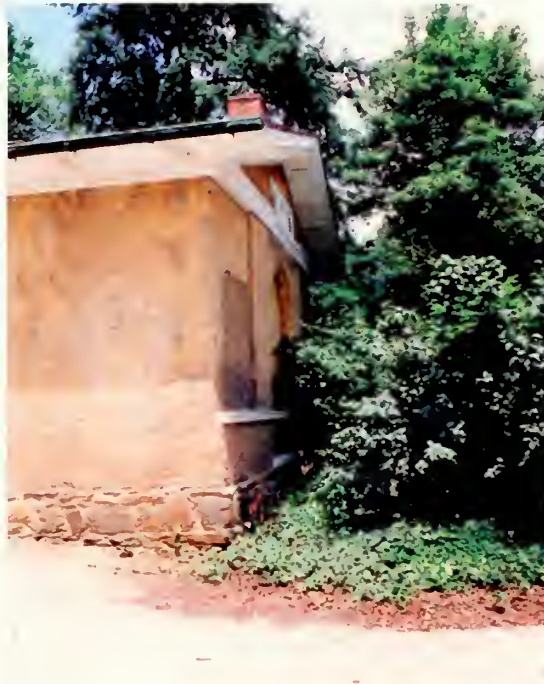
Figure 3. Vegetation on east elevation contributing to the buildings moisture problem.
