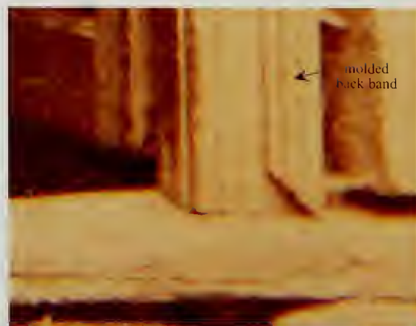
North Dependency, detail of 1865 photograph of molded back band
