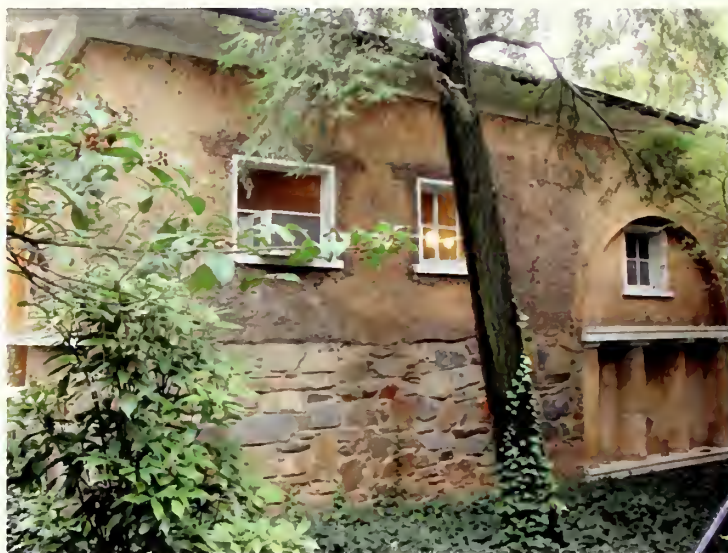
Figure 3. North elevation, 2003. Grade changes and window infill help conceal the historic two-story appearance of the facade.
