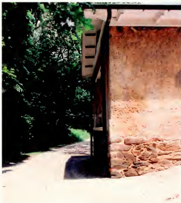
Figure 2. Road along west elevation where vehicular traffic splashes water onto the masonry wall and damages historic masonry and finishes.
