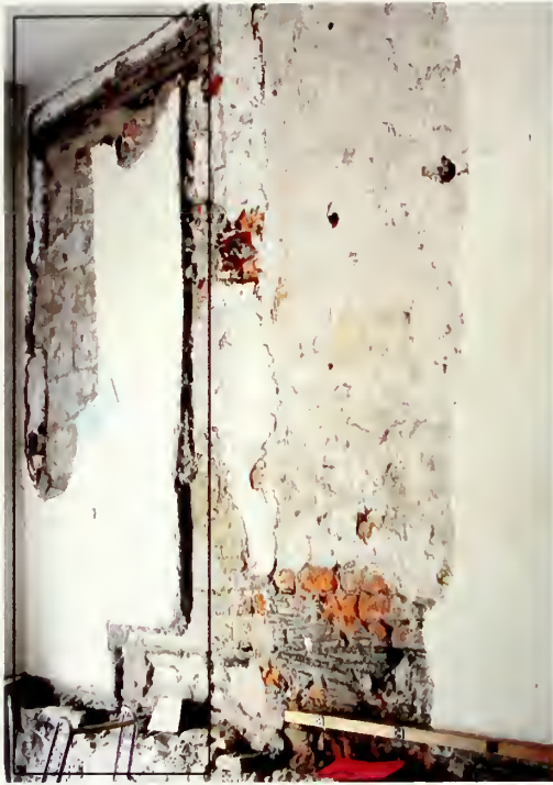
Figure 7. Center room, south corner of west wall, 2003, shows the infilled original door set between a wood lintel above and the masonry shoulder below. This door led to the upper floor of the west room. NPS plaster and concrete block from 1964 conceal much of the historic opening. The partition dividing the forward vestibule and the rear living space ran perpendicular to this wall joining it near the center of the image (to the right of the door).
