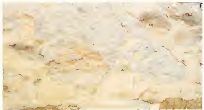
Figure 4. Numerous areas of paint on the stone foundation may be evidence of an early coatings treatment.
