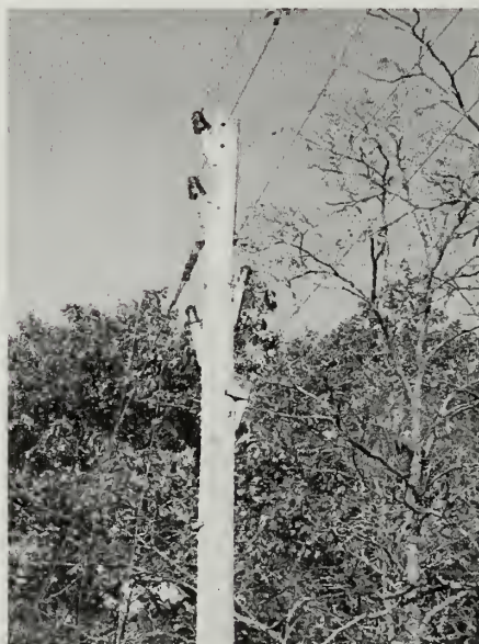
Figure 64 . U.S.C.G. utility pole and lines with glass insulators attached directly to the pole, 2004. (OCLP)
