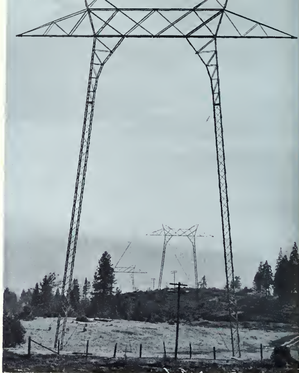
Guyed towers of P.G. & E.'s 500-kv a-c system are already in place near Round Mountain, Calif.—a segment of the Pacific Northwest-Pacific Southwest Intertie. (P.G. & E. photo).
