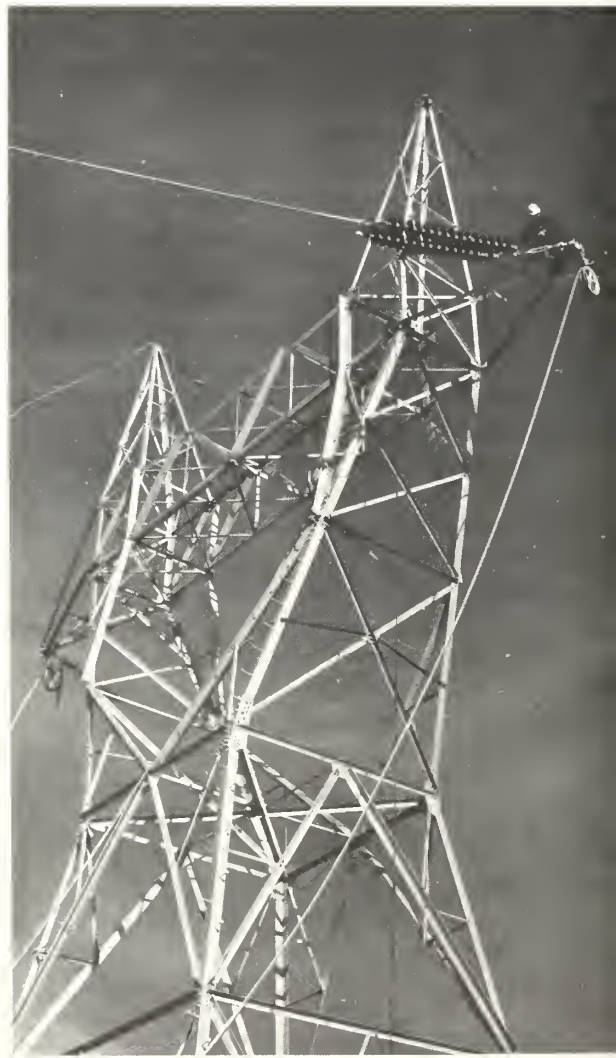
A FINISHING TOUCH ON A CONVENTIONAL TOWER —A lineman perches on a high beam and attaches an insulator assembly. This conventional structure was raised by the crane in another part of the transmission line spanning the 182 miles from Glen Canyon Powerplant in Arizona, to Shiprock, N. Mex.
