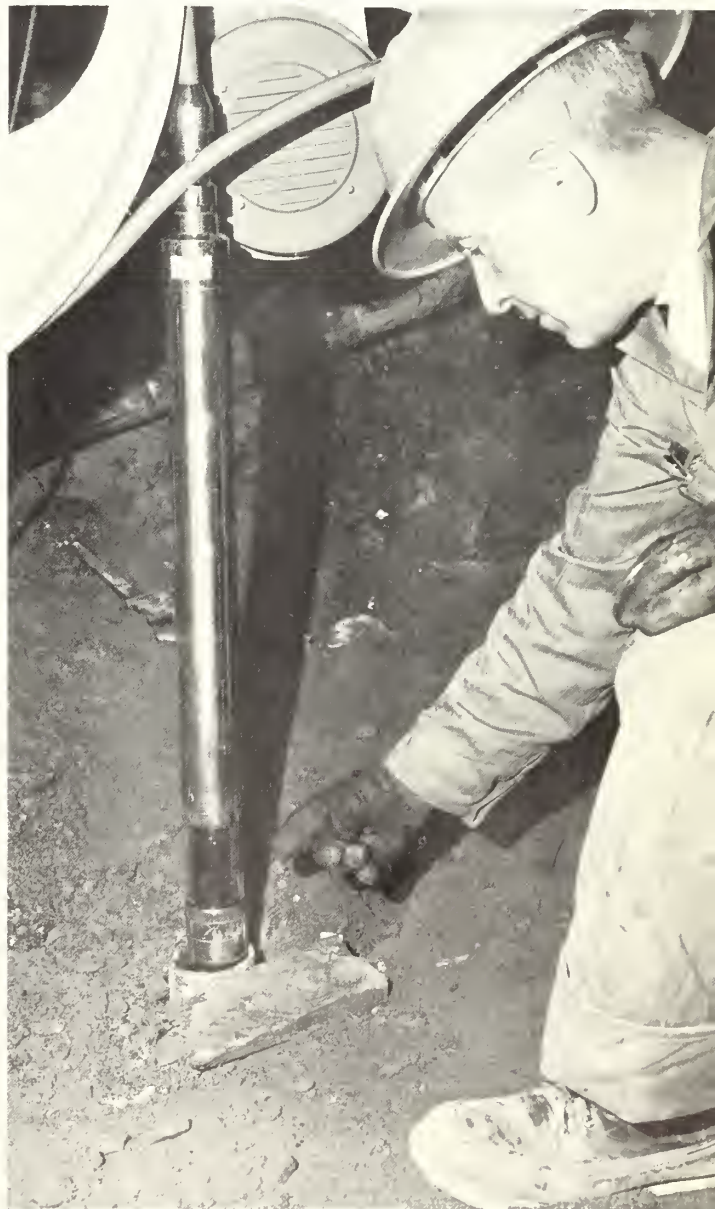
Pointing to the probe of the TV borehole telescope as it is entering a 3-inch borehole is, Roxy Root, geologist.
