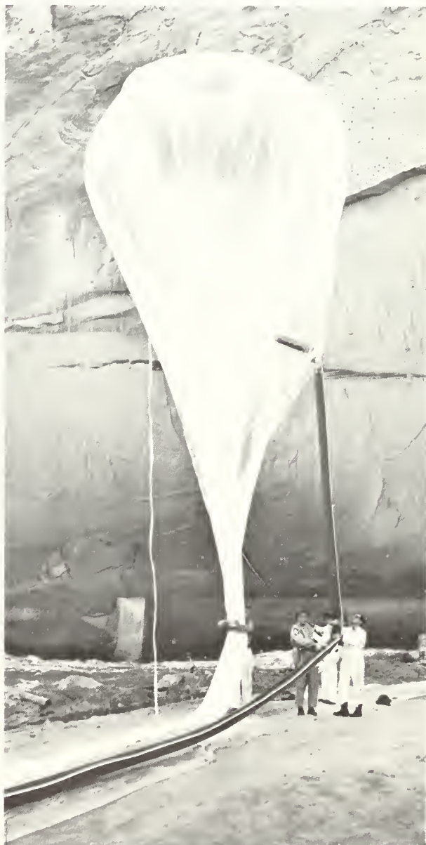
Large tube attached to the side of the balloon carries helium to inflate the balloon.
