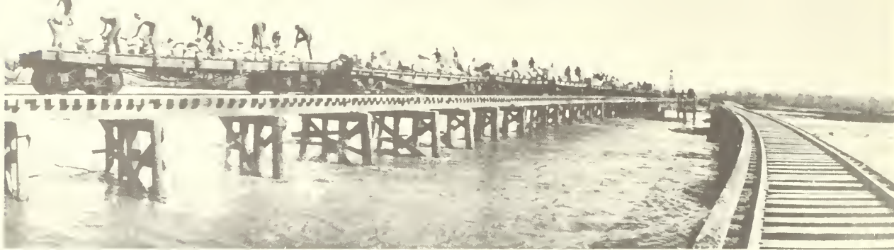
Crewmen tumbled rocks off flat cars to dam the rampaging waters. (Southern Pacific photo)
