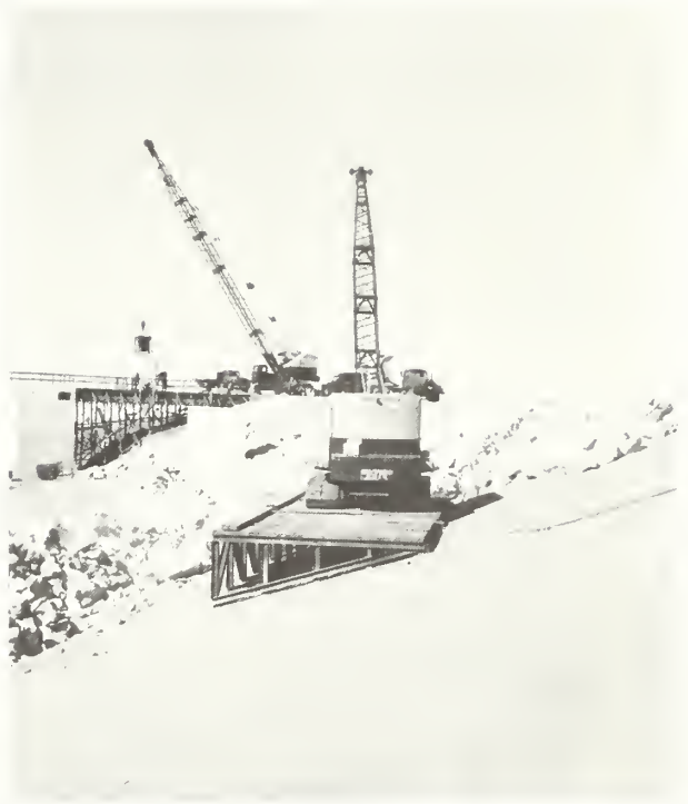
Work on the Amarillo Regulating Reservoir, also on the Canadian River Project, shows the crane in the foreground, the bulldozer below, and the man near the top of the slope all helping to place riprap (large boulder-rock) on the dike slope. The crane in the background is placing concrete on the walkway for the inlet structure.
