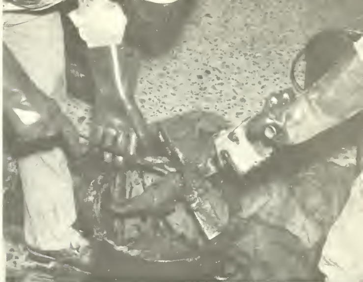
Workmen wear rubber gloves and remove epoxy mortar from paddle with spatula.
