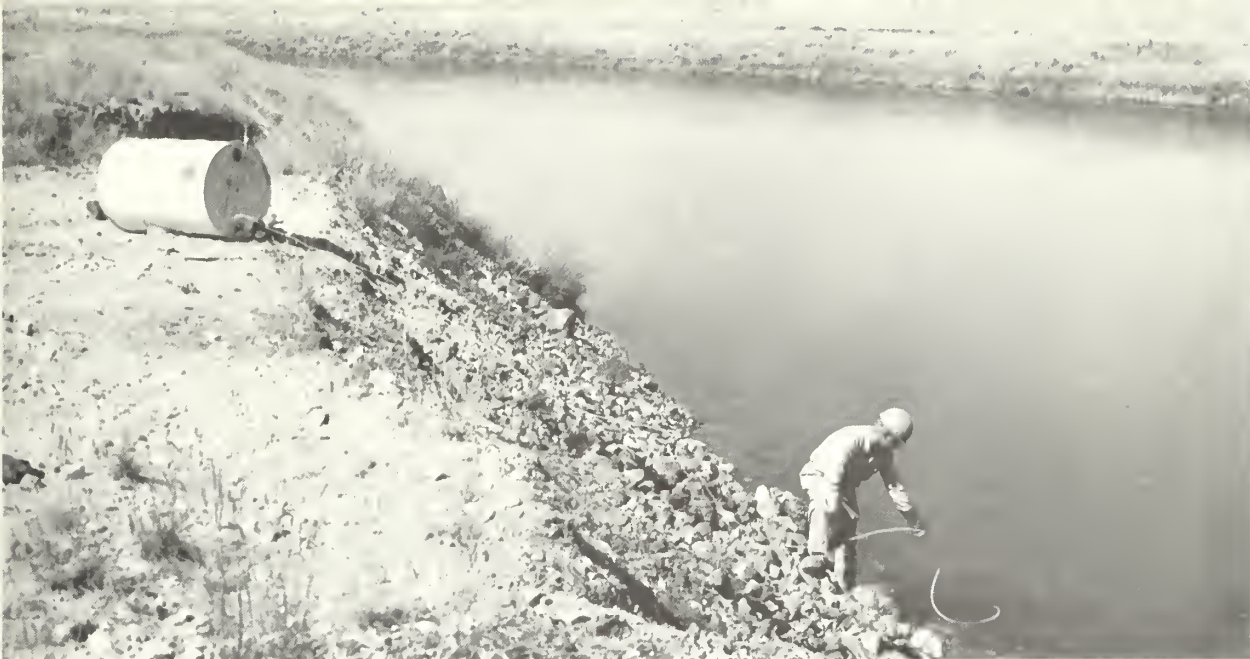
Figure 1.—Chemical is fed into a project canal by Adam Focht, Assistant Watermaster. Concentrations as low as one part Aerolein to ten million parts water were successful.
