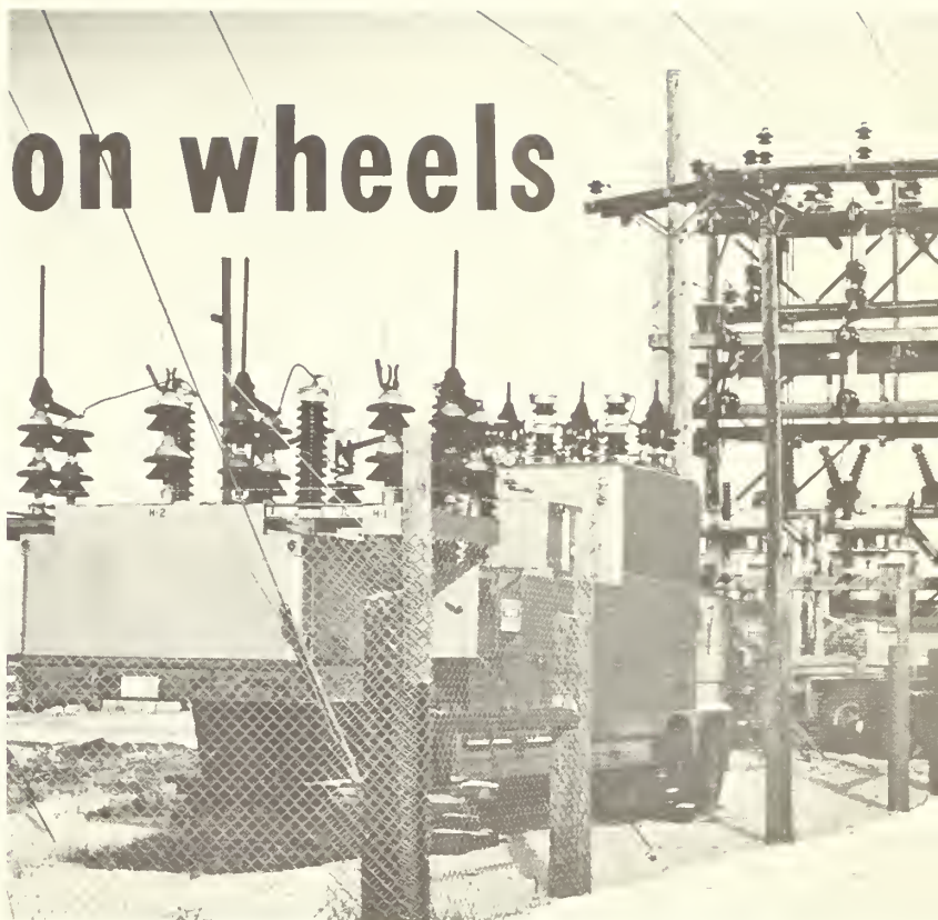
This mobile substation was put to use in the enclosure of the Whately Substation, Fort Peck, Mont.
