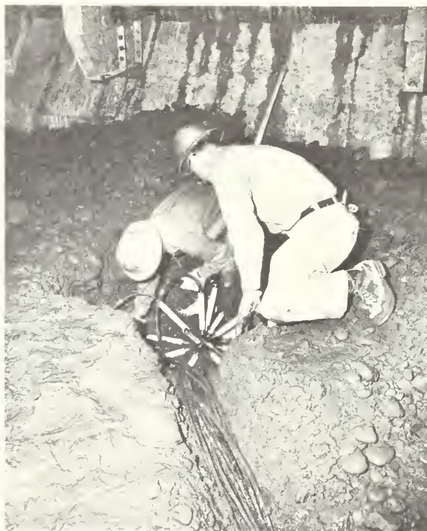
Concrete is freshly poured, strainmeters and their cables are placed by hand—this is early in the construction of Glen Canyon Dam.
