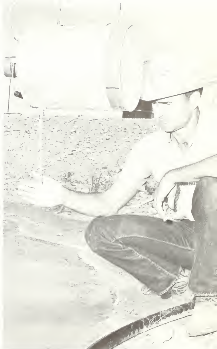
This specialist is checking the operation of the dispenser can, which is the constant pressure type, another variety used in experimental retardation tests.
