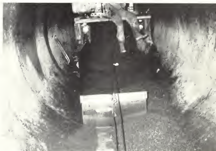
A special power scraper (at top of photo) was devised to go in Eklutna Tunnel and clean out the sandy muck.
