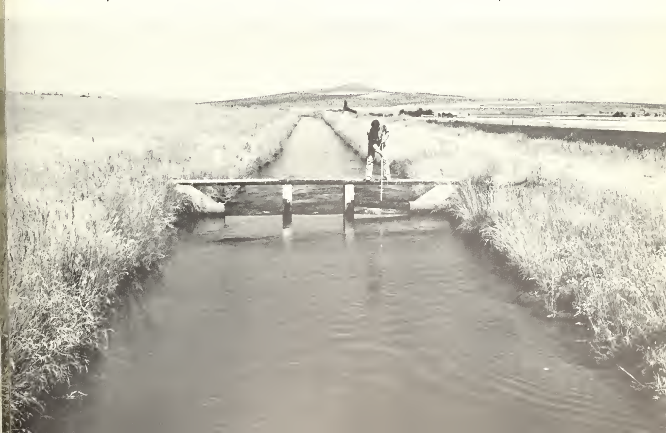
Checkboards are pulled from a check structure to maintain a constant water surface elevation in a major Deschutes lateral.
