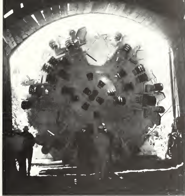
The giant tunneling "Mole" looms into the portal to take over its work on the already started Tunnel No. 1 of the water development project.
