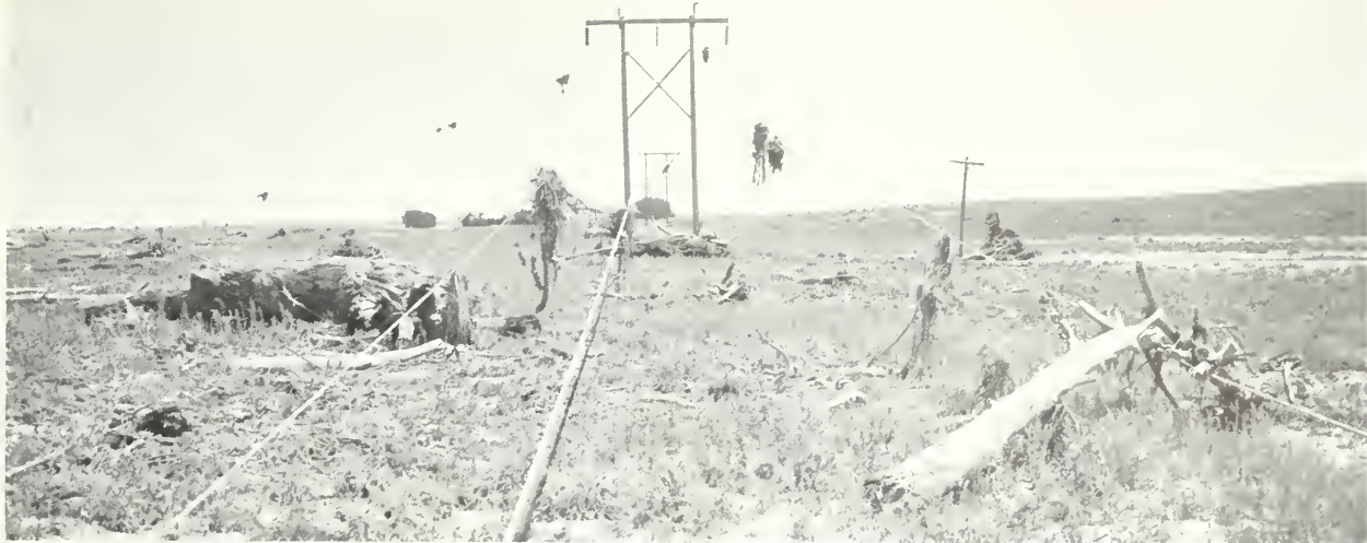
Five-foot-deep floodwaters passed through this area on the Colorado-Big Thompson Project, Colo. Several emergency outages of electric power and widespread and costly damage resulted in several areas. One of the hazards was flood debris and trash, such as is shown here.
