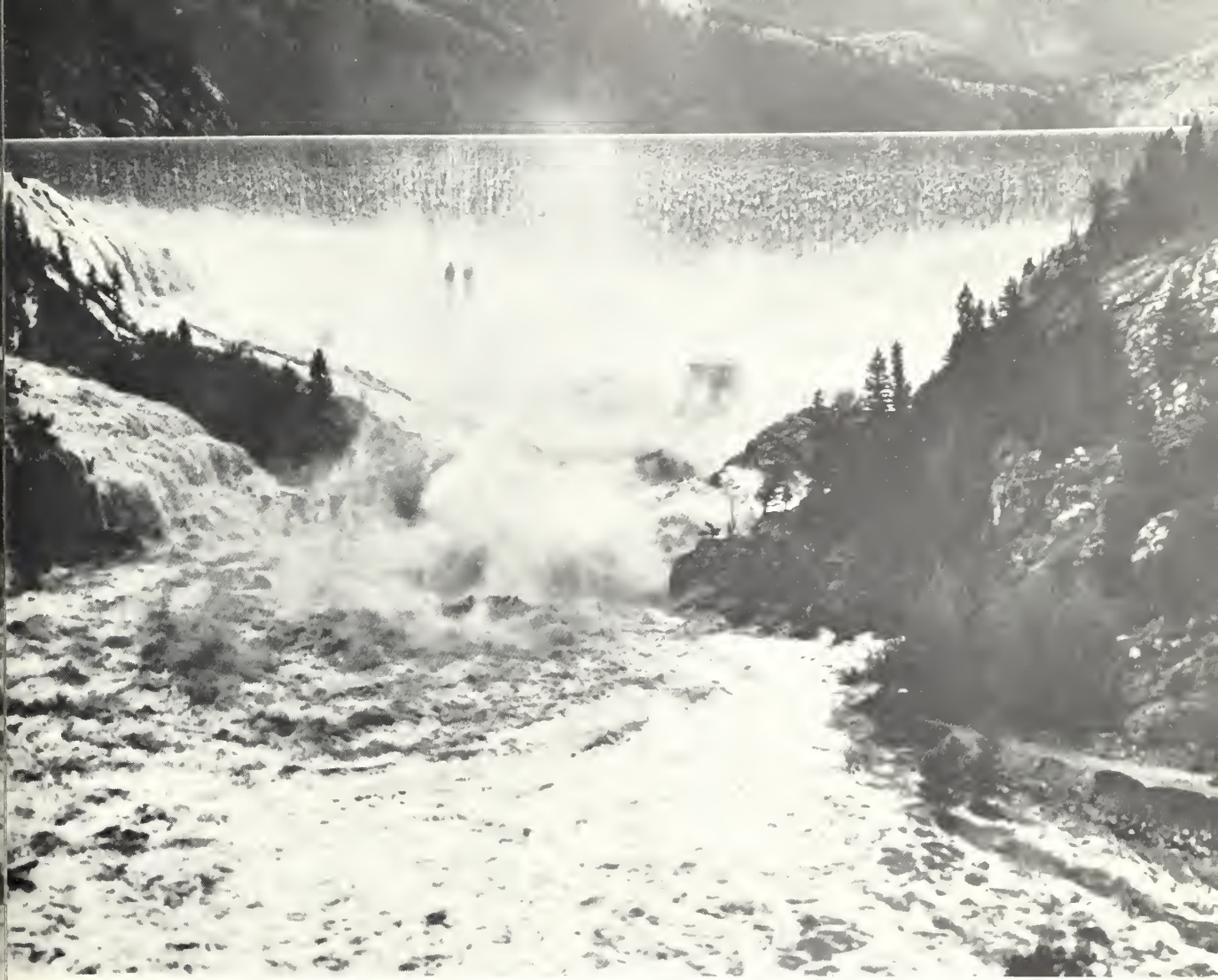
Though not designed to pass water over the top as do some dams, Gibson Dam is shown with more than a foot of treacherous flood waters tumbling over its concrete rim. Coming around both ends of the dam, the flood washed soil and loose stones down to bedrock. The dam was constructed primarily for storage of Sun River waters, but with a structural safety bonus for such emergency situations. (Photo taken on June 9, 1964, by George F. Roskie, U.S. Forest Service.)
