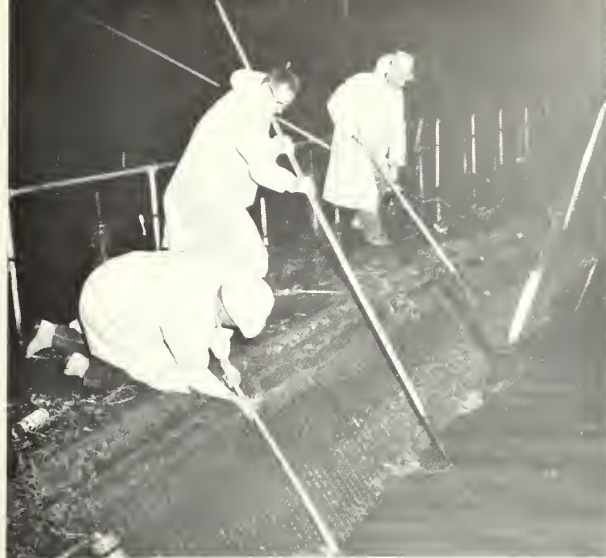
A night trouble crew works on the walkway above the steel guard, raking out objects which would impede the flow of the heavy murky waters.
