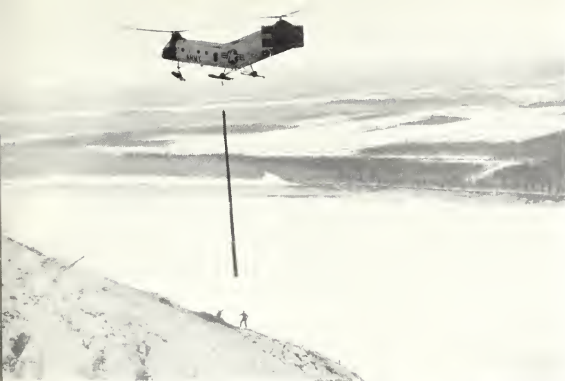
Army helicopter assisting in setting poles on Eklutna-Palmer 115,000-volt line.
