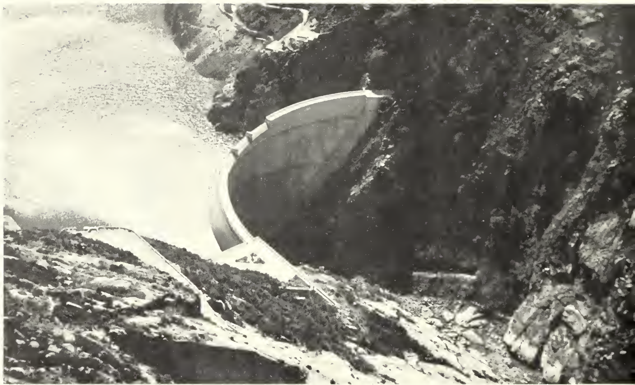
Spain's double curvature, thin, concrete-arch Eume Dam has an overflow spillway.
