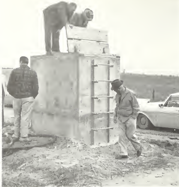
A newly constructed wasteway box on a lateral in the Boise Project area also is inspected.
