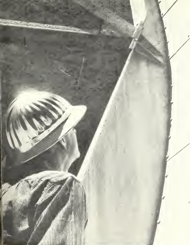
Large radial gates, which control the flow of water over the spillway of a dam, are periodically inspected.
