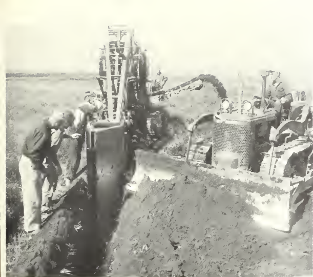
The Buckeye trencher machine at left has "dug in" to a trench depth of about 10 feet for a cutoff, curtain-laying trial on the Columbia Basin project.
