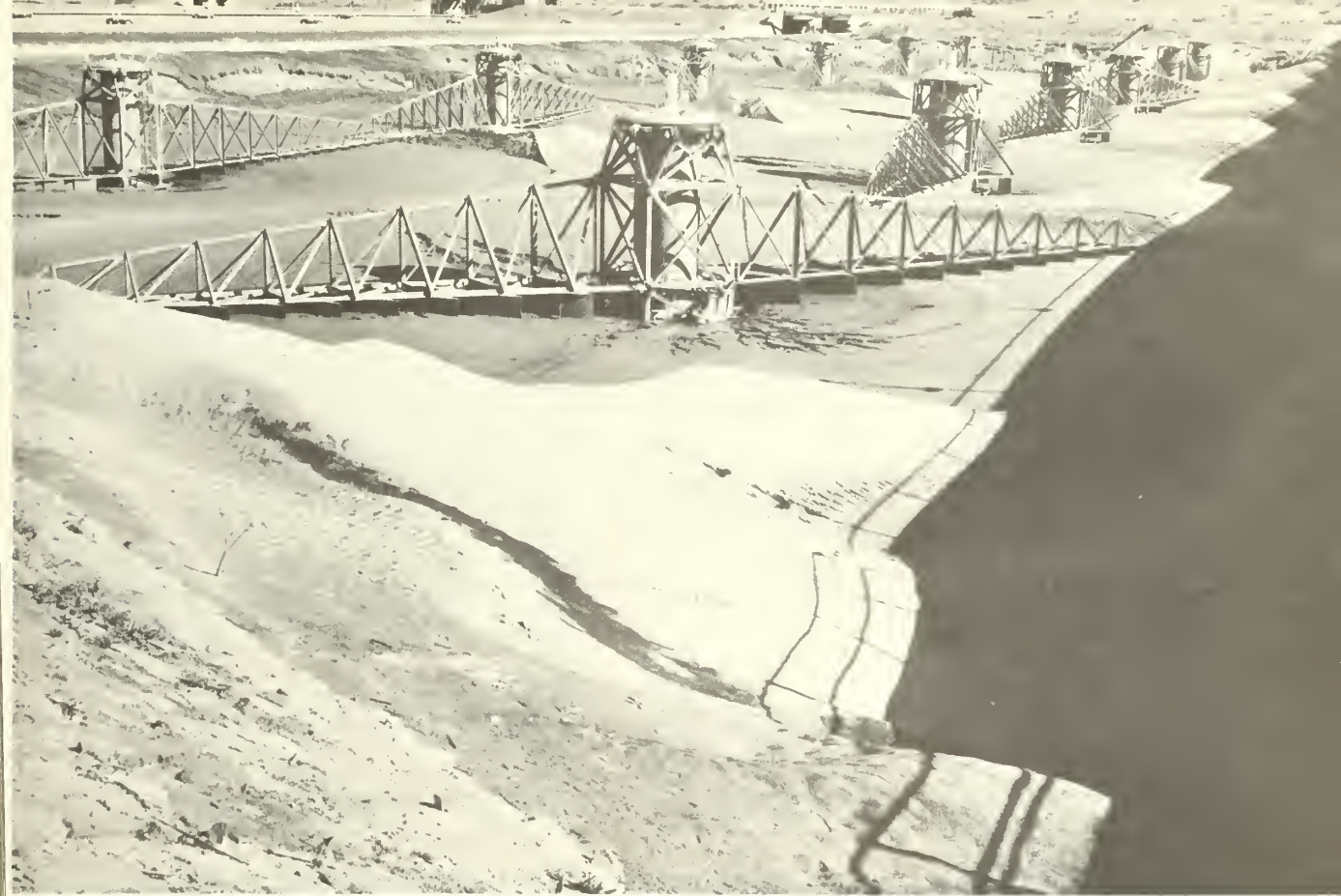
When operating, the water level comes to the top of this desilting equipment located near Imperial Dam on the Colorado River. Clear water is moved to irrigate fields while the silt is returned to the river.
