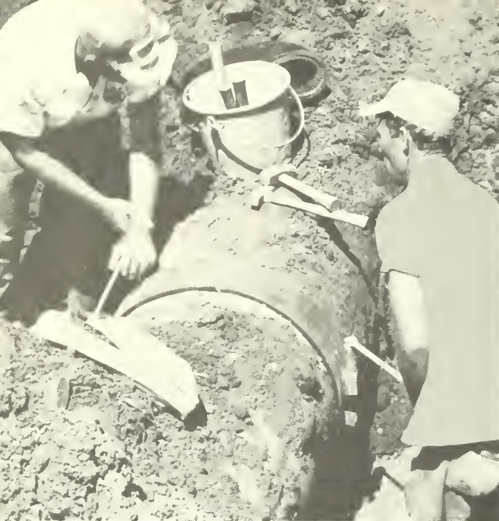
An inservice leaking pipe is repaired with rubber liner, metal band and mortar.
