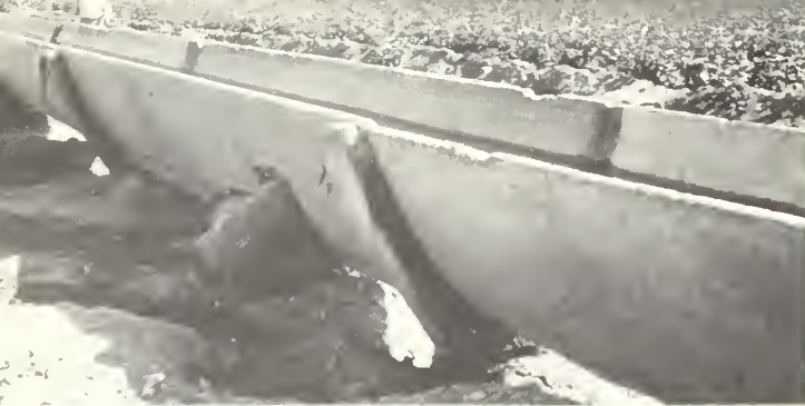
U.S. irrigation specialists queried Soviet officials about their wide use of concrete flumes as shown here rather than going to buried concrete pipe.
