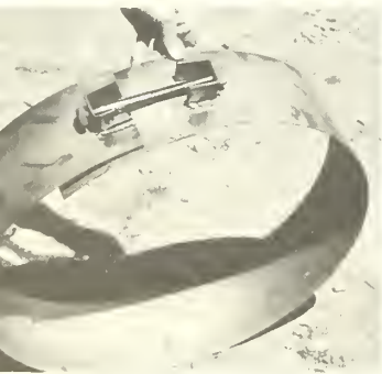
An inservice leaking pipe is repaired with rubber liner, metal band and mortar.
