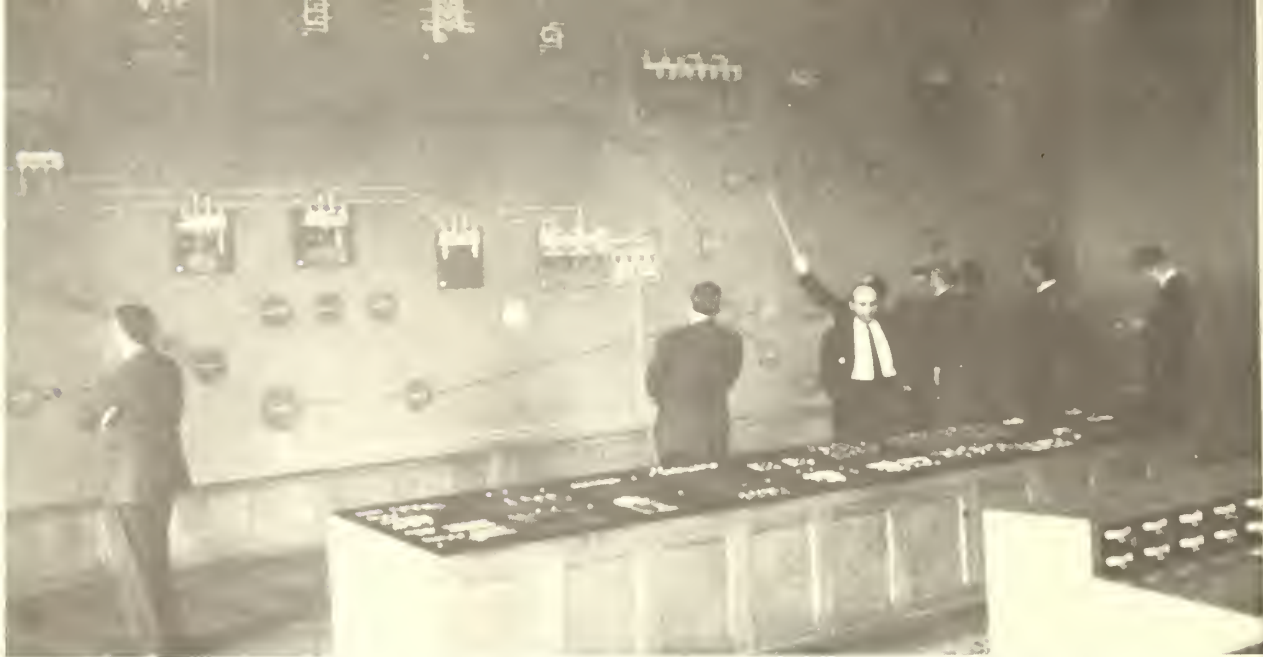
Central Dispatching Center in Moscow is being observed by members of Secretary Udall's group. Practically all of European Russia's power, 30 million kilowatts, is under unified control and is dispatched here.
