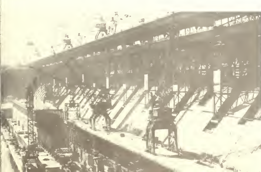
Construction underway on the downstream face of Bratsk Dam.
