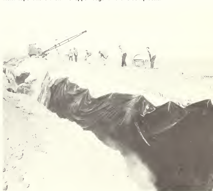
Test curtain installation at the East Low Canal area shows filament tape anchors on the upper edge of the black plastic.
