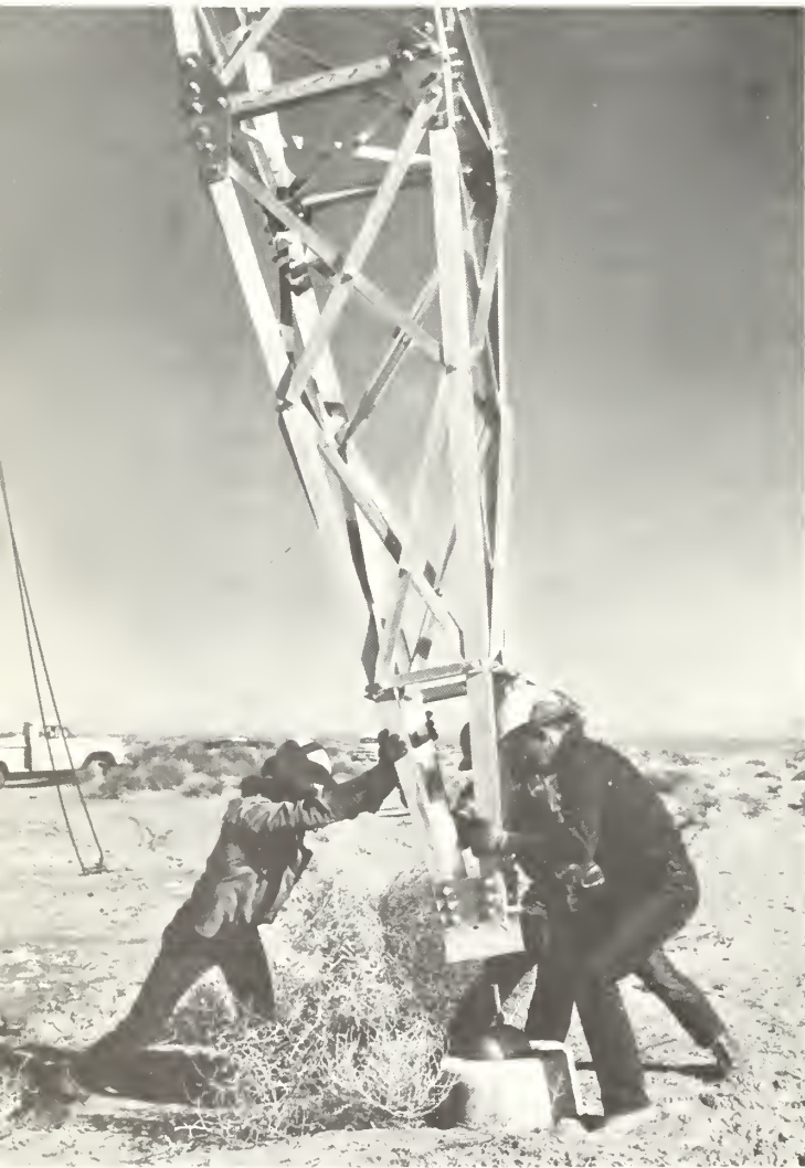
RAISED BY CRANE —Three linemen guide the leg of an aluminum H-frame structure onto a foundation ball. It is part of the test section of towers described in the story, but the leg was raised by the crane shown in other photos.
