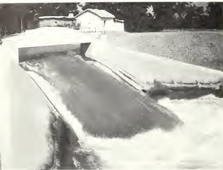
A Grand Fergana canal high velocity check and drop structure in operation.
