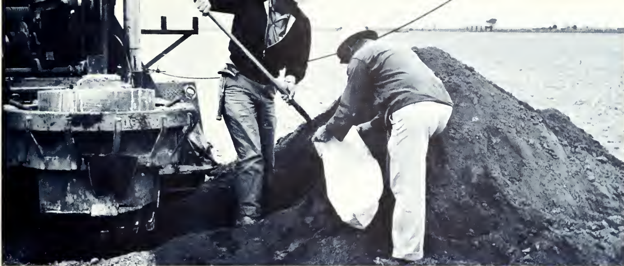
Initial drilling, sampling, and testing of foundation conditions for steel tower transmission lines and substations. Geologists are taking a sample of materials removed from the hole with a bucket auger.
