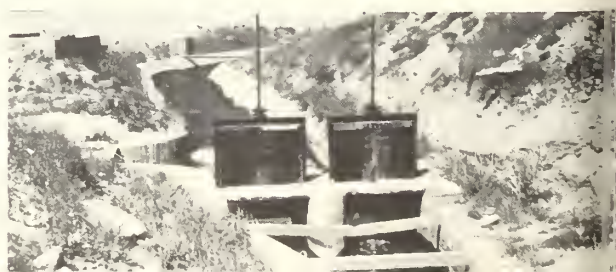
This small canal brings water to the vertical intake to a siphon in the right foreground.
