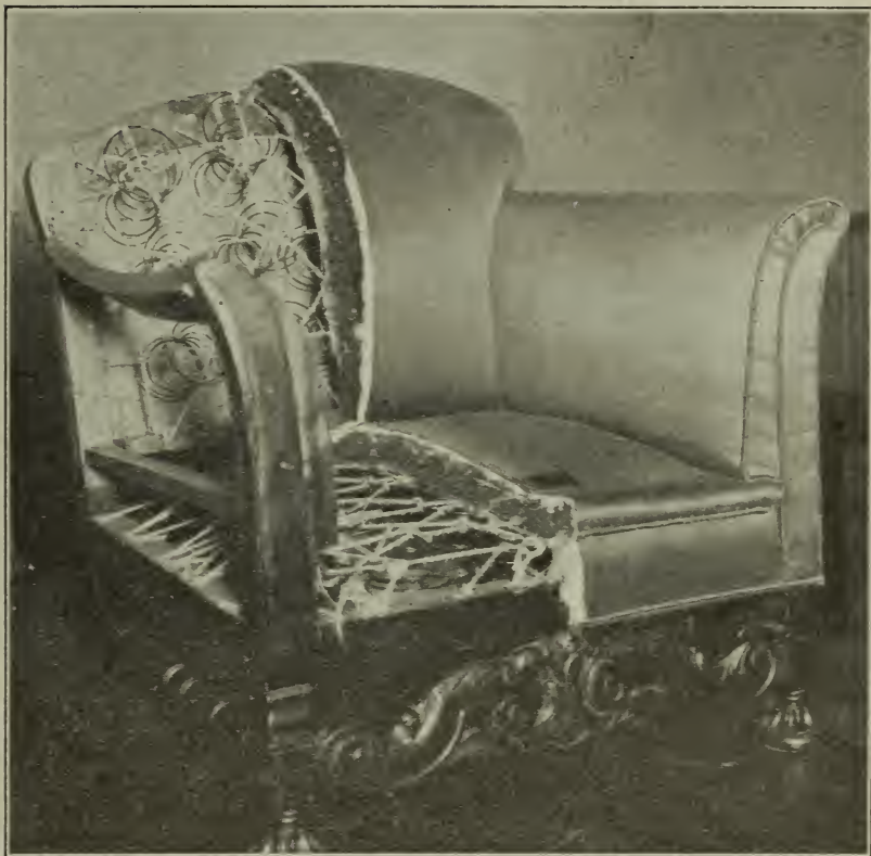
FIGURE 17.—Type of construction which will assist in preventing injury to furniture resulting from feeding of moths from beneath the cover. Observe that the chair has been formed with a stout cotton cover over which the outer cover will be applied; observe also the use of cotton batting at the front and everywhere beneath the cotton or inner cover. Although moths might get into the spaces about the springs and from there pass through the burlap covering them, into the moss or hair, they can not eat their way through the unbroken layers of cotton batting
