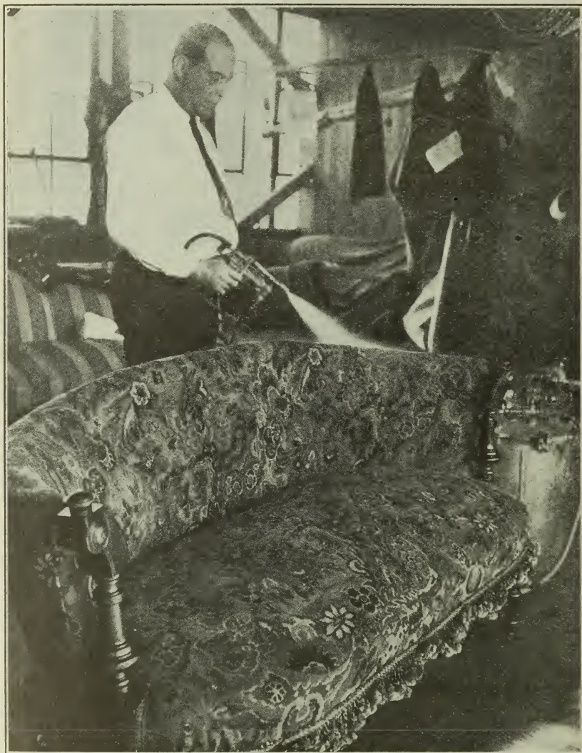
FIGURE 35.—Man applying under air pressure an aqueous fluoride solution to a couch covered with wool tapestry. The couch was fumigated before the solution was applied
