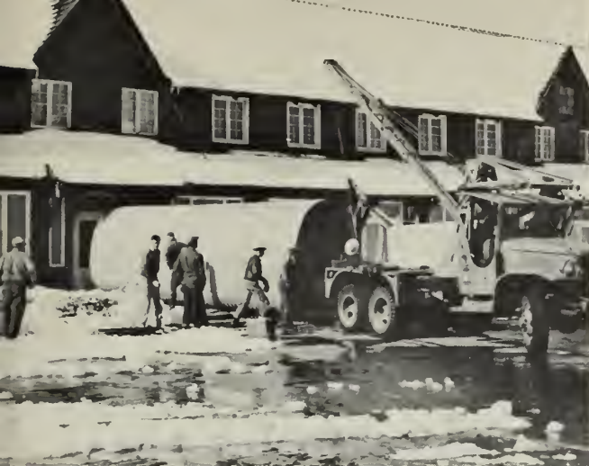
A multi-plate steel snow tunnel leading to the entrance is being erected. (Photograph by Bender.)
