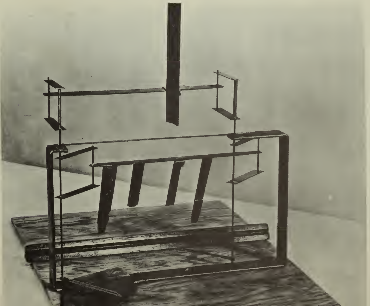
Reproduction of lift balance used in 1901 wind tunnel; model airfoil in testing position. The original balance is in the Franklin Institute.
