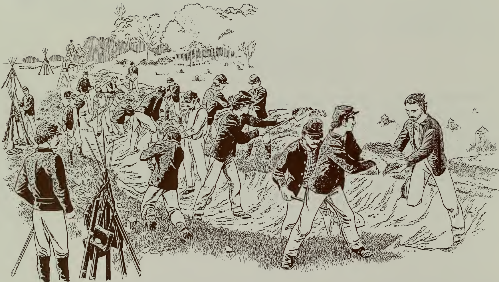
Union General Philip Sheridan's men constructing a 2-mile line of large earthwork defenses connecting six artillery redoubts along the crest of Bolivar Heights in 1864.
