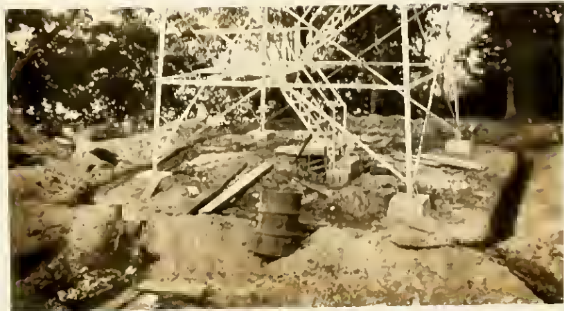
Barnett Knob look-out, showing trenches for laying copper wire for lightning protection.
