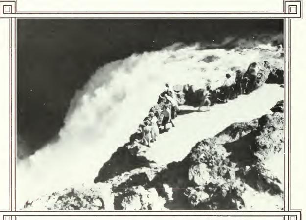
In keeping with the 1930s master plans for the Grand Canyon of the Yellowstone, the wooden overlooks constructed about 1920 were rebuilt with flagstone terraces and naturalistic stonemasonry guardrail shaped to blend with the irregular, curvilinear contours of the natural cliffs. Viewed from a distance the manmade walls were indistinguishable from the walls of the natural gorge. (National Park Service Historic Photography Collection)
