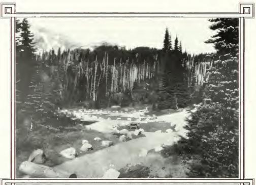
The Paradise Camp Grounds at Mount Rainier were reconstructed in the early 1930s according to E. P. Meinecke's principles of camp planning and landscape protection. Parking spurs were laid out on one-way roads and marked with boulders and log barriers. Each campsite was equipped with a table, fireplace, and tent clearing. (National Archives, Record Group 79)
